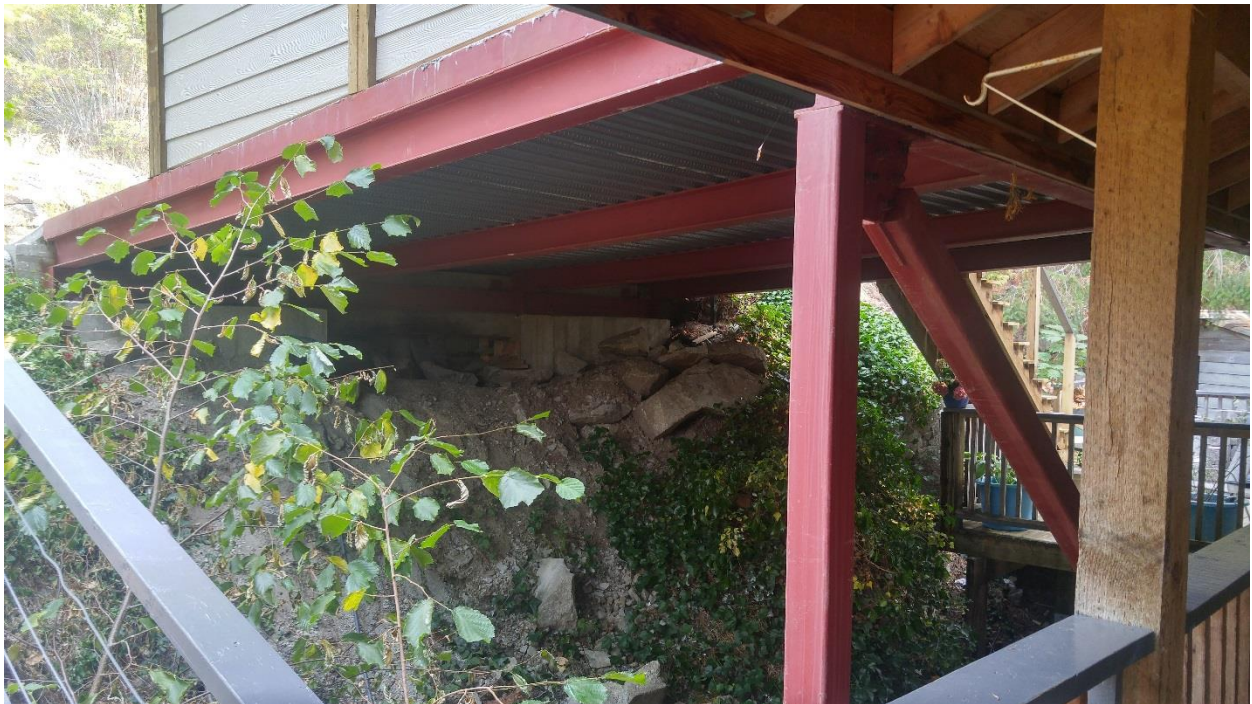
Figure 2 - Support structure for parking platform. (Note steepness of property)
