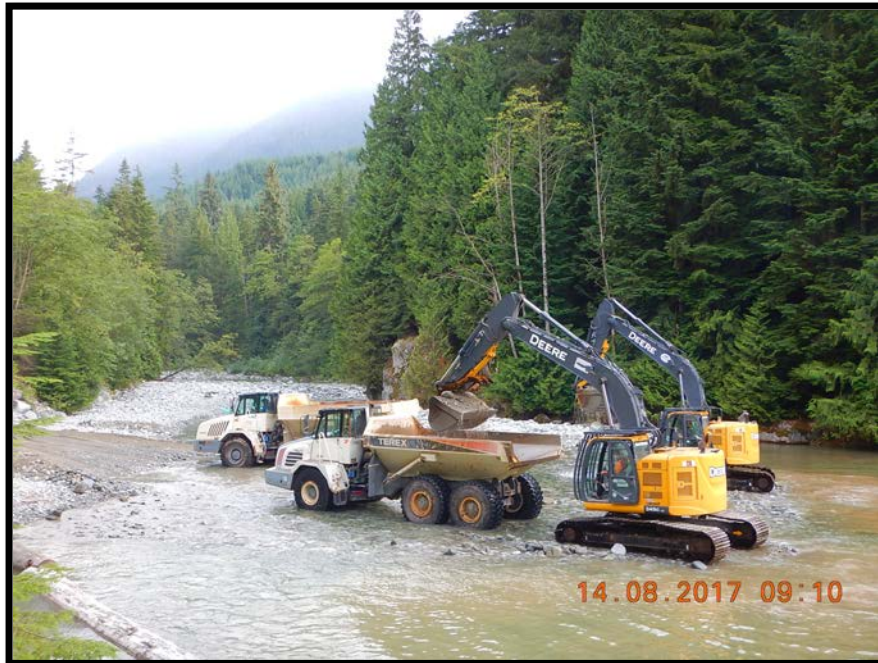
Photo 4: A sediment plume released during the removal of the headpond sediment wedge. Turbidity was monitored constantly below the work site and work was stopped when turbidity exceeded 8 NTU.
