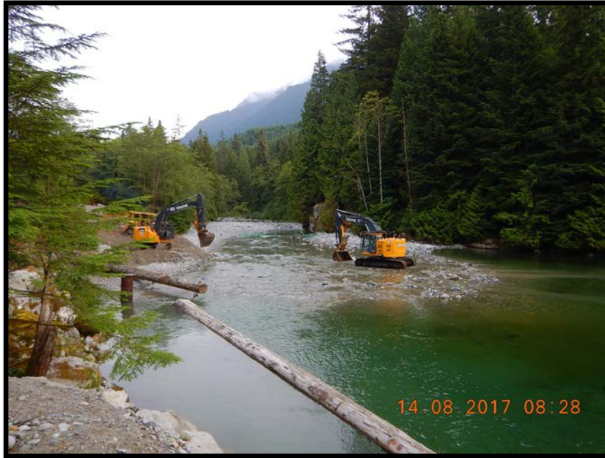
Photo 3: Excavators worked from within the wetted stream channel on top of the sediment wedge. The wedge was excavated in an upstream direction with bailed materials being end hauled to the spoil site 100-m away.
