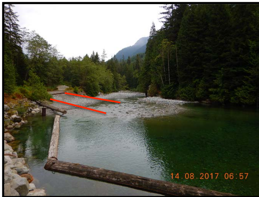
Photo 2: The HSPP headpond on the Rainy River, Howe Sound. The location of the access ford across the stream is shown with red lines. The approximate area to be excavated is highlighted. The work required river crossings throughout the day. Turbidity was monitored downstream.
