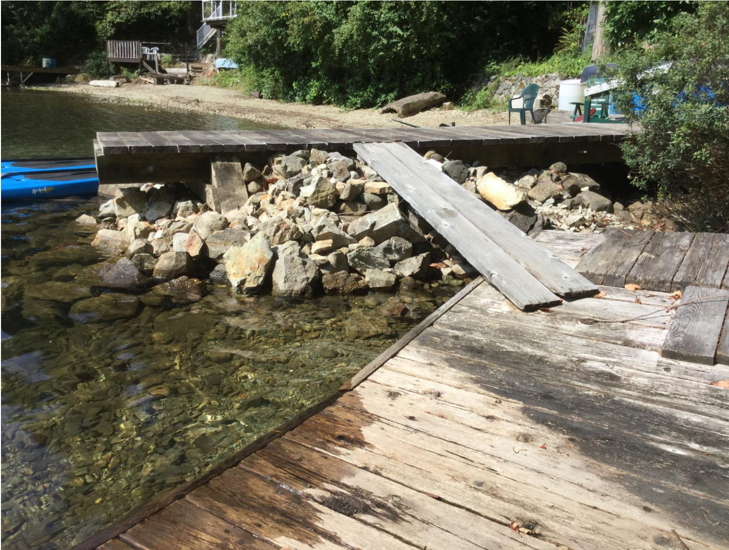
Figure 3 - Existing pier located on rock fill with damaged dock in foreground.
