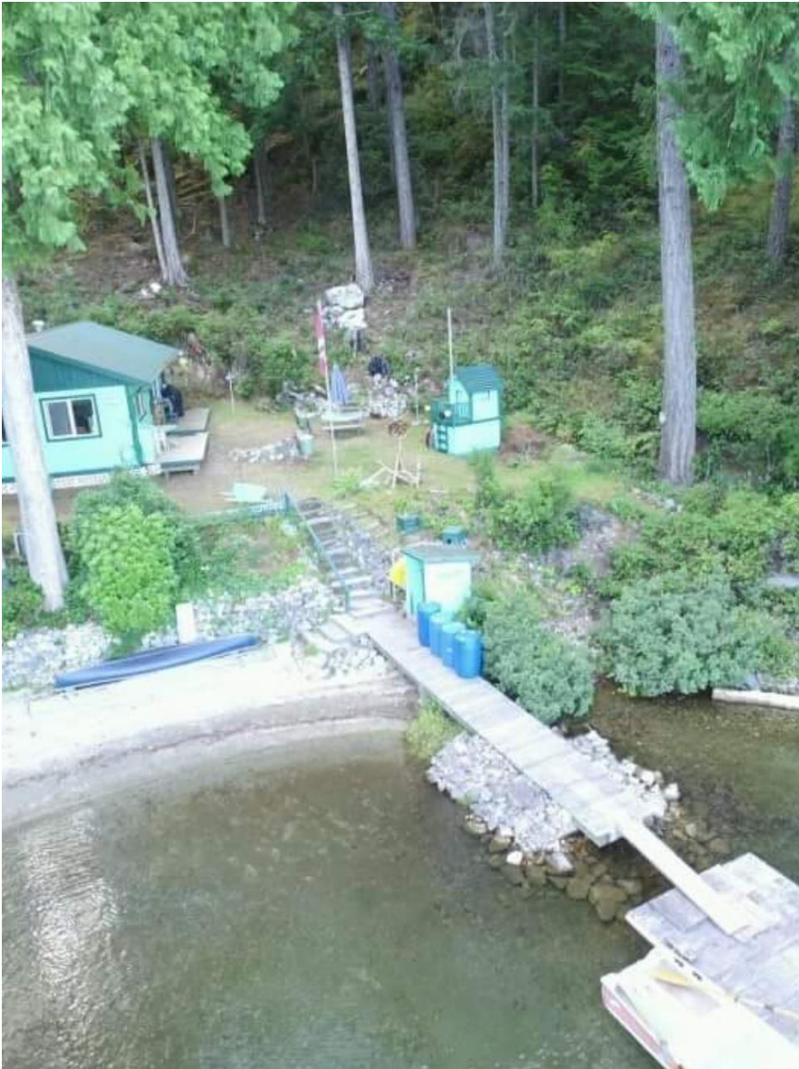
Figure 1 - Existing pier and fill. Dock in lower right damaged in storm.
