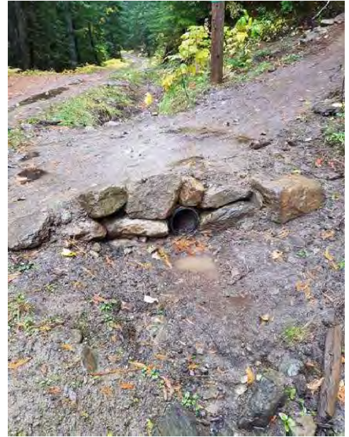
Figure 2. Example of good culvert installation
