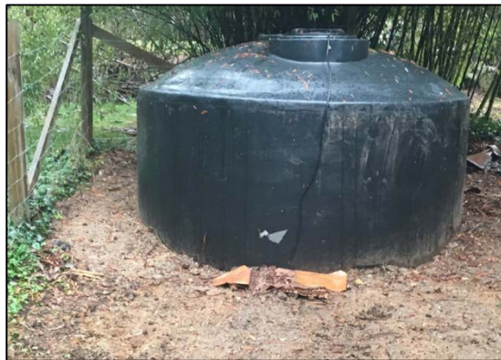
6,546 litre cistern with pump and yard hydrants
