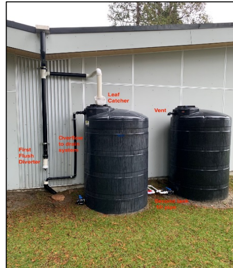
Two smaller tanks to make 4,728 litres of storage
