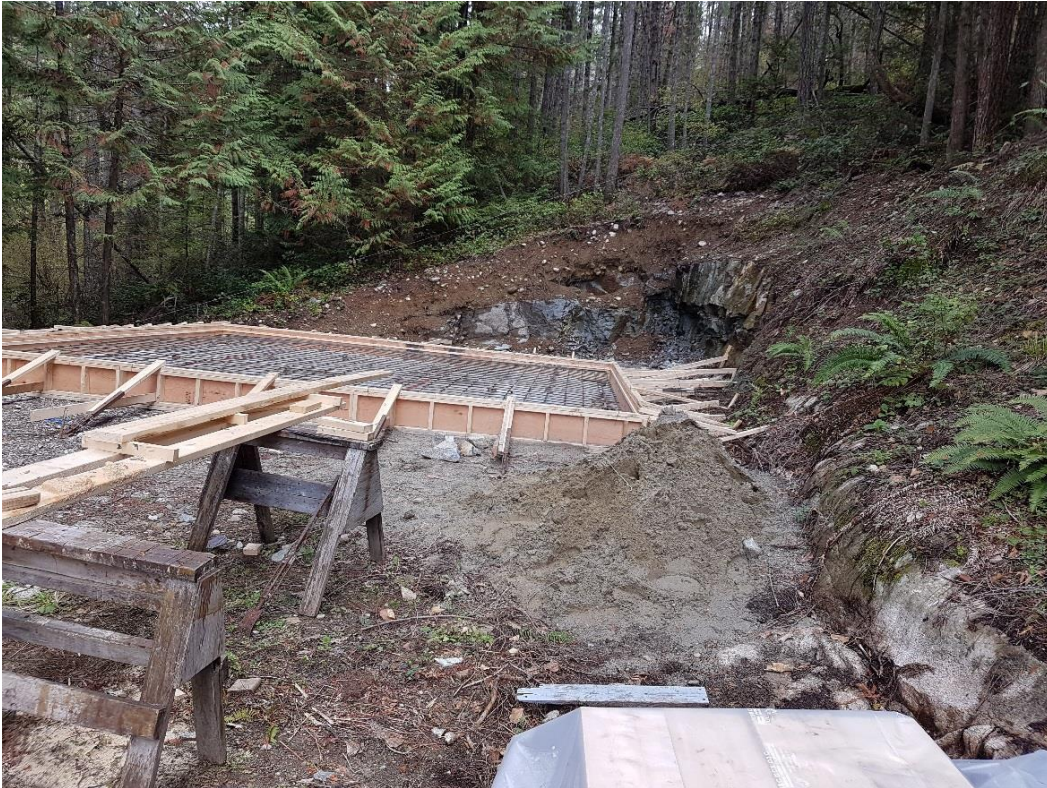
Existing foundation forms and bedrock outcrop
