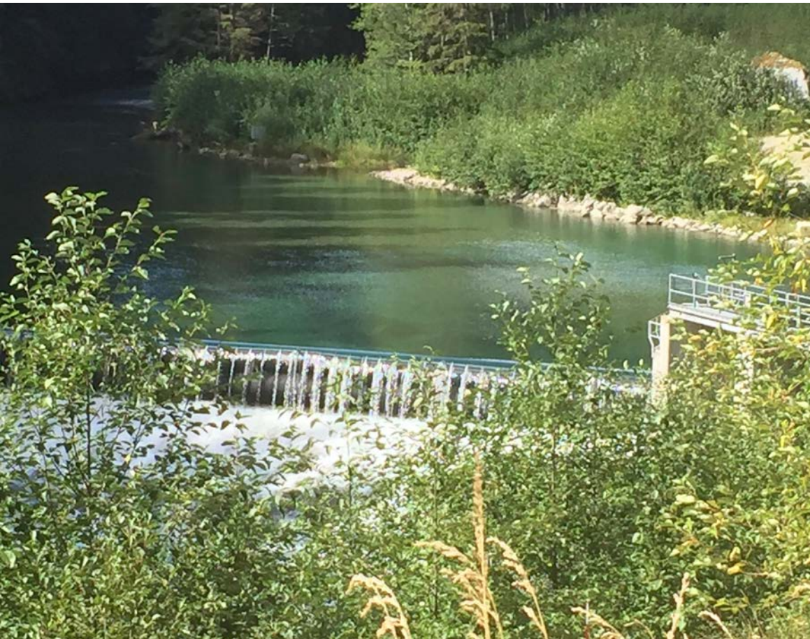
Blue Earth IPP weir at km 22 Clowhom River
