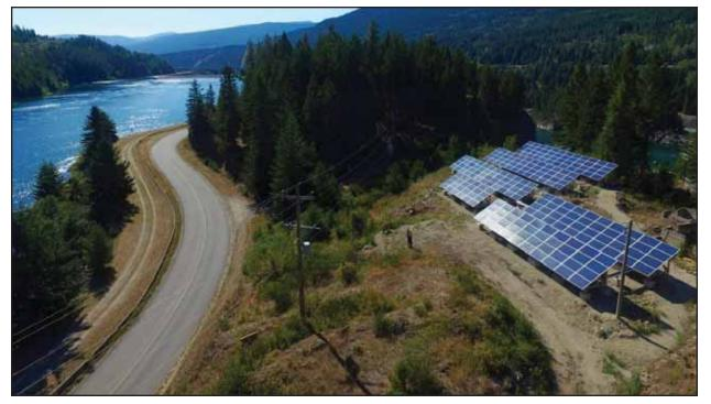
The City of Nelson Community Solar Garden is situated in the vicinity of the Bonington Generating Station in Nelson, BC. The 60 kW solar PV array is comprised of 248 panels, and is operated by Nelson Hydro.
