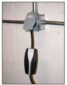
Very few EV vehicles are provided with charger cables for connecting to Level 2 receptacles. Typically what is provided is a connecting cable for Level 1 receptacles with NEMA 5-15 plugs. In this photo a Tesla owner was able to plug in as the vehicle manufacturer makes available a wide range of plug adapters for use with the vehicle charge cable connector kit.
