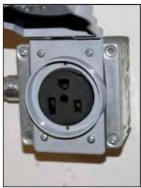
Some municipal EV charging ready bylaws may require Level 2, 240 VAC "energized outlets," without specifying any details. The result is ambiguity with respect to the Canadian Electric Code which only provides a specification for Level 1, 120 VAC receptacles. In this City of North Vancouver located shopping mall, the developer has installed NEMA 6-50 receptacles and no Level 2 chargers.
