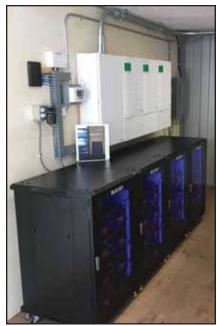
The integrated solar PV battery system at Pender Harbour School. Activated within hours of commissioning due to a grid power outage.
