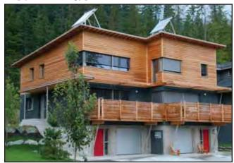
Solar thermal collectors installed at this Whistler, BC certified Passive House Canada duplex. Known as the *Whistler Rainbow Duplex*. Built by Durfeld Constructors.
