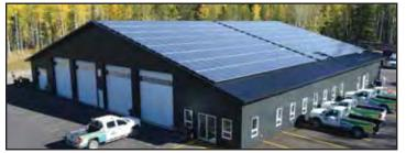
The Public Works Shop with a 92 kW solar PV array.
