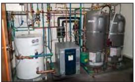
The electric domestic hot water heater (at right) receives pre-heated water from the hydronic heat exchanger tank (at left). Pre-heat water is supplied by the geothermal heat pump (2nd from left), which performs its primary task of heating water for the hydronic in-floor heating.
