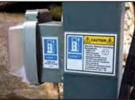
Typically, EV charger bylaws do not provide specifics as to labelling requirements for EV receptacles. Note the photo on the left. Depicted above are some prototype label examples done to address both Level 1 & Level 2 receptacle installations. Development of labelling standards is something that needs attention.
