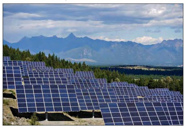
The City of Kimberley's SunMine community solar project situated on the former Teck Sullivan Mine site. The 1.05 mW project is comprised of 4,032 solar PV panels mounted on trackers, and covers an area of 5 acres.
