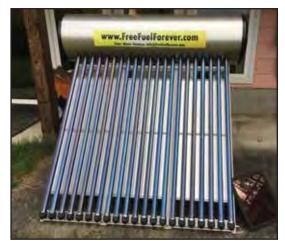
Solar thermal vacuum tube collector array installed at SCCSA member Gerry Pageau's residence on the Sunshine Coast.
