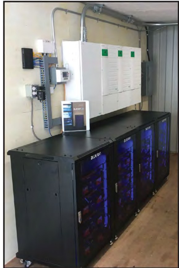
The 80 kWh integrated solar PV lithium battery backup system at Pender Harbour School.
