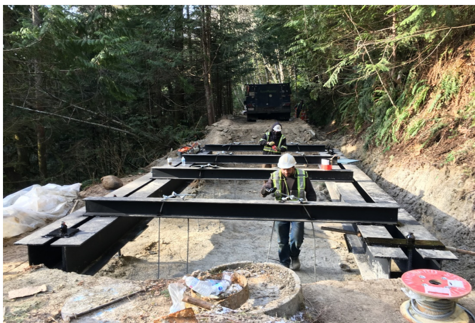
Figure 2: Steel Cradle Assembly and Attachment to Micro Piers
