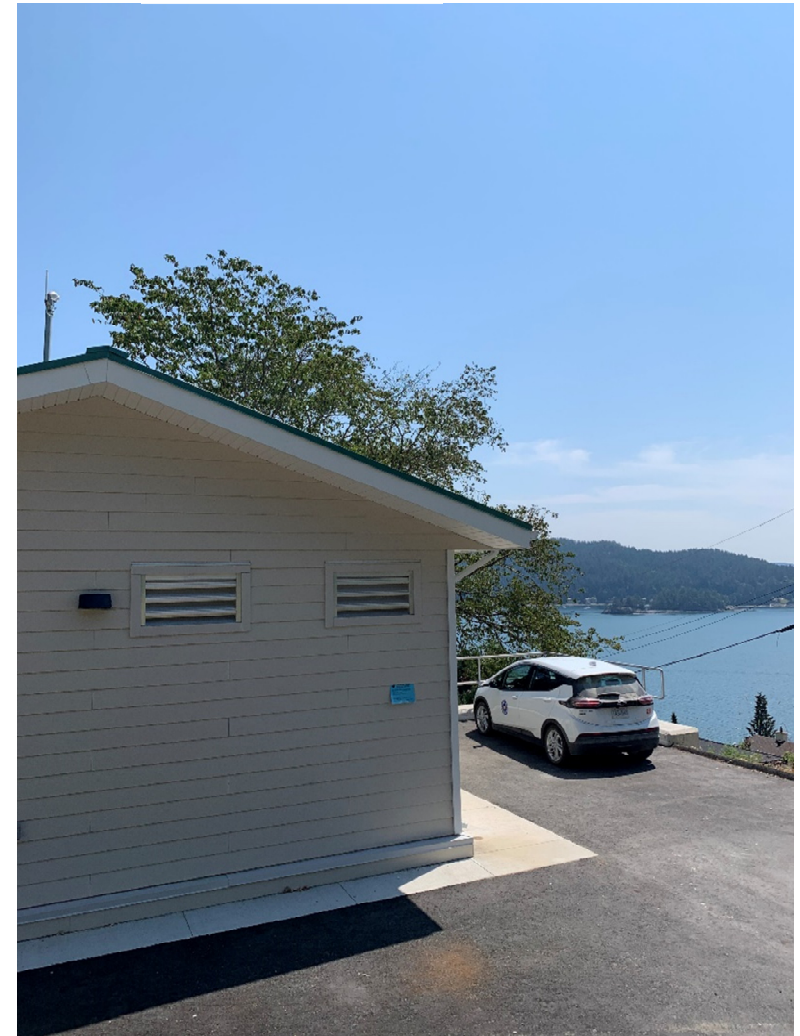
Church Road Water Treatment Plant
