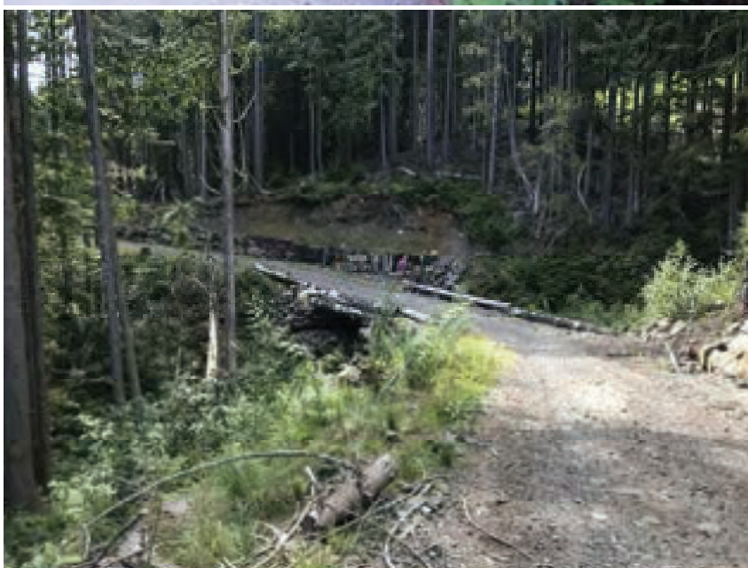
FIGURE 6.9 View of the Sechelt Roberts FSR (7575 Br 23) crossing of a tributary to Chaster Creek at an elevation of 620 m. This example shows a retaining wall that was constructed to stabilize the cutslope and minimize sediment delivery to the stream below. Photo IMG_3093 (Placemark 36), August 24, 2020.
