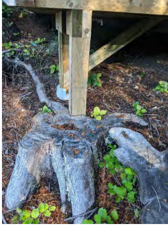
View of the footings, several footings are placed directly on the ground/stumps or concrete deck blocks.
