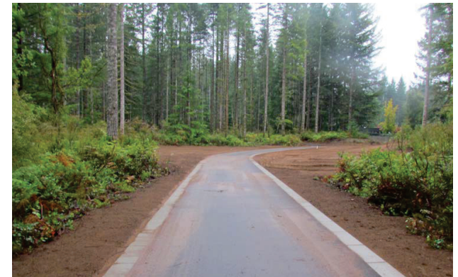
Figure 39: Example of an asphalt driveway with flush concrete curbs. Elk Falls Cemetery, BC. Source: LEES+Associates
