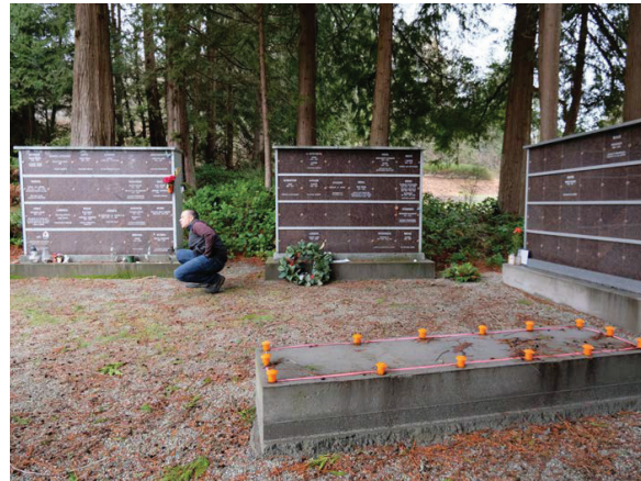
Figure 13: Existing one sided columbaria units and concrete columbaria base.
