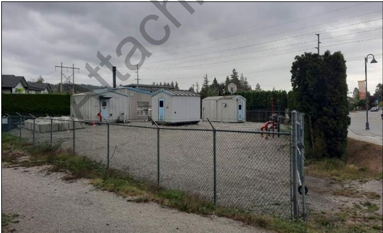
Figure 3 - FortisBC Standard building structures at the Sechelt facility.
