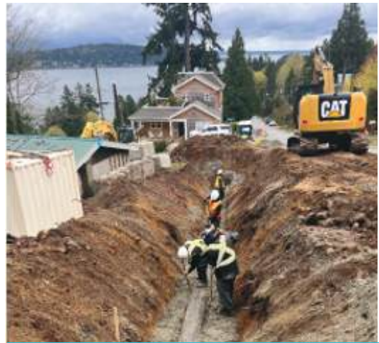
On June 30, 2023, the Church Road well field began operating. The well will contribute 4.6 million litres of water per day to the Chapman water system during dry summer months.
