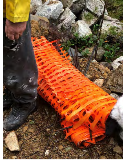
Photo 2. Snow fencing ready to be installed at the SPEA to manage encroachment and protection of trees.
