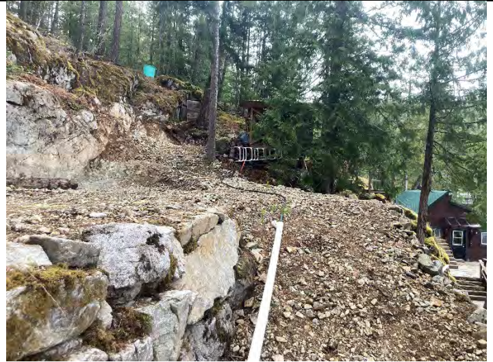
Photo 4. Upland building site, viewing north portion of site.
