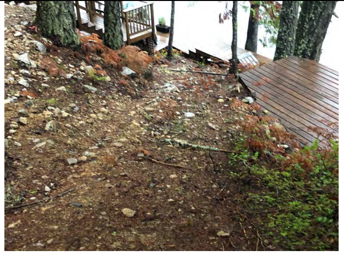
Photo 8: CIA disturbance in foreground, resulting from heavy equipment access for upland site preparation. Viewing northeast. Temporary disturbance will be restored (Restoration Area-1).
