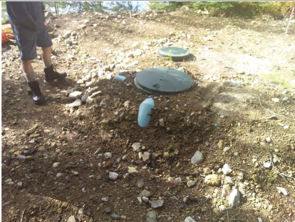
Photo 5. Restoration Area 2 - Encroachment area.
