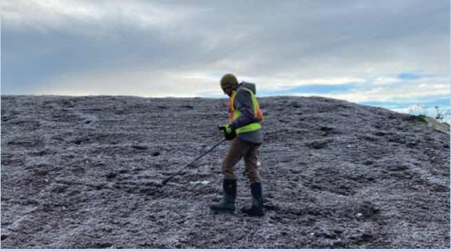
Biocover material was placed at the Sechelt landfill to capture landfill gas. A biocover is a type of landfill final cover that is designed to oxidize methane emissions into carbon dioxide to reduce greenhouse gas emissions.
