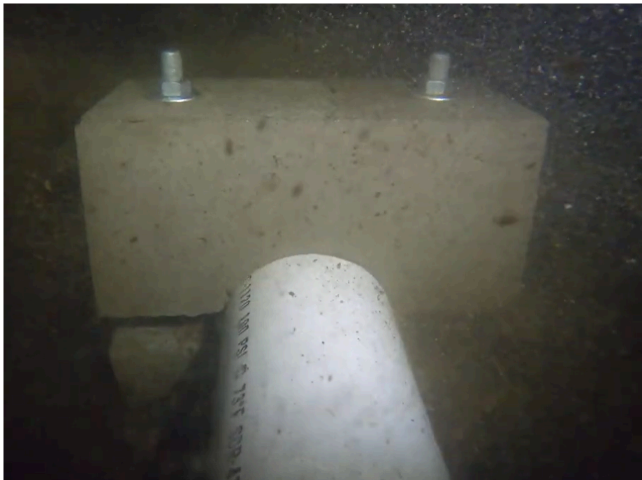
Photo 4: Anchor weights around the existing pipe
