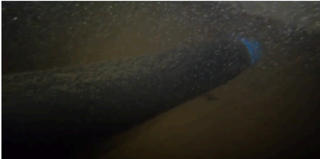
Photo 1: New 4" HDPE pipe installed.
