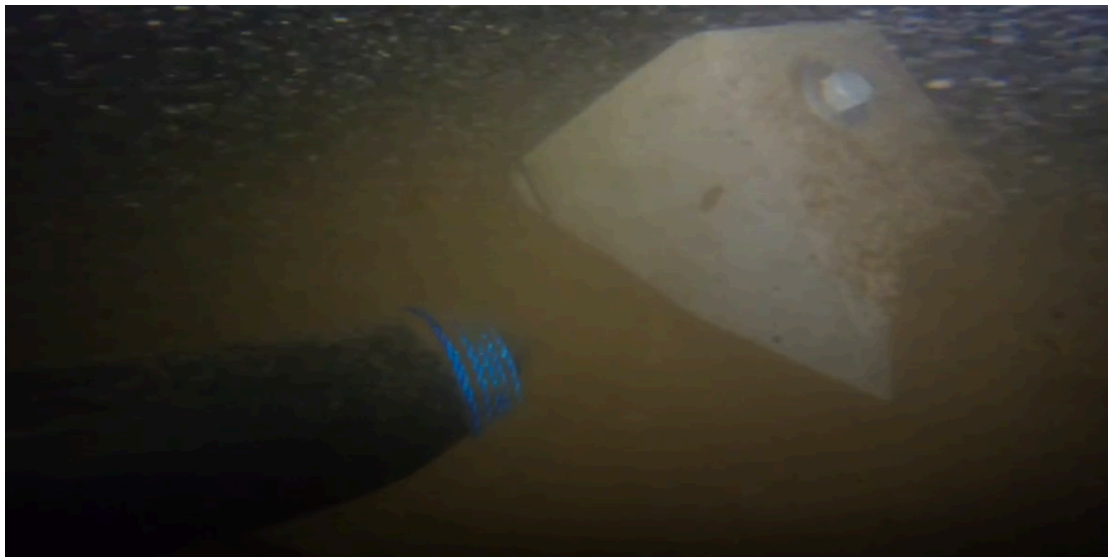
Photo 2: Anchor weights around the new pipe.
