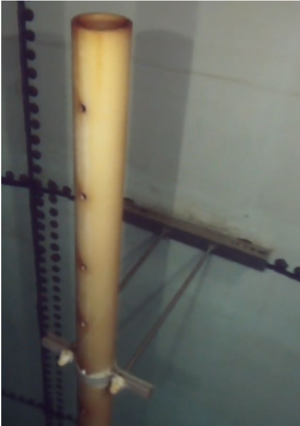
Image 2 - Upper portion of Inlet pipe and Support bracket
