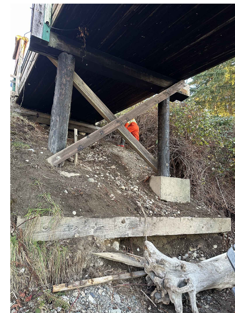
PHOTO OF GRID 1 PILES
