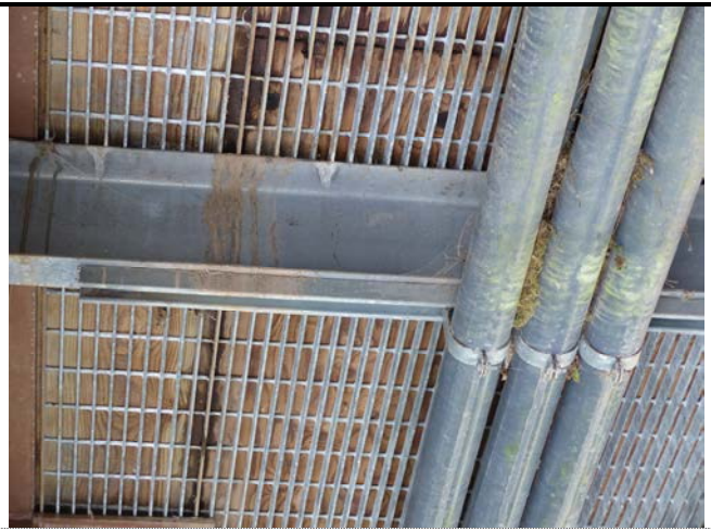
008 – Plywood, Steel Grating and Steel Floor beam, Typical (C.1)
