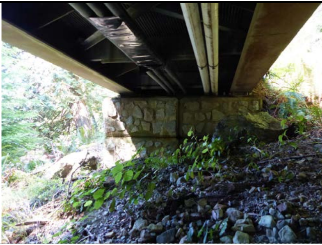
001 – Lock Block Foundation at West end of Bridge (B.1)
