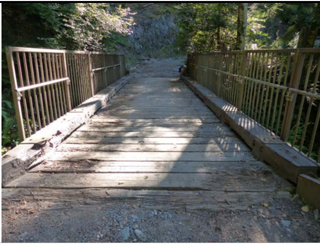
007 – View of Bridge Deck, View from West End of Bridge (D)
