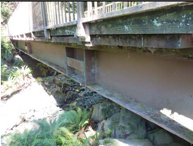
005 – View of Steel Girder along South side of Bridge (C.3)
