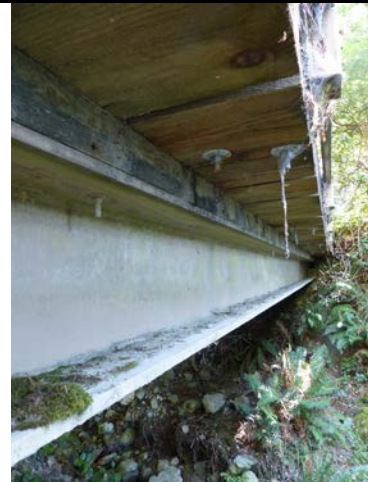
006 – Girder spanning E-W along South side of Bridge (C.3)
