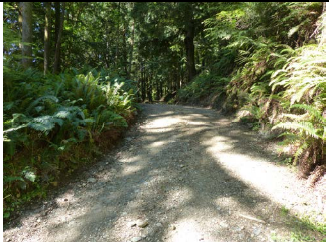
018 – Steep Uphill Grade and Curve at Roadway Approach at West end of Bridge (E.2)
