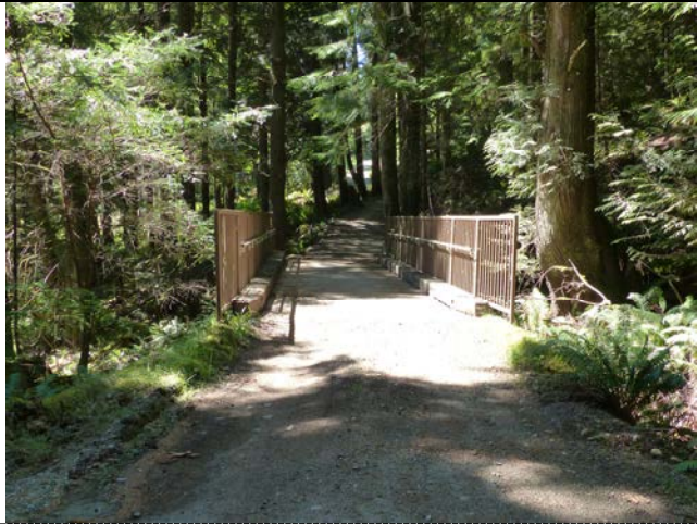
010 – View of Bridge Deck, View from East End of Bridge (D)
