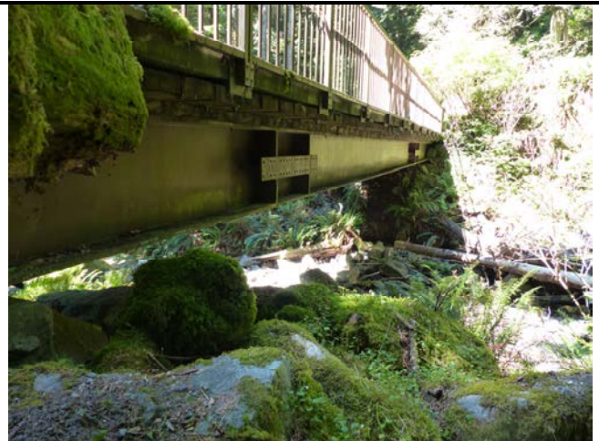
006 – View of Steel Girder along North side of Bridge (C.3)
