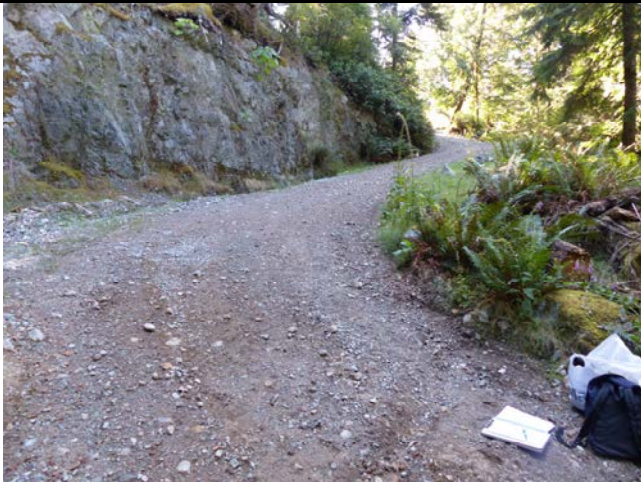
017 – Road Approach at East End of Bridge (E.2)
