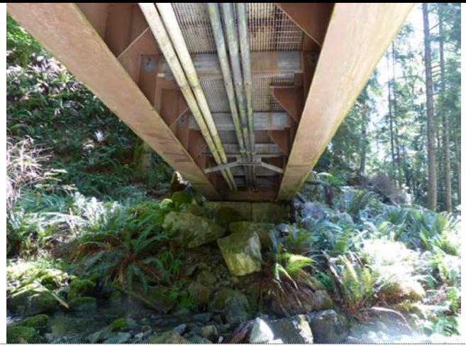
002 – View Underneath Deck and Foundation at East End of Bridge (B.1)
