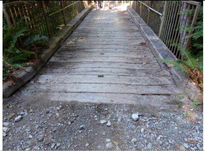
016 – Deck and Approach at East end of Bridge (D.2, E.2)
