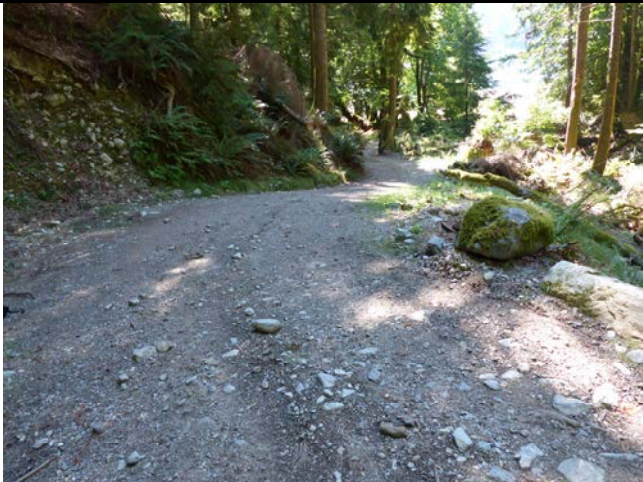
017 – Downhill Road Approach at East End of Bridge (E.2)
