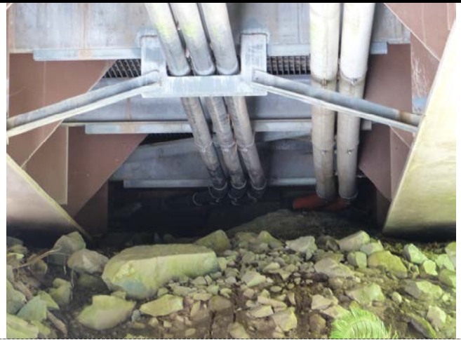
004 – View Underneath Deck at West End of Bridge (B.1)
