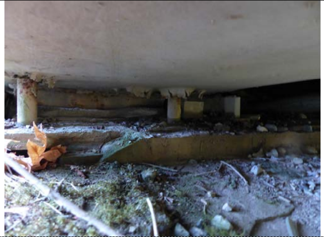
004 – Anchor Bolts at SW Corner of Bridge (B.6)
