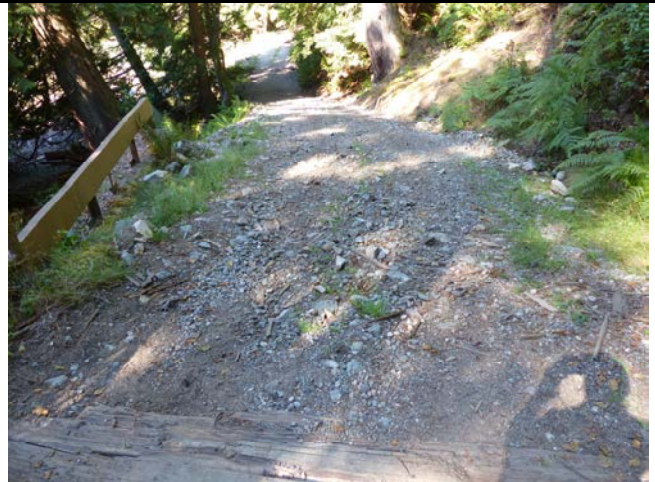
018 – Steep Grade and Curve at Roadway Approach at West end of Bridge (E.2)
