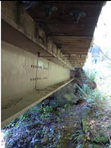
005 – E-W spanning Girder at North Side of Bridge (C.3)
