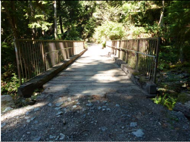
009 – View of Bridge Deck, View from East End of Bridge (D.2)
