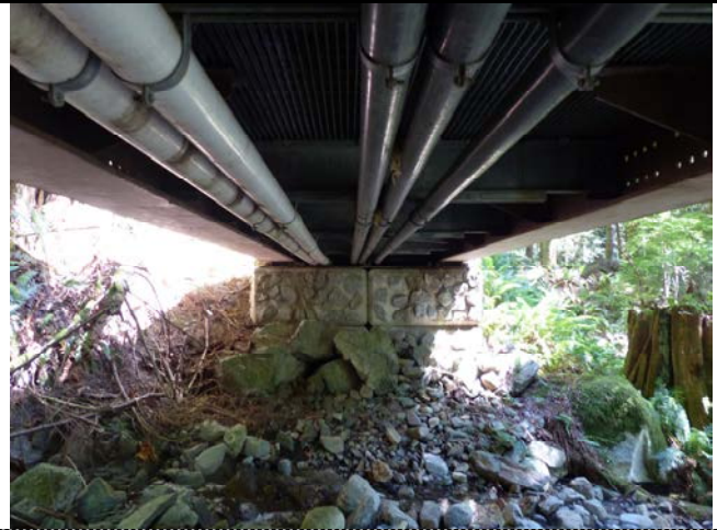
004 – View Underneath Deck and Foundation, East End of Bridge (B.1)
