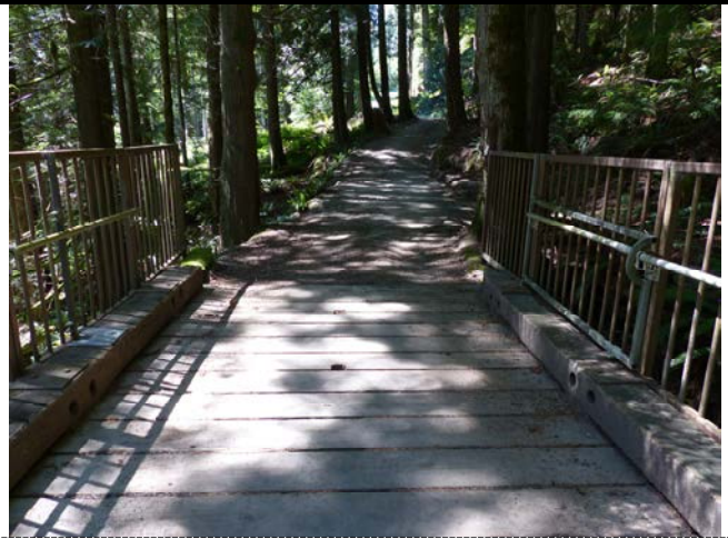
016 –Roadway Approach at West end of Bridge (E.2)
