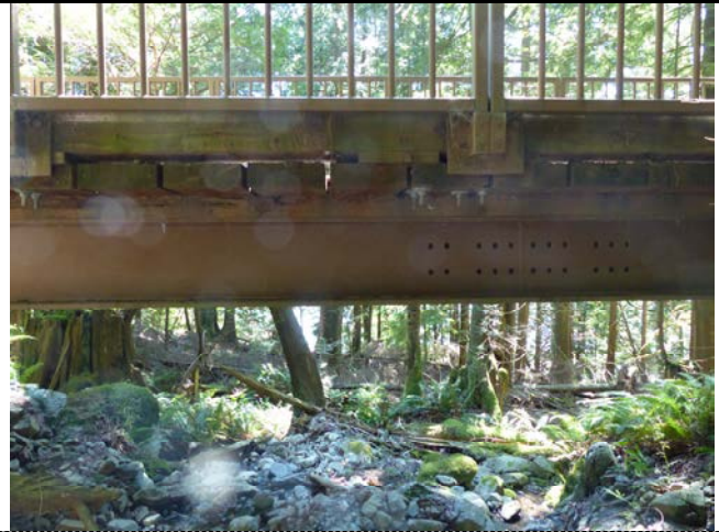
006 – Typical Condition of Bridge, View of North Side of Bridge (C.3)
