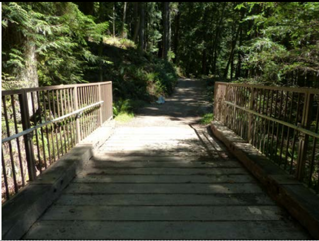
015 – Roadway Approach at East End of Bridge (E.2)
