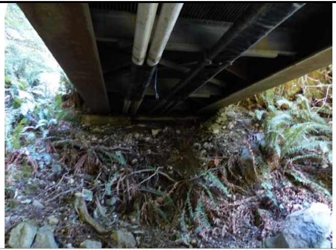
002 – Foundation at East End of Bridge (B.1)
