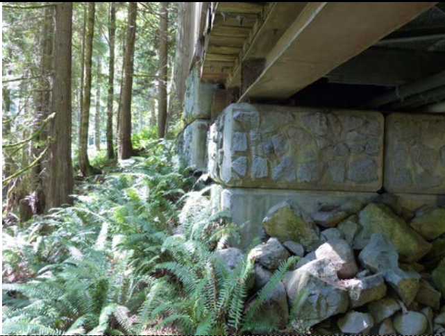
005 – Lock Block Foundation at West End of Bridge (B.1)
