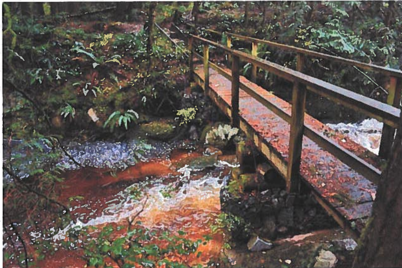
Coop Bridge from the South-East
