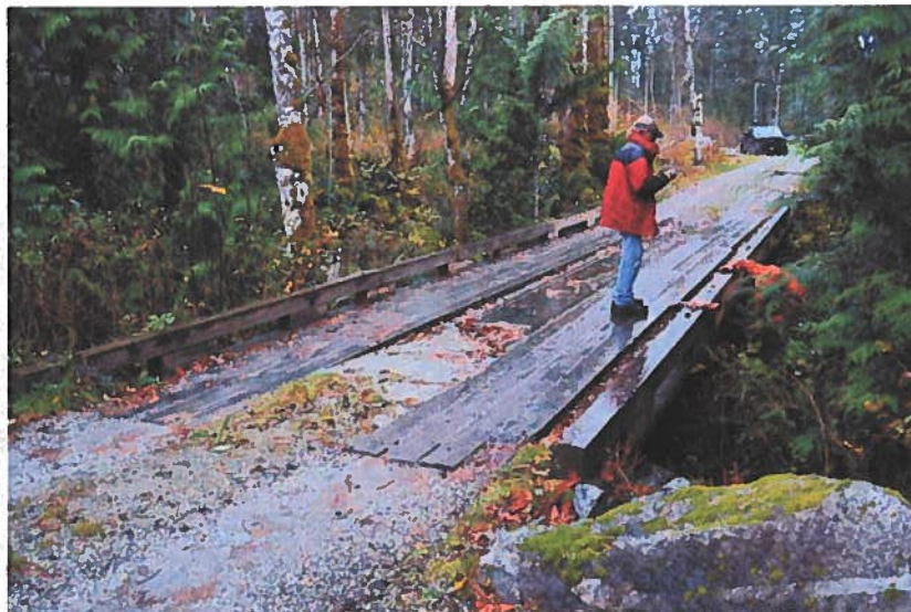
Photo 1 Lions Field Bridge from the South
