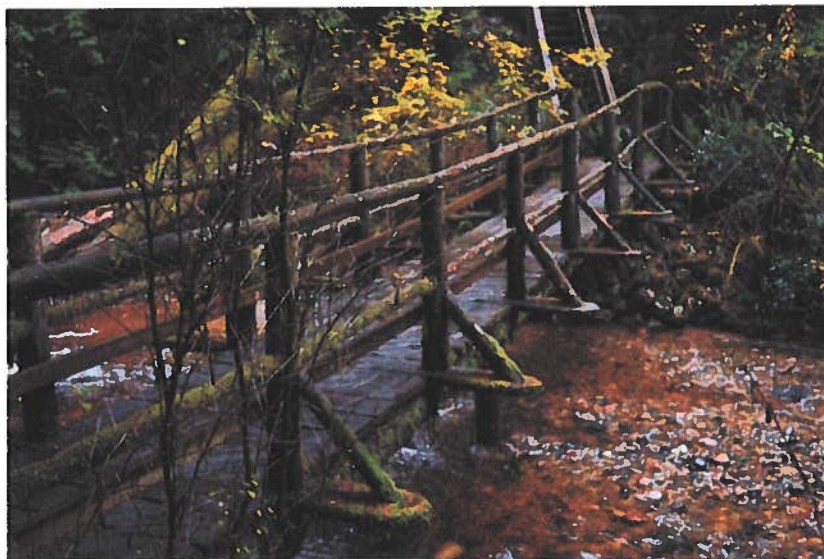
CLIFF GILKER PARK Blue Trail Roberts Creek Bridge from the South
