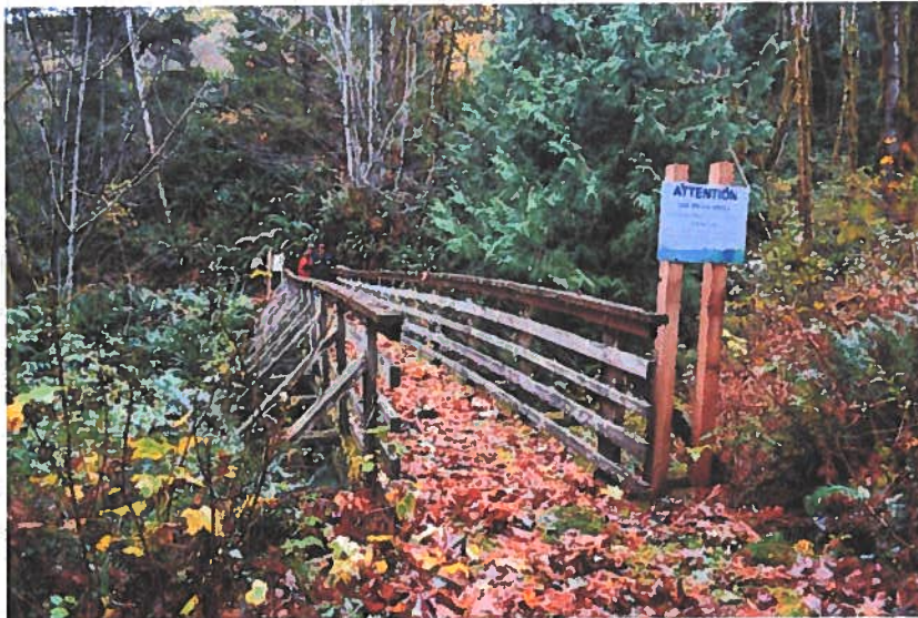
Photo 1 Vine Brook Bridge from the East
