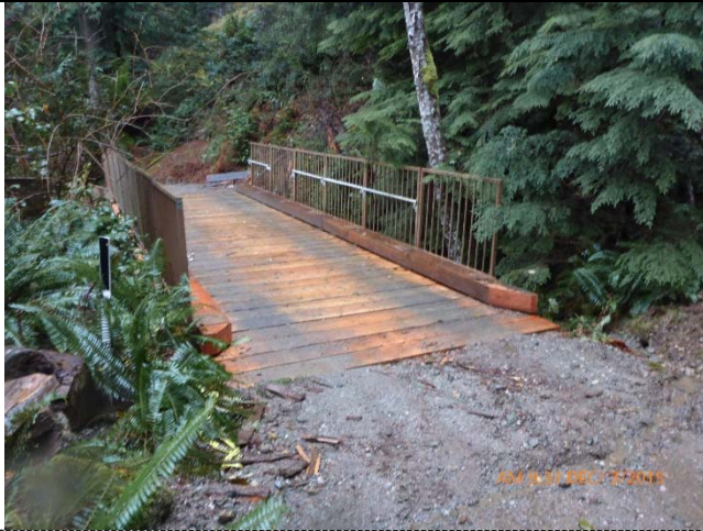
001 – View of Bridge from East Approach – Note missing handrails at N side
