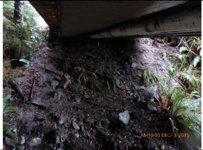
002 – Embankment at East End of Bridge (B.1)
