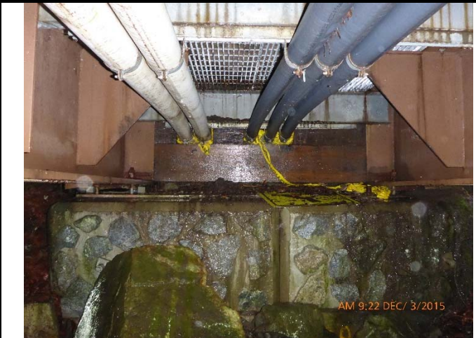
004 – View of Service Lines Underneath Deck and West Abutment (B.1)
