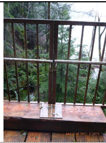
008 – Typical Guard Rail & Curb Rail Condition (D.4, D.6)
