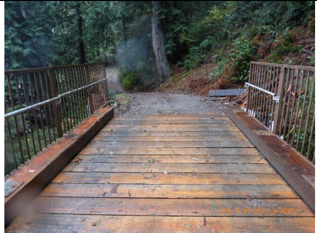
004 – Bridge Deck at West Approach, View from Center of Bridge (D)
