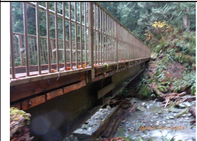
006 – View of Steel Girder and North side of Bridge (C.3)
