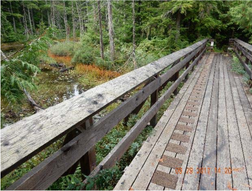
P03 – West railing (DSCN0033.jpg)
