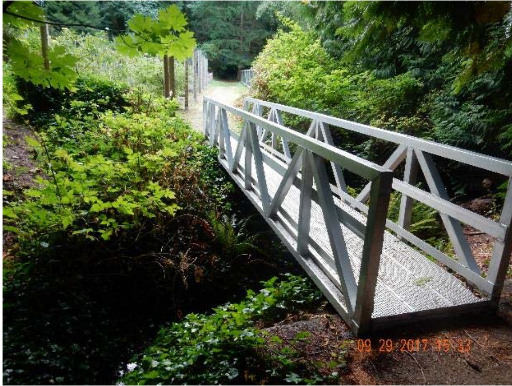
P03 – East side of the bridge (DSCN0066.jpg)
