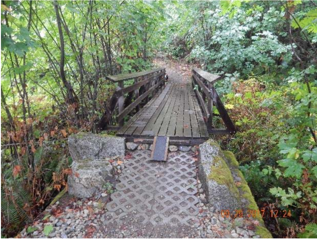
P07 – South approach (DSCN0005.jpg)
