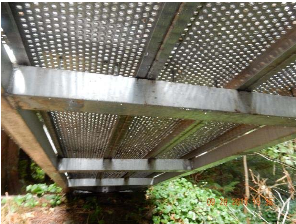
P14 – Under side of the bridge (DSCN0078.jpg)
