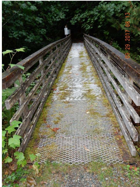
P02 – Overall decking (DSCN9846.jpg)
