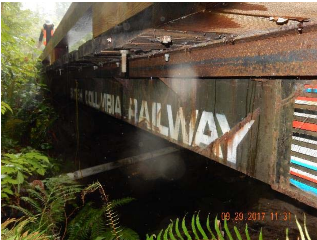
P10 – East side of the bridge (DSCN9965.jpg)
