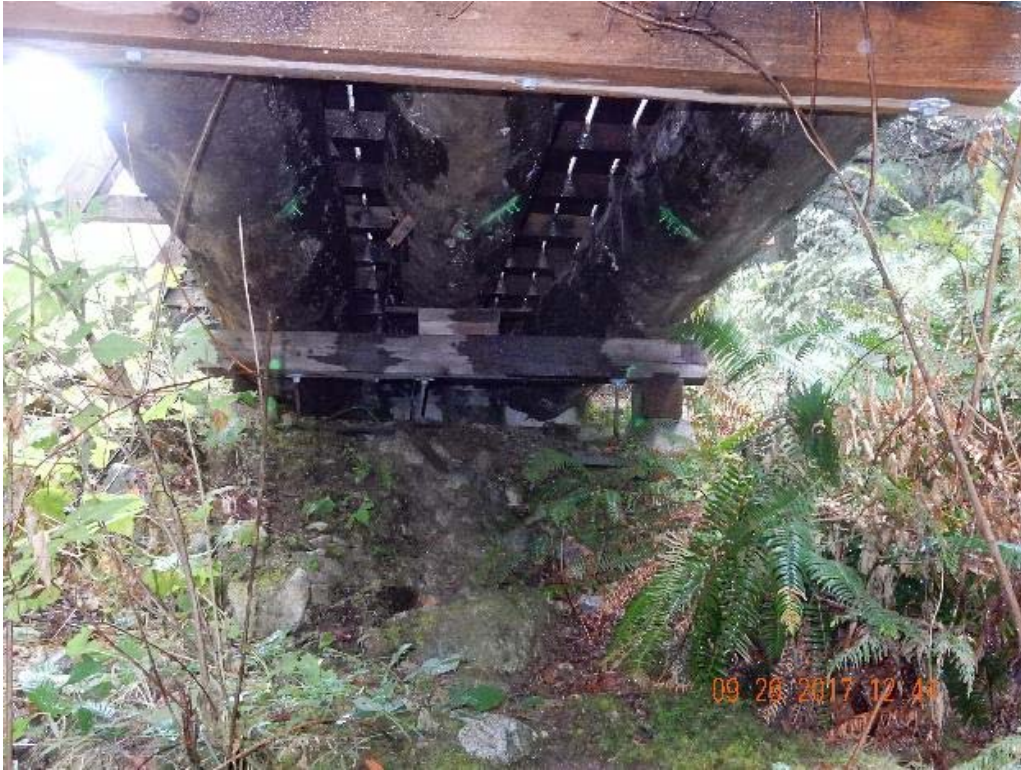
P11 – South embankment (DSCN0027.jpg)
