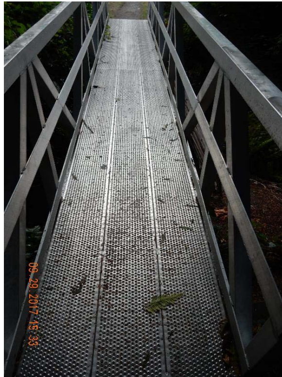
P04 – Overall decking (DSCN0067.jpg)
