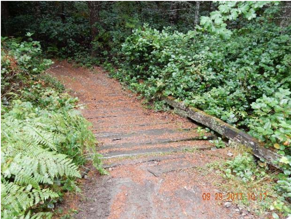
P01 – South approach (DSCN9924.jpg)
