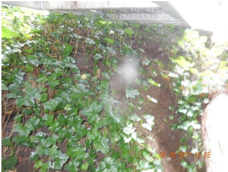
P12 – South embankment (DSCN0076.jpg)
