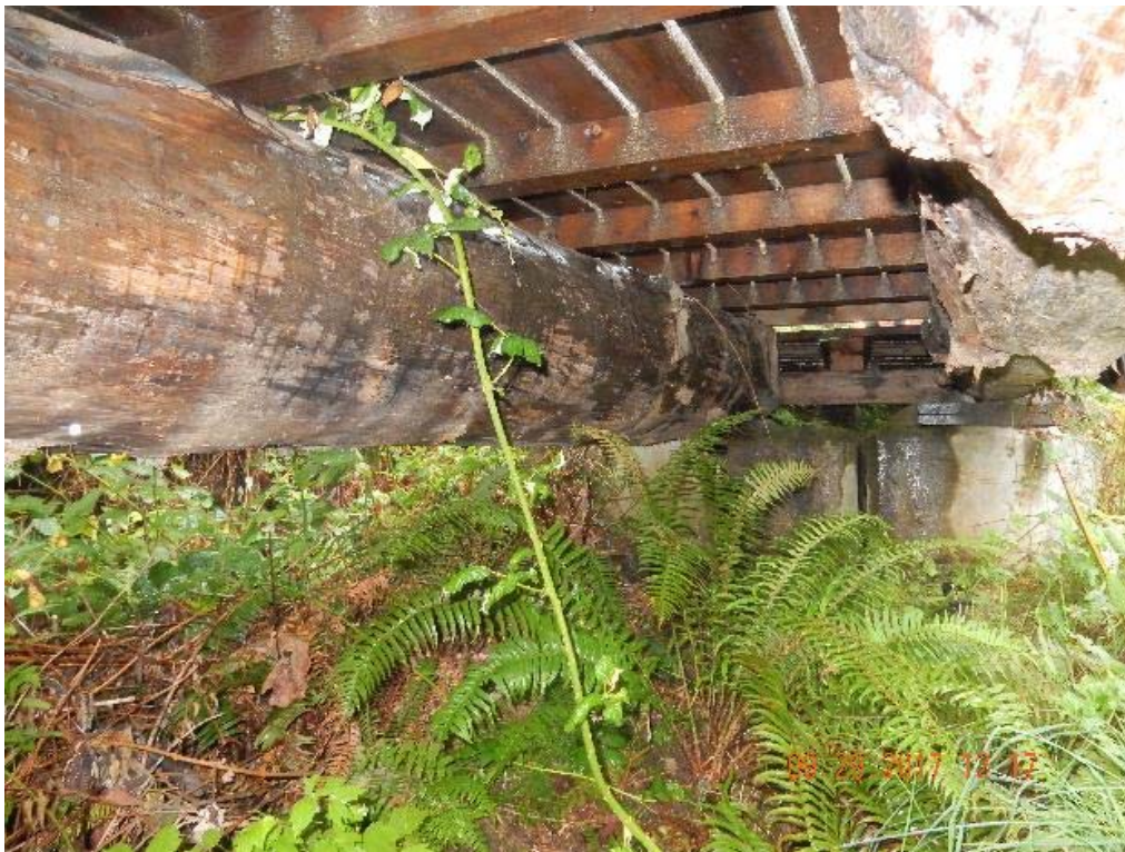
P10 – Under side of the bridge (DSCN9992.jpg)
