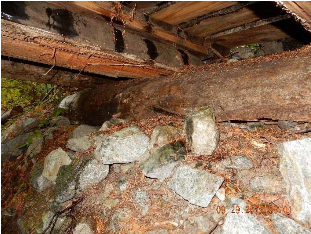
P07 – North abutment (DSCN9912.jpg)
