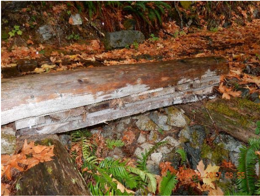
P05 – West side of the bridge (DSCN9889.jpg)
