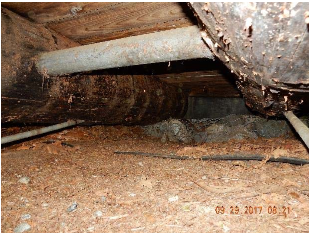
P16 – North abutment (DSCN9867.jpg)
