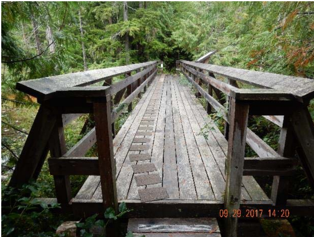
P02 – Overall decking (DSCN0032.jpg)
