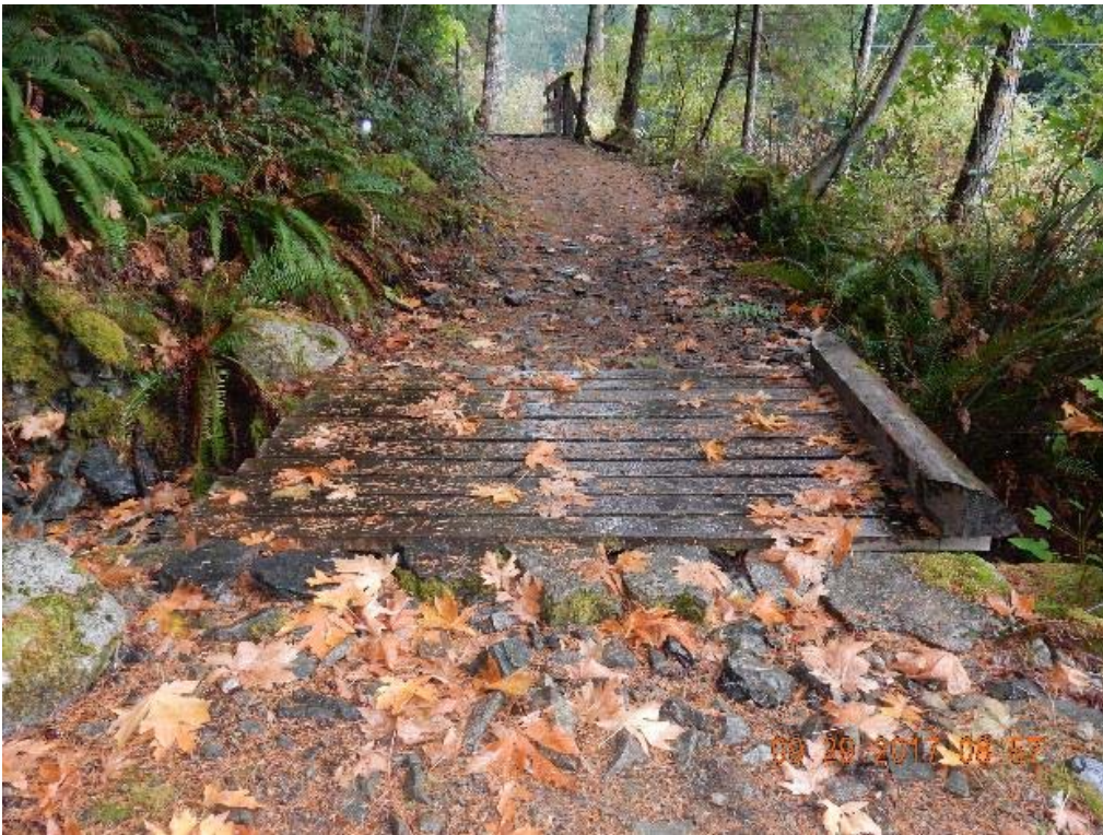
P04 – North side of the bridge (DSCN9898.jpg)
