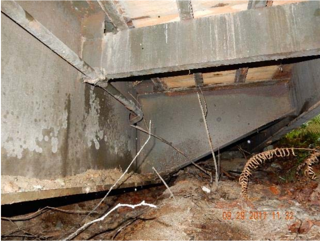
P11 – West side of the bridge, looking at triangular diaphragm (DSCN9966.jpg)
