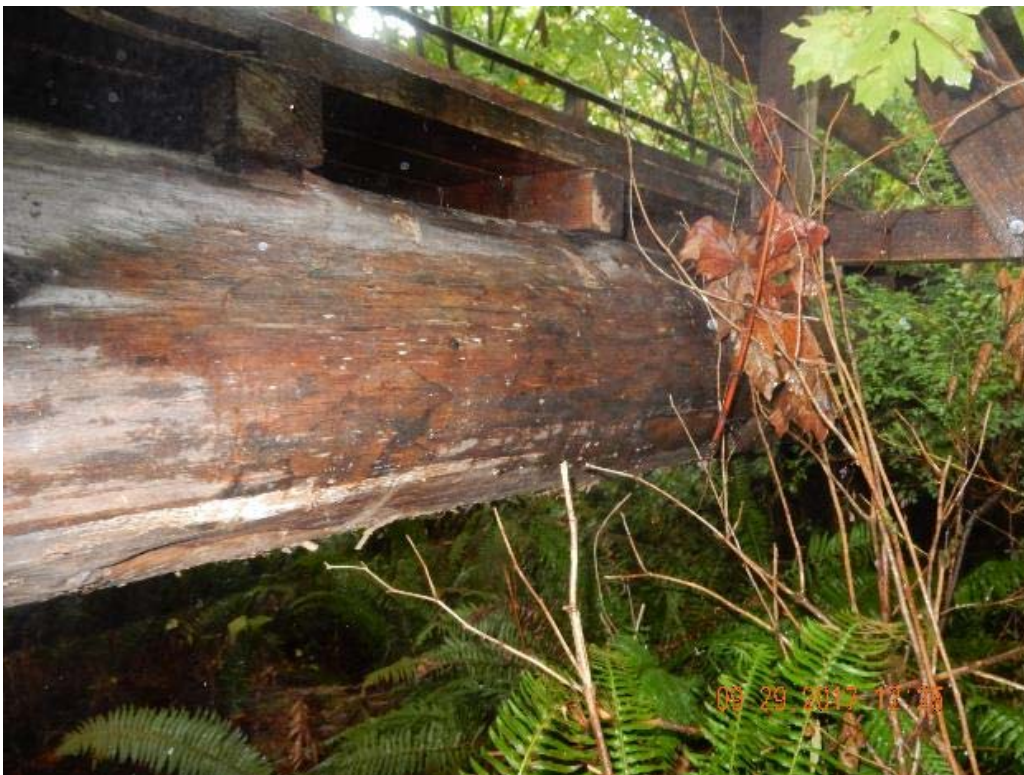
P08 – East side of the bridge (DSCN0006.jpg)
