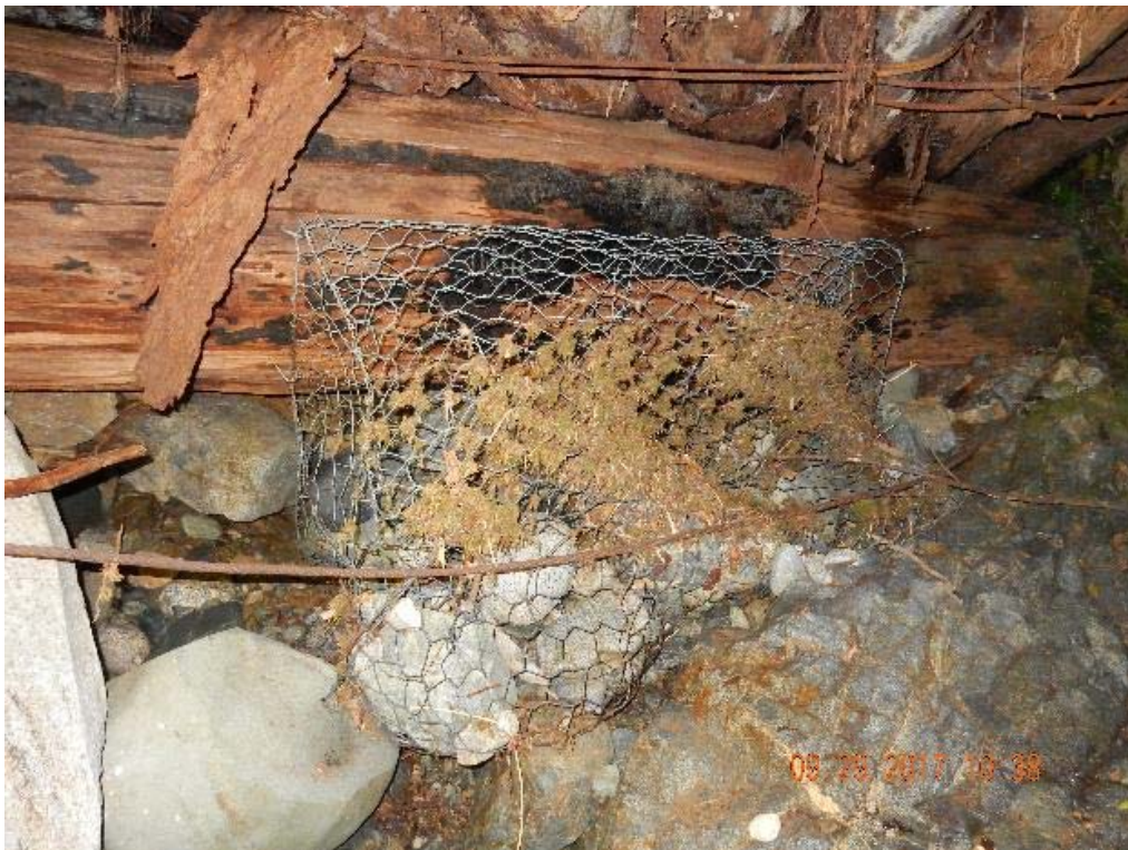
P10 – Gabion basket at north abutment (DSCN9944.jpg)
