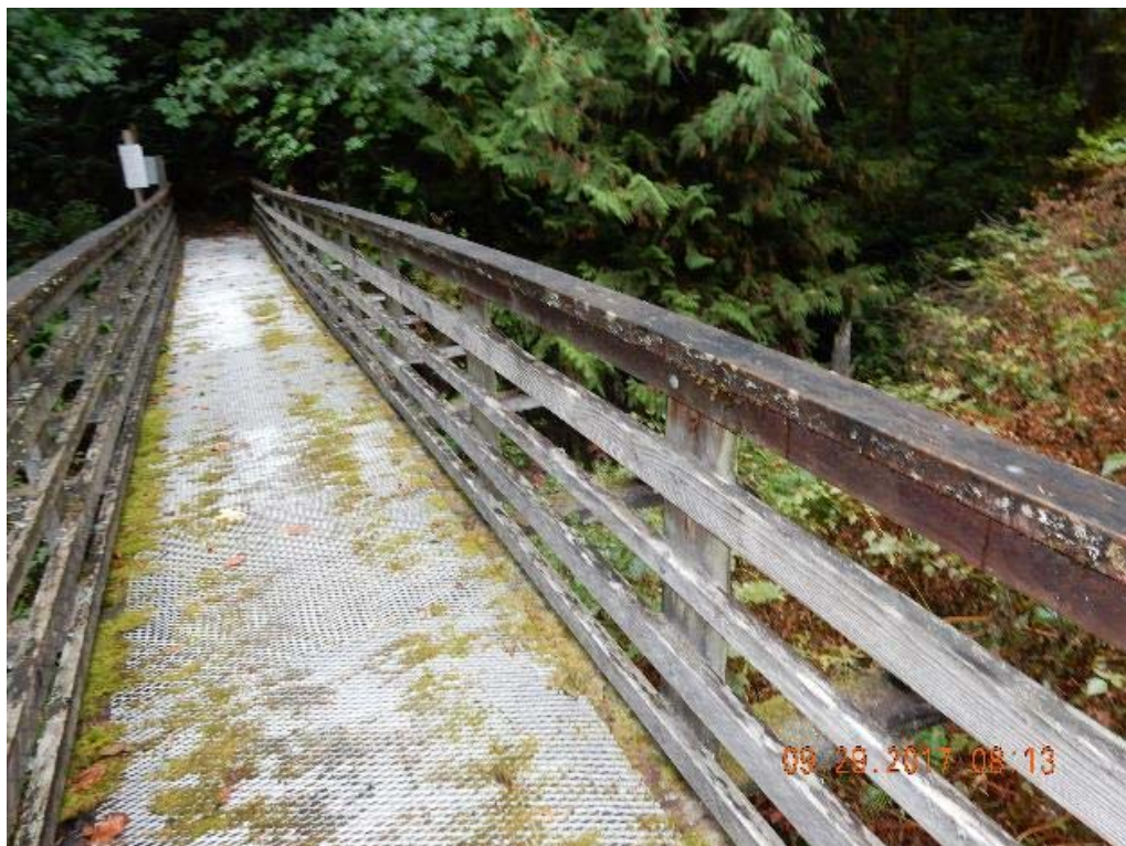
P04 – East railing (DSCN9848.jpg)
