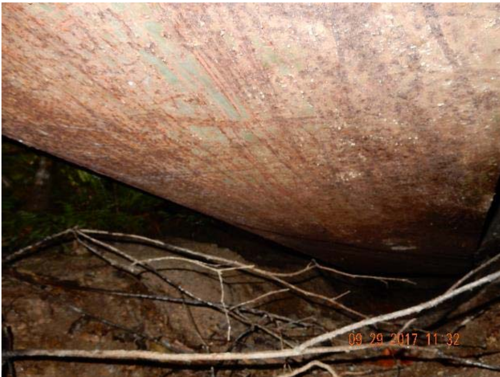
P12 – Under side of the main box girder (DSCN9967.jpg)
