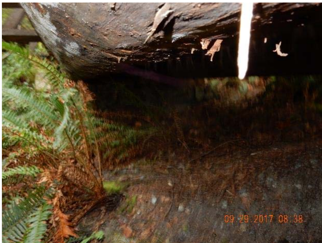
P08 – Under side of the bridge (looking at north abutment) (DSCN9879.jpg)
