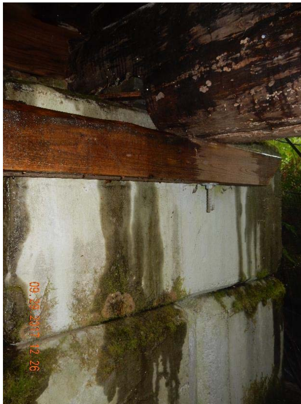
P10 – South abutment (DSCN0008.jpg)
