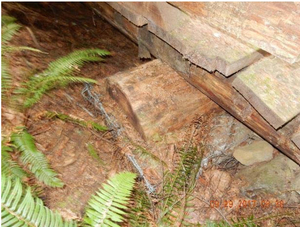
P10 – North abutment (DSCN9881.jpg)
