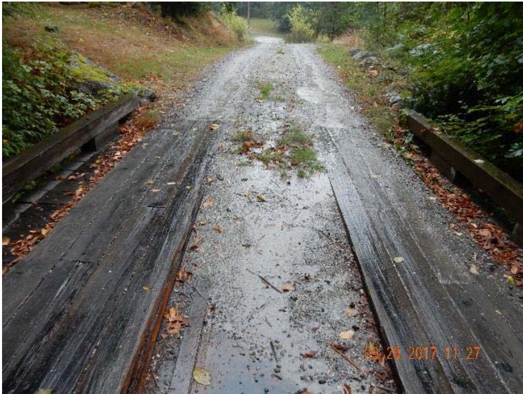
P05 – South end of the bridge (DSCN9958.jpg)
