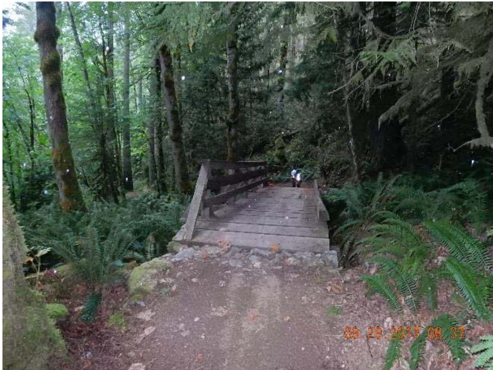
P04 – South approach (DSCN9873.jpg)
