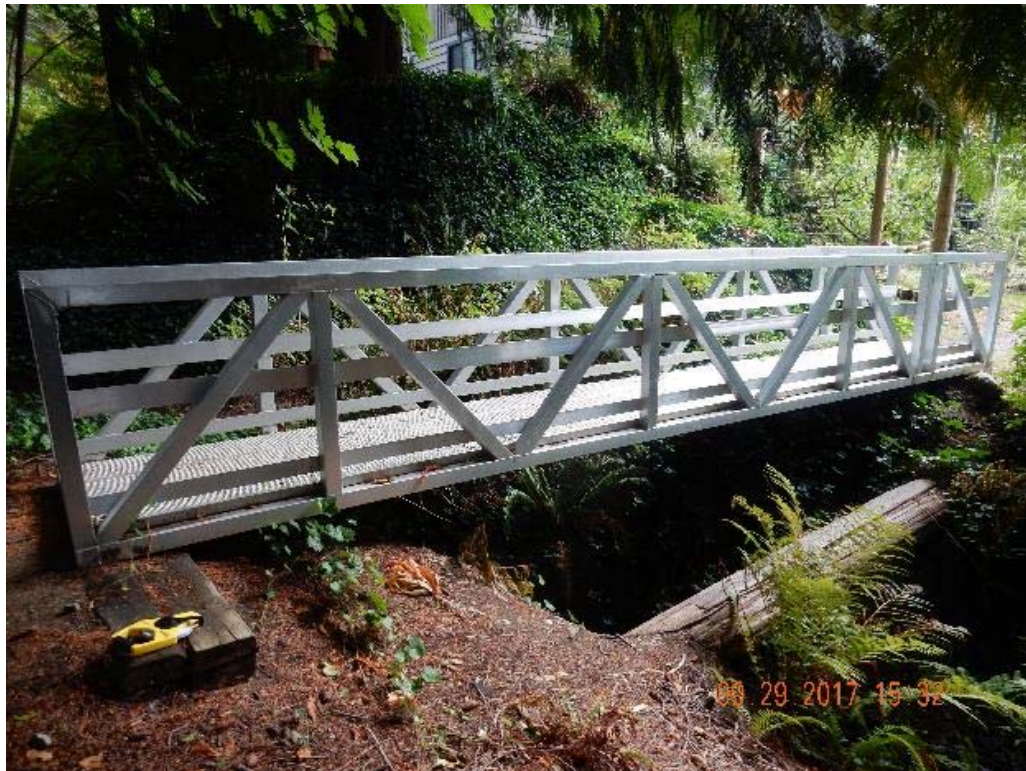
P02 – West side of the bridge (DSCN0065.jpg)
