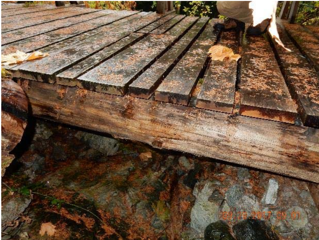
P05 – East side of the bridge (DSCN9910.jpg)
