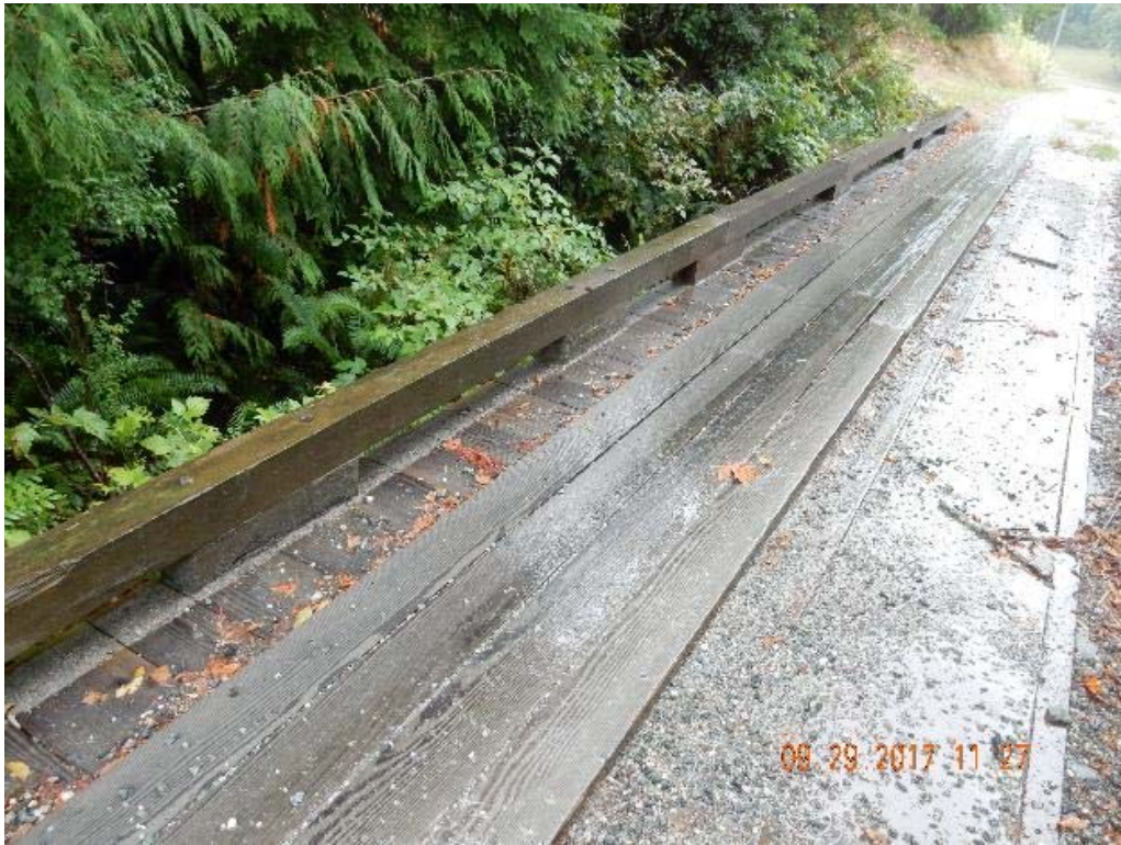
P03 – East curb (DSCN9955.jpg)
