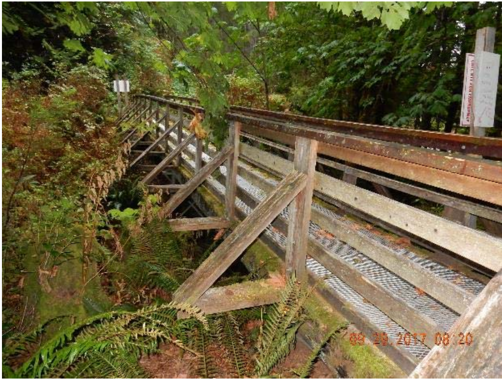
P15 – East side of the bridge (DSCN9866.jpg)
