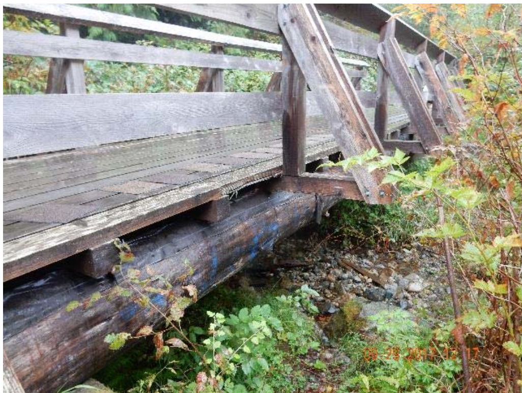
P08 – East side of the bridge (DSCN9989.jpg)
