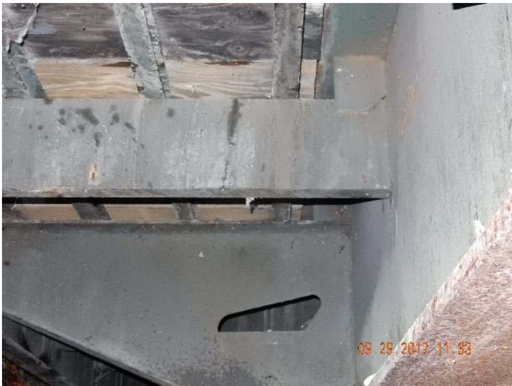
P16 – Detail view of floor beam (DSCN9973.jpg)
