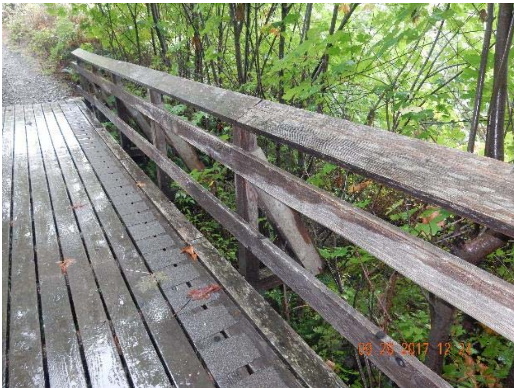
P04 – West railing (DSCN0002.jpg)
