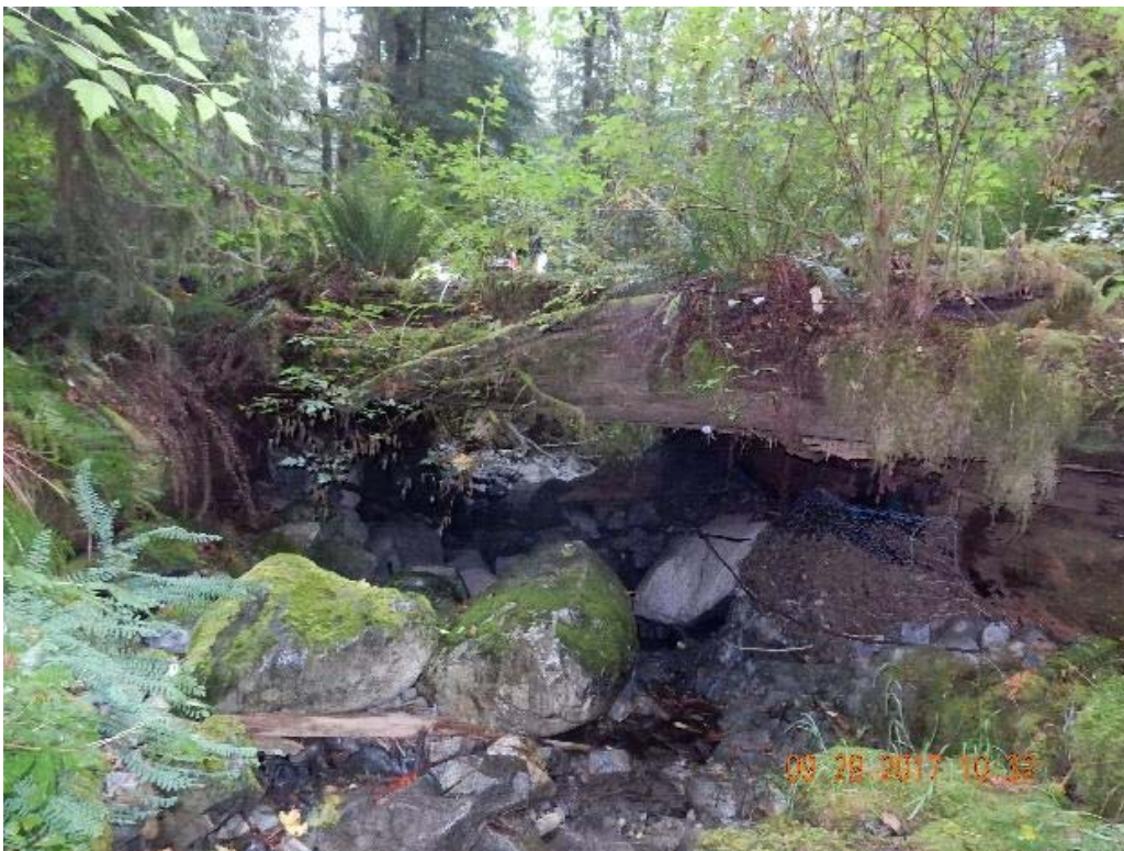
P06 – East side of the bridge (DSCN9937.jpg)
