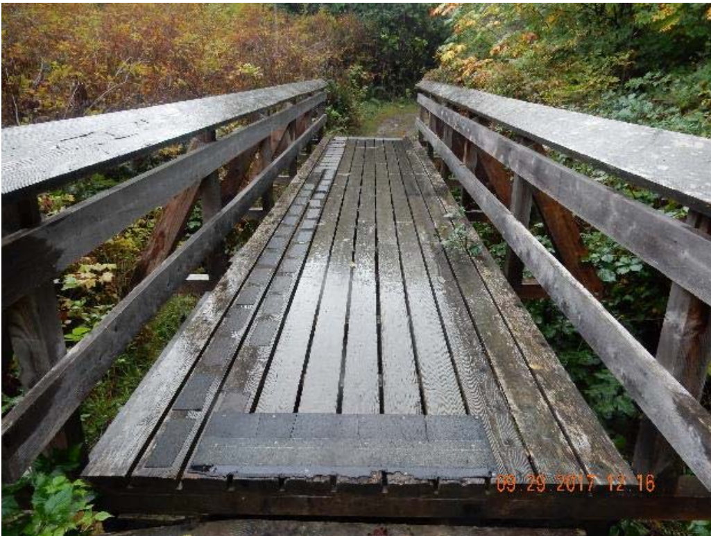
P02 – Overall decking (DSCN9983.jpg)
