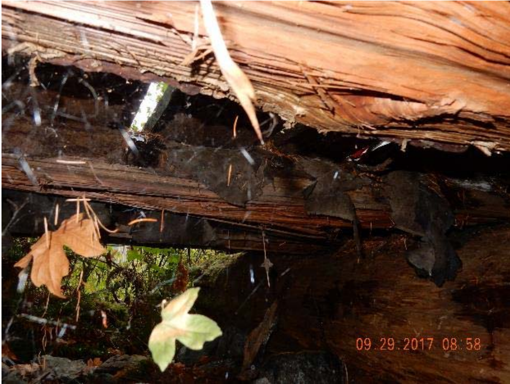
P09 – Under side of the bridge (DSCN9903.jpg)
