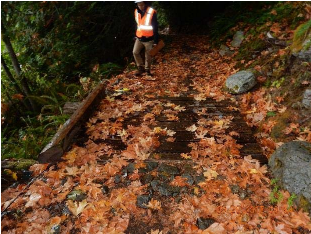
P01 – South approach, suggest adding anti-slip pad (DSCN9884.jpg)
