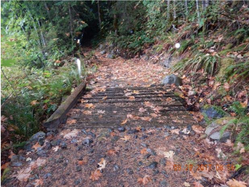
P01 – South approach (DSCN9894.jpg)
