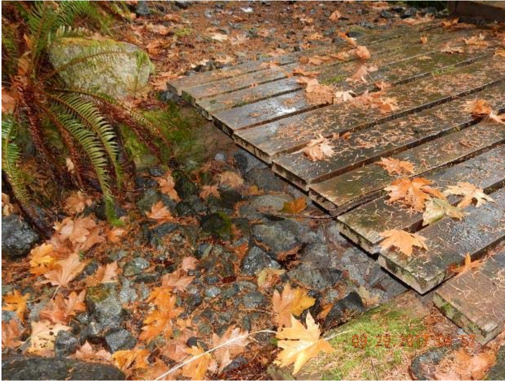
P05 – East side of the bridge (DSCN9899.jpg)
