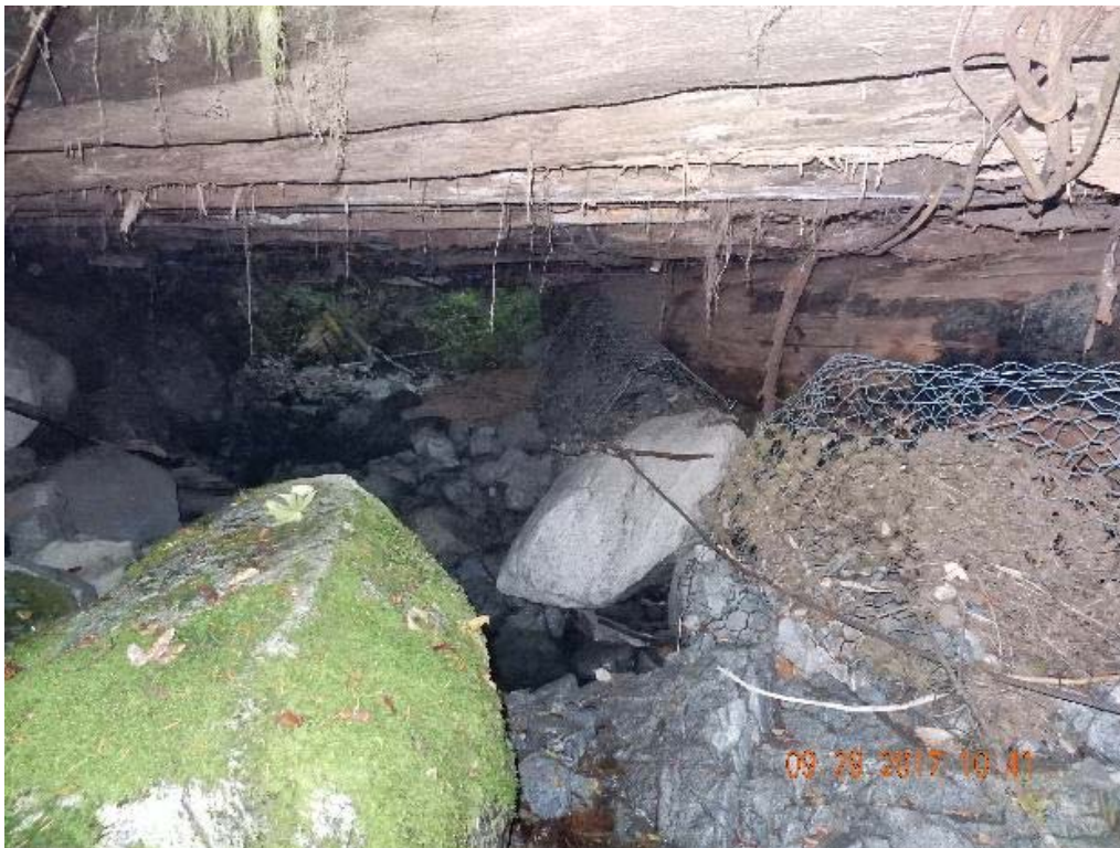
P12 – East side of the bridge (looking at north abutment) (DSCN9949.jpg)
