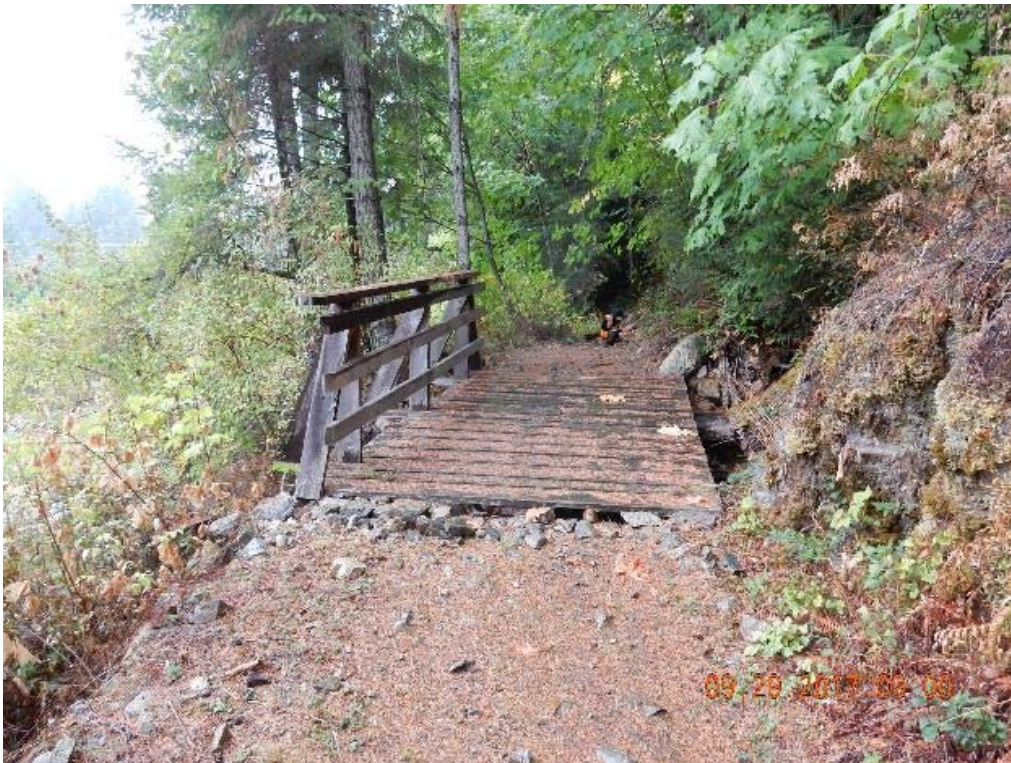
P04 – South approach (DSCN9908.jpg)
