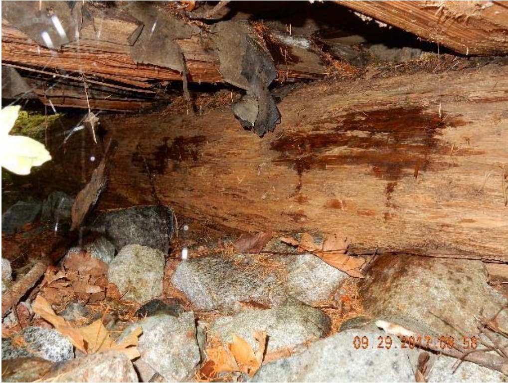
P07 – North abutment (DSCN9901.jpg)
