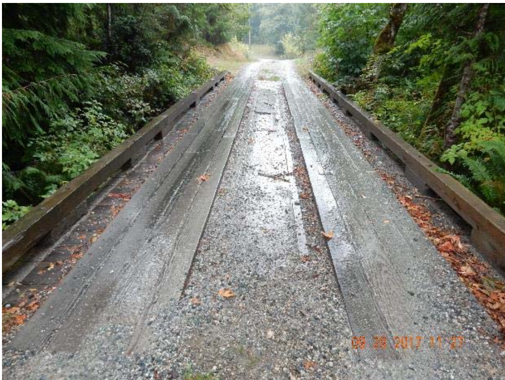
P02 – Overall decking (DSCN9954.jpg)
