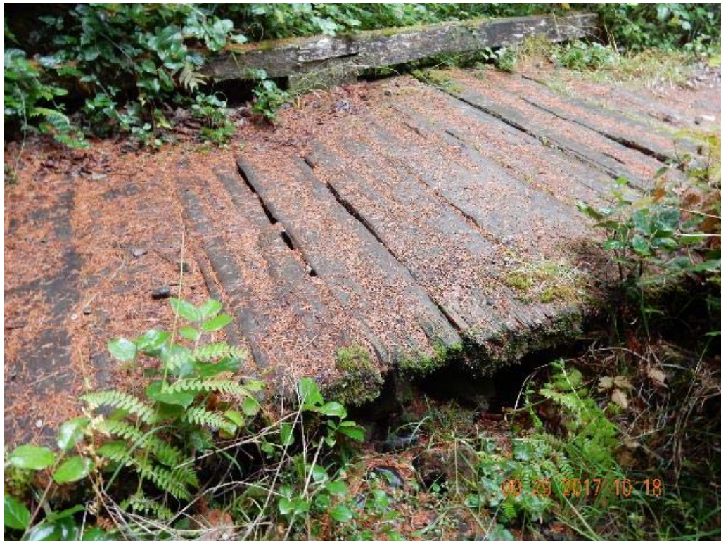
P04 – West side of the bridge (DSCN9927.jpg)
