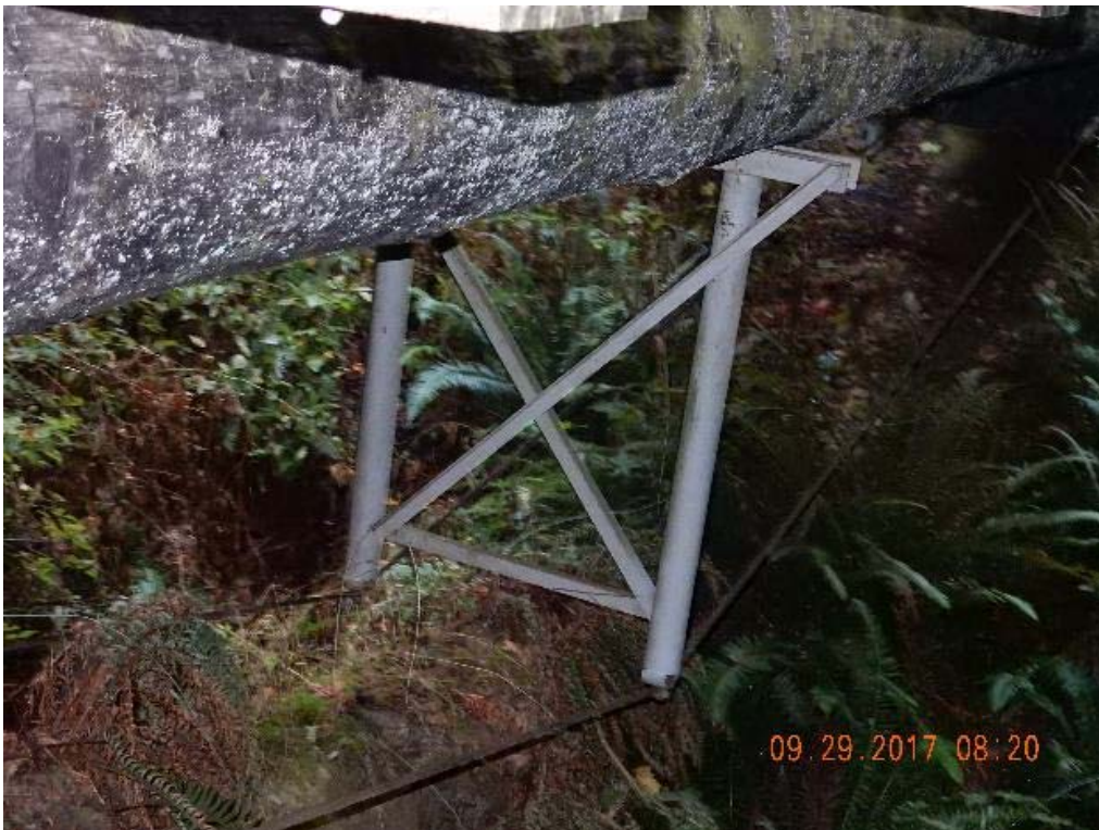
P14 – Middle pier (DSCN9864.jpg)
