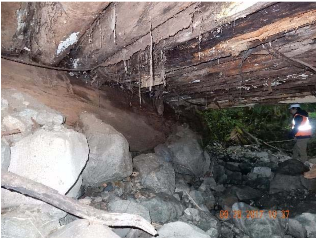
P08 – Under side of the bridge (looking at south abutment) (DSCN9940.jpg)
