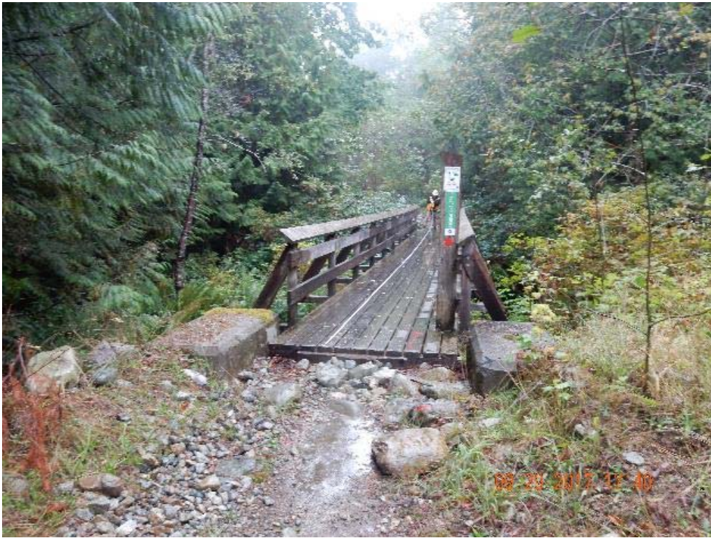
P01 – South approach (DSCN0011.jpg)
