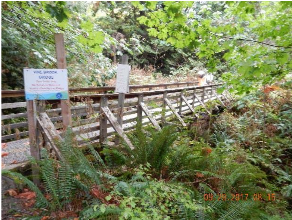
P09 – West side of the bridge (DSCN9855.jpg)
