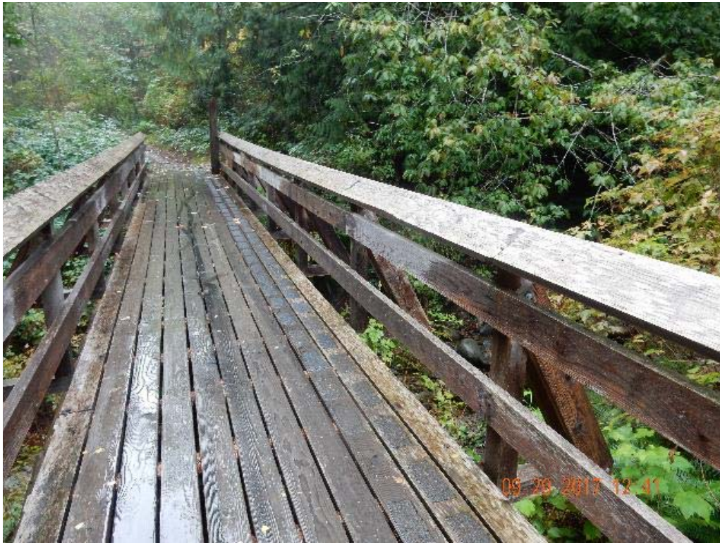
P05 – East railing (DSCN0020.jpg)
