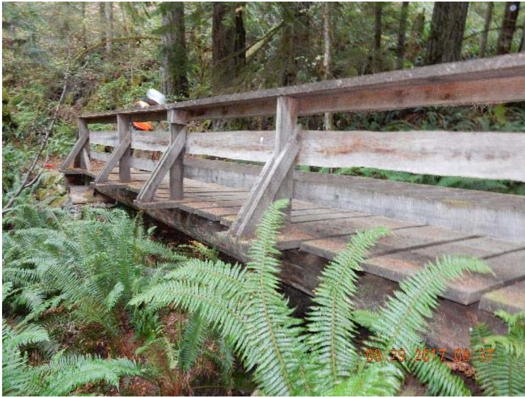
P05 – West side of the bridge (DSCN9876.jpg)
