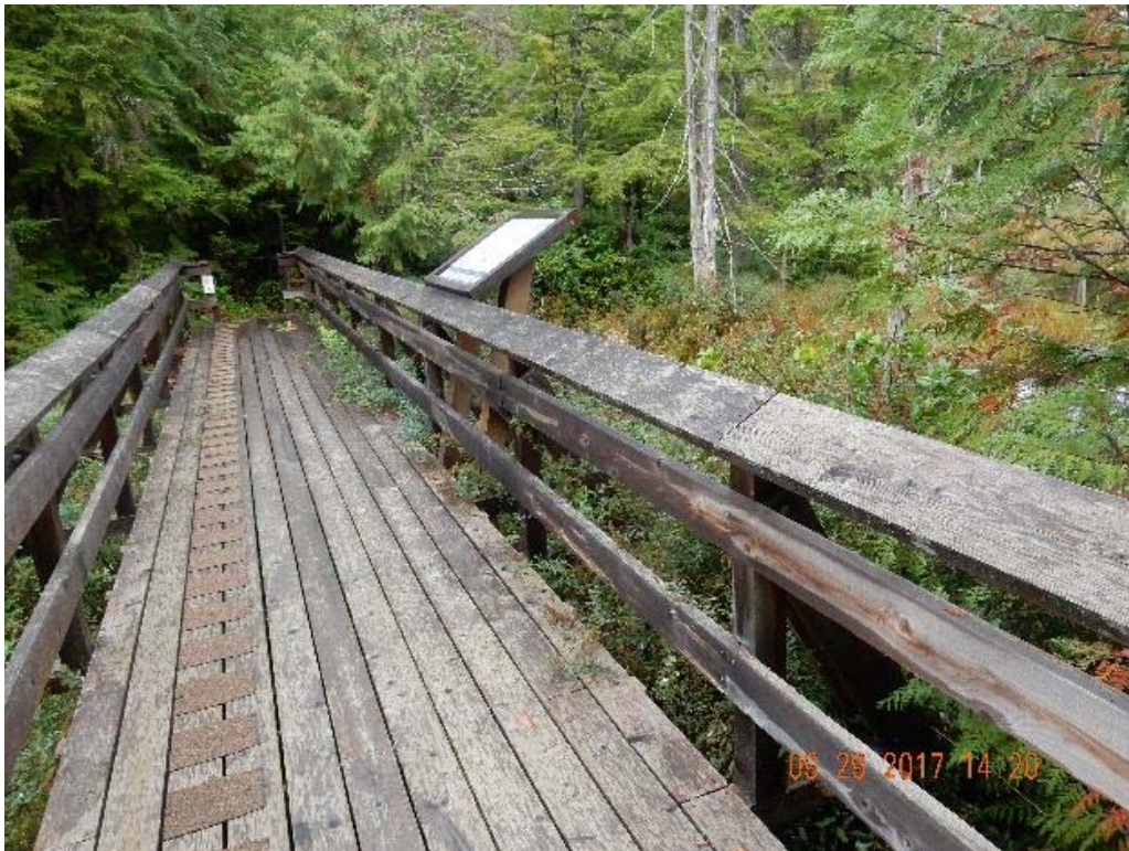
P04 – East railing (DSCN0034.jpg)
