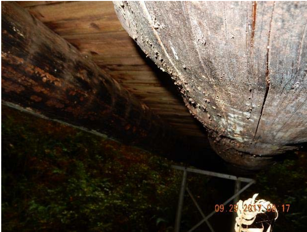
P13 – Under side of the bridge (DSCN9863.jpg)
