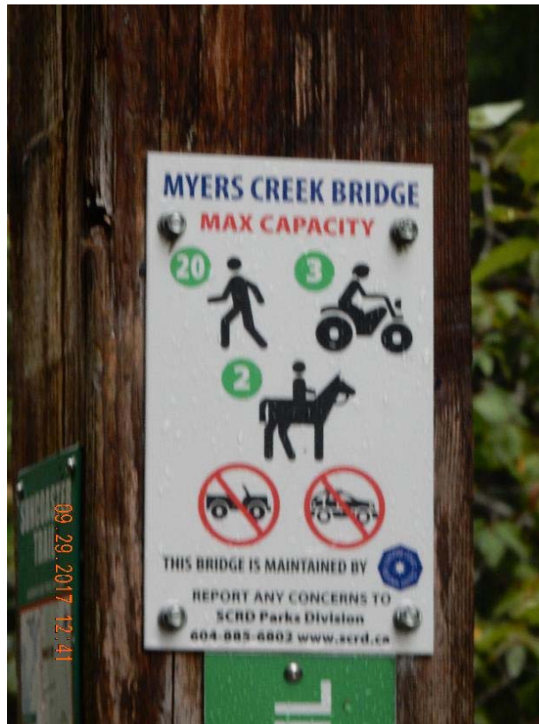
P03 – Loading rating sign at the southeast corner of the bridge (DSCN0014. jpg)
