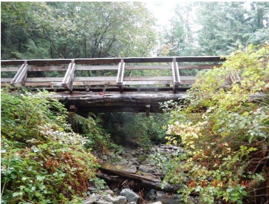
P12 – West side of the bridge (DSCN0029.jpg)
