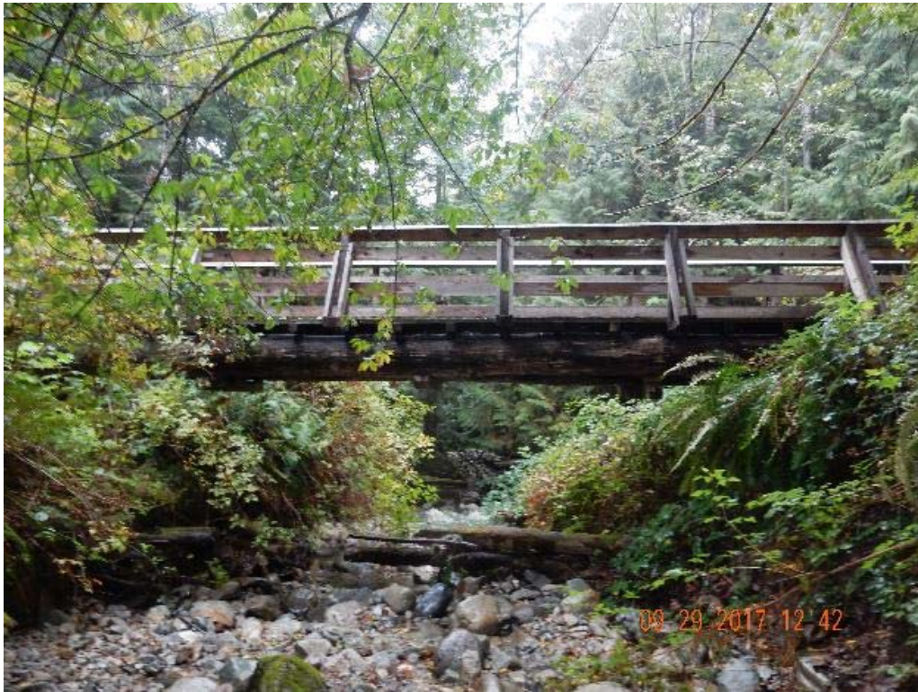
P09 – East side of the bridge (DSCN0025.jpg)
