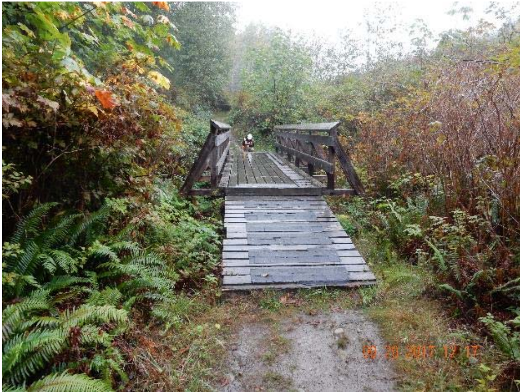
P07 – South approach (DSCN9988.jpg)
