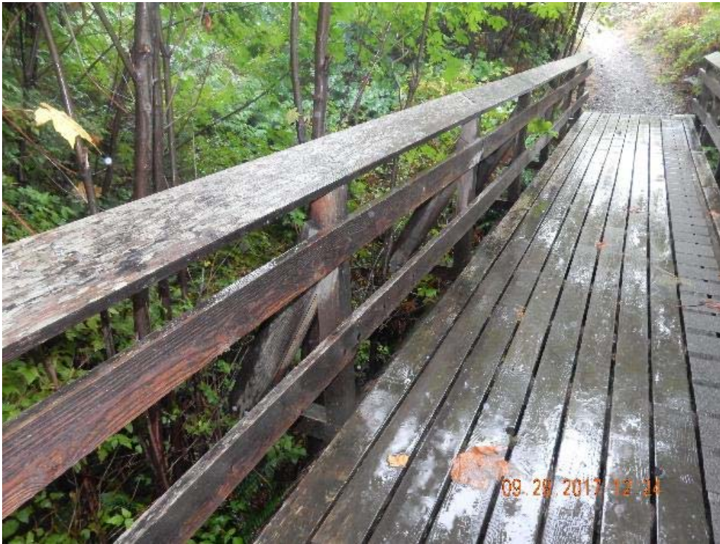
P03 – East railing (DSCN0001.jpg)
