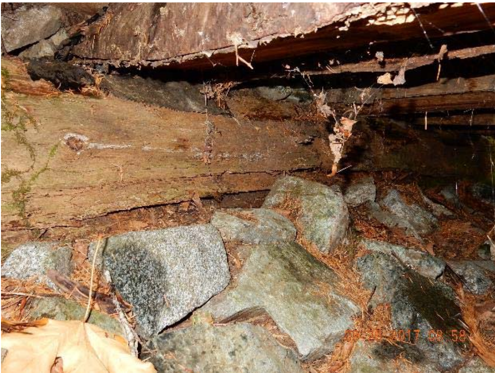
P08 – South abutment (DSCN9902.jpg)
