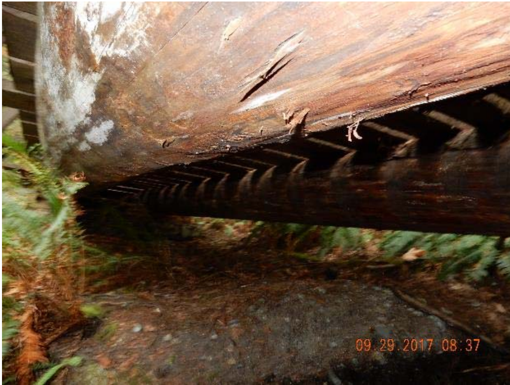
P07 – Under side of the bridge (DSCN9878.jpg)
