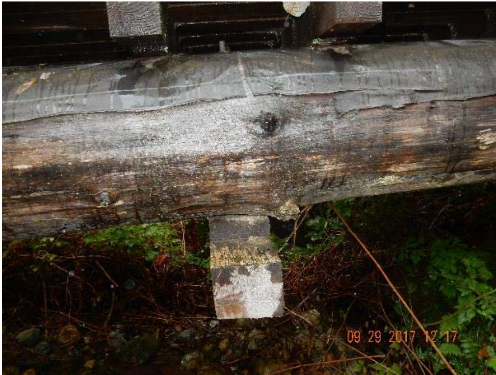
P09 – East side of the bridge (detail view) (DSCN9990.jpg)
