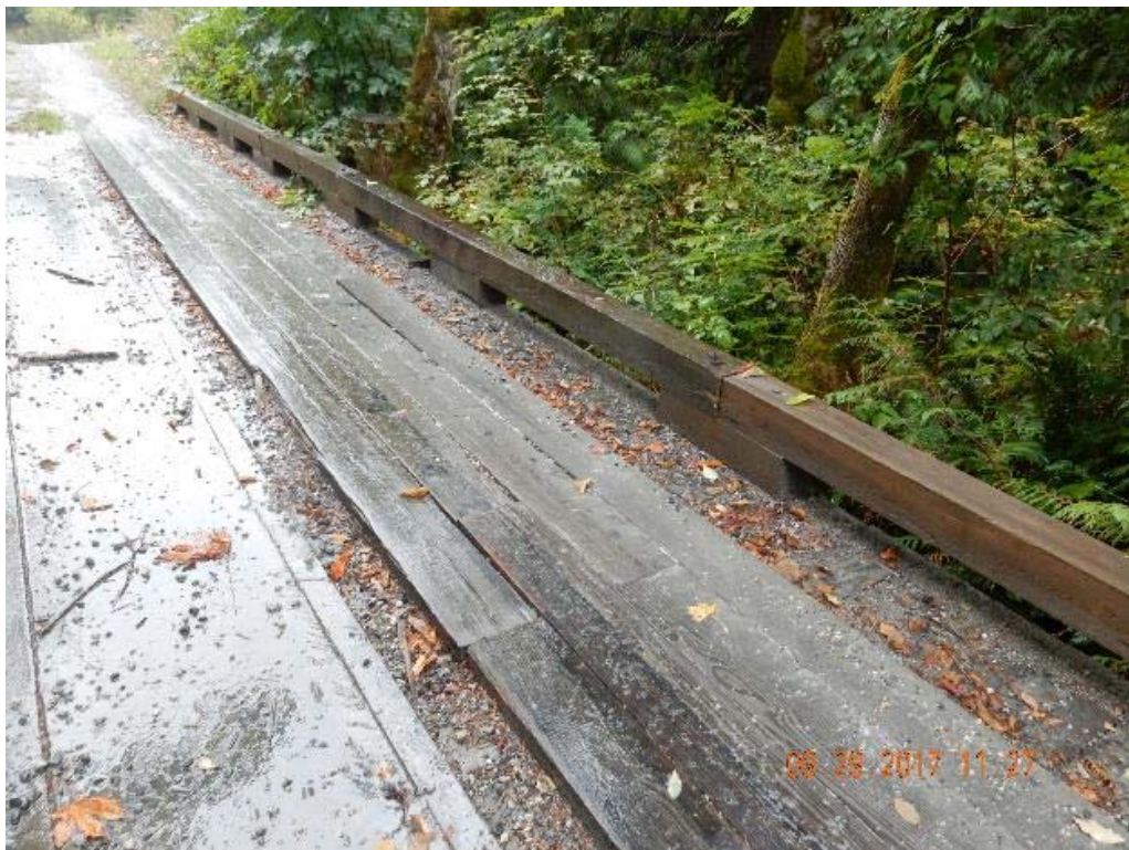
P04 – West curb (DSCN9956.jpg)
