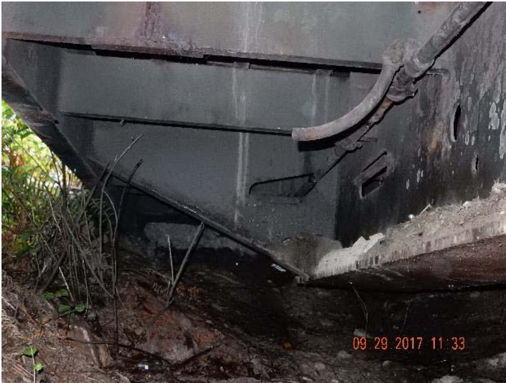
P15 – East side of the bridge, looking at south abutment (DSCN9970.jpg)
