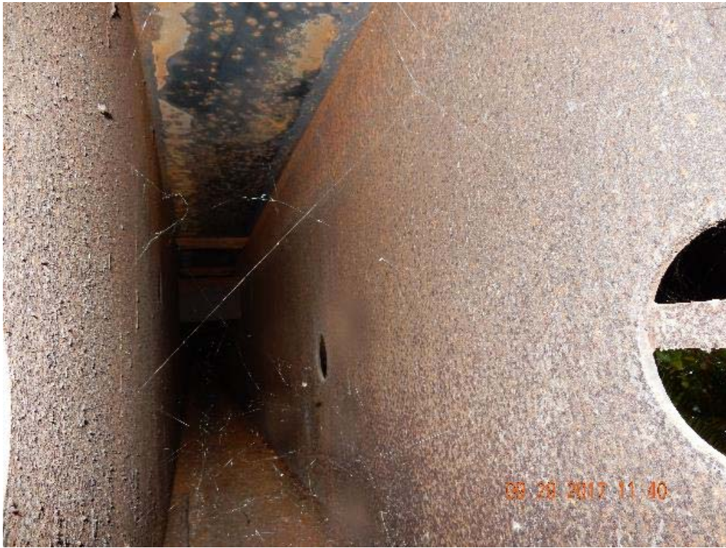
P17 – Looking inside of the main box girder (DSCN9975.jpg)
