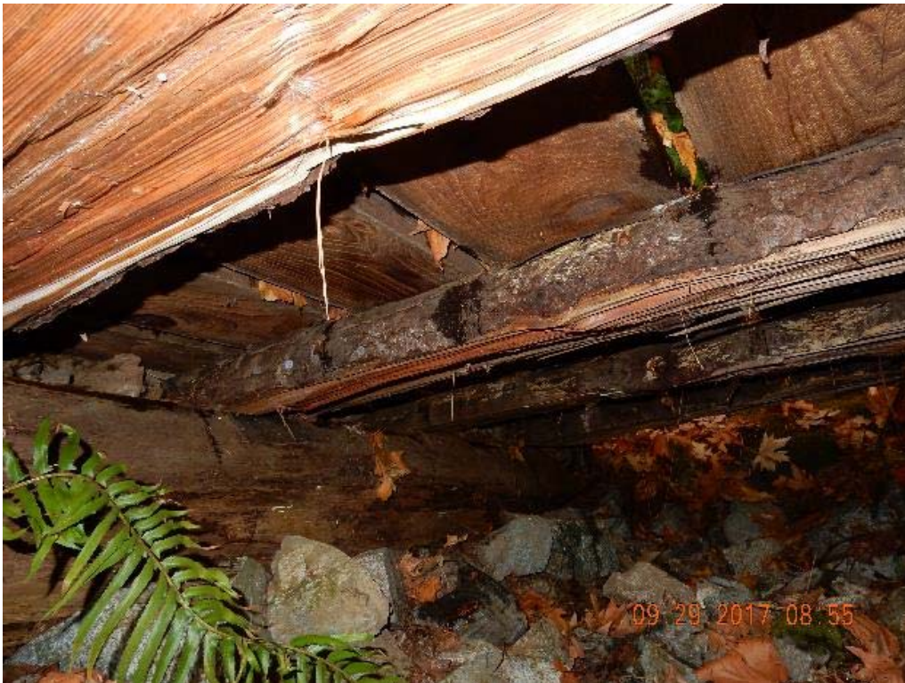
P06 – Under side of the bridge (DSCN9890.jpg)
