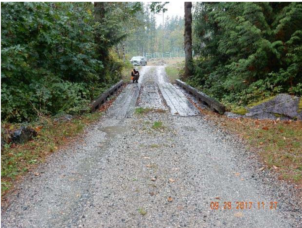
P06 – South approach (DSCN9960.jpg)
