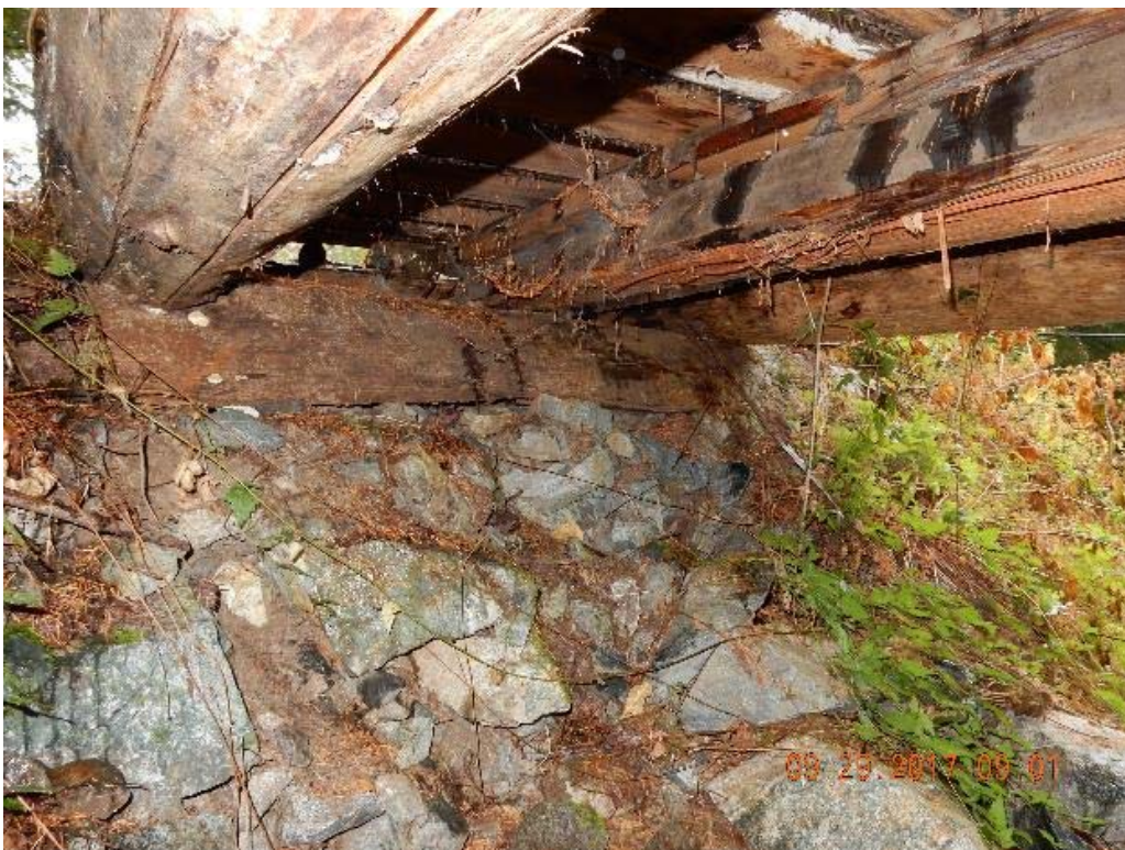
P06 – South abutment (DSCN9911.jpg)
