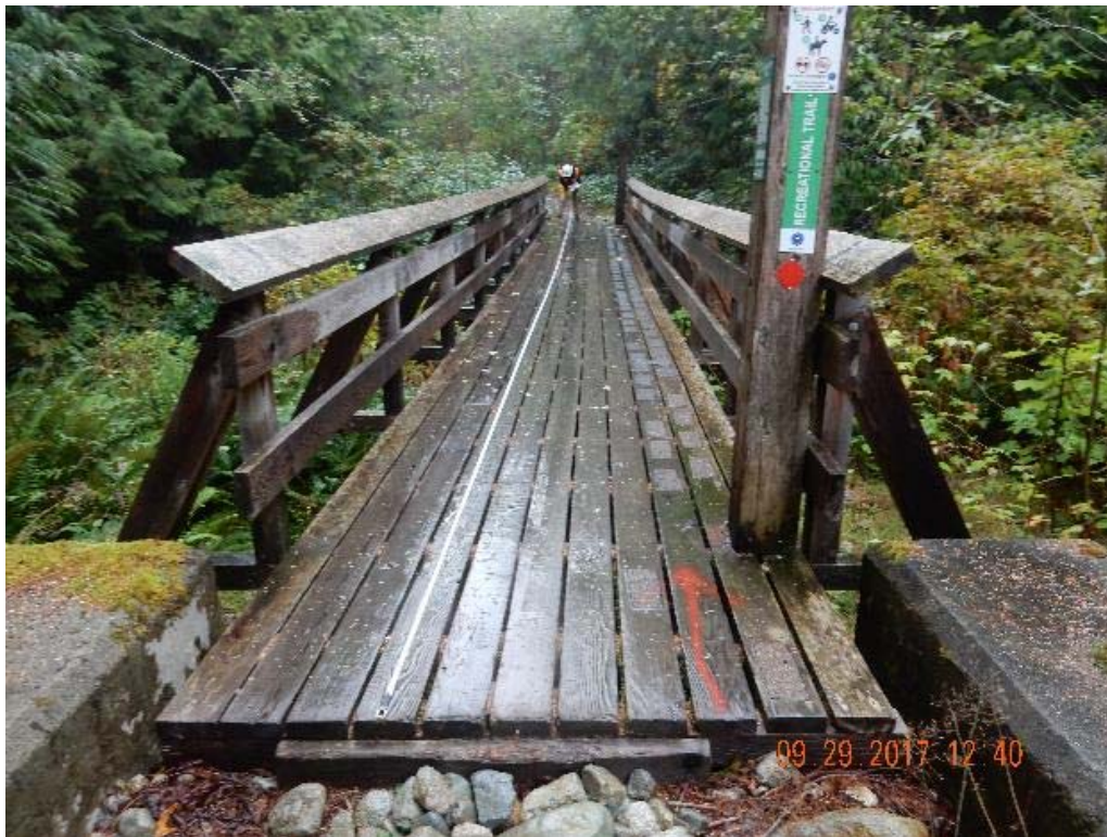
P02 – South end of the bridge (DSCN0012.jpg)
