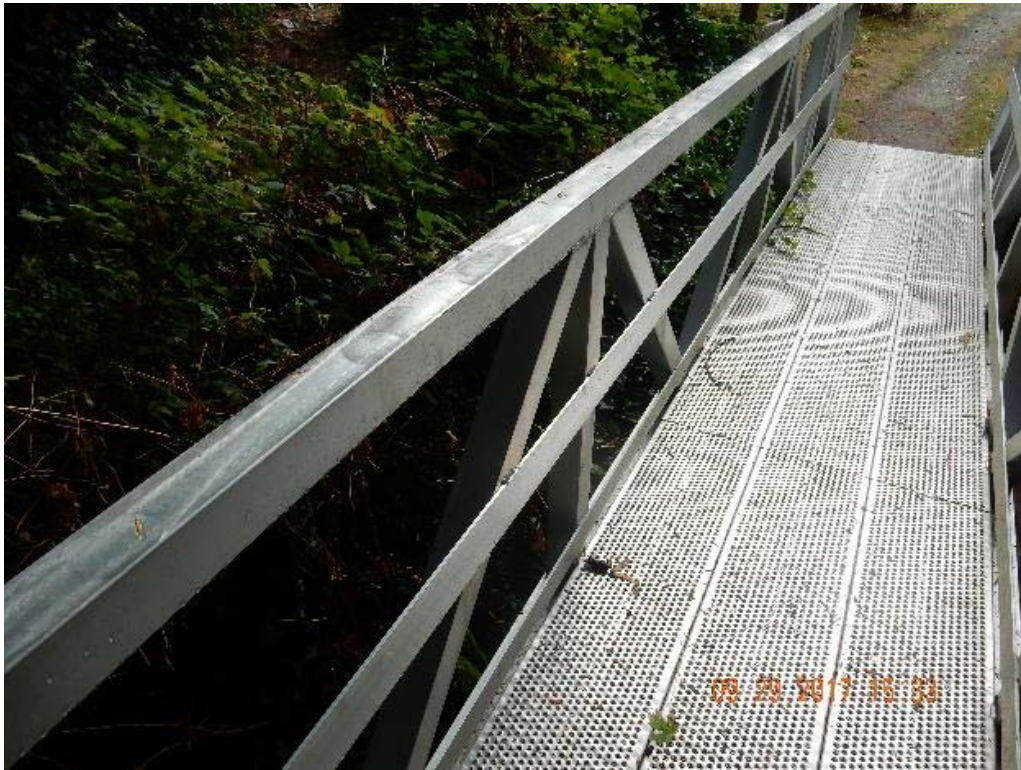
P05 – East railing (DSCN0068.jpg)
