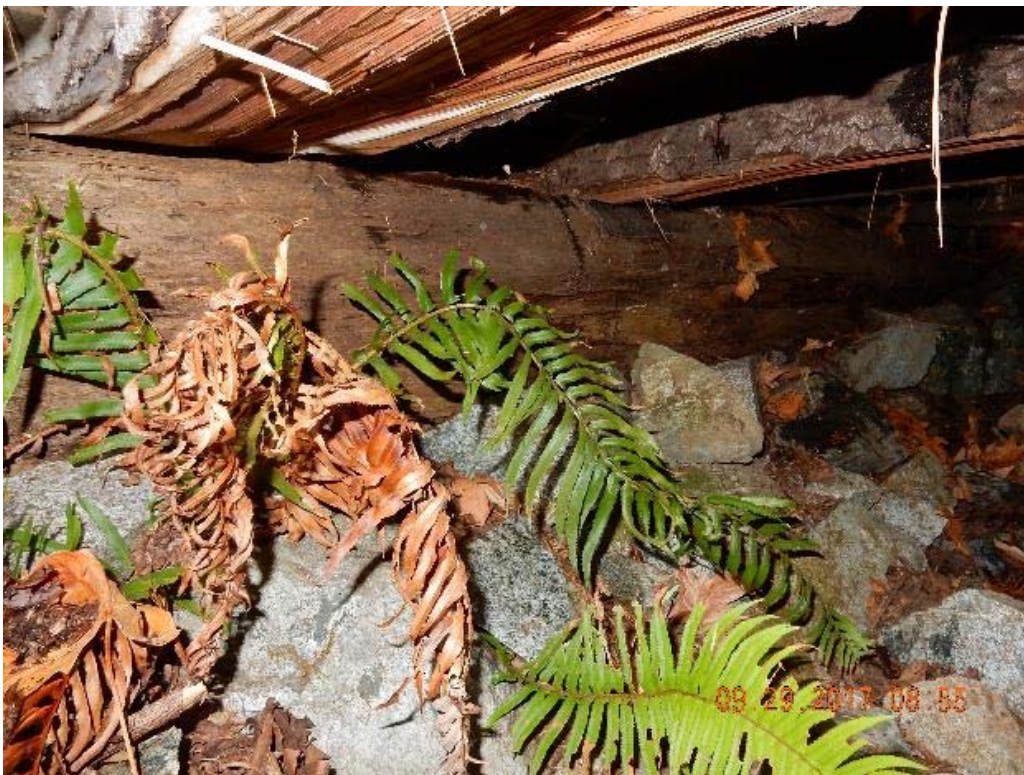
P08 – North abutment (DSCN9892.jpg)
