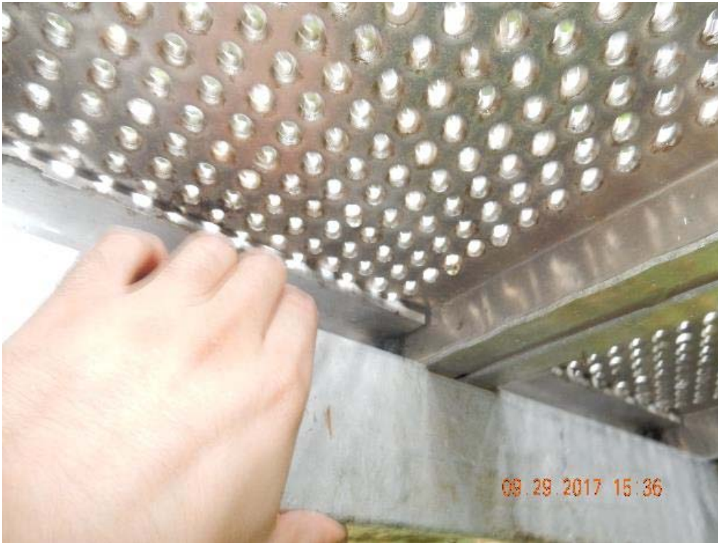
P15 – Detail view of the stringer (DSCN0080.jpg)
