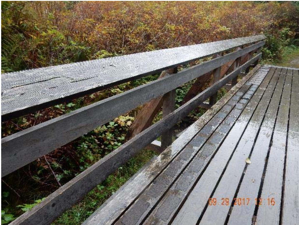
P03 – East railing (DSCN9984.jpg)
