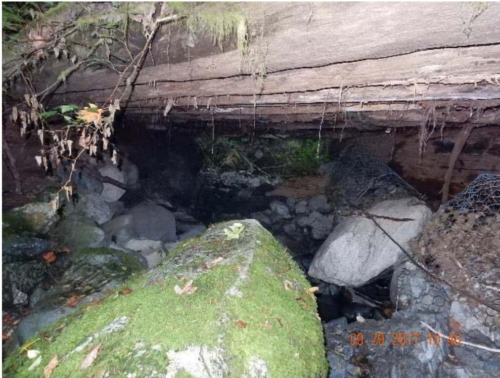
P11 – East side of the bridge (DSCN9948.jpg)
