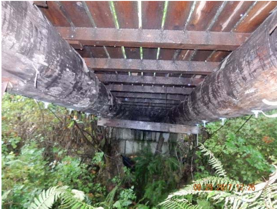
P09 – Under side of the bridge (looking north) (DSCN0007.jpg)
