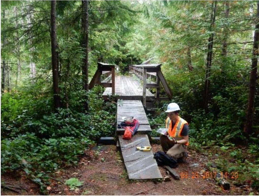
P01 – South approach (DSCN0031.jpg)
