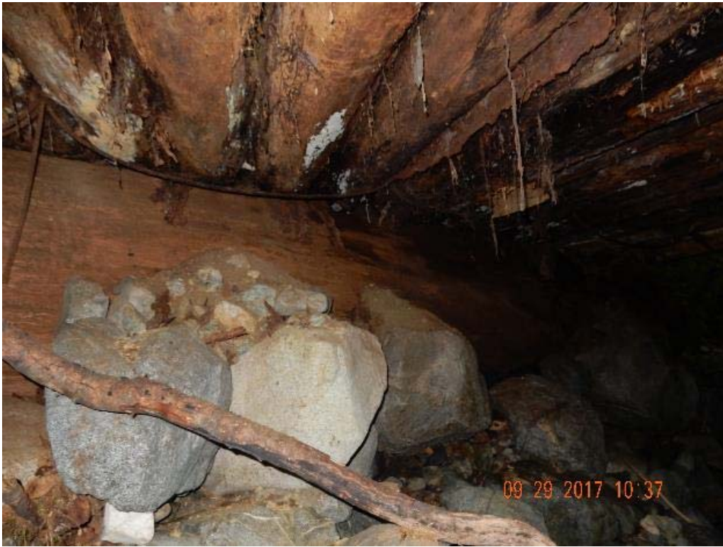
P07 – South abutment (DSCN9939.jpg)
