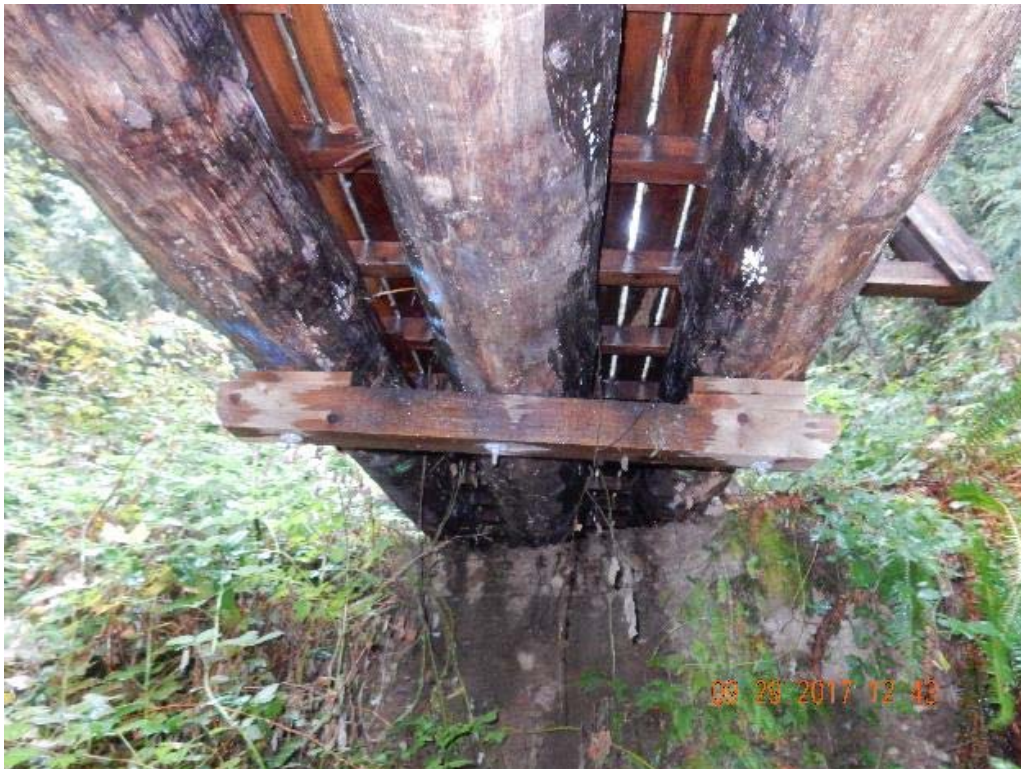
P10 – North embankment (DSCN00026.jpg)
