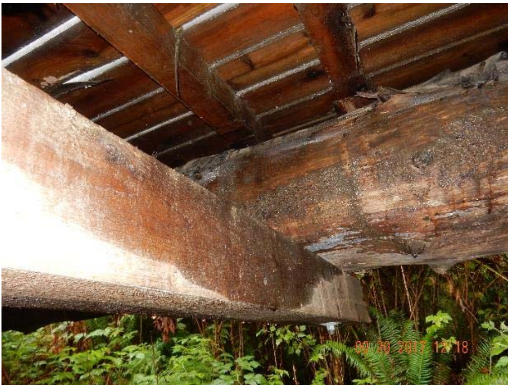
P12 – Under side of the bridge (detail view) (DSCN9994.jpg)
