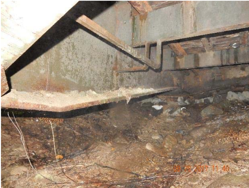
P19 – West side of the bridge (looking at south abutment) (DSCN9978.jpg)
