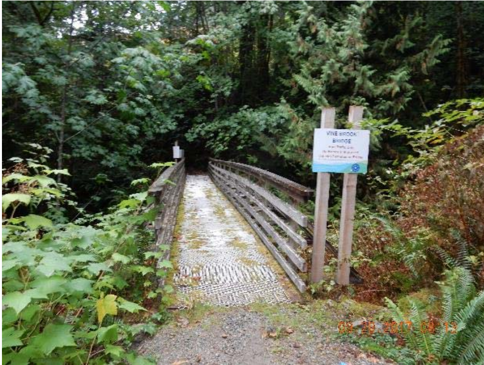
P01 – South approach (DSCN9844.jpg)
