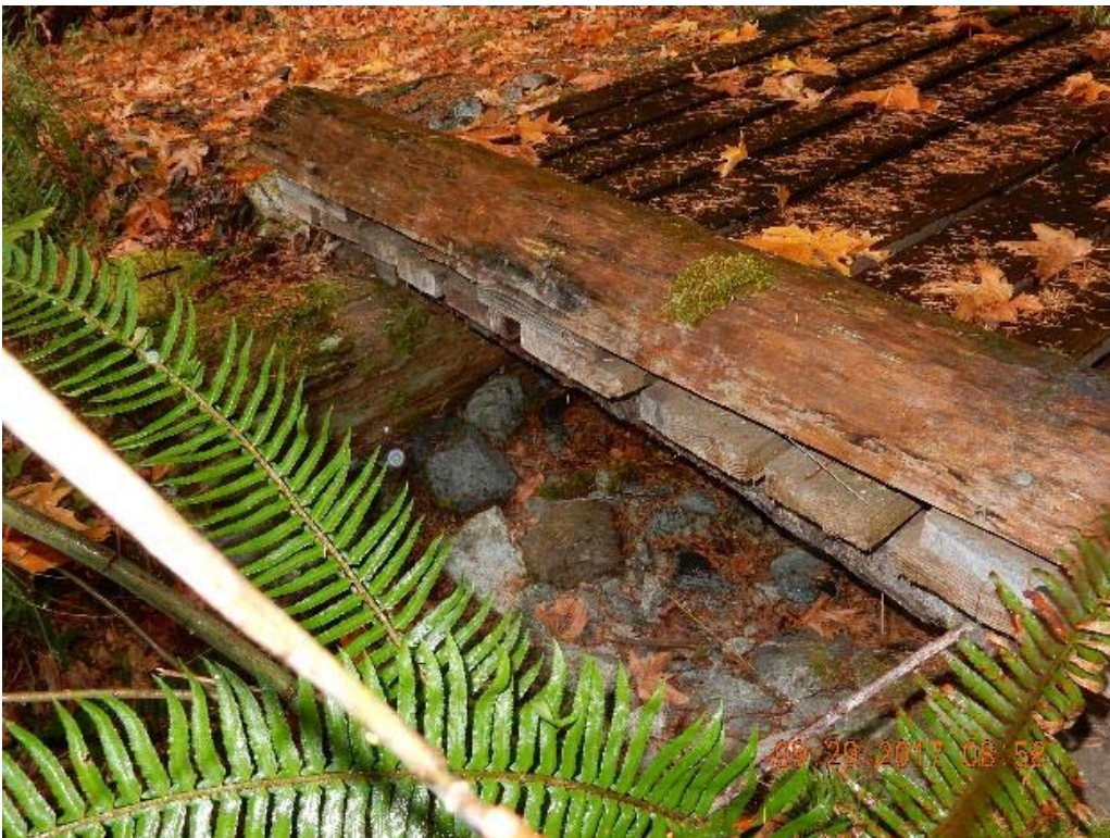
P06 – West side of the bridge (DSCN9900.jpg)
