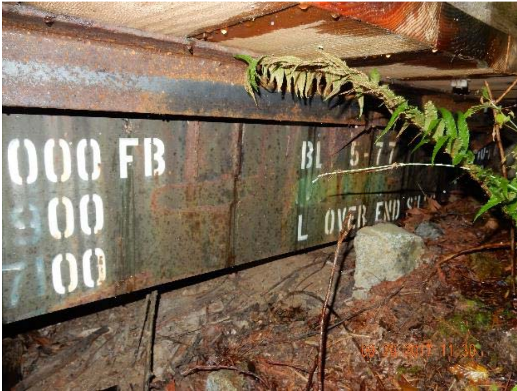
P07 – Side view of the main C-Channel (DSCN9961.jpg)
