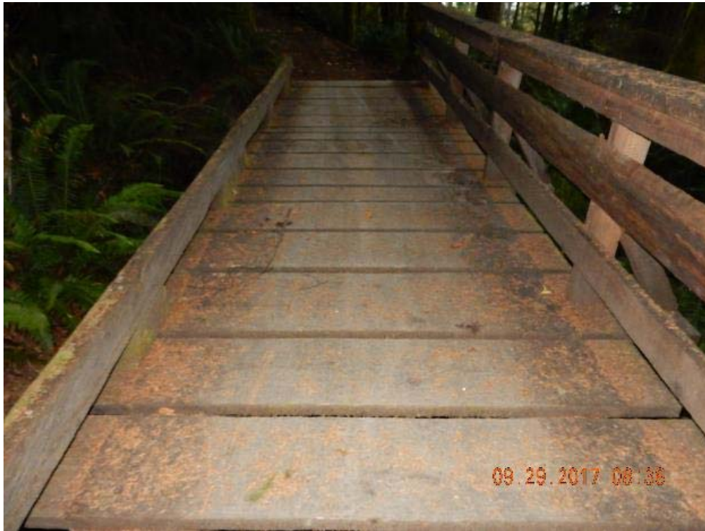
P03 – Overall decking (DSCN9872.jpg)
