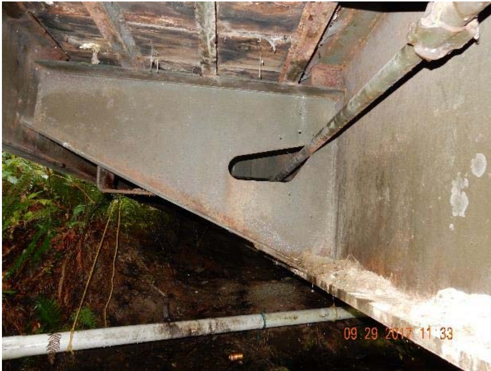
P13 – East side of the bridge, looking at triangular diaphragm (DSCN9968.jpg)
