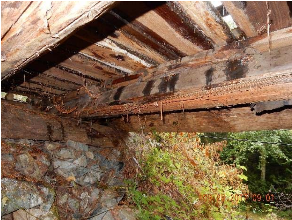
P08 – Under side of the bridge (DSCN9913.jpg)
