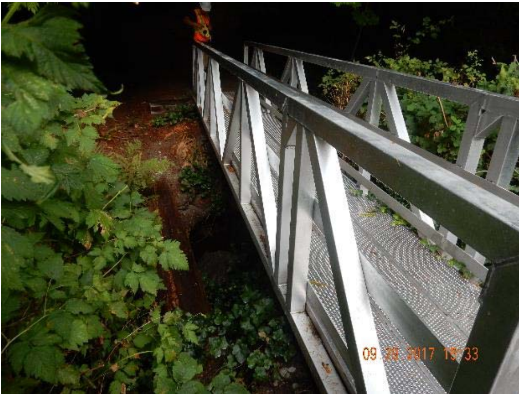
P10 – West side of the bridge (DSCN0073.jpg)
