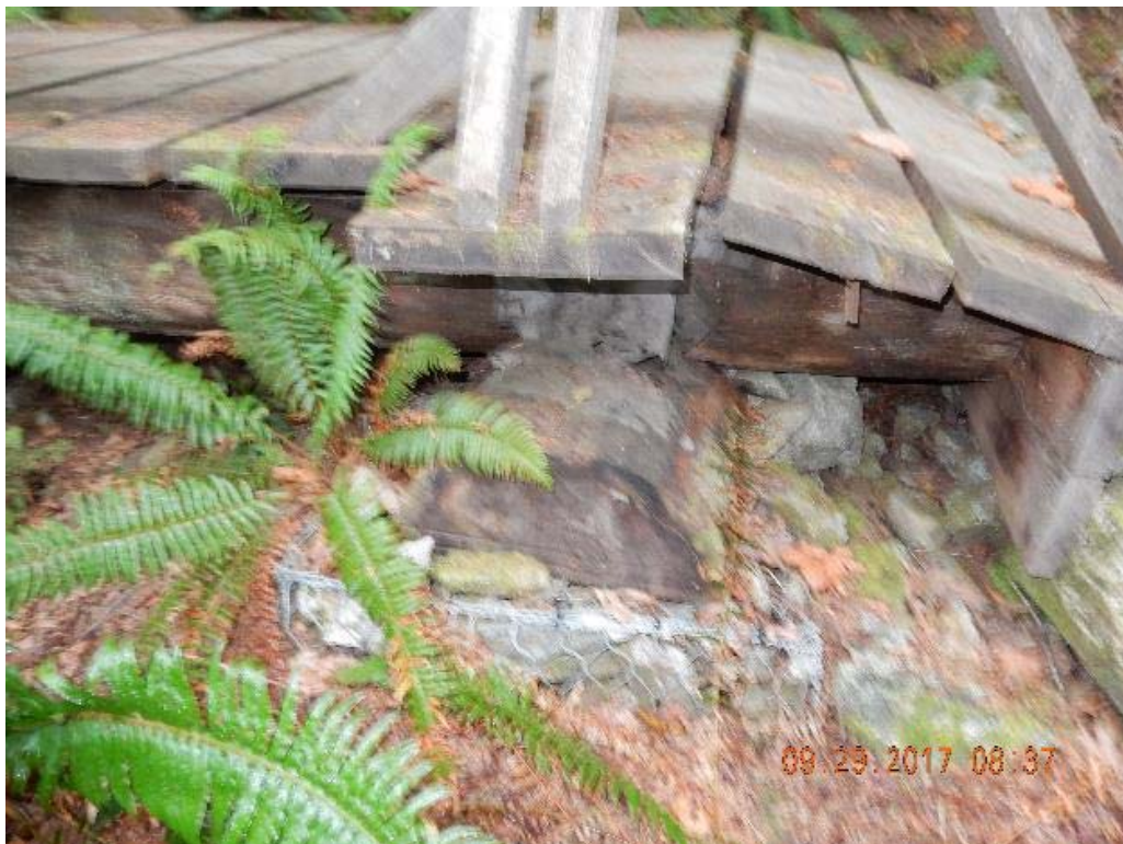
P06 – South abutment (DSCN9877.jpg)
