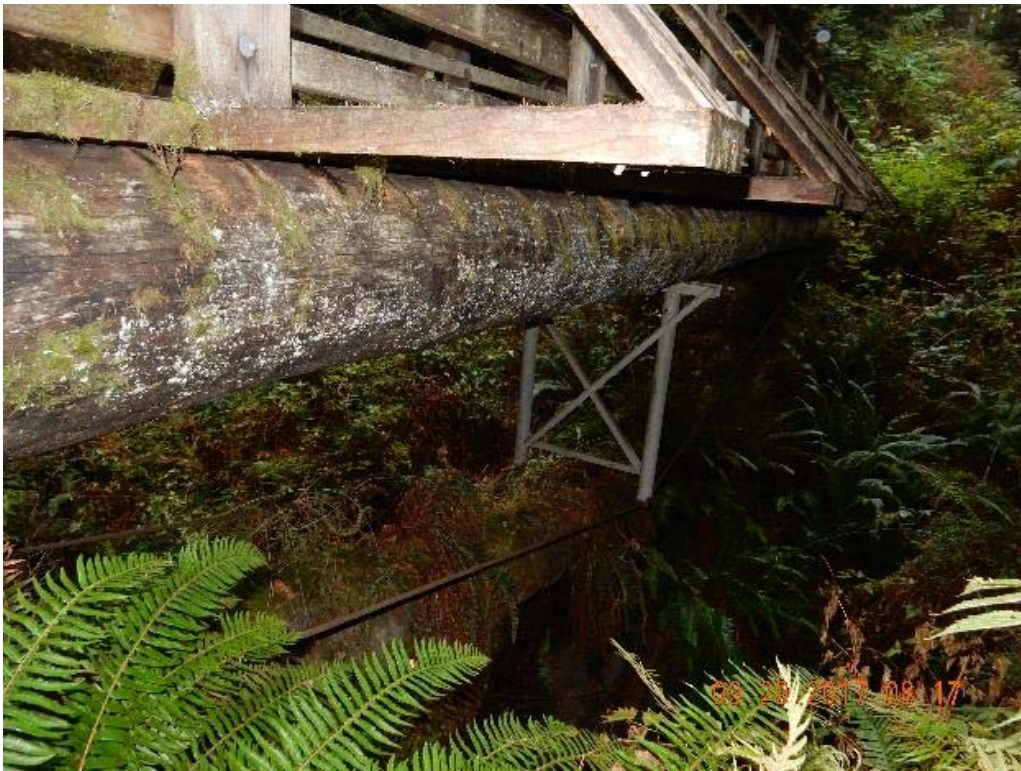
P12 – West side of the bridge (looking at middle pier) (DSCN9860.jpg)
