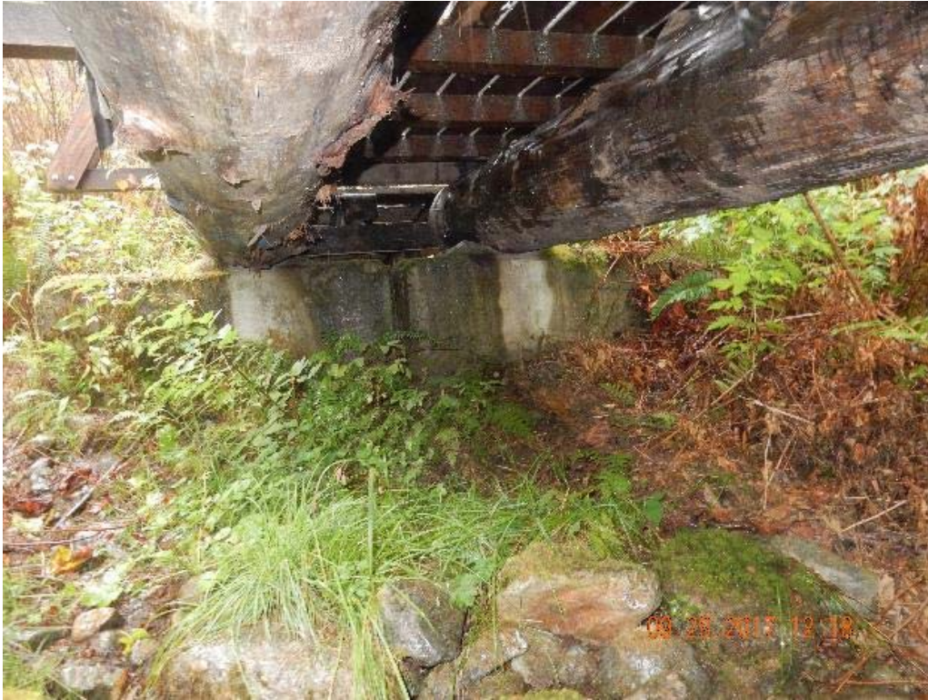
P11 – South abutment (DSCN9993.jpg)
