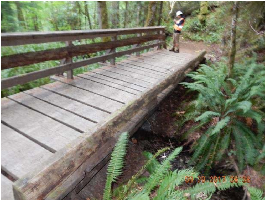
P09 – East side of the bridge (DSCN9880.jpg)
