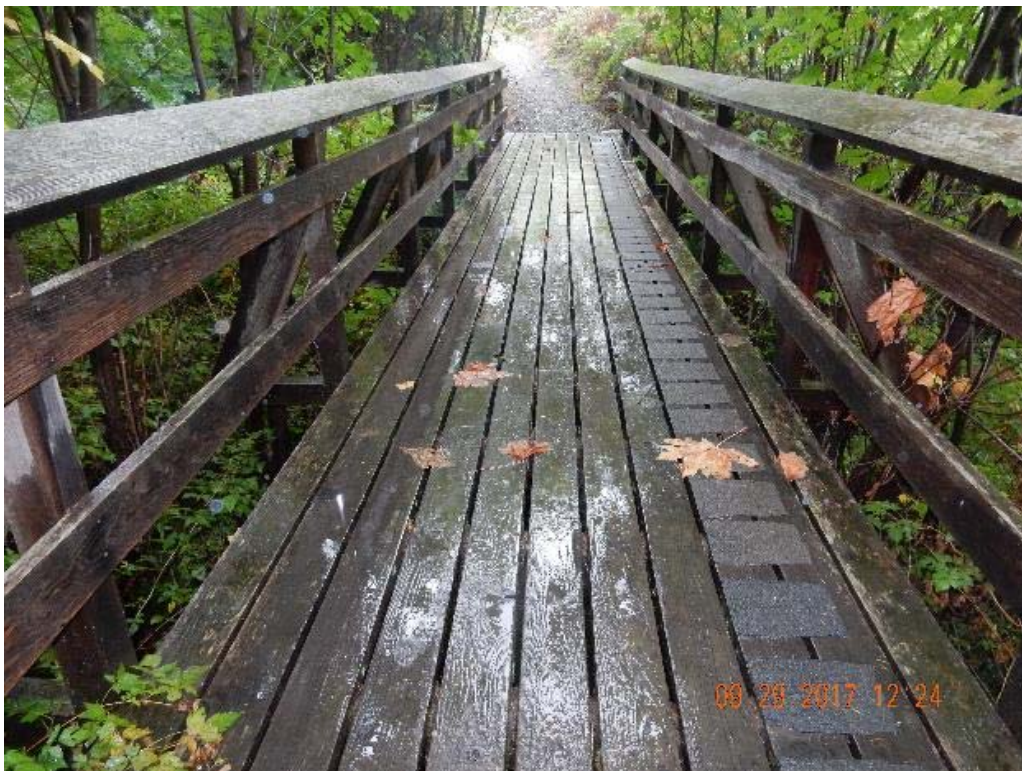
P02 – Overall decking (DSCN9999.jpg)
