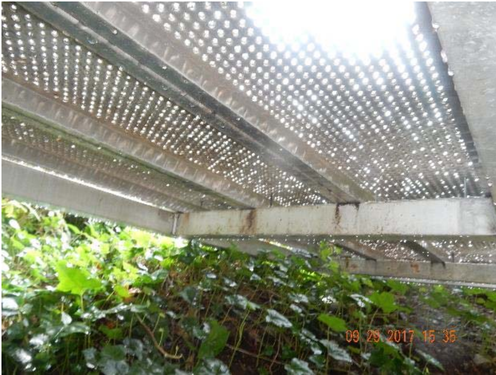
P13 – Under side of the bridge (DSCN0077.jpg)
