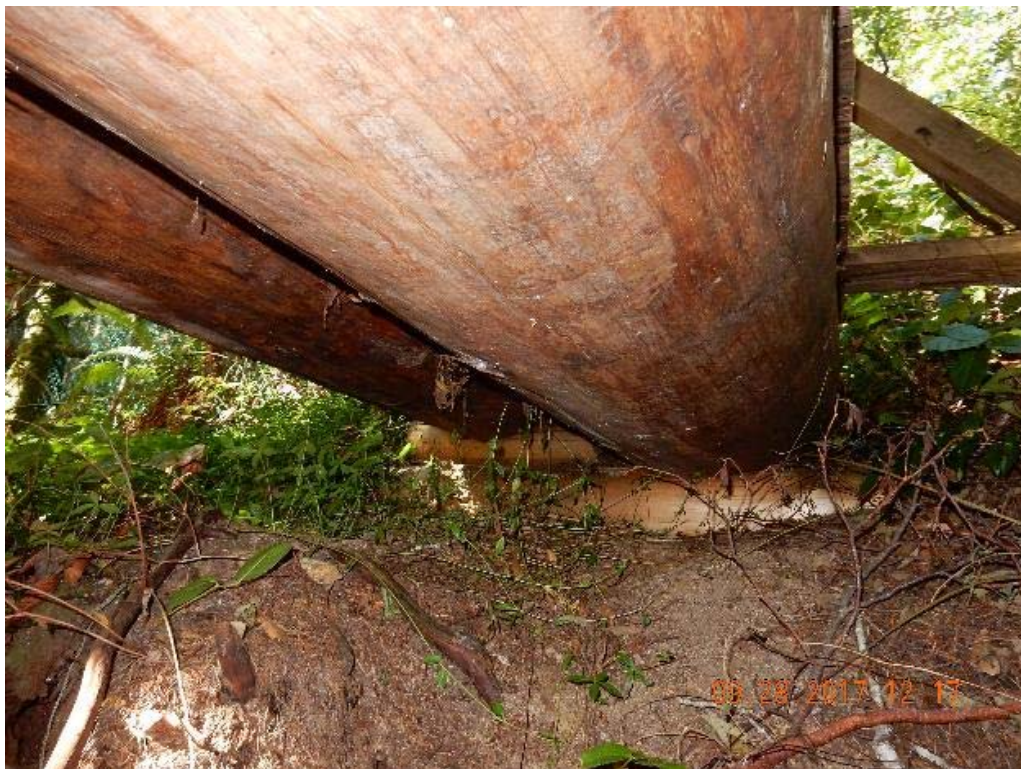
P08 – North abutment (DSCN9529.jpg)
