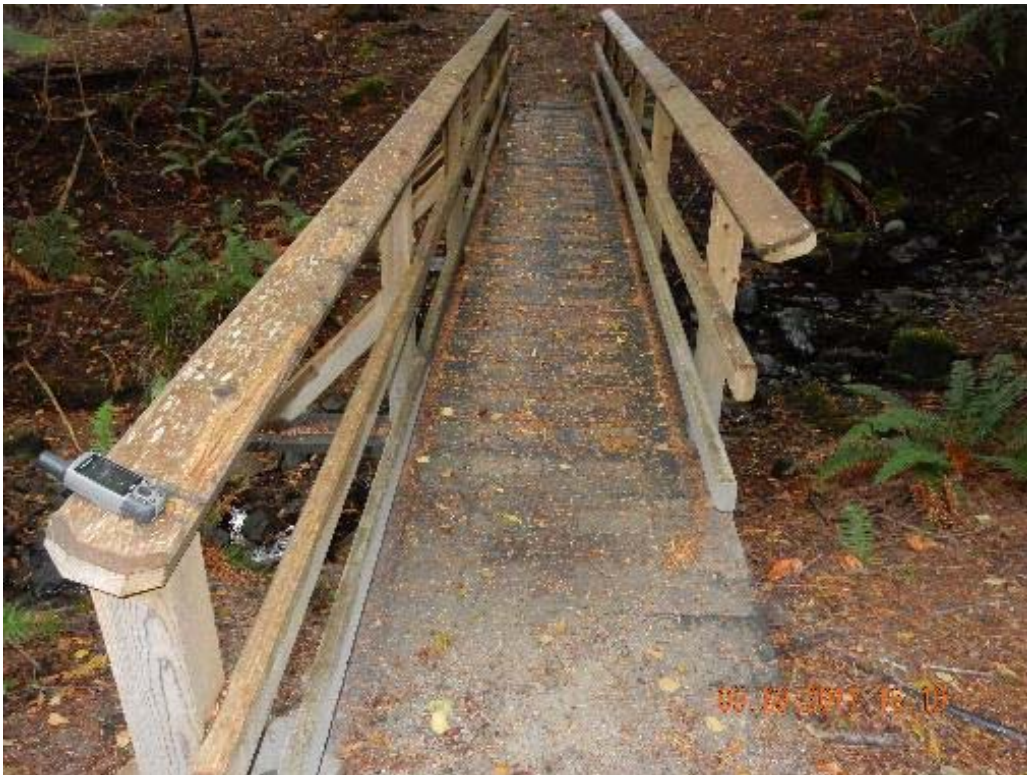
P02 – North end of the bridge (DSCN0085.jpg)
