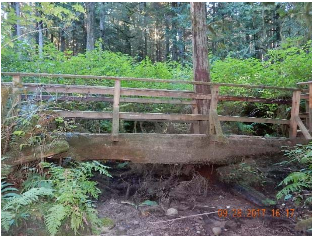
P06 – South side of the bridge (west span) (DSCN9699.jpg)
