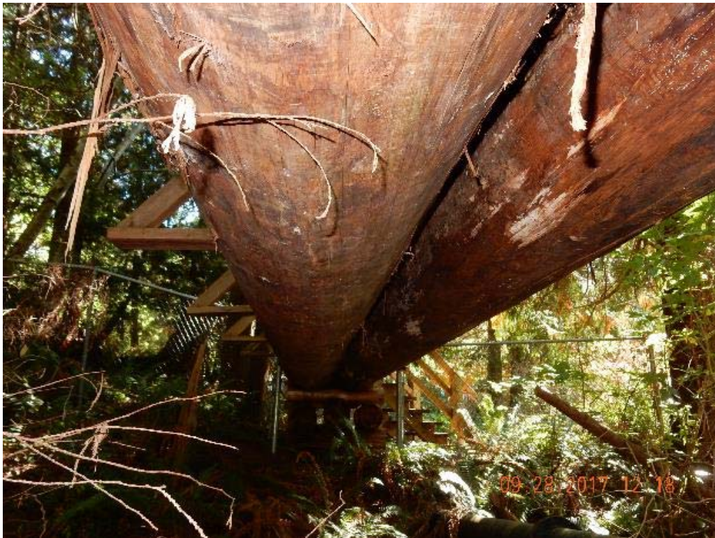
P10 – Under side of the bridge (DSCN9533.jpg)
