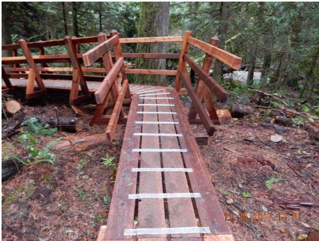
P02 – West Approach (DSCN0688.jpg)
