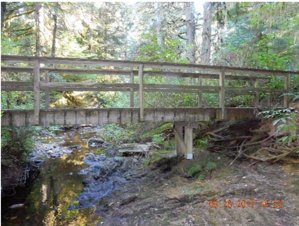
P10 – North side of the bridge (west span) (DSCN9632.jpg)
