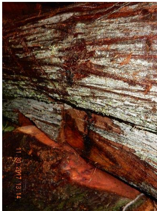
P09 – Rebar driven through main log into abutment (DSCN0692.jpg)
