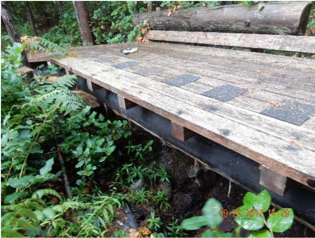
P07 – East side of the bridge (DSCN0056.jpg)
