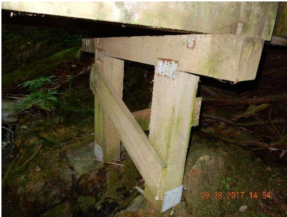
P12 – West span pier 1 (DSCN9634.jpg)
