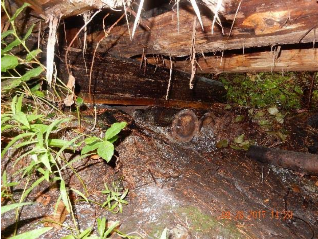
P11 – South abutment (DSCN0058.jpg)
