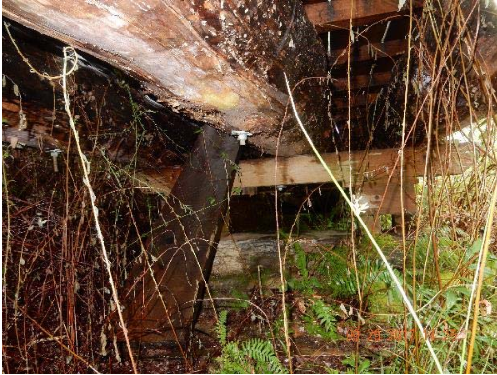
P11 – Middle pier (DSCN0045.jpg)
