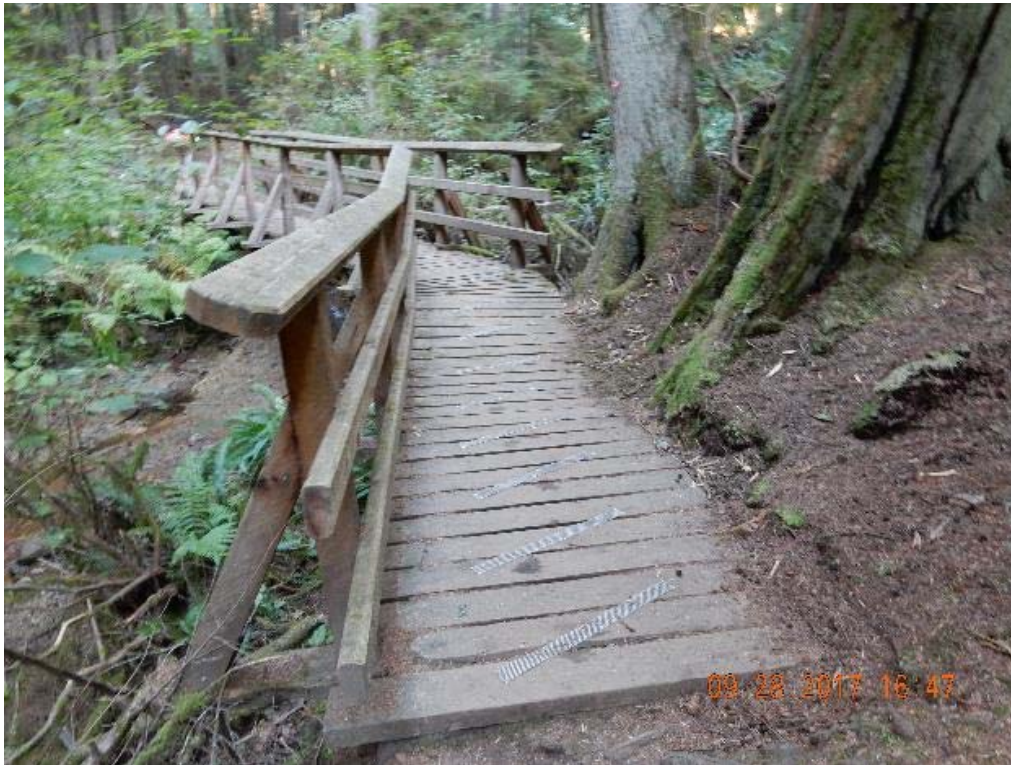
P03 – South approach (DSCN9754.jpg)
