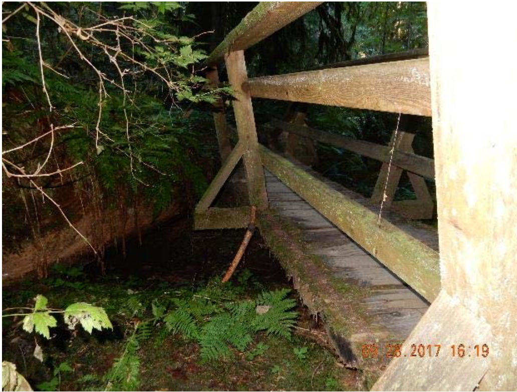
P13 – North side of the bridge (east span) (DSCN9706.jpg)
