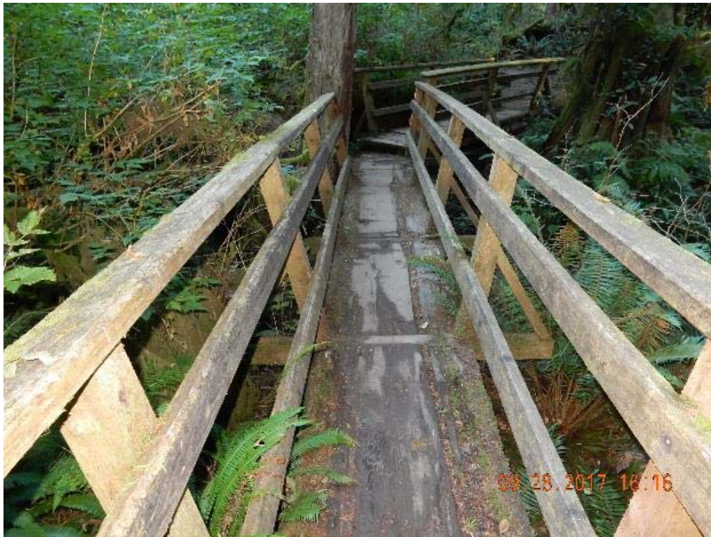
P02 – Overall decking (west span) (DSCN9694.jpg)
