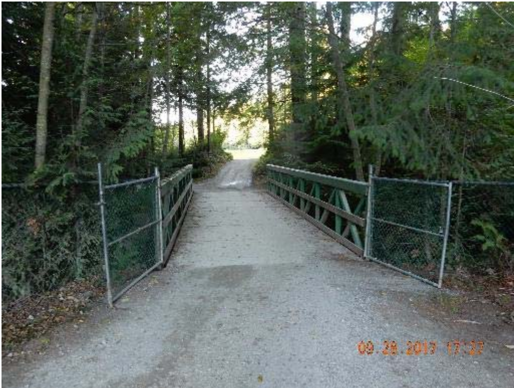
P01 – East approach (DSCN9799.jpg)
