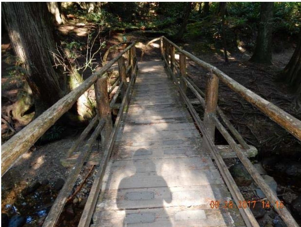
P06 – Overall decking (east span) (DSCN9583.jpg)
