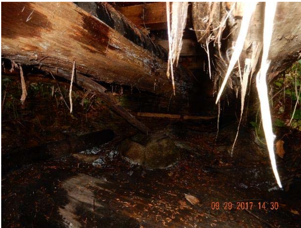
P10 – Under side of the bridge (east and middle log) (DSCN0060.jpg)
