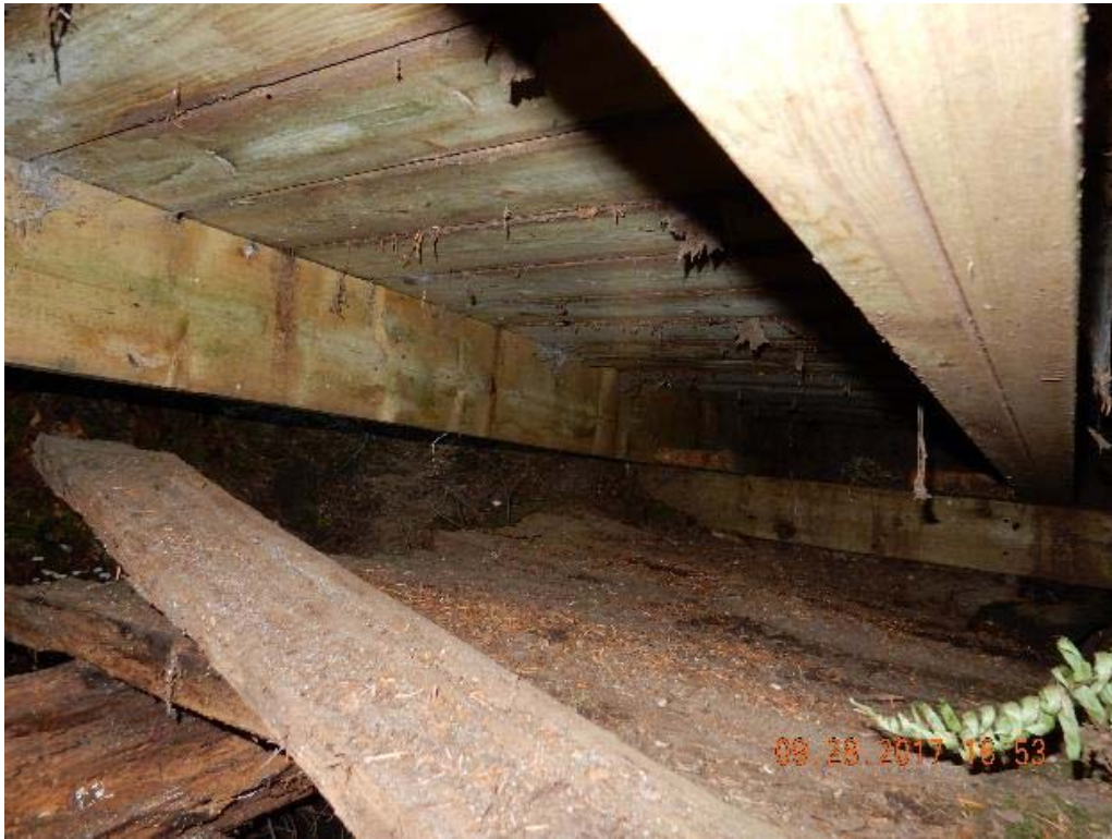
P05 – Under side of the bridge (east abutment) (DSCN9769.jpg)
