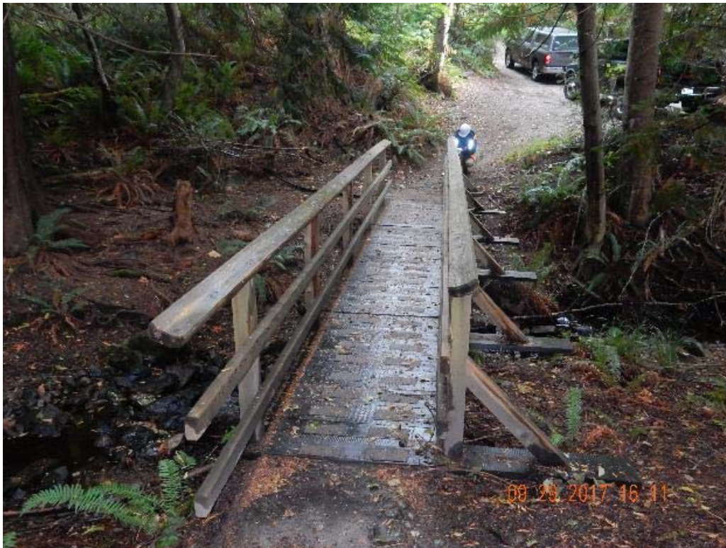
P08 – South approach (DSCN0091.jpg)
