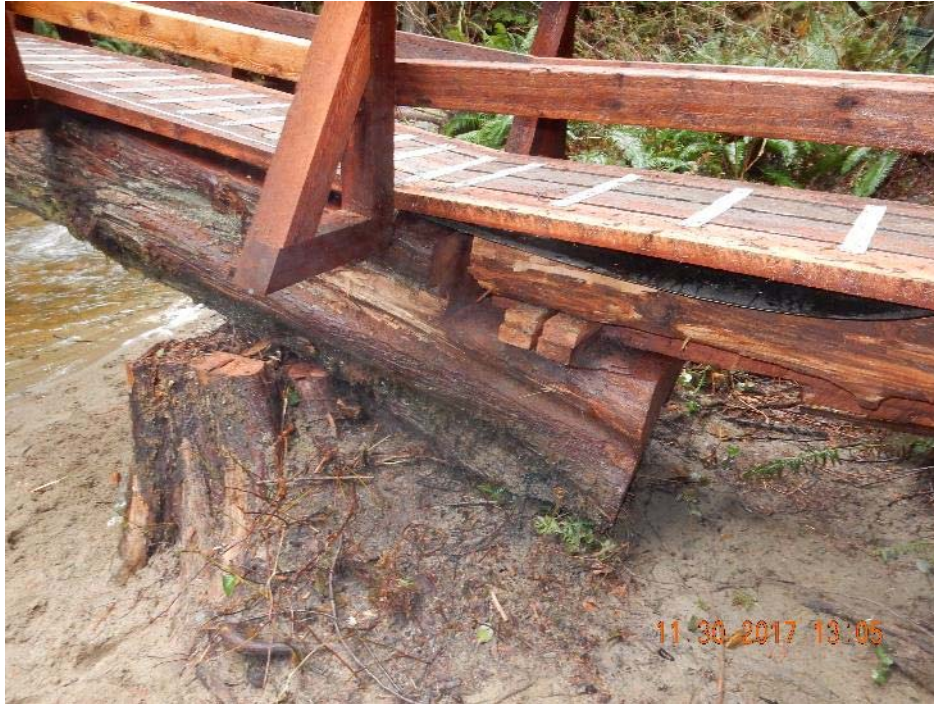
P08 – Main support of bridge (DSCN0667.jpg)
