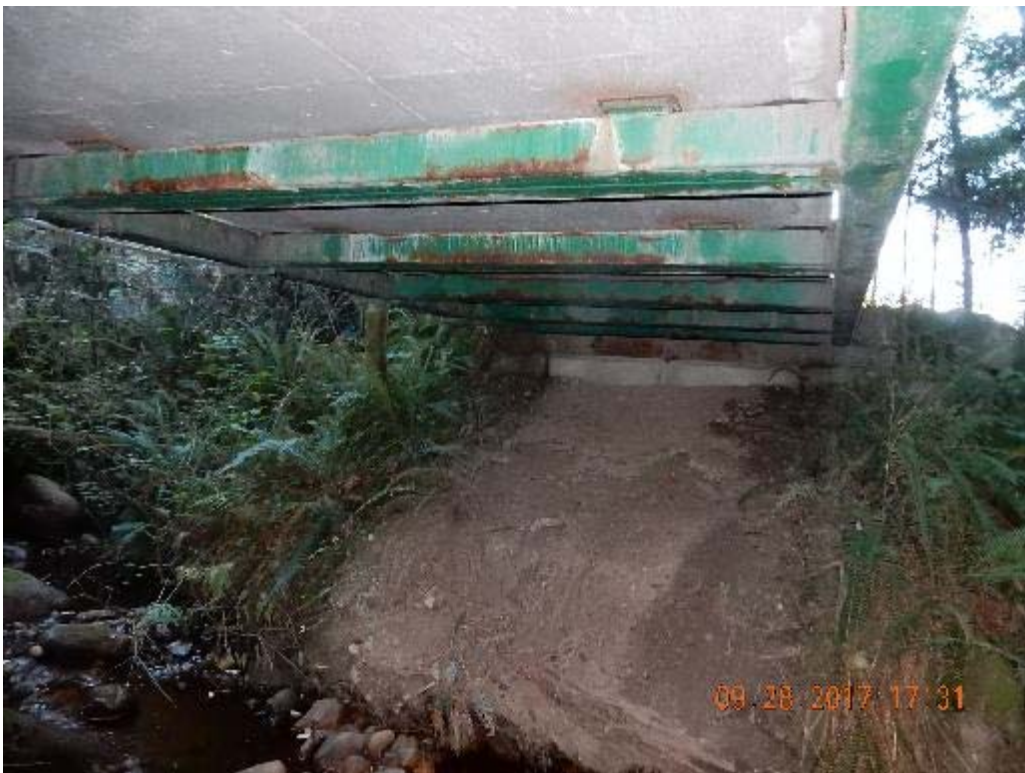
P10 – Under side of the bridge (DSCN9812.jpg)
