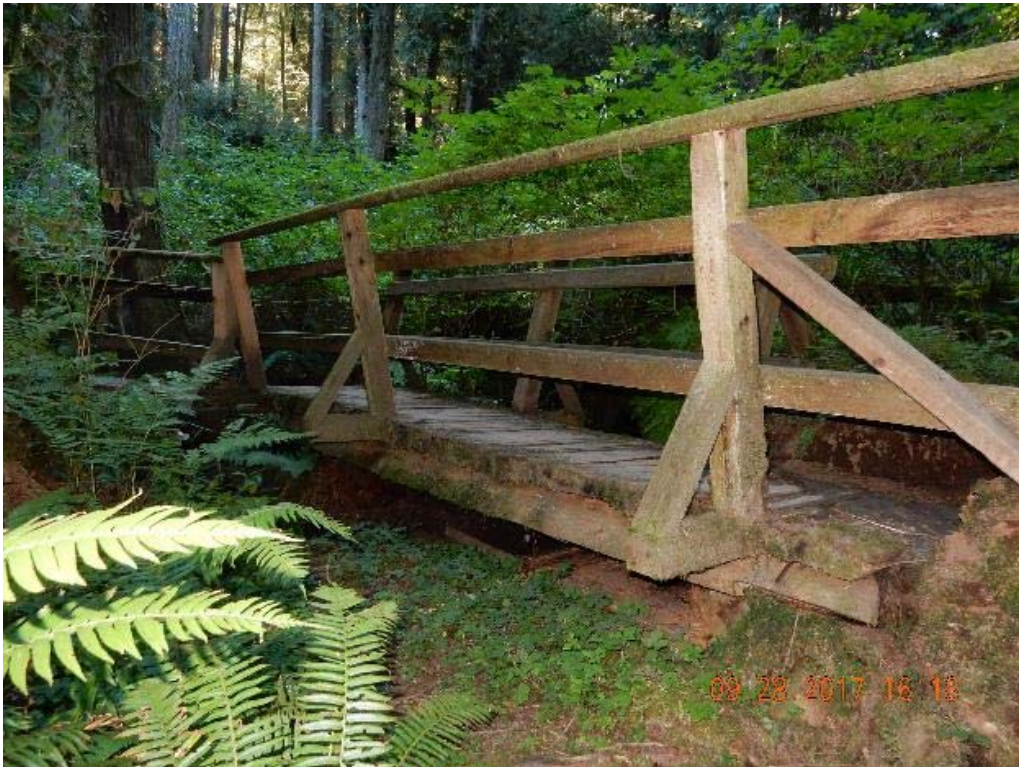
P10 – South side of the bridge (east span) (DSCN9703.jpg)
