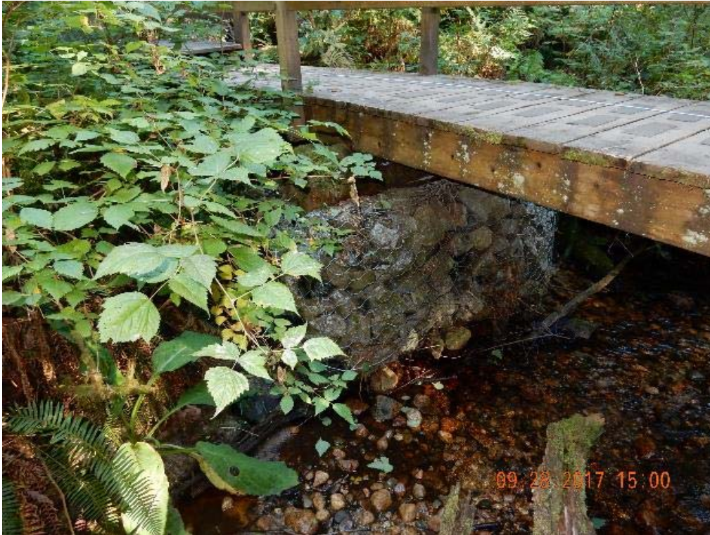
P21 – East abutment (DSCN9646.jpg)
