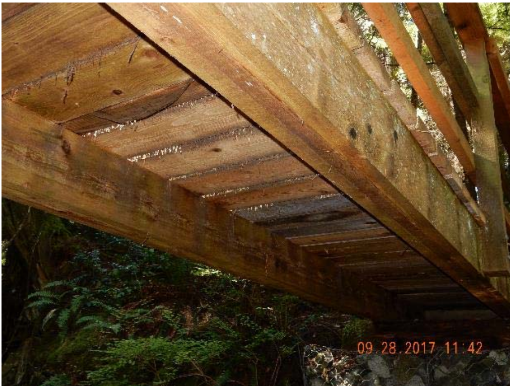
P14 – Under side of the bridge (west span) (DSCN9518.jpg)
