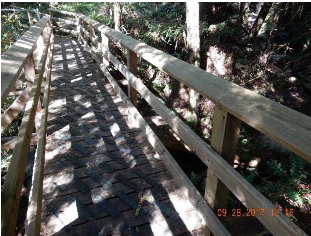
P04 – East railing (DSCN9525.jpg)
