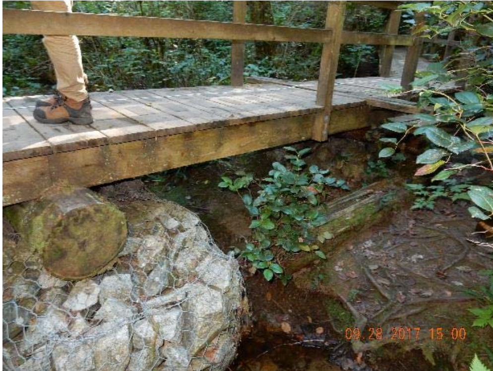
P19 – North side of the bridge (east span) (DSCN9644.jpg)
