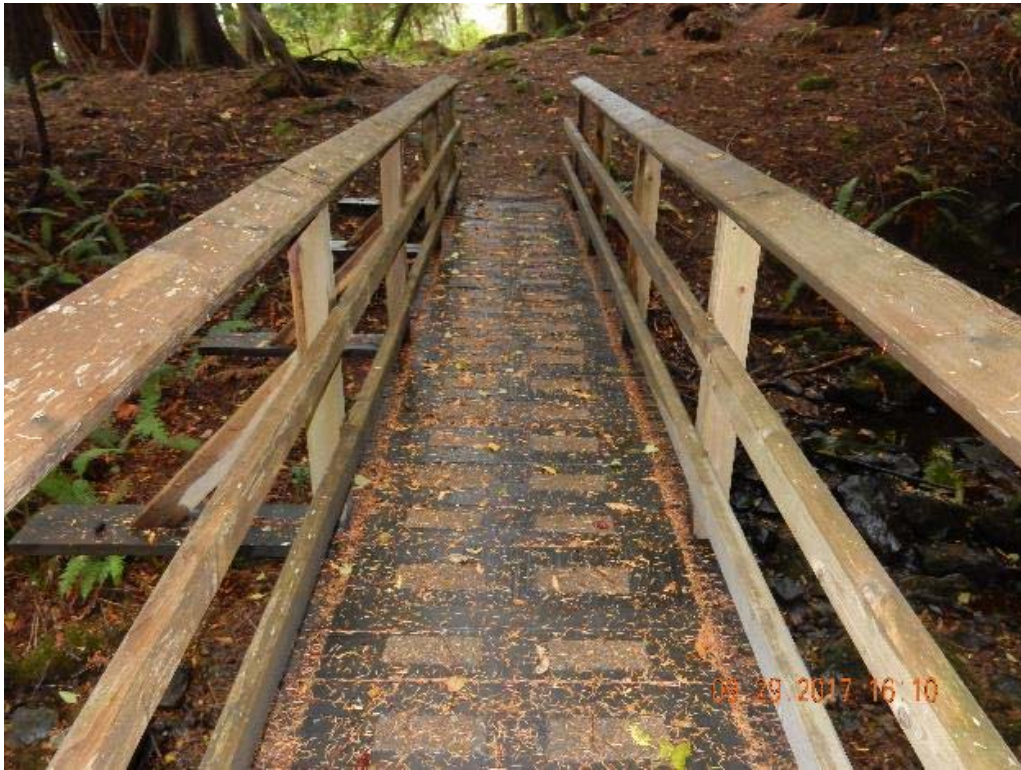
P03 – Overall decking (DSCN0086.jpg)
