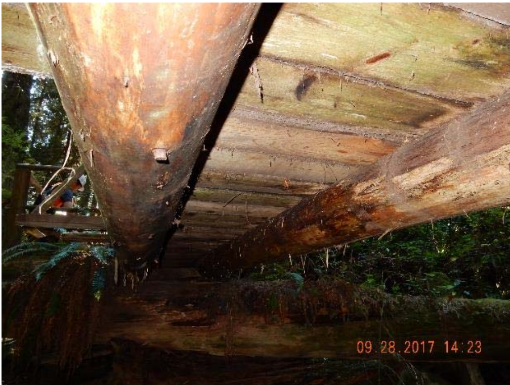
P20 – Under side of the bridge (middle span) (DSCN9597.jpg)
