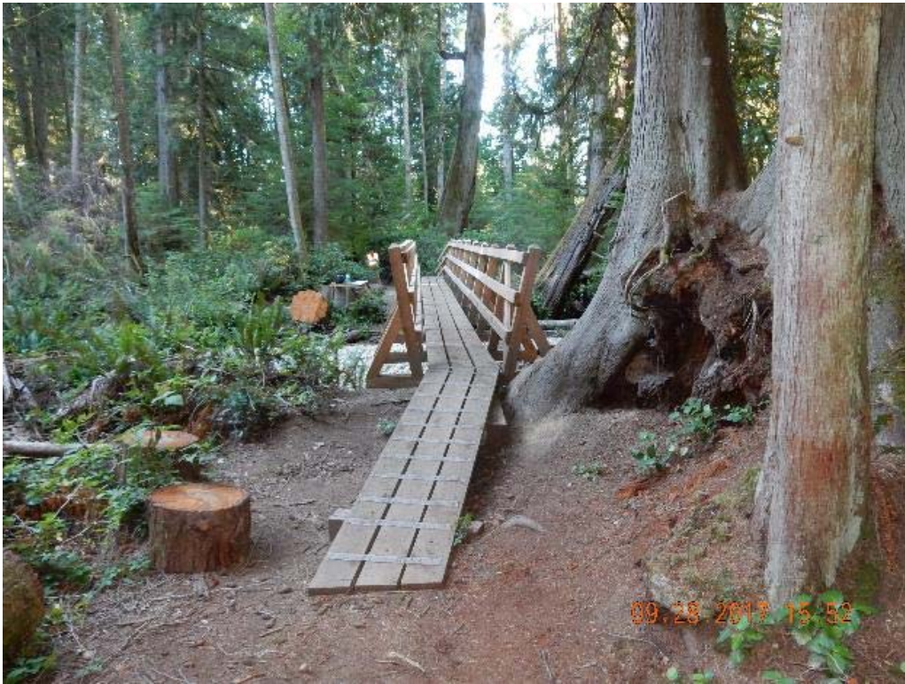
P05 – East approach (DSCN9687.jpg)
