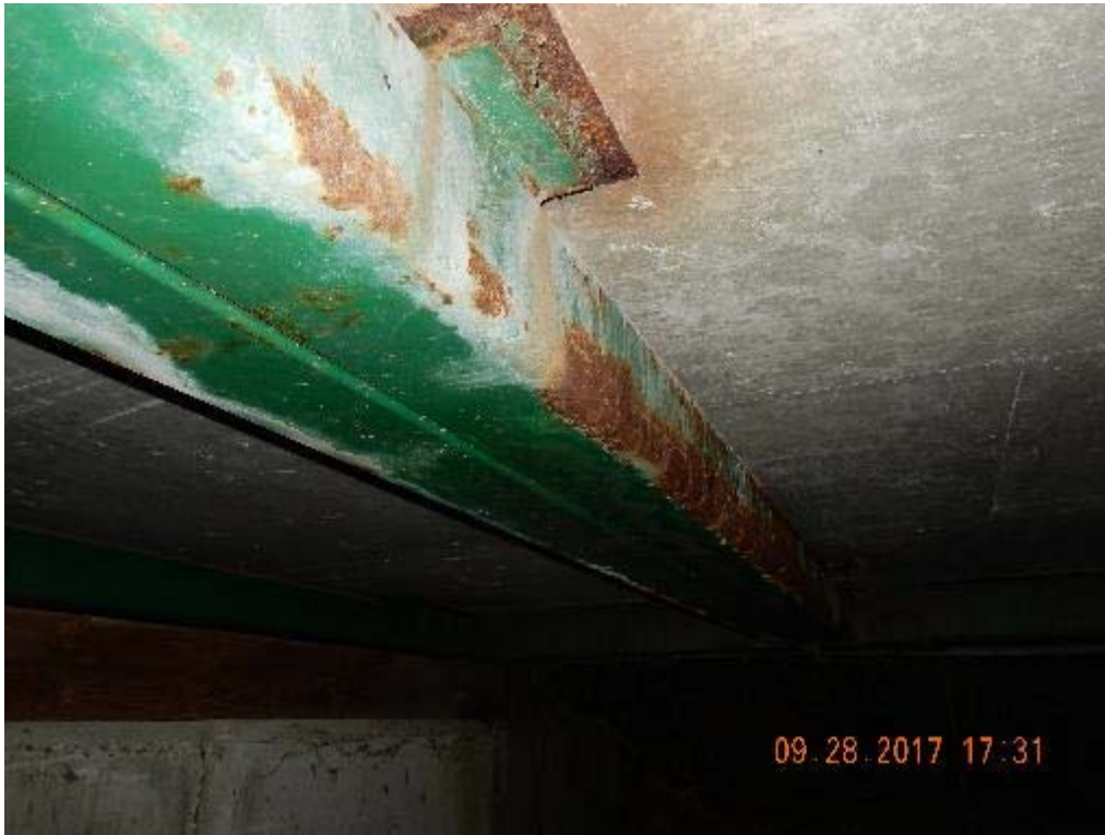
P11 – Floor beam (DSCN9813.jpg)
