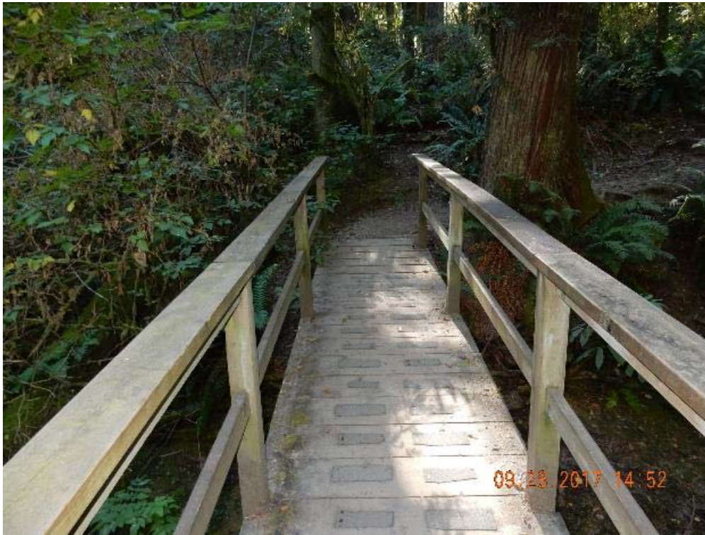
P05 – West end of the bridge (DSCN9627.jpg)
