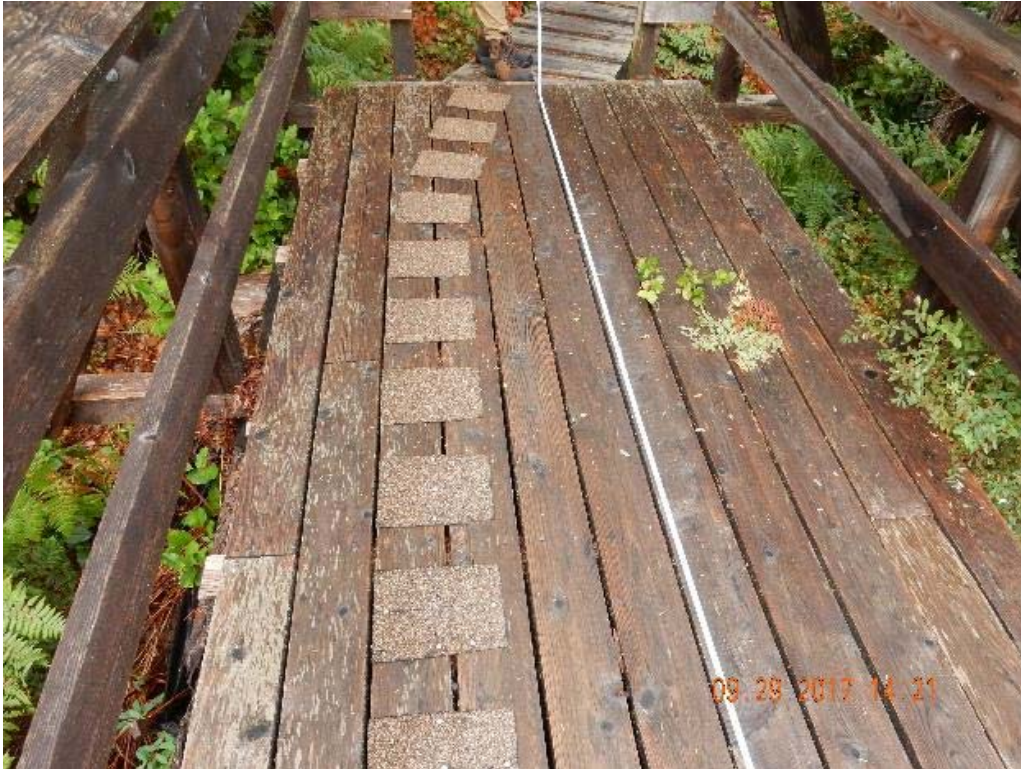
P07 – North end of the bridge (DSCN0038.jpg)
