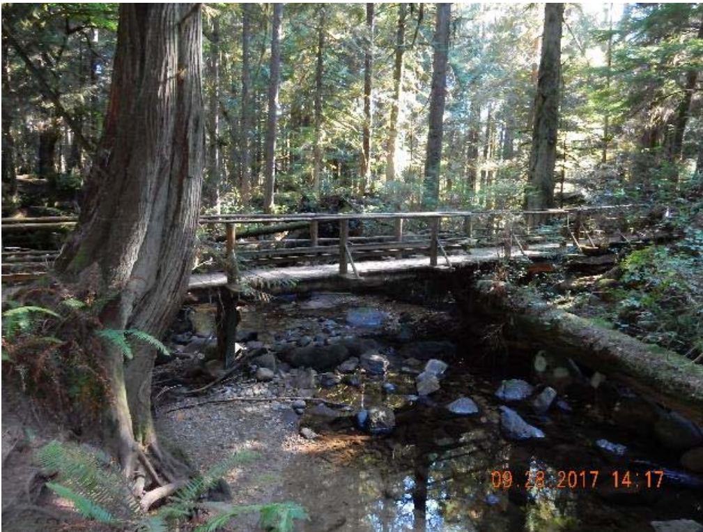
P10 – North side of the bridge (DSCN9587.jpg)
