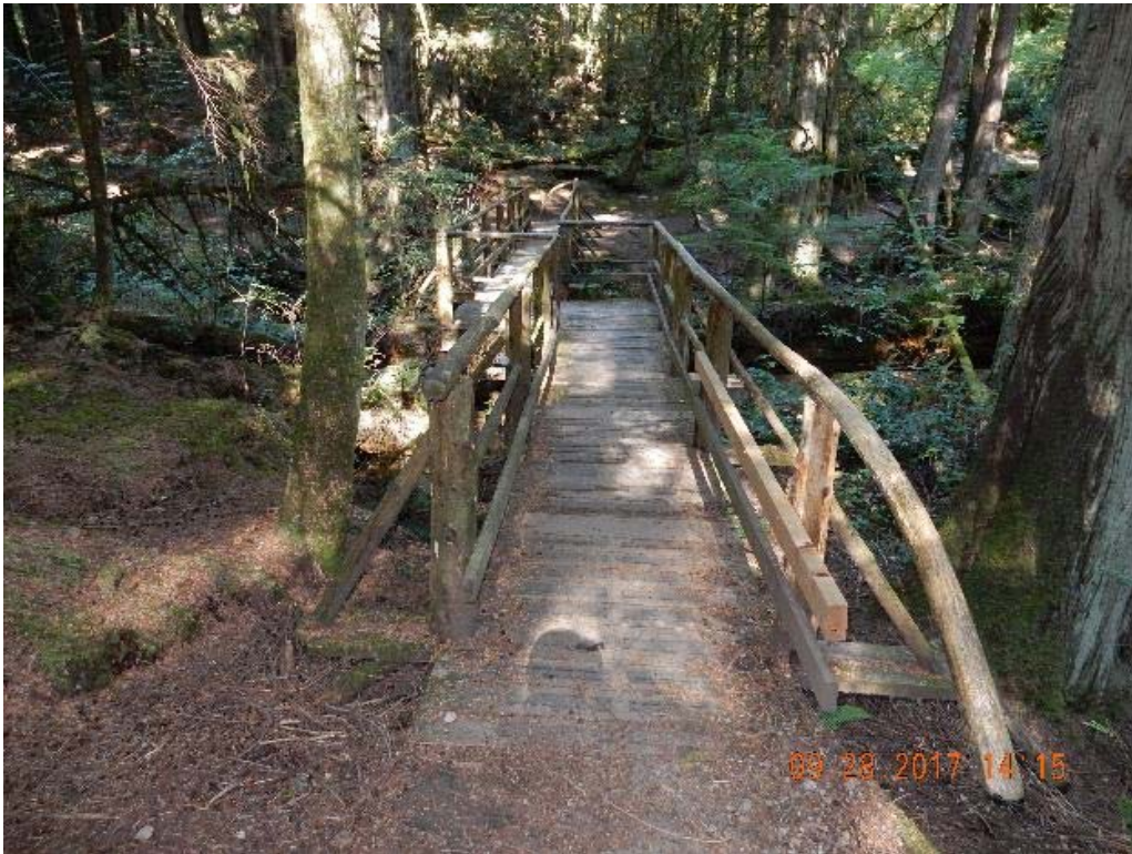
P01 – West approach (DSCN9578.jpg)
