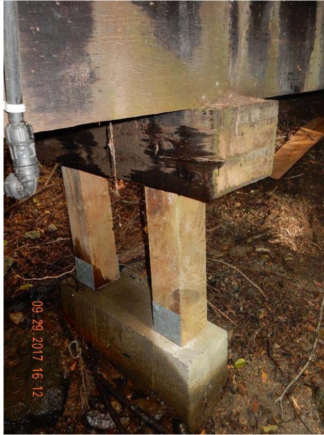
P13 – Middle pier (DSCN0097.jpg)
