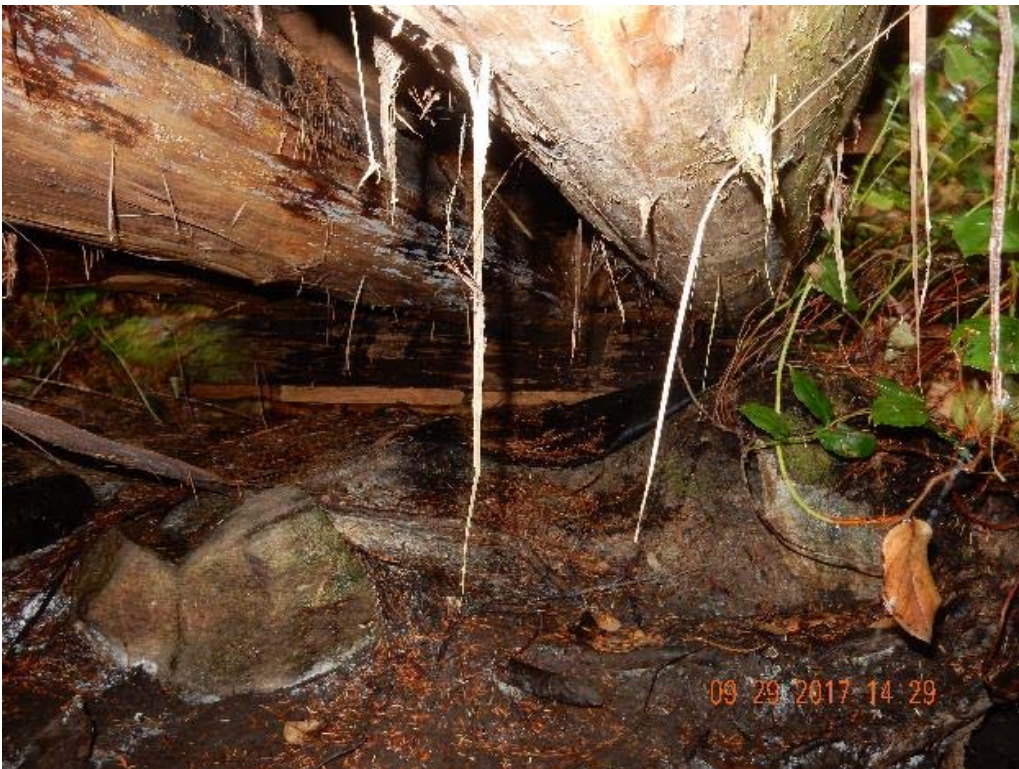
P08 – North abutment (DSCN0057.jpg)
