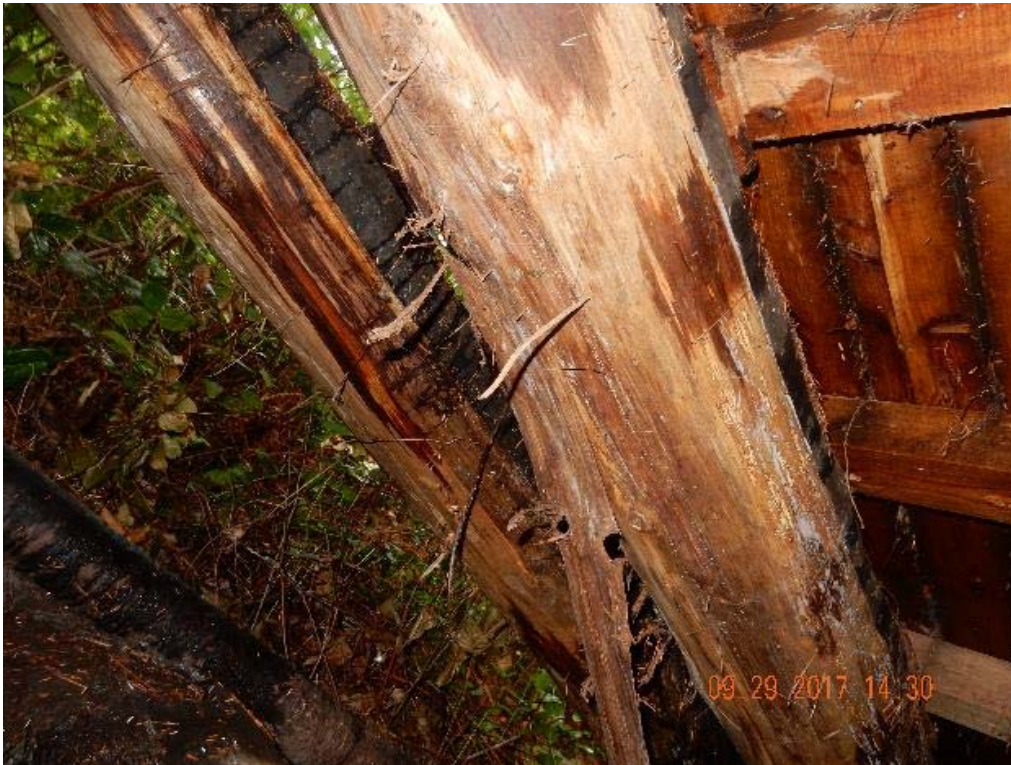
P09 – Under side of the bridge (west and middle log) (DSCN0059.jpg)
