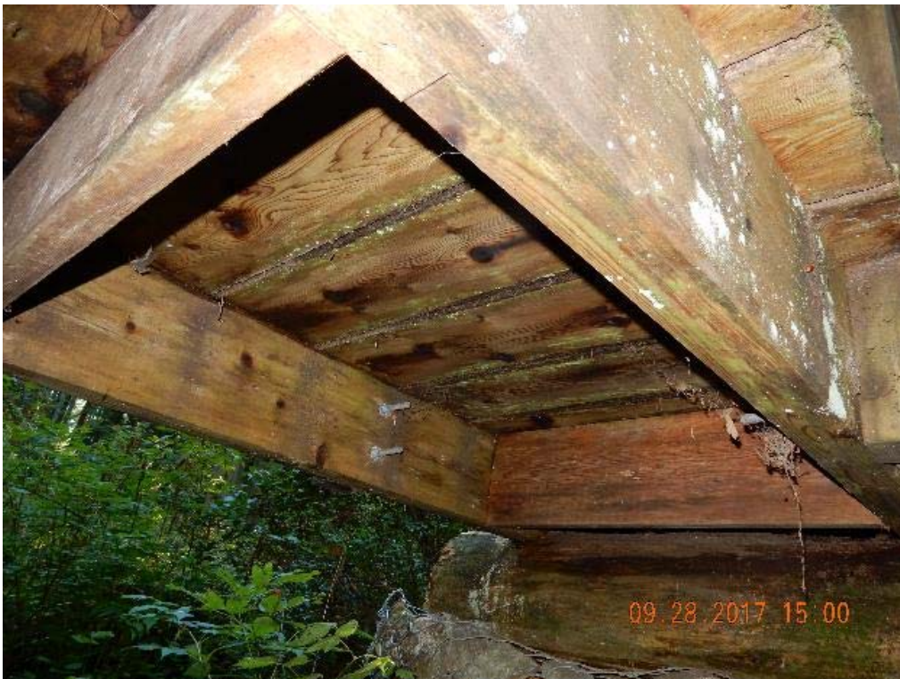
P22 – Under side of the bridge (east span) (DSCN9647.jpg)
