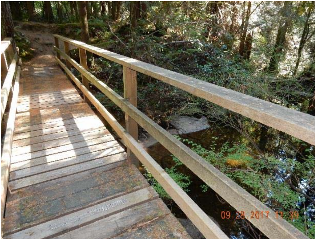
P04 – South railing (DSCN9508.jpg)
