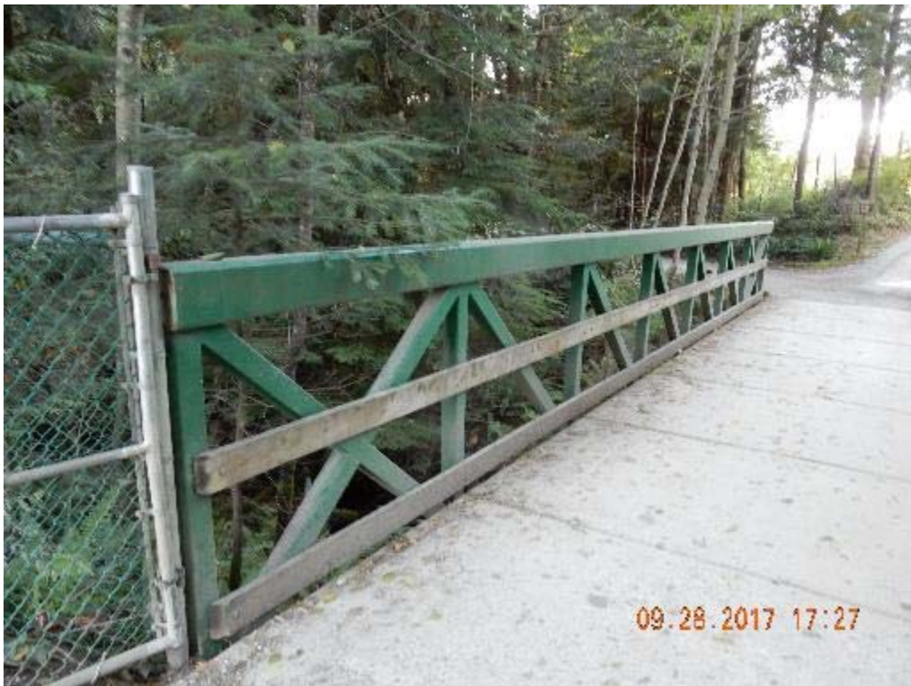
P02 – South railing (DSCN9800.jpg)
