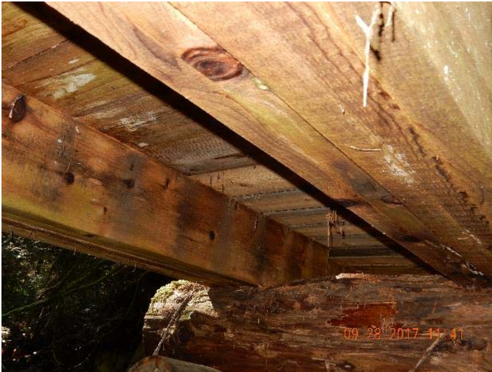
P13 – Under side of the bridge (east span) (DSCN9517.jpg)
