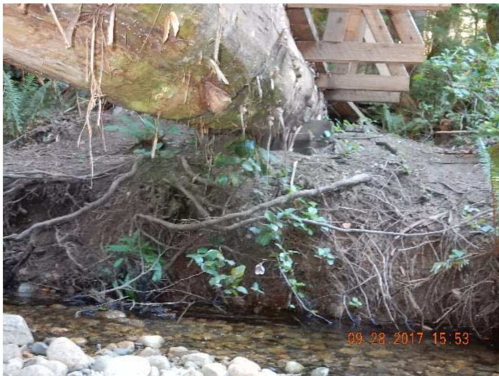
P08 – East abutment (DSCN9690.jpg)
