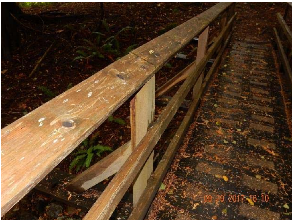
P04 – East railing (DSCN0087.jpg)
