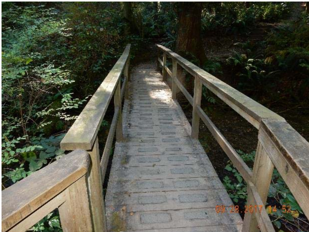
P04 – Overall decking (west span) (DSCN9626.jpg)
