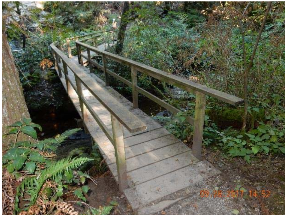
P06 – West approach (DSCN9628.jpg)
