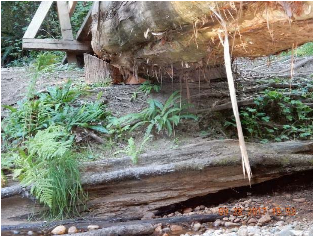
P09 – West abutment (DSCN9691.jpg)
