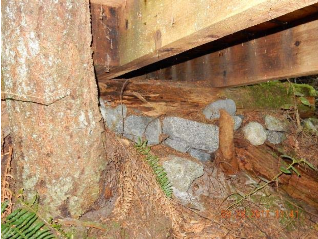
P11 – East abutment (DSCN9515.jpg)
