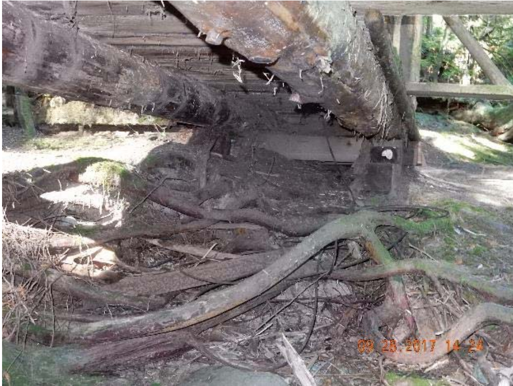
P21 – East abutment (DSCN9598.jpg)
