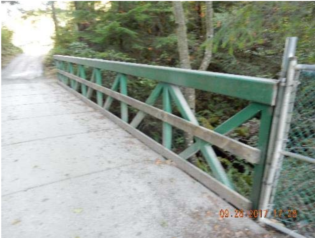
P03 – North railing (DSCN9802.jpg)
