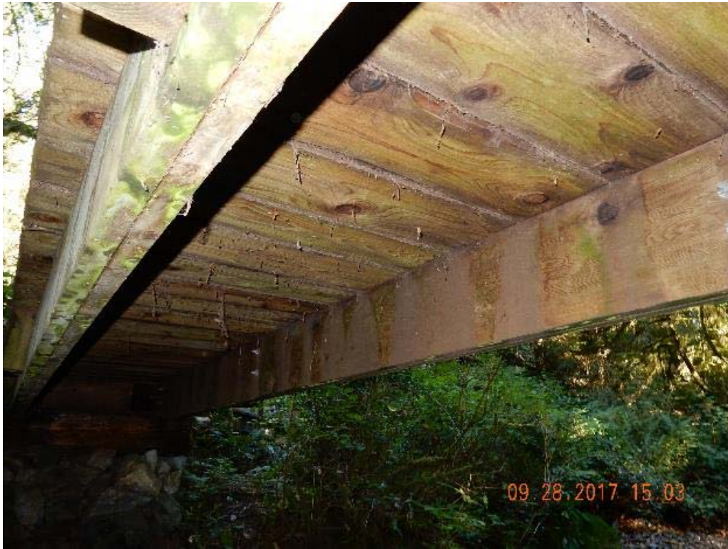
P23 – Under side of the bridge (west span) (DSCN9649.jpg)
