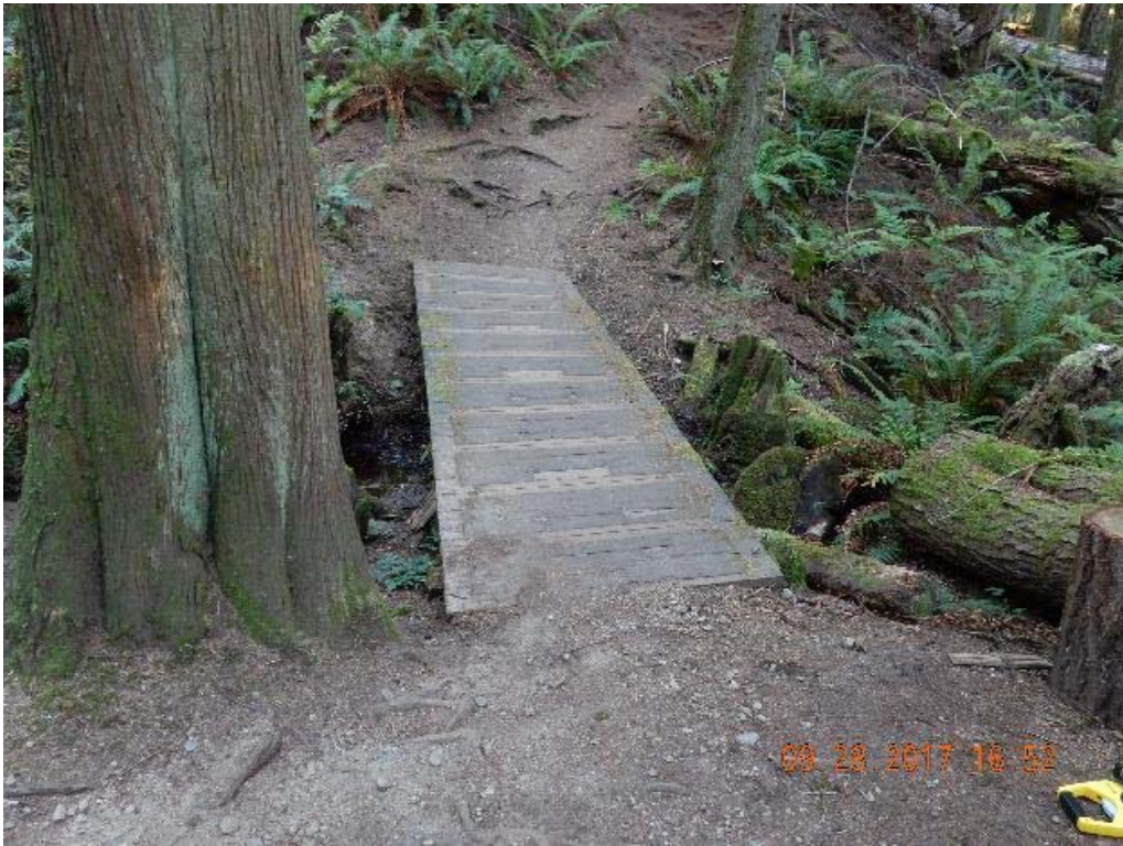
P01 – West approach (DSCN9764.jpg)
