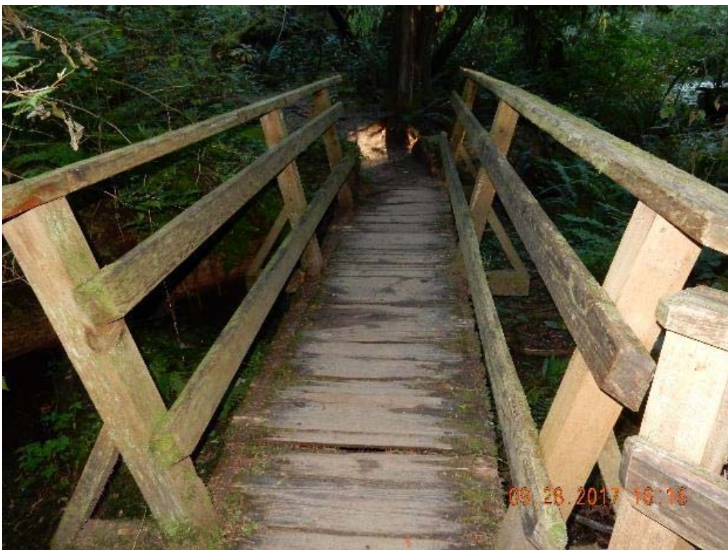
P04 – Overall decking (east span) (DSCN9697.jpg)
