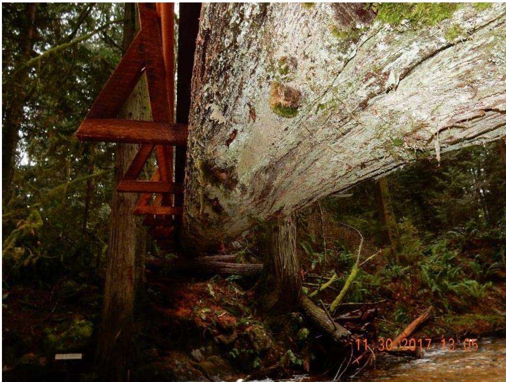
P07 – Under side of the bridge (DSCN0671.jpg)
