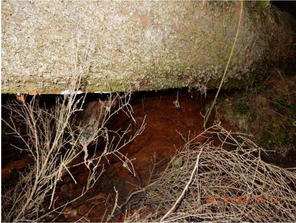
P09 – East abutment of the west span (DSCN9702.jpg)
