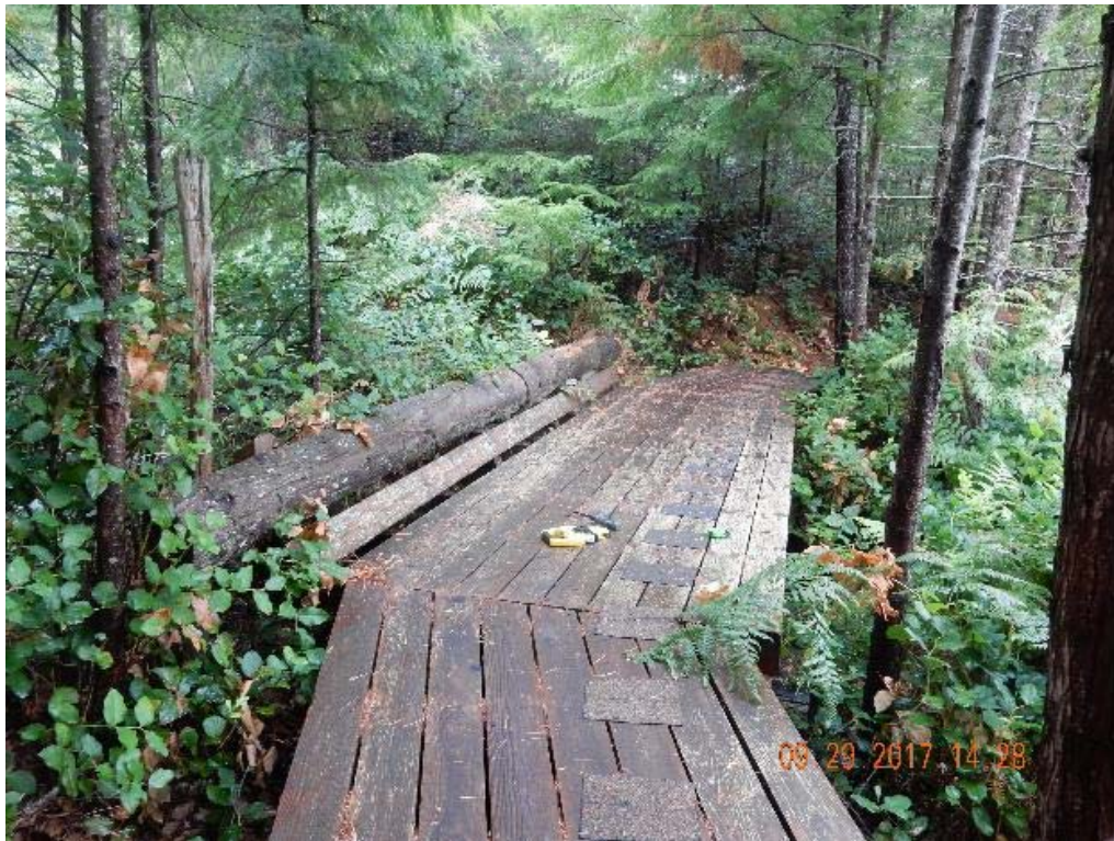
P02 – Overall decking (DSCN0051.jpg)
