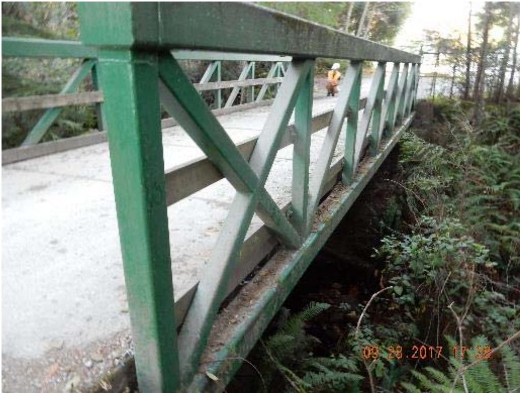
P07 – South side of the bridge (DSCN9806.jpg)
