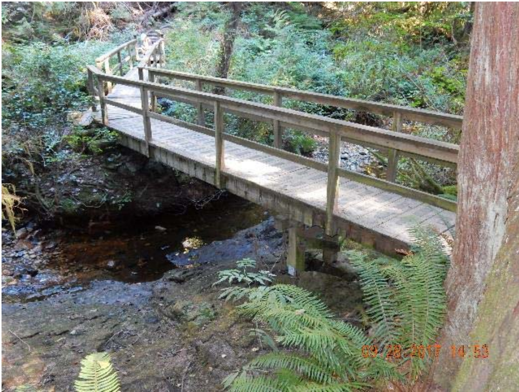
P09 – North side of the bridge (west span) (DSCN9631.jpg)
