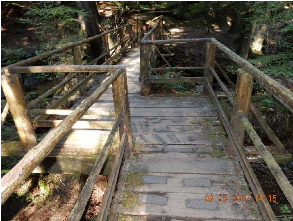
P03 – Overall decking (pier between west and middle span) (DSCN9580.jpg)
