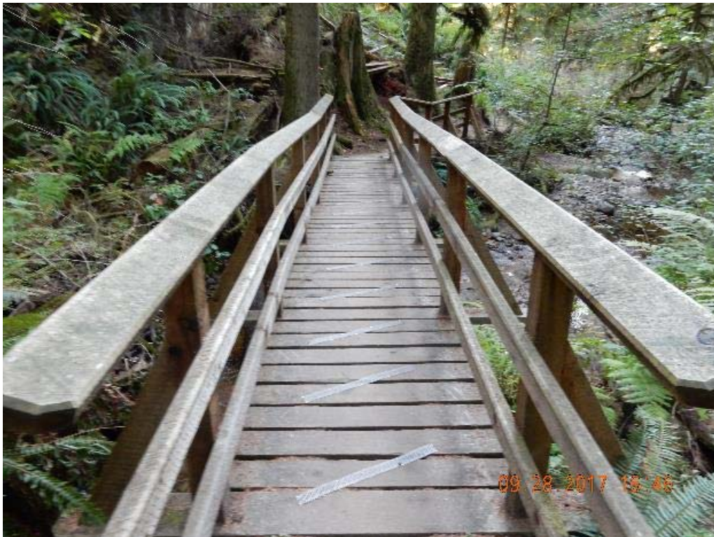
P02 – Overall decking (DSCN9752.jpg)
