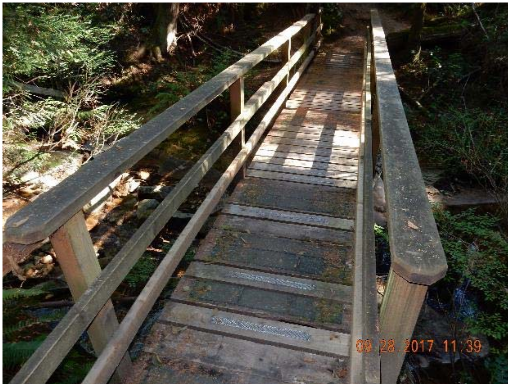
P02 – Overall decking (DSCN9506.jpg)
