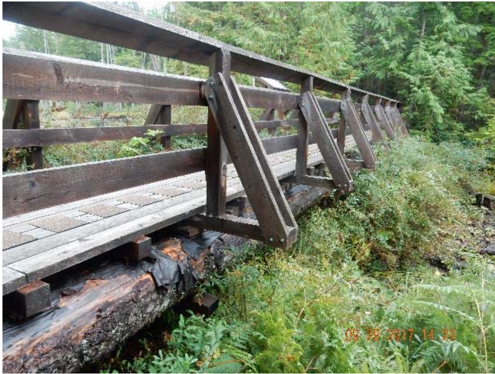
P09 – East side of the bridge (DSCN0040.jpg)
