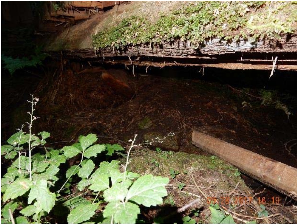
P11 – West abutment of the east span (DSCN9704.jpg)
