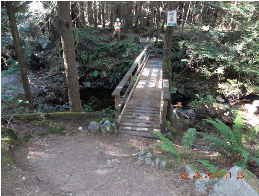
P05 – East approach (DSCN9509.jpg)
