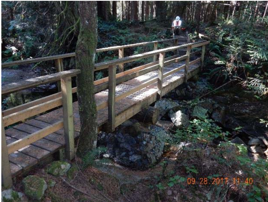
P07 – North side of the bridge (DSCN9511.jpg)
