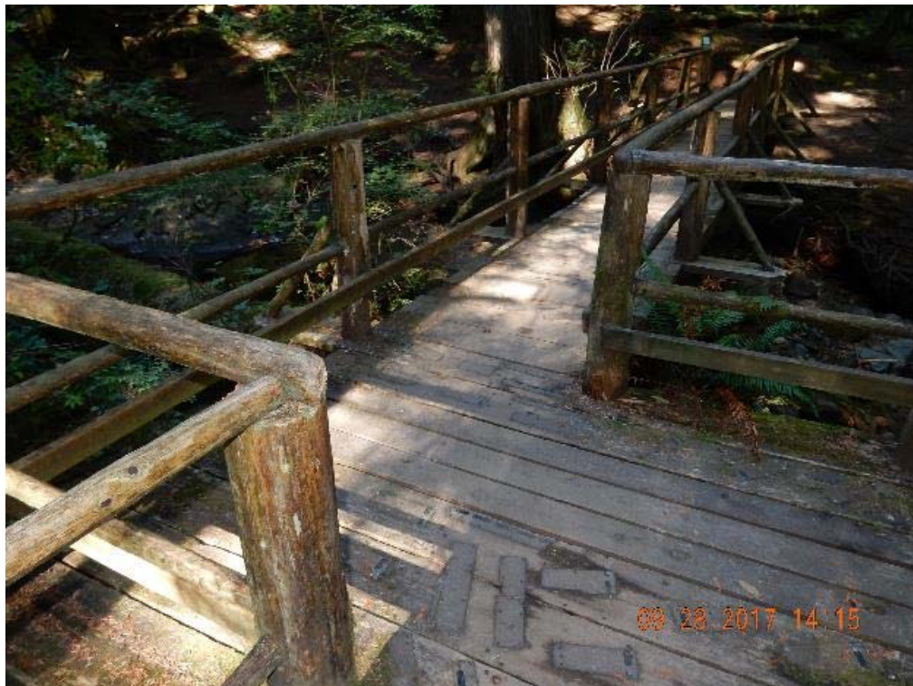
P04 – Overall decking (pier between west and middle span) (DSCN9581.jpg)
