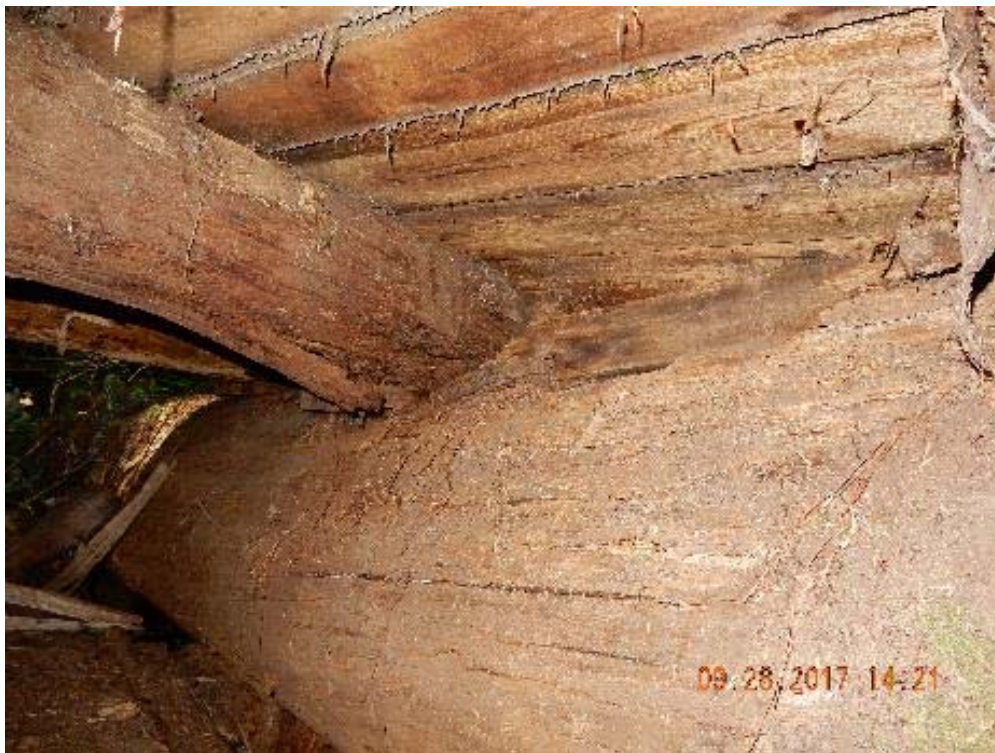
P18 – Pier between west and middle span (detail condition) (DSCN9595.jpg)
