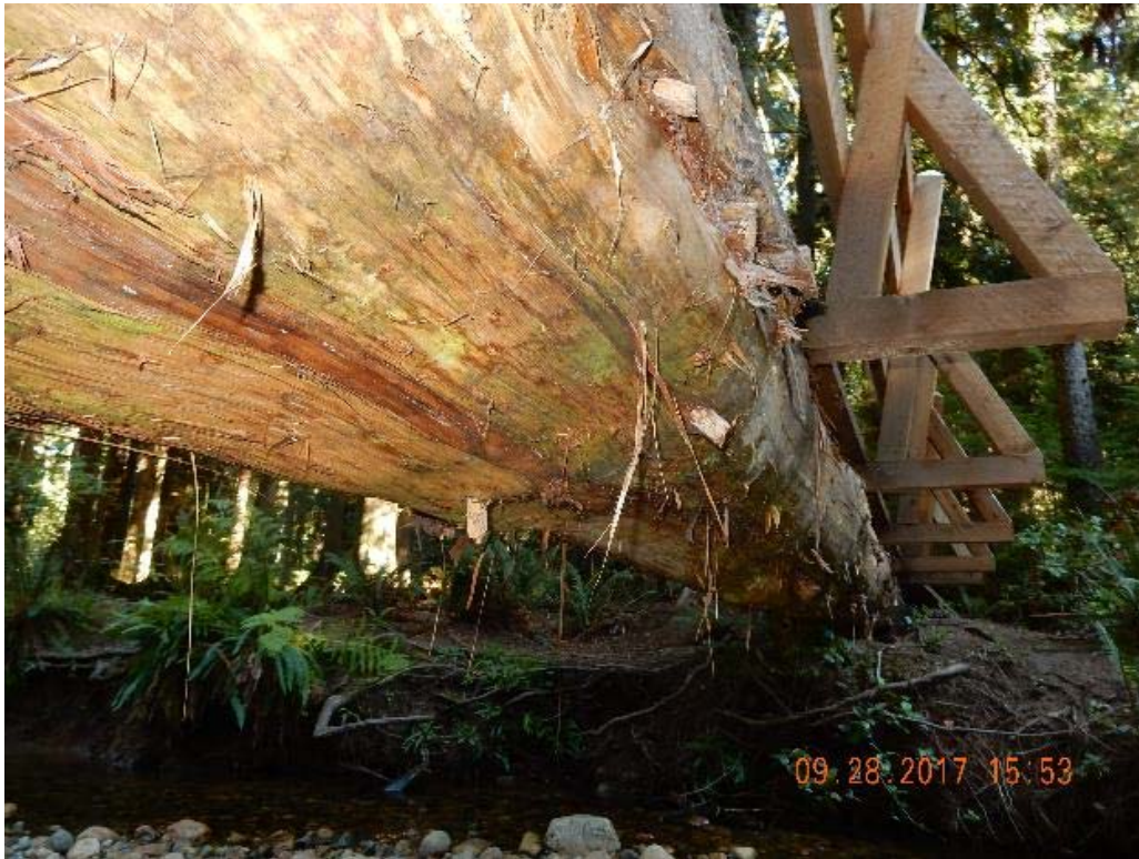
P07 – Under side of the bridge (DSCN9689.jpg)
