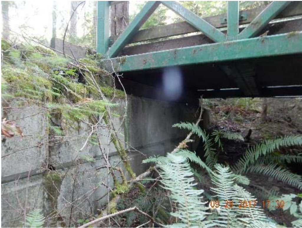
P09 – West abutment (DSCN9809.jpg)
