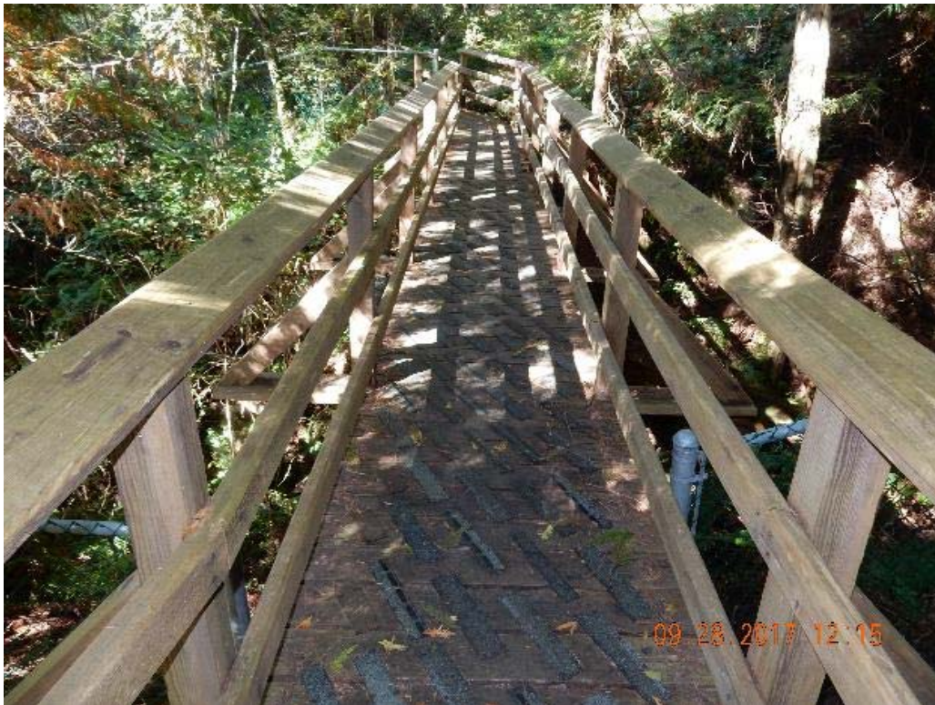
P02 – Overall decking (DSCN9523.jpg)
