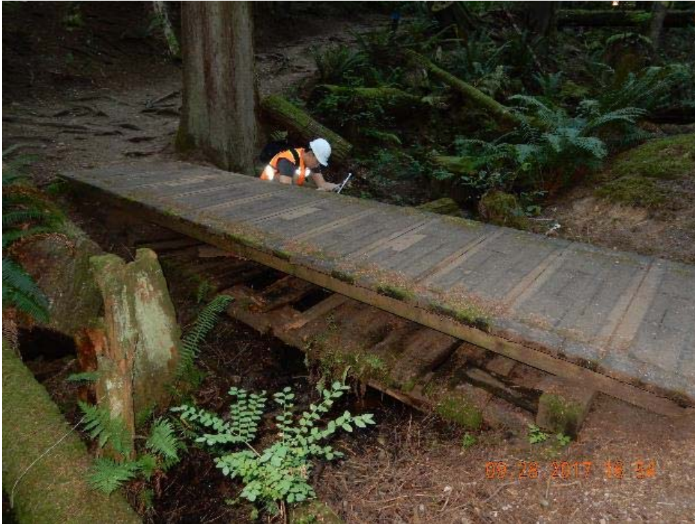
P07 – South side of the bridge (DSCN9771.jpg)
