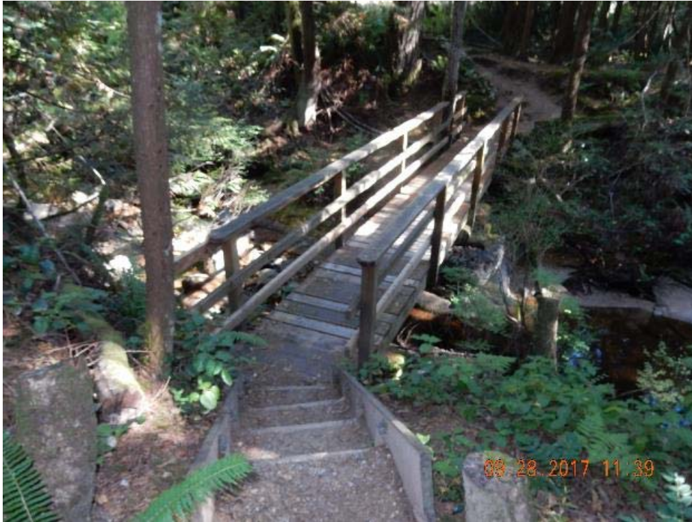
P01 – West approach (DSCN9505.jpg)
