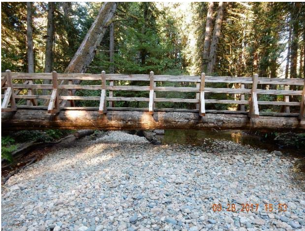
P06 – South side of the bridge (DSCN9688.jpg)
