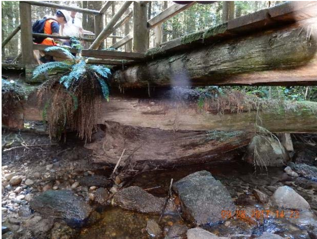
P19 – Pier between west and middle span (DSCN9596.jpg)
