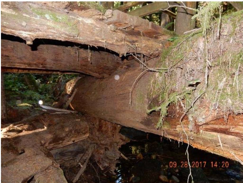
P16 – Pier between west and middle span (DSCN9590.jpg)
