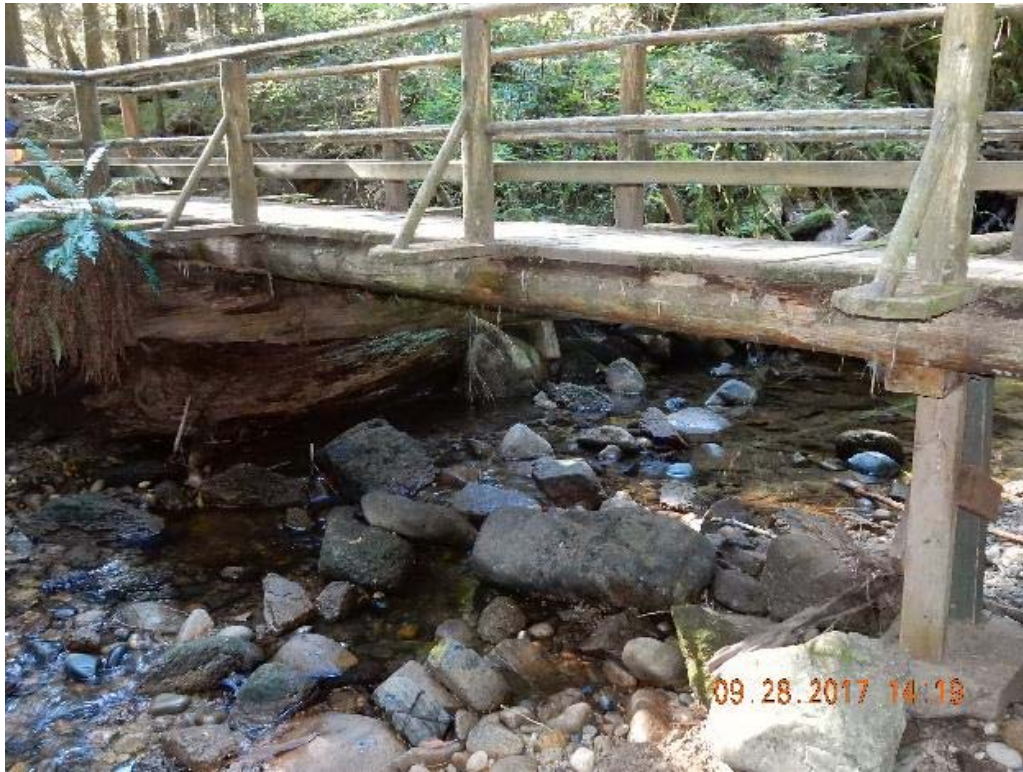
P13 – South side of the bridge (middle span) (DSCN9590.jpg)
