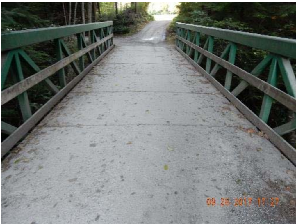
P04 – Overall decking (DSCN9801.jpg)
