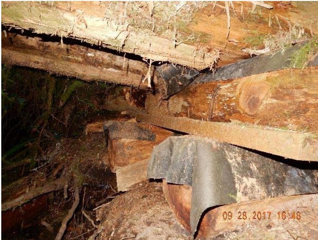
P07 – South abutment (DSCN9759.jpg)
