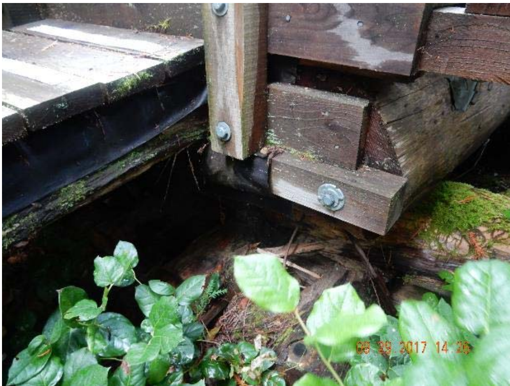
P12 – South abutment (DSCN0047.jpg)
