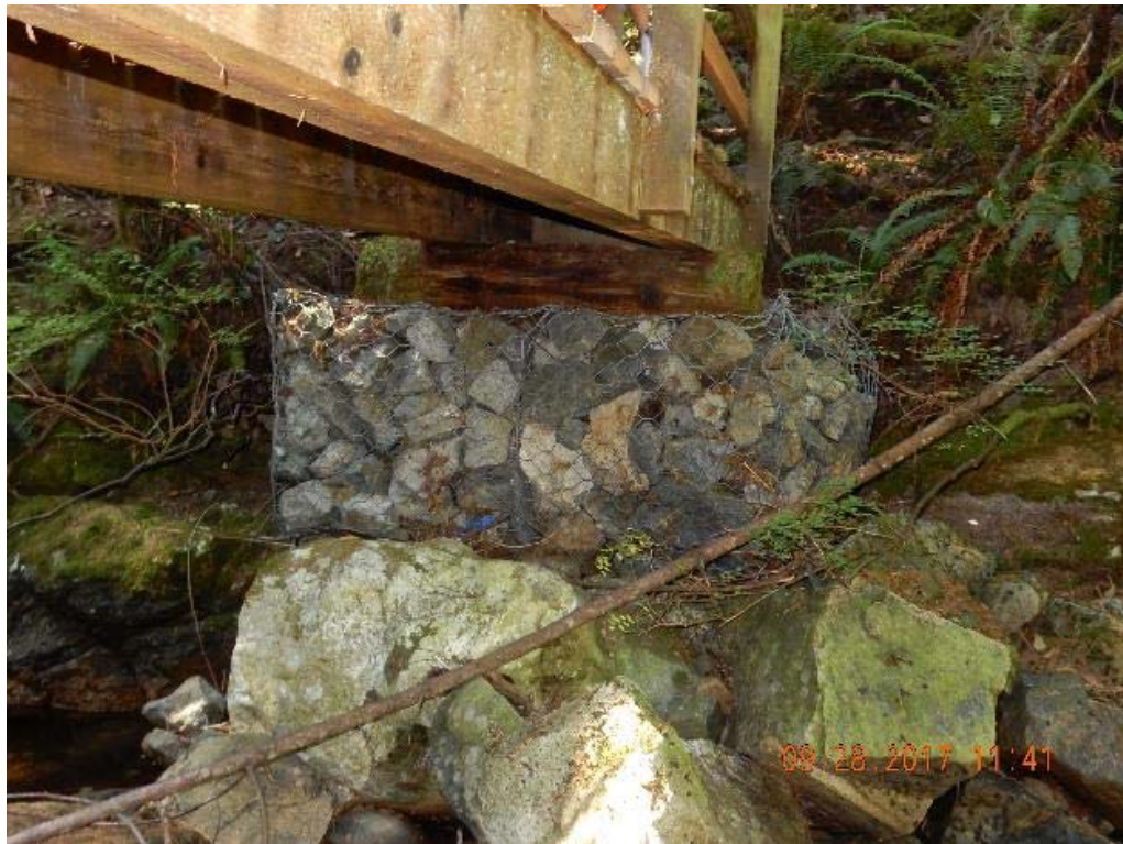
P10 – West abutment (DSCN9514.jpg)
