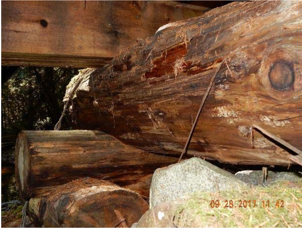
P15 – Middle pier (detail condition) (DSCN9519.jpg)
