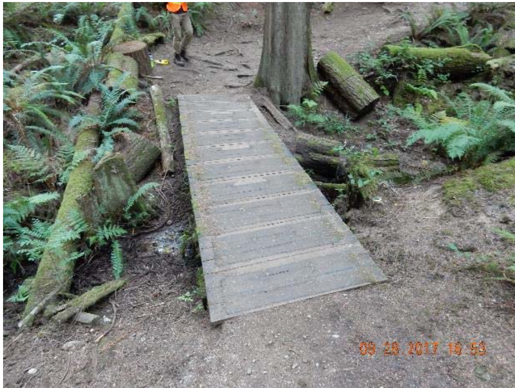
P02 – East approach (DSCN9766.jpg)
