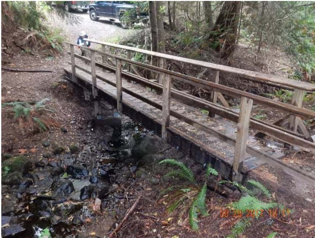
P09 – West side of the bridge (DSCN0092.jpg)
