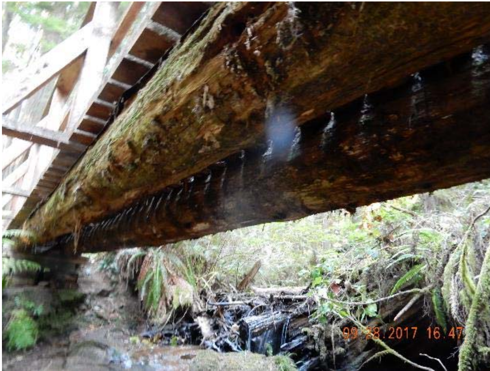
P05 – Under side of the bridge (DSCN9756.jpg)
