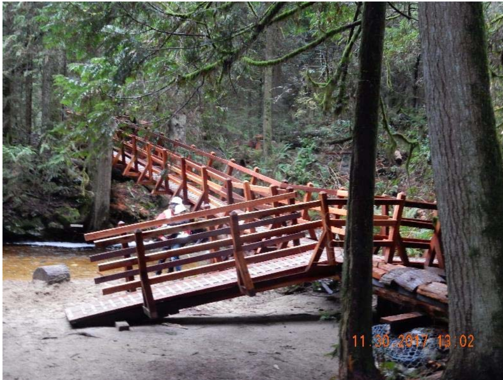
P01 – East approach (DSCN0639.jpg)
