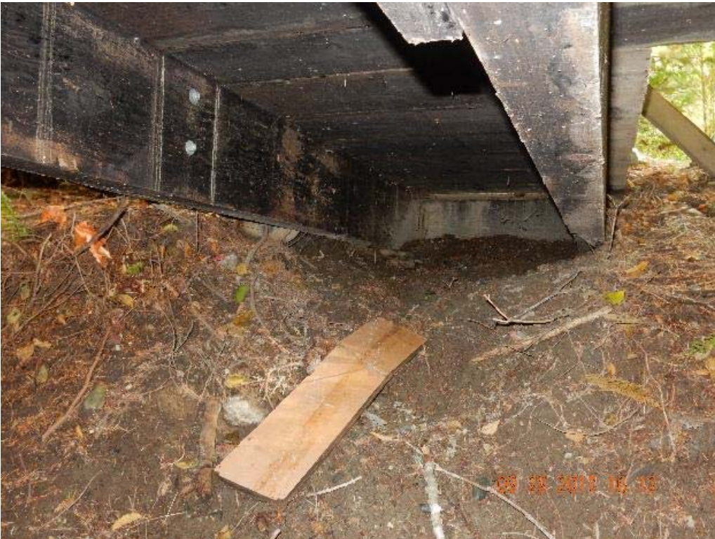
P12 – North abutment (DSCN0096.jpg)
