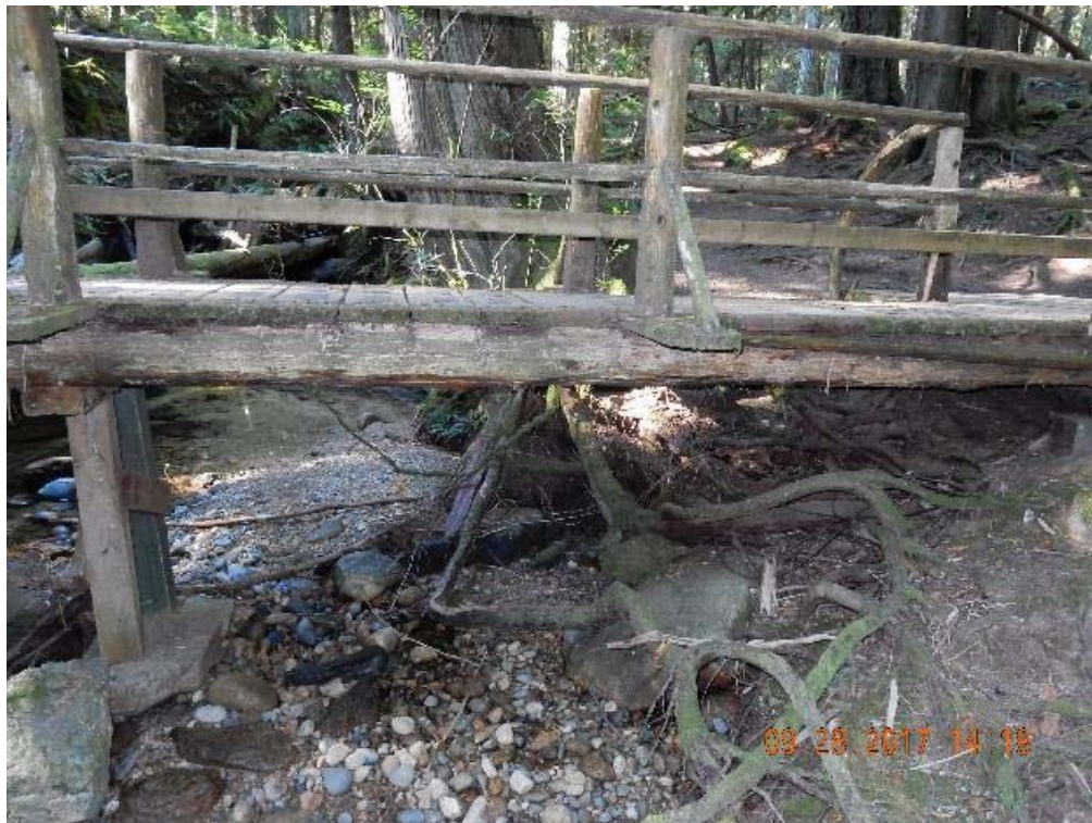
P12 – South side of the bridge (east span) (DSCN9589.jpg)
