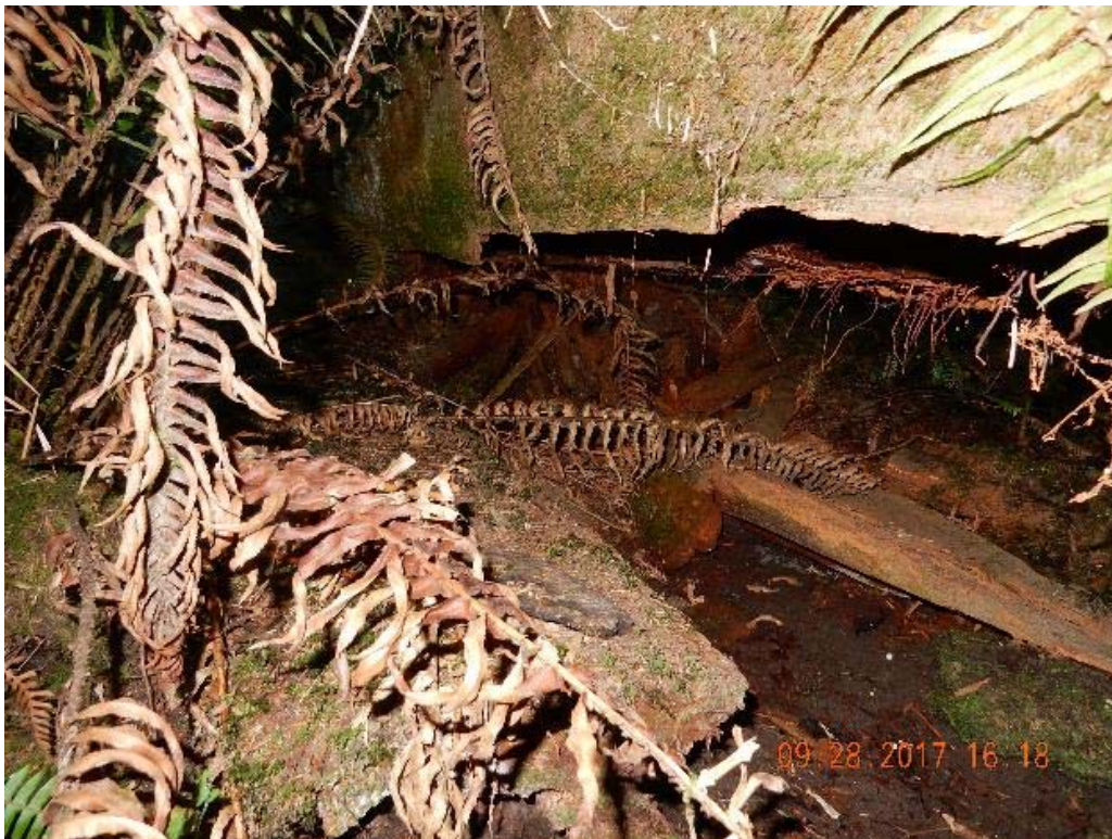
P08 – West abutment of west span (DSCN9701.jpg)
