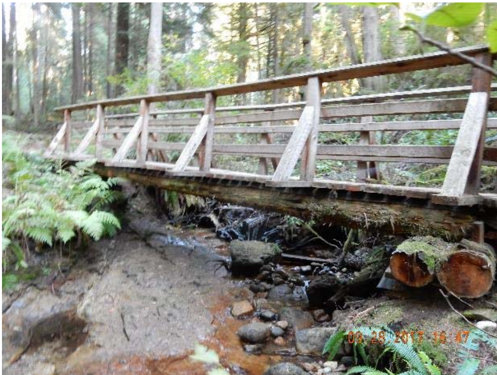
P04 – West side of the bridge (DSCN9755.jpg)
