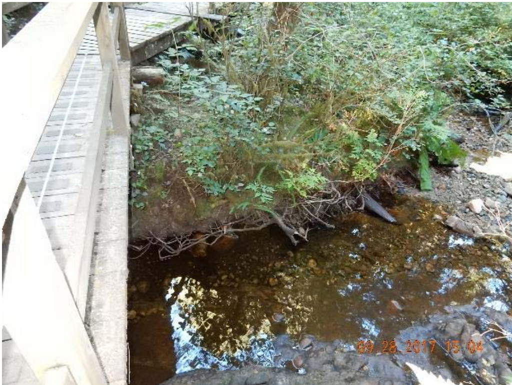
P24 – West span pier 2 (south side) (DSCN9650.jpg)
