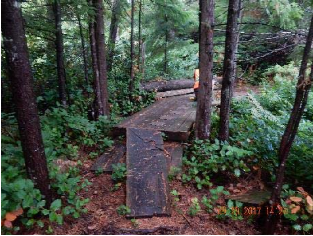
P01 – South approach (DSCN0050.jpg)
