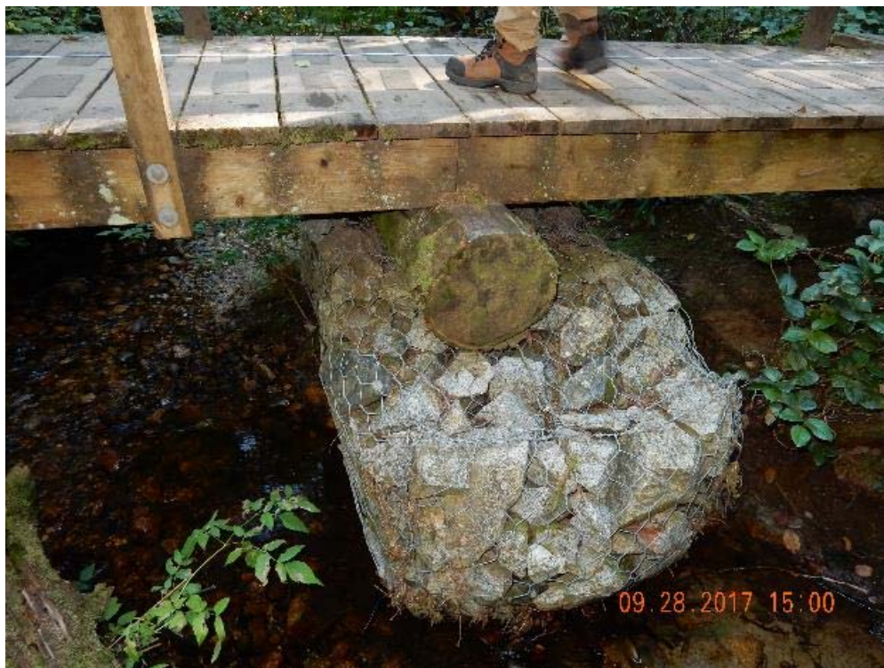
P20 – East span pier 3 (DSCN9645.jpg)
