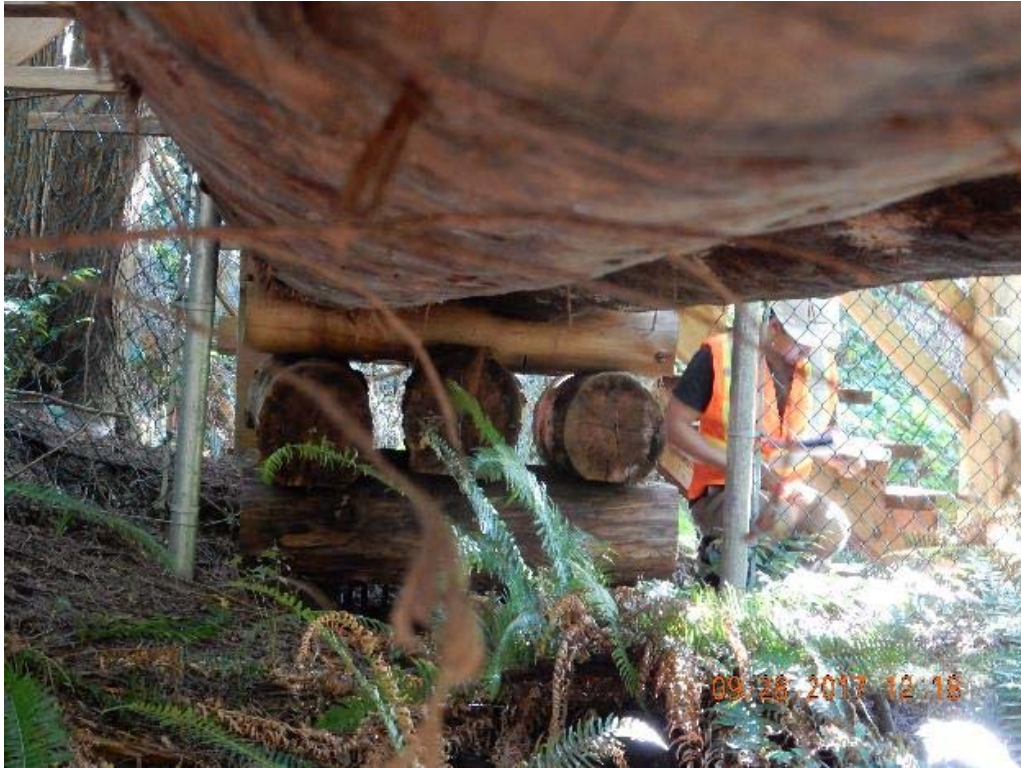
P09 – South abutment (DSCN9531.jpg)
