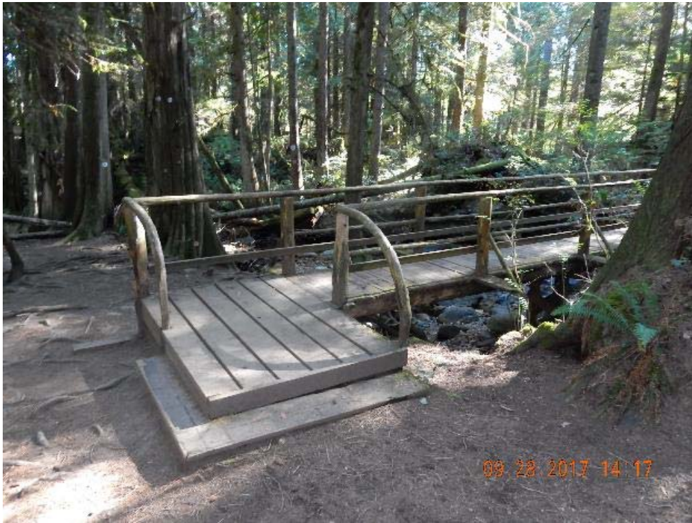
P09 – East approach (DSCN9586.jpg)
