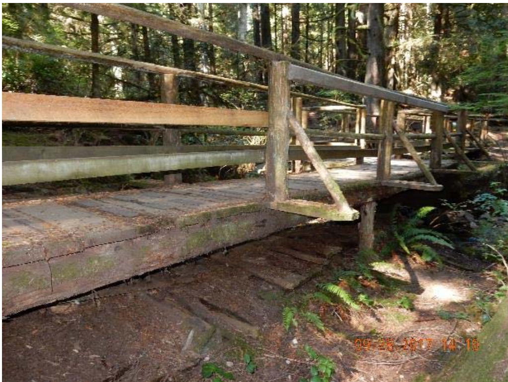
P14 – South side of the bridge (west span) (DSCN9591.jpg)
