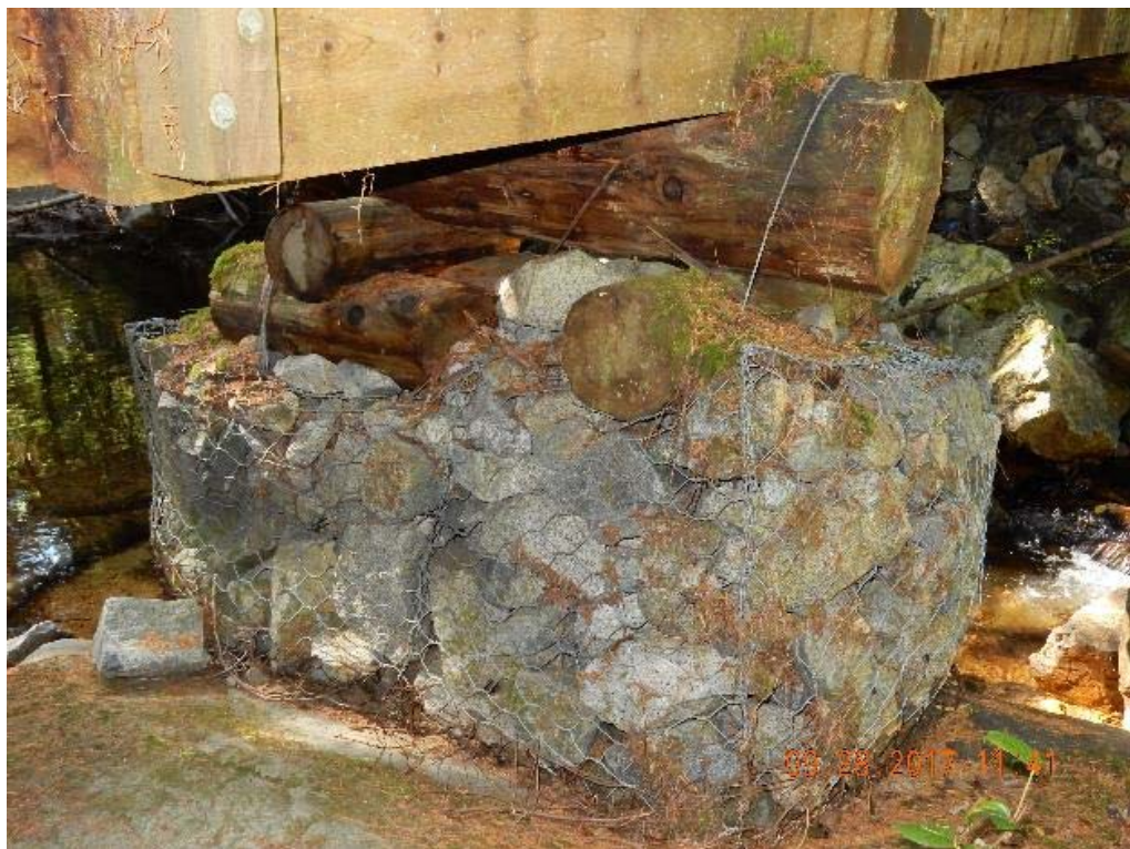
P12 – Middle pier (DSCN9516.jpg)
