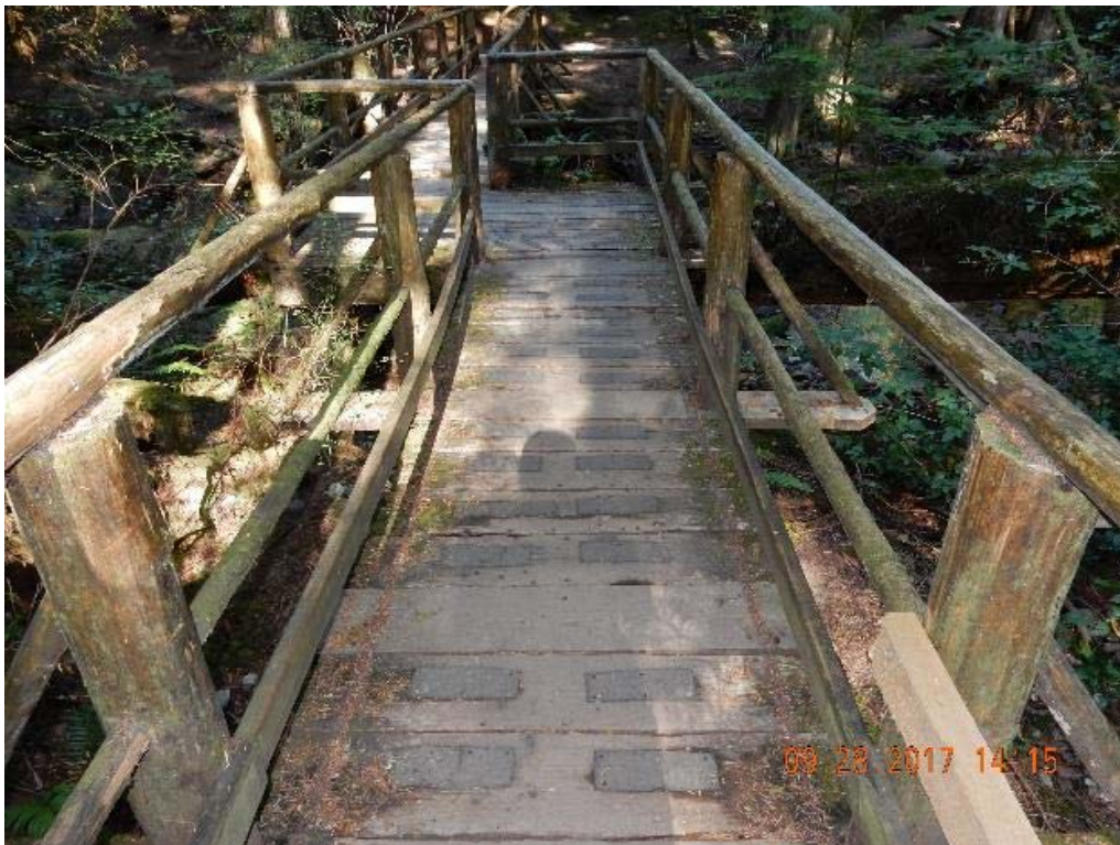
P02 – Overall decking (west span) (DSCN9579.jpg)
