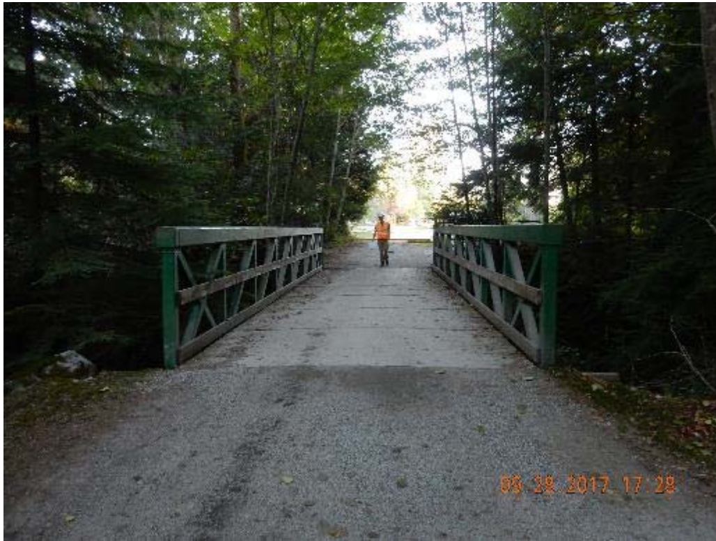
P05 – West approach (DSCN9803.jpg)
