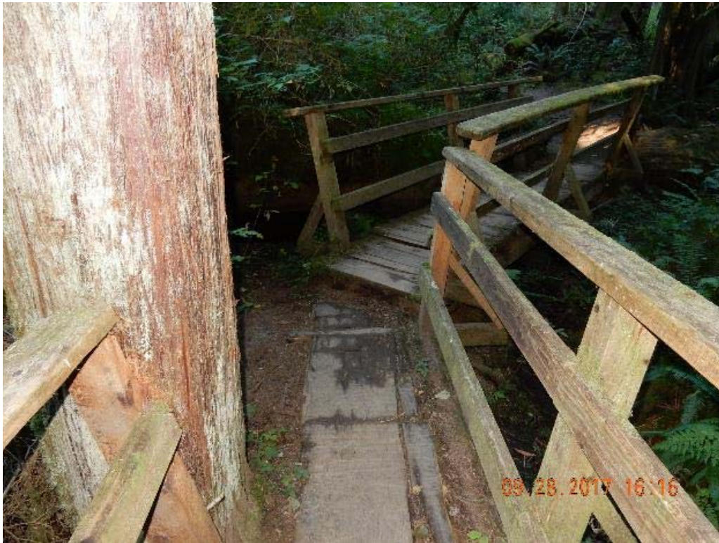
P03 – Overall decking (between west and east span) (DSCN9696.jpg)
