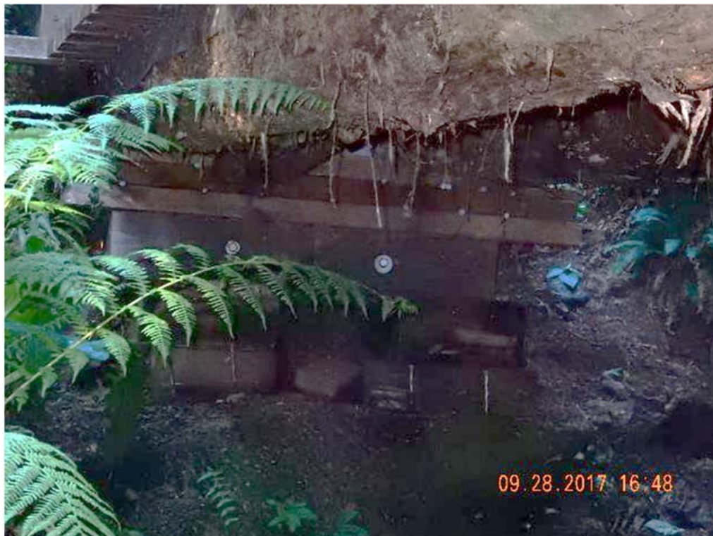
P06 – North abutment (DSCN9758.jpg)
