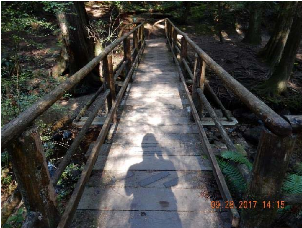
P05 – Overall decking (middle span) (DSCN9582.jpg)
