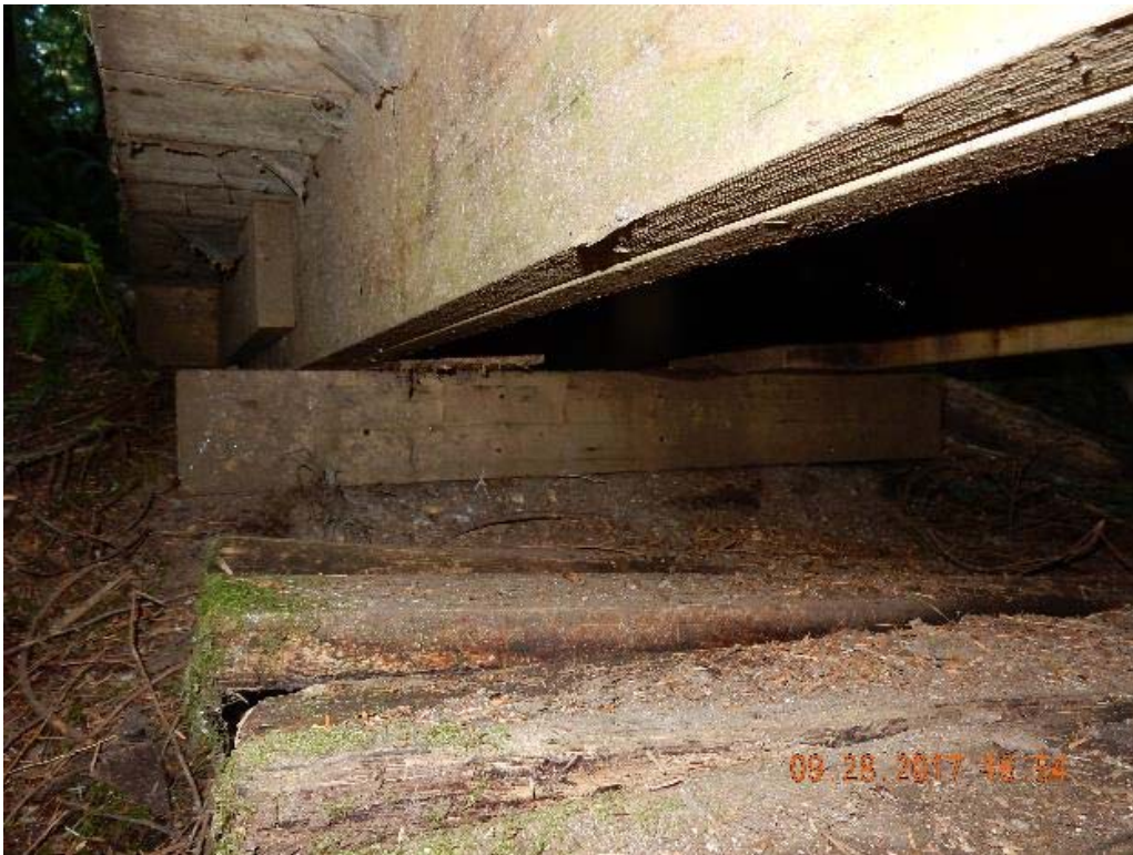
P06 – West abutment (DSCN9770.jpg)
