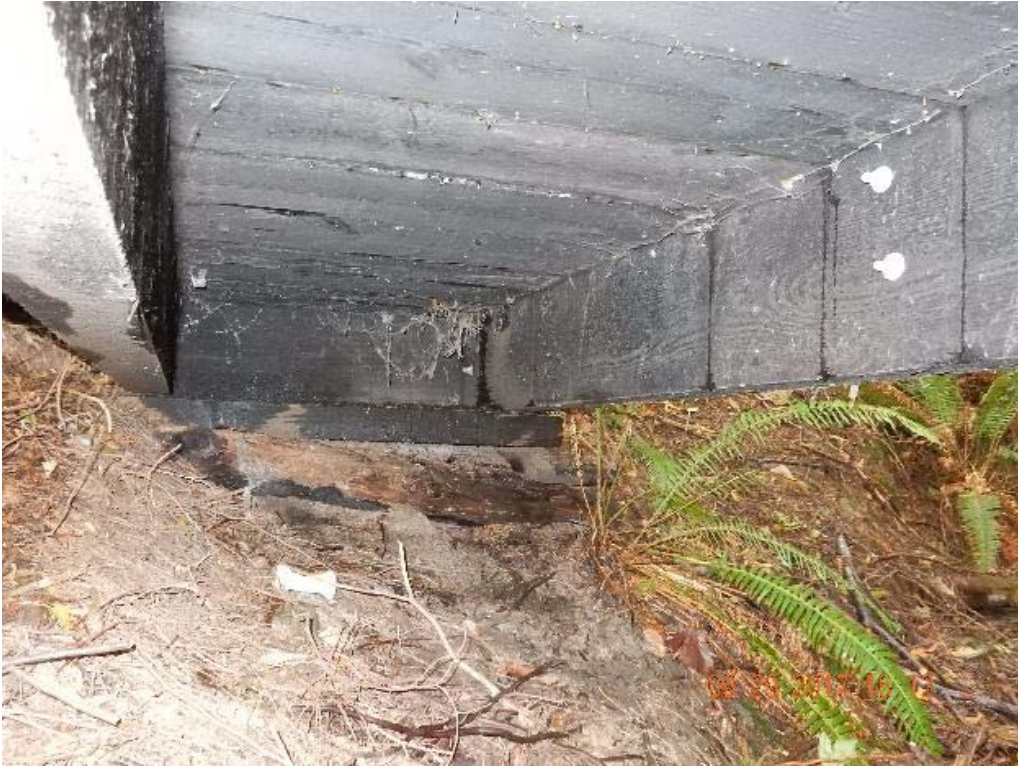
P11 – South abutment (DSCN0095.jpg)
