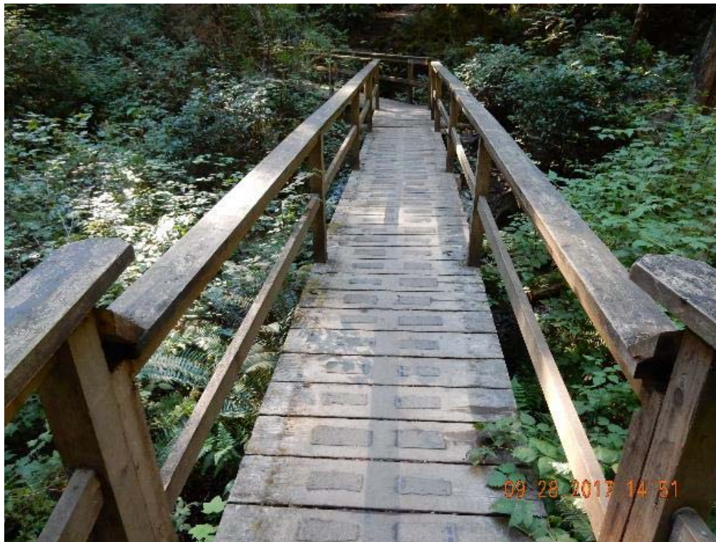
P02 – Overall decking (east span) (DSCN9622.jpg)
