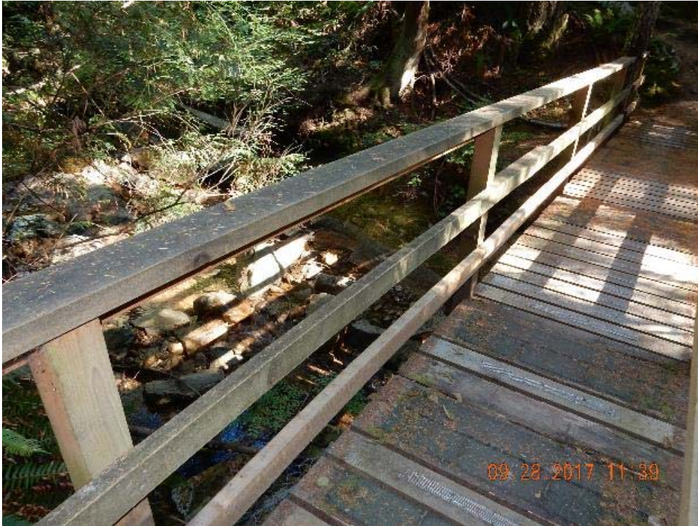
P03 – North railing (DSCN9507.jpg)
