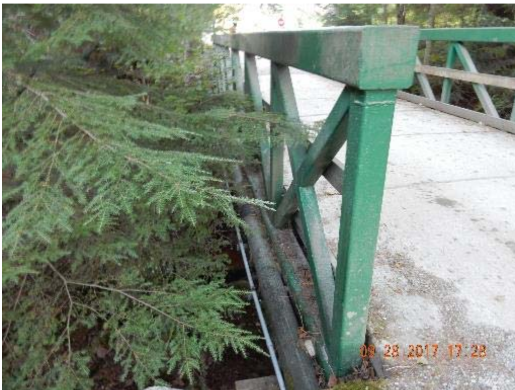
P06 – North side of the bridge (DSCN9805.jpg)
