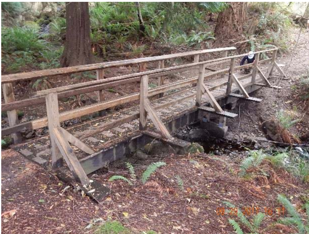
P10 – East side of the bridge (DSCN0093.jpg)
