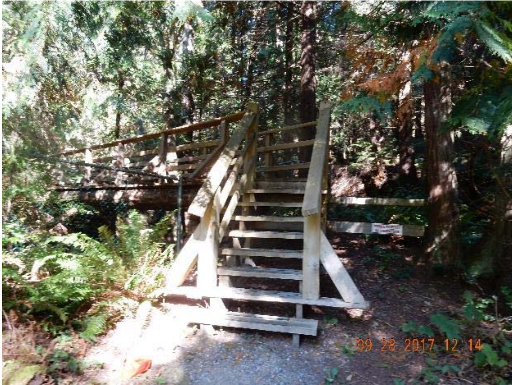
P01 – South approach (DSCN9521.jpg)
