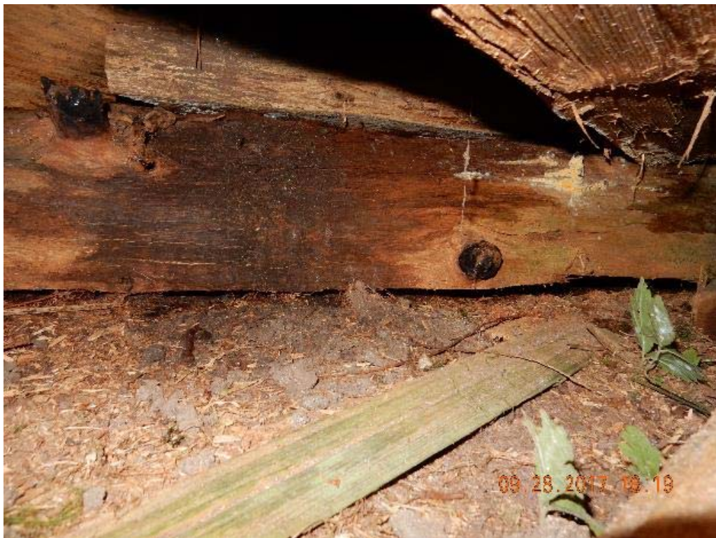
P12 – East abutment of east span (DSCN9705.jpg)
