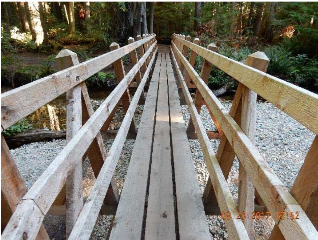
P02 – Overall decking (DSCN9683.jpg)
