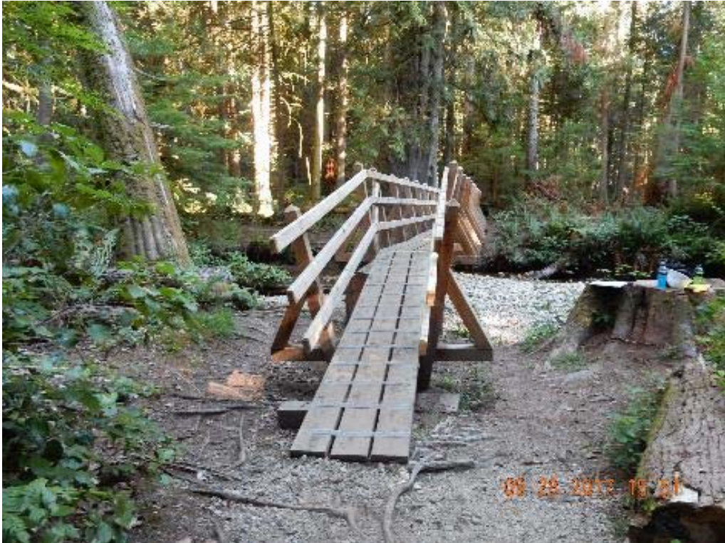
P01 – West approach (DSCN9680.jpg)
