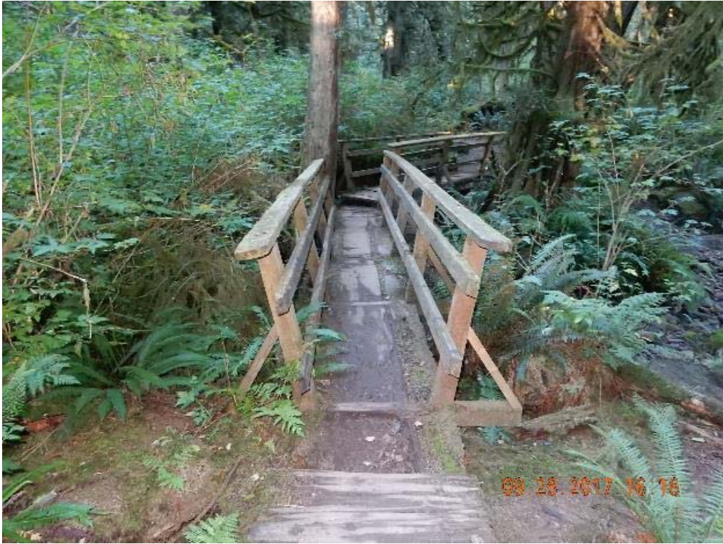
P01 – West approach (DSCN9693.jpg)
