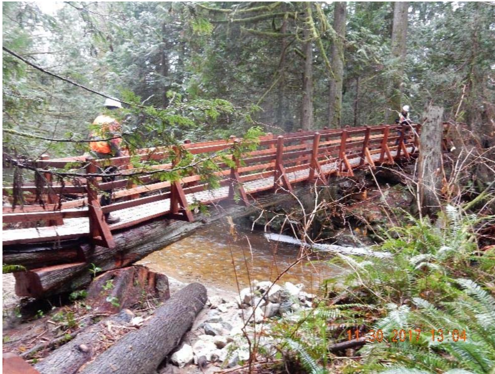
P06 – North side of the bridge (DSCN0664.jpg)
