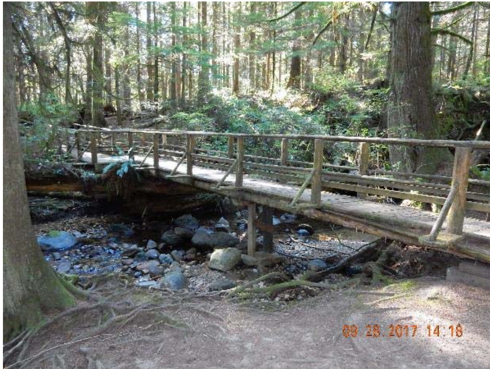
P11 – South side of the bridge (DSCN9588.jpg)
