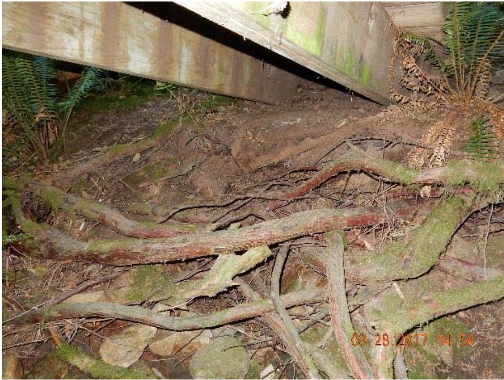
P11 – West abutment (DSCN9633.jpg)
