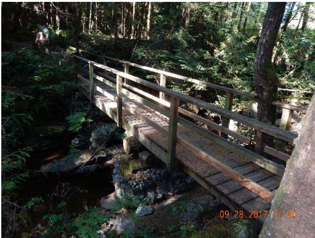
P06 – South side of the bridge (DSCN9510.jpg)
