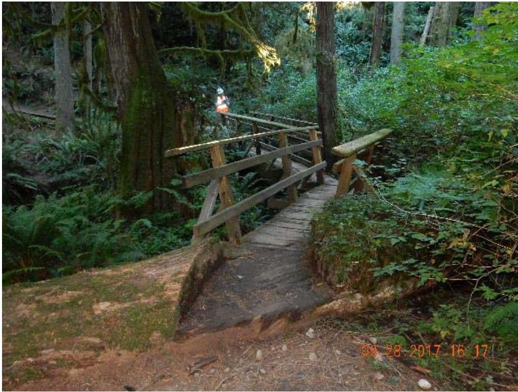
P05 – East approach (DSCN9698.jpg)
