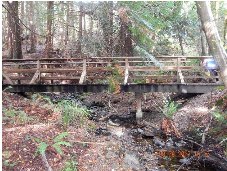
P14 – East side of the bridge (DSCN0098.jpg)
