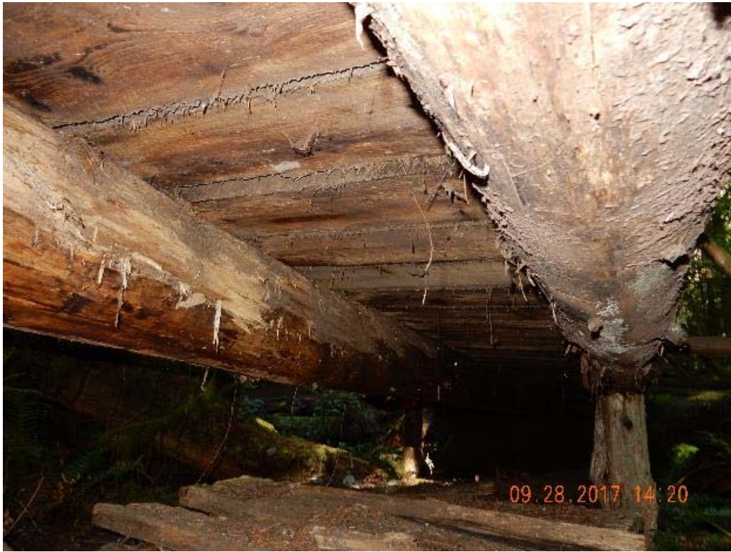
P15 – Under side of the bridge (west span) (DSCN9592.jpg)
