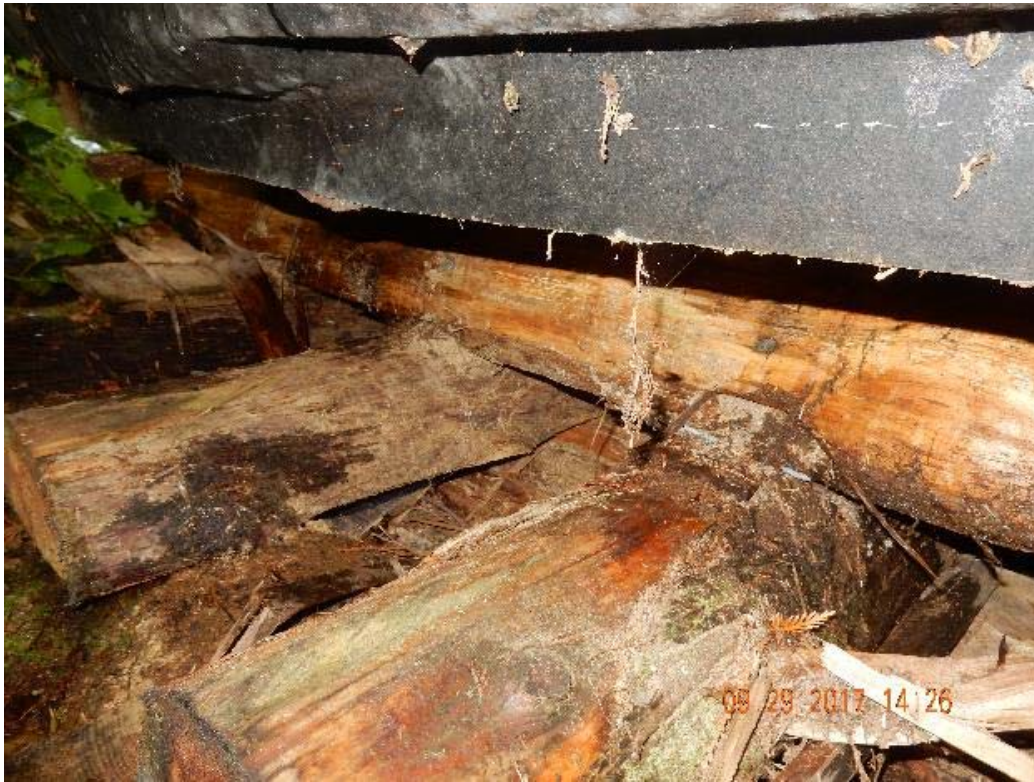
P13 – South abutment (DSCN0048.jpg)
