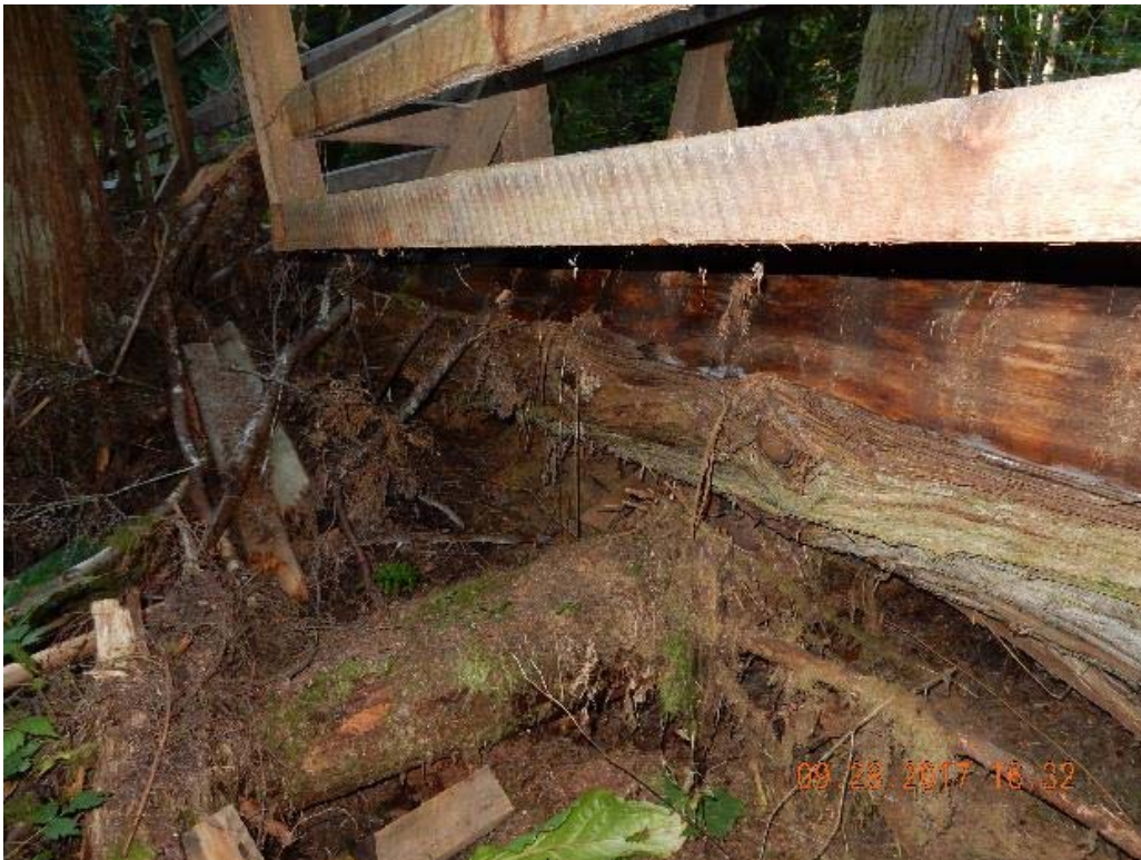
P18 – Side view of the board walk (detail view) (DSCN9732.jpg)
