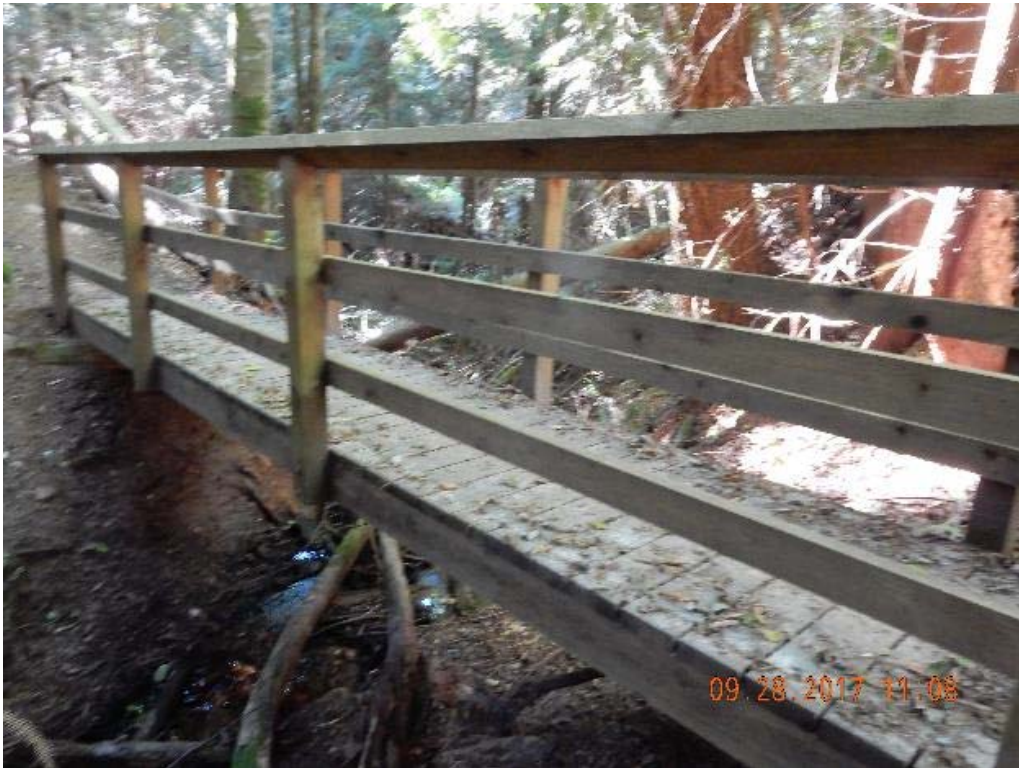
P05 – East side of the bridge (DSCN9493.jpg)
