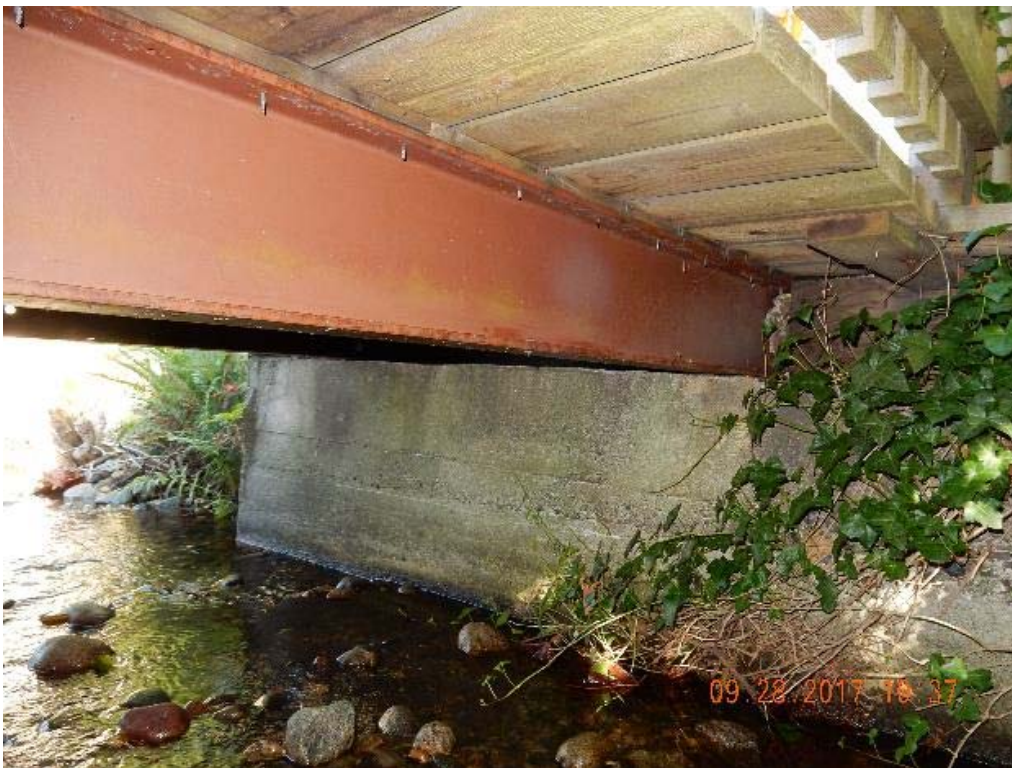
P10 – North abutment (DSCN9483.jpg)
