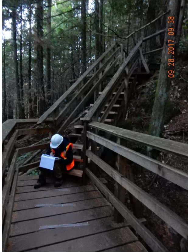
P05 – North end of the bridge (DSCN9449.jpg)
