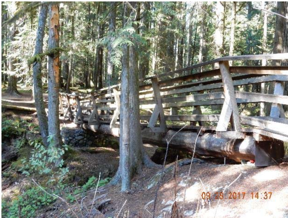
P06 – South side of the bridge (east span) (DSCN9611.jpg)
