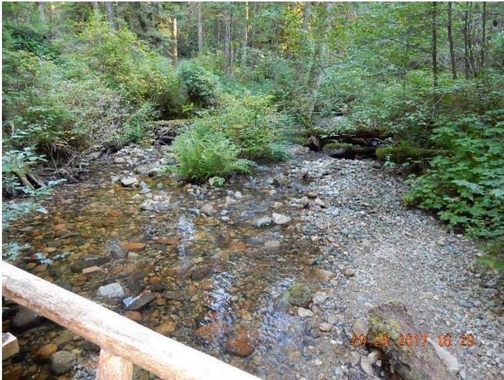
P05 – Downstream (looking south) (DSCN9712.jpg)
