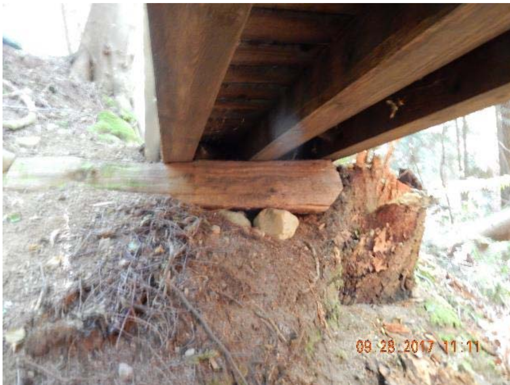
P12 – South abutment (DSCN9502.jpg)
