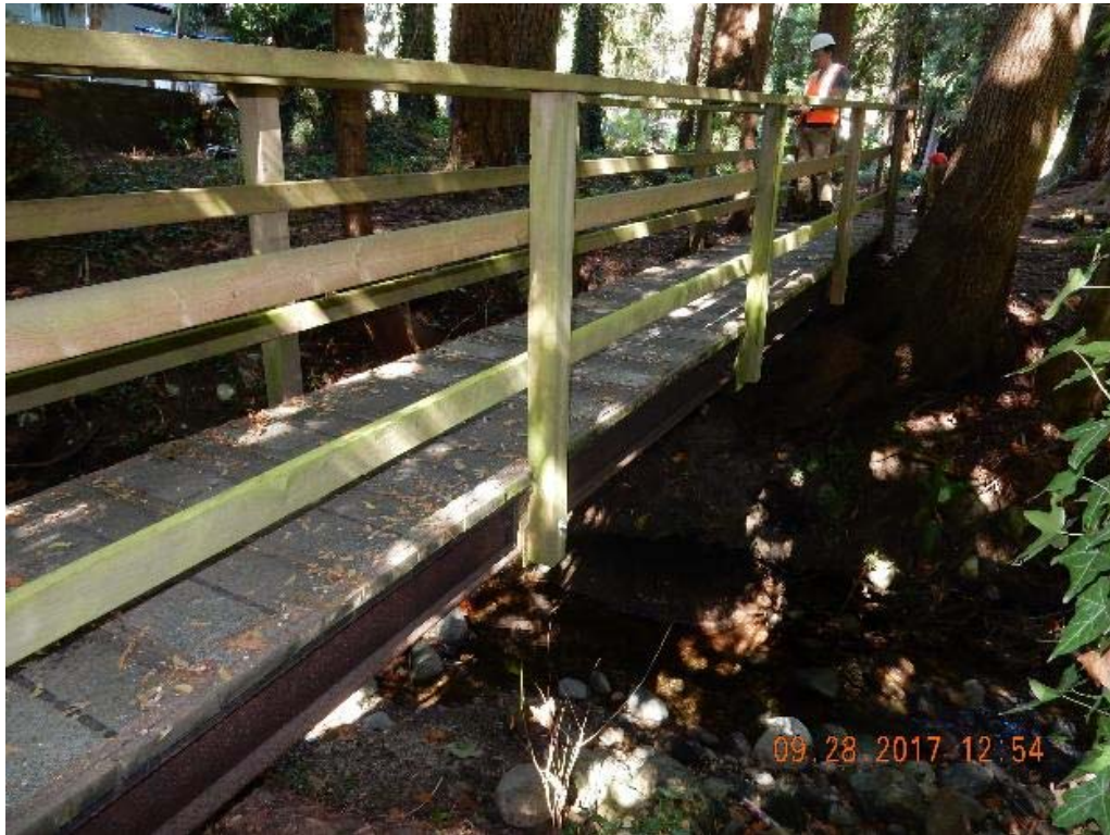
P07 – East side of the bridge (DSCN9568.jpg)
