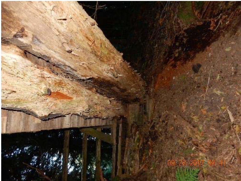
P10 – East abutment (DSCN9413.jpg)
