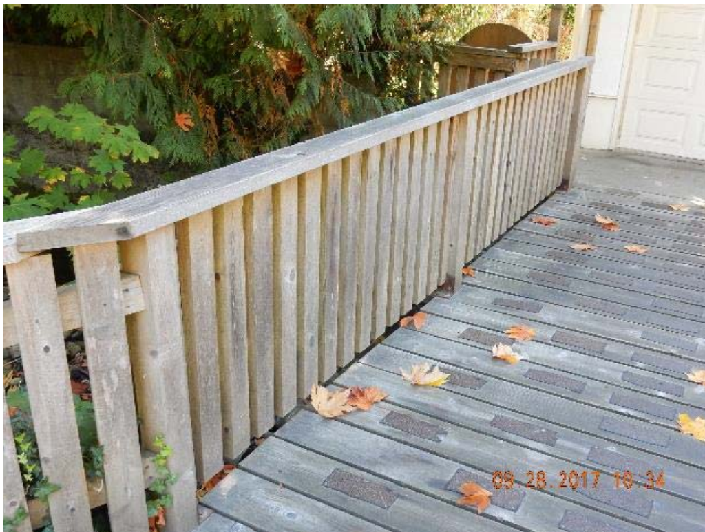
P04 – East railing (DSCN9476.jpg)
