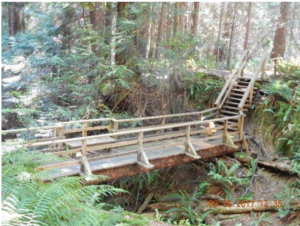
P10 – North side of the bridge (DSCN9551.jpg)
