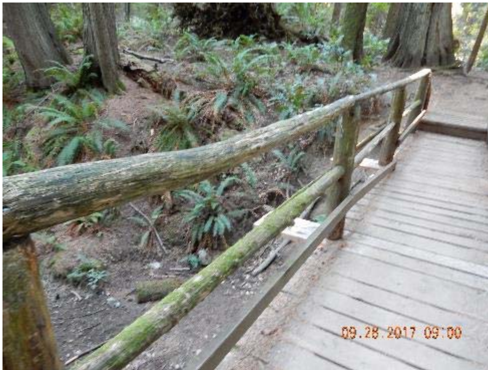
P04 – North railing (DSCN9425.jpg)
