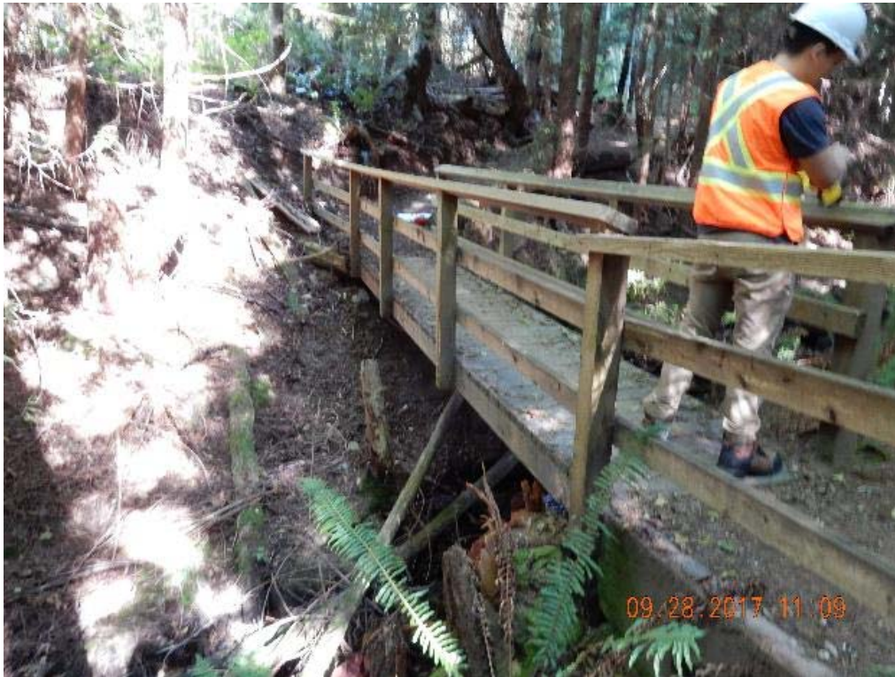
P09 – West side of the bridge (DSCN9498.jpg)
