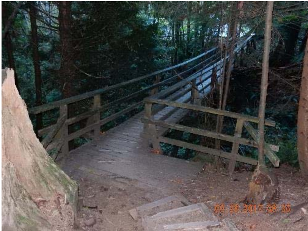
P08 – East approach (DSCN9409.jpg)
