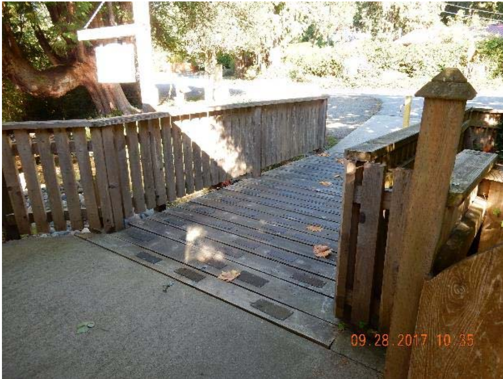
P07 – South approach (DSCN9479.jpg)
