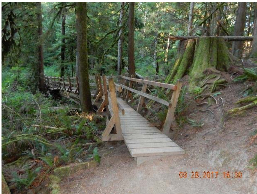
P14 – East approach (DSCN9725.jpg)
