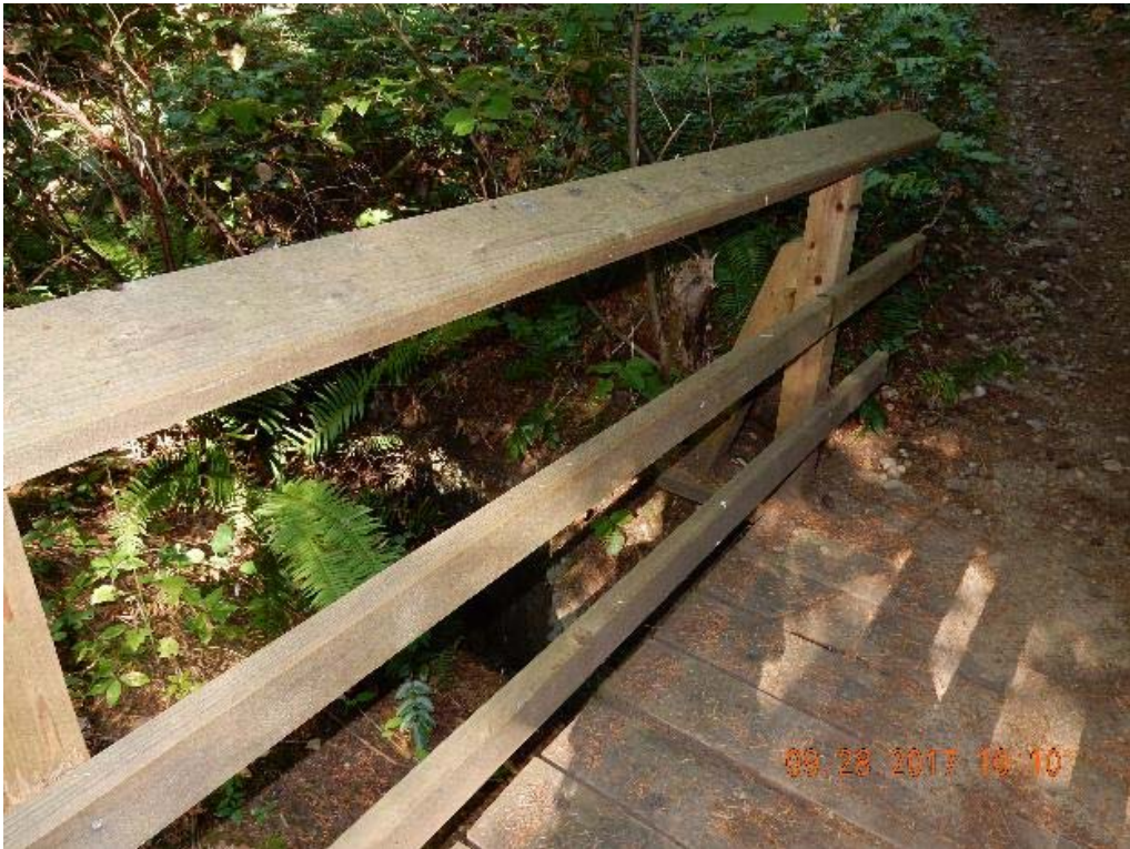
P03 – West railing (DSCN9462.jpg)
