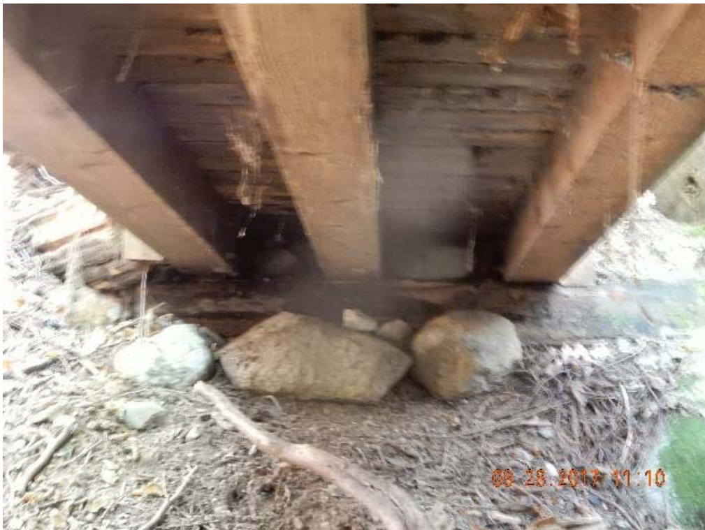
P10 – North abutment (DSCN9500.jpg)
