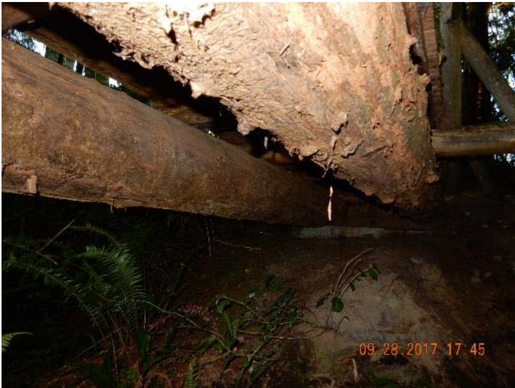
P06 – Under side of the bridge (DSCN9822.jpg)
