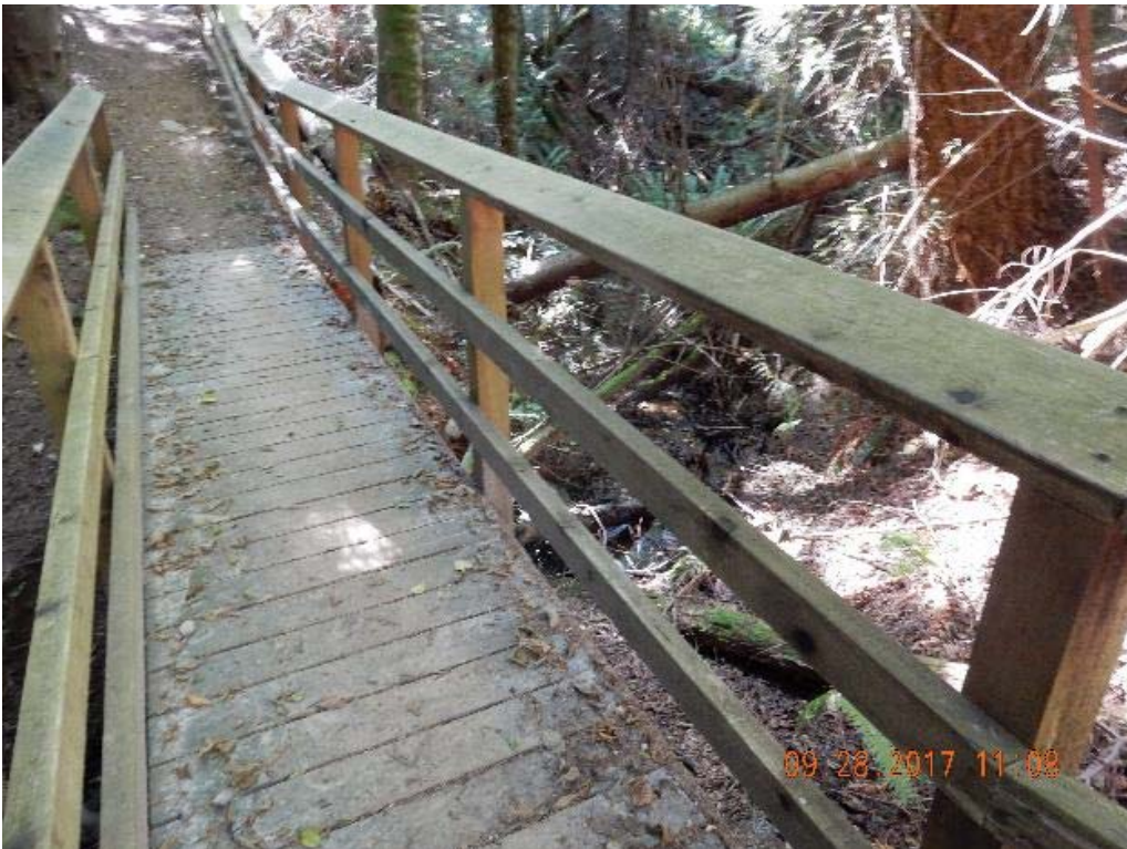
P04 – West railing (DSCN9492.jpg)
