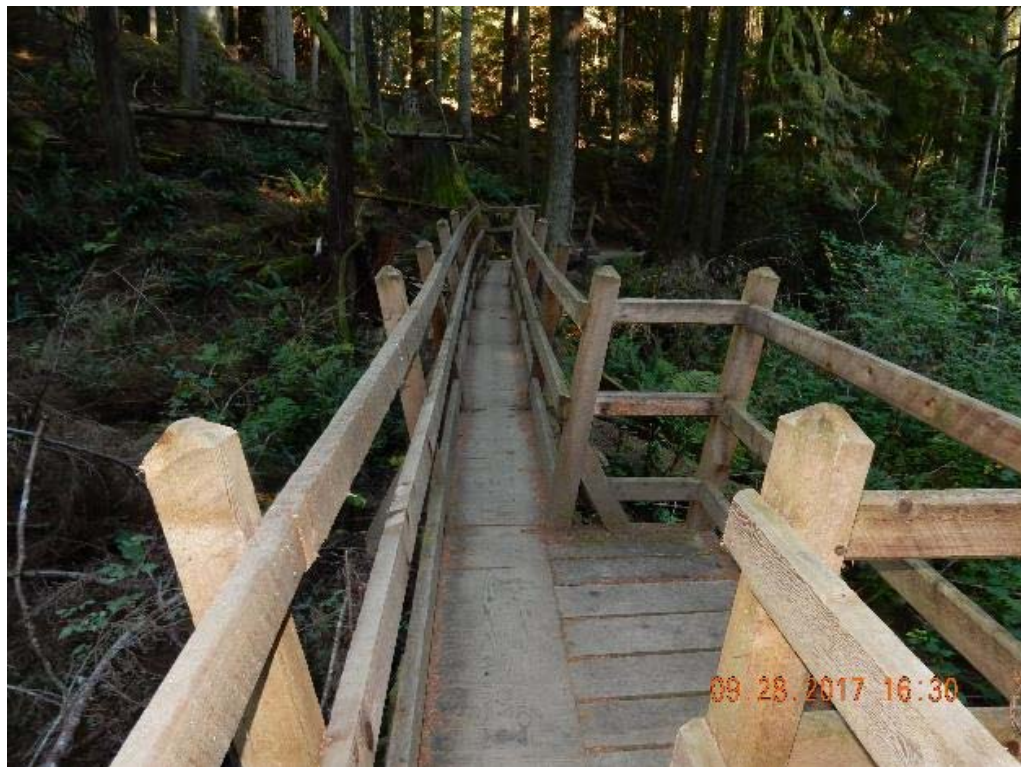
P12 – Overall decking (board walk) (DSCN9721.jpg)
