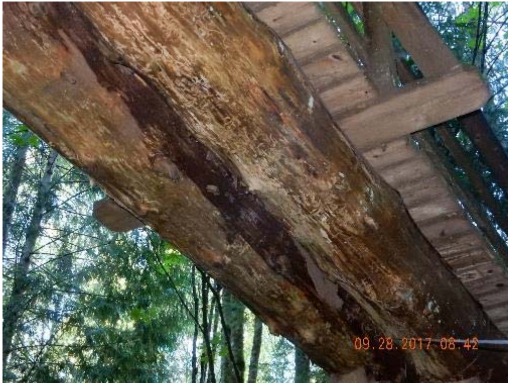
P13 – Underside of the bridge (DSCN9417.jpg)
