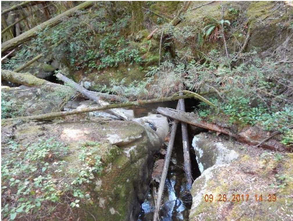
P11 – Downstream (looking south) (DSCN9616.jpg)
