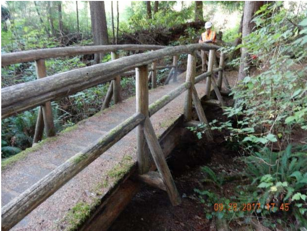
P05 – East side of the bridge (DSCN9821.jpg)
