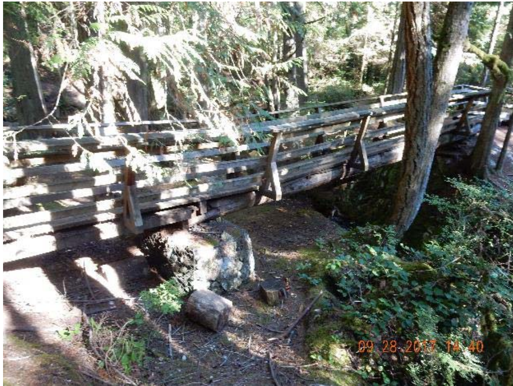
P13 – South side of the bridge (DSCN9618.jpg)
