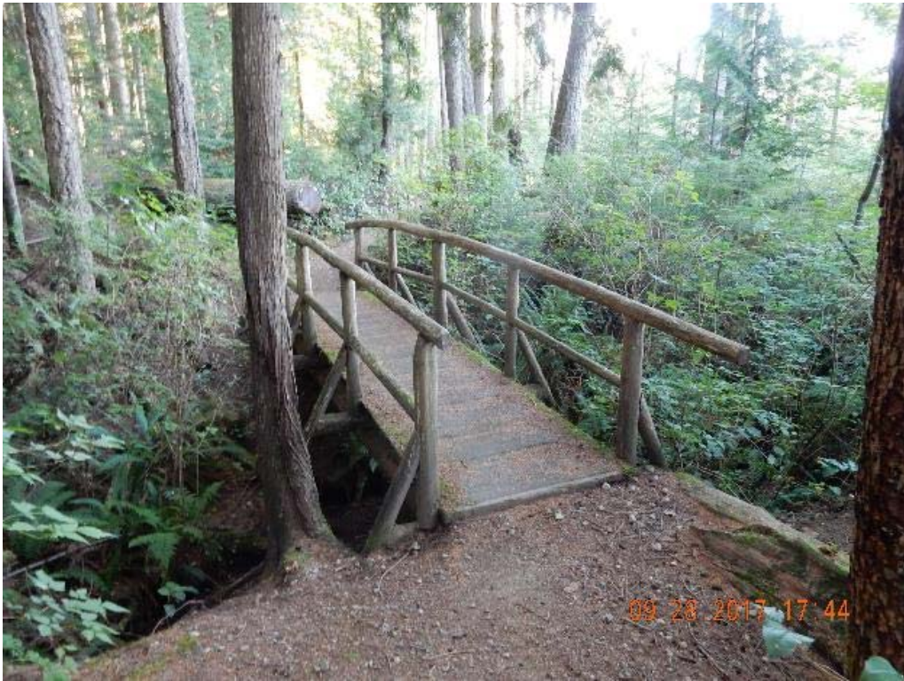
P01 – North approach (DSCN9816.jpg)
