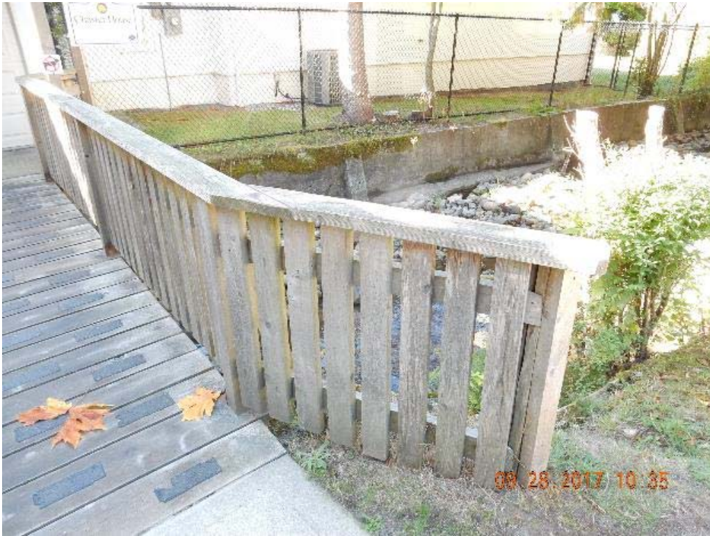
P05 – West railing (DSCN9477.jpg)
