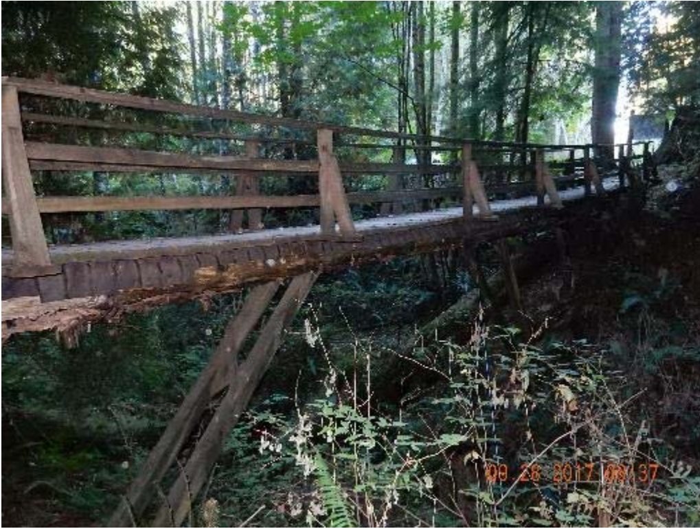
P09 – North side of the bridge (DSCN9410.jpg)
