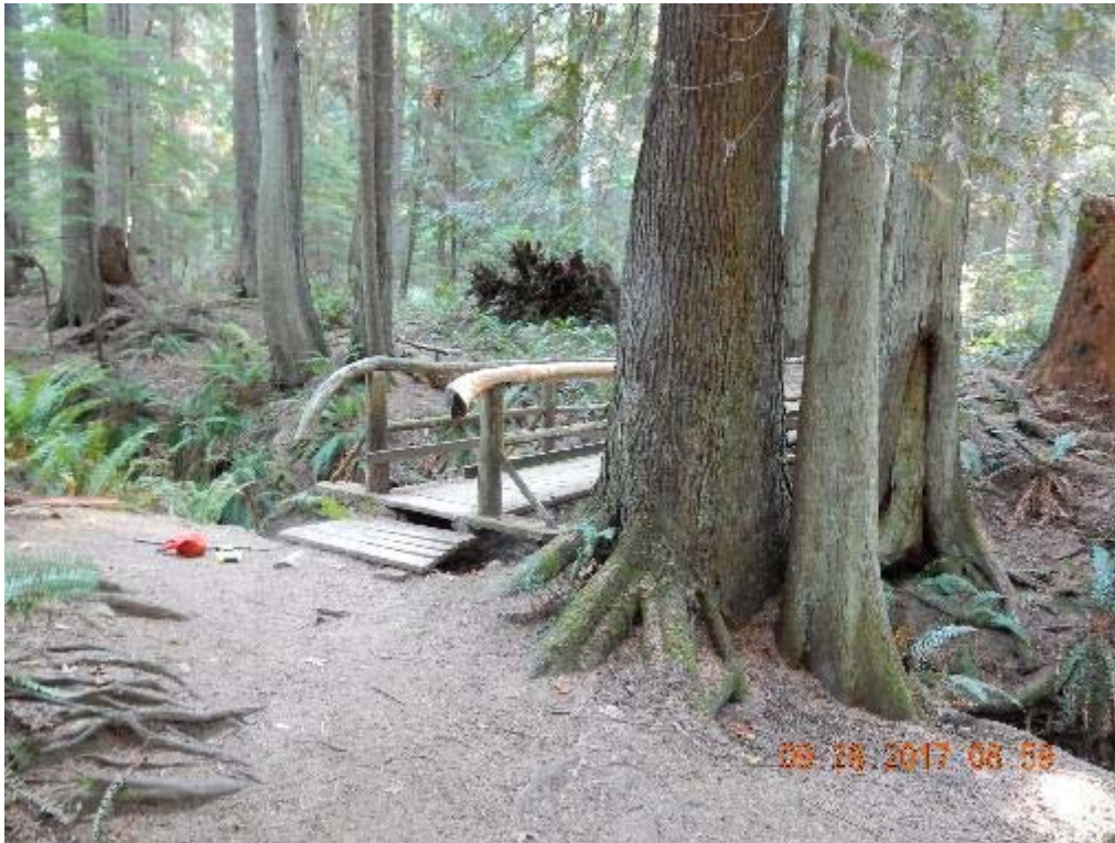
P01 – West approach (DSCN9422.jpg)
