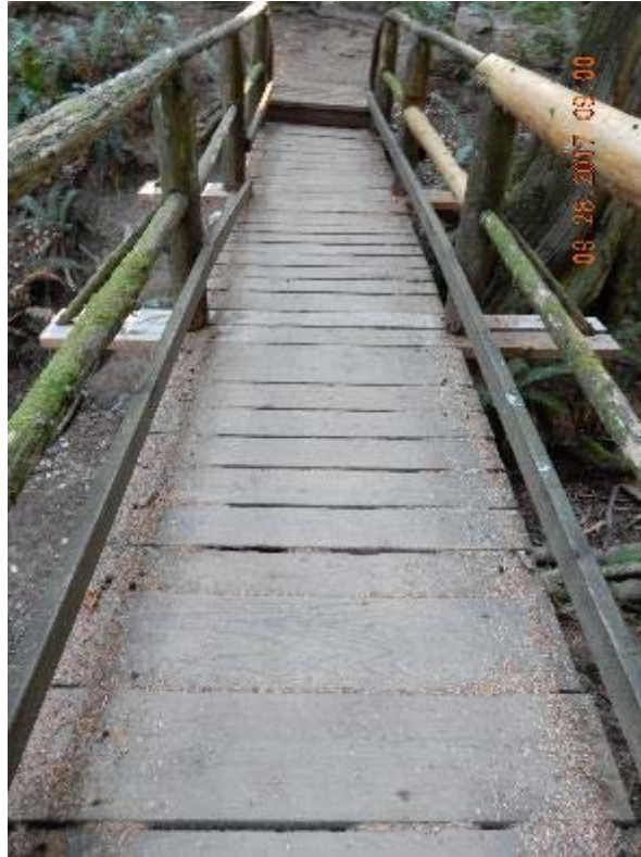
P03 – Overall decking (DSCN9424.jpg)
