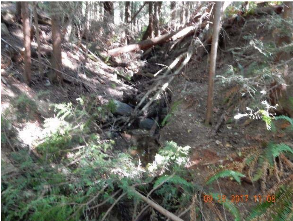
P06 – Upstream (looking east) (DSCN9495.jpg)
