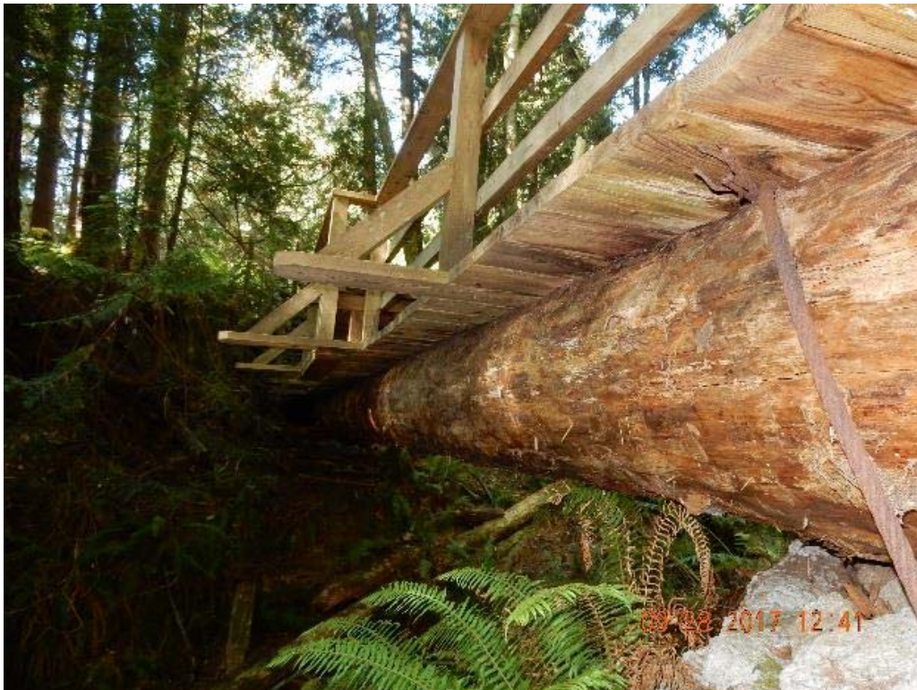
P14 – South side of the bridge (detail view) (DSCN9552.jpg)
