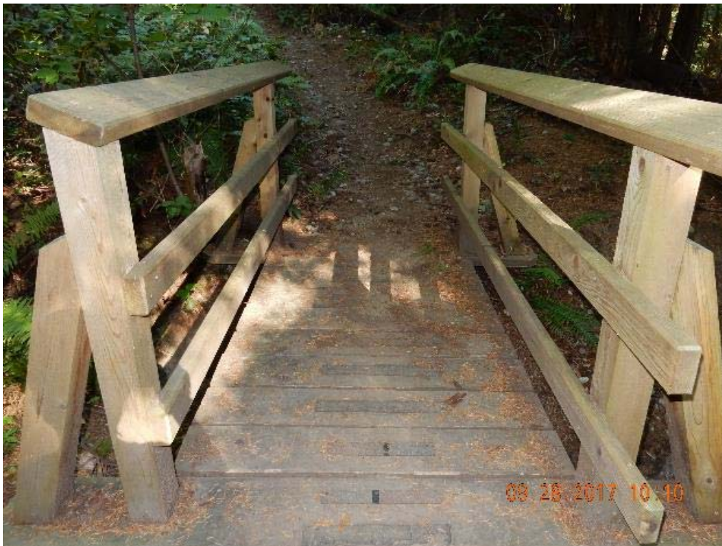
P02 – Overall decking (DSCN9461.jpg)
