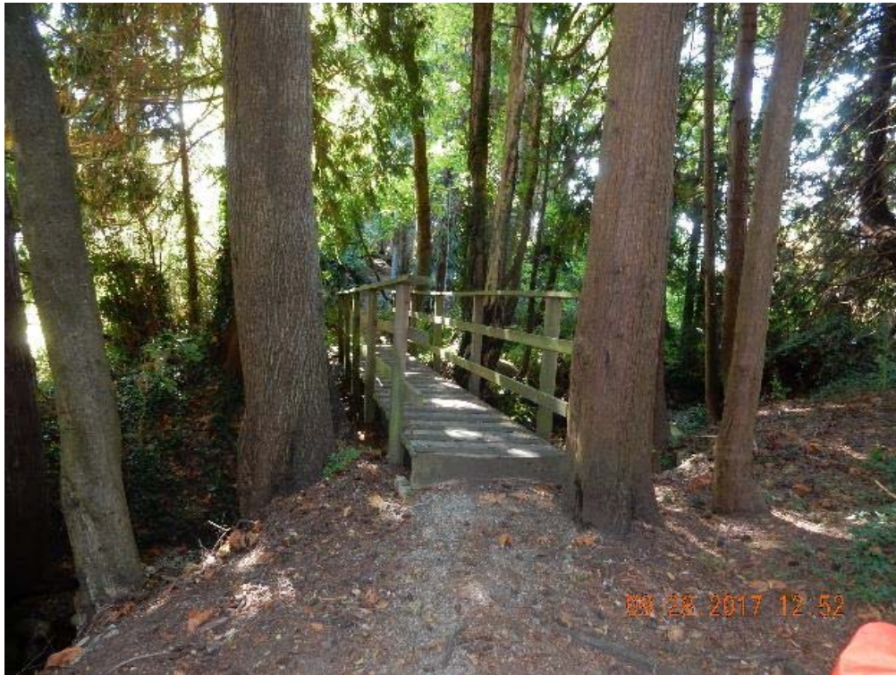
P01 – North approach (DSCN9562.jpg)
