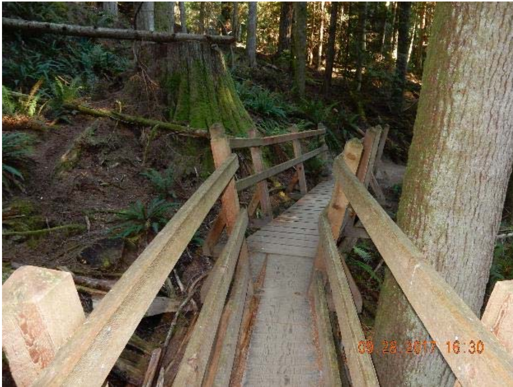
P13 – East end of the bridge (DSCN9723.jpg)
