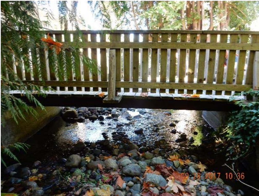
P09 – East side of the bridge (DSCN9481.jpg)
