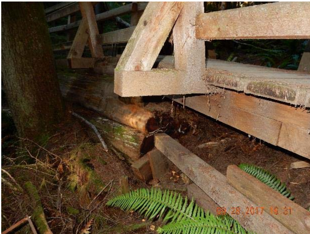
P16 – Side view of the board walk (detail view) (DSCN9727.jpg)
