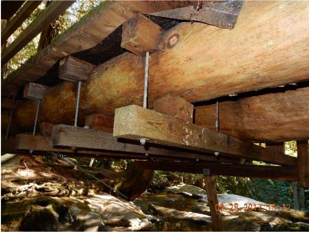
P11 – North side of the bridge (detail view) (DSCN9666.jpg)
