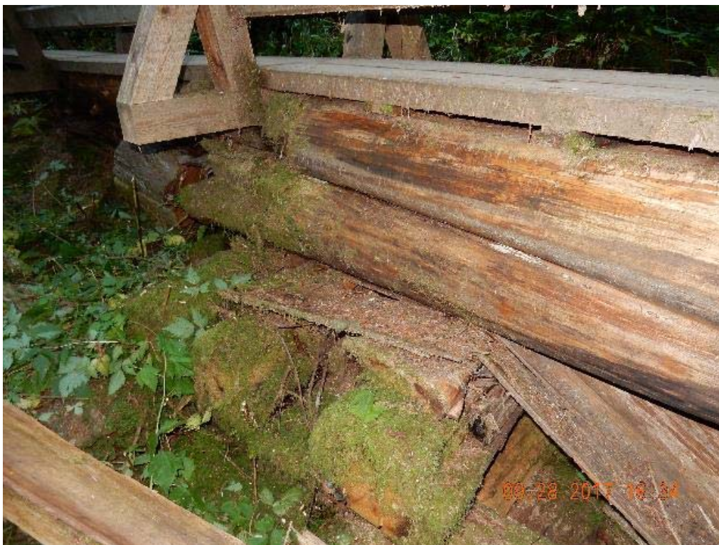
P22 – Side view of the board walk abutment (DSCN9740.jpg)
