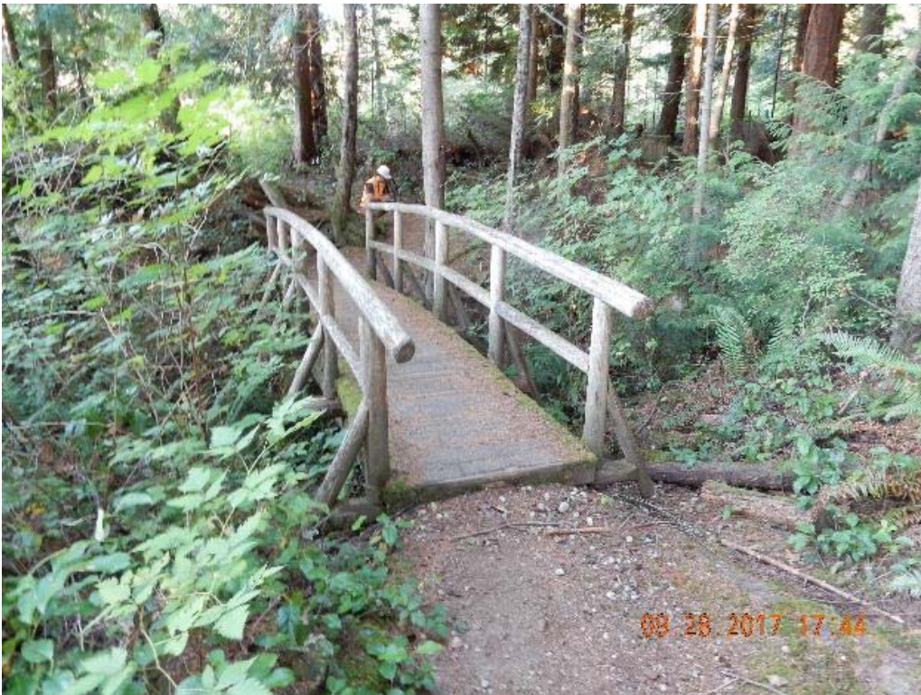
P04 – South approach (DSCN9819.jpg)
