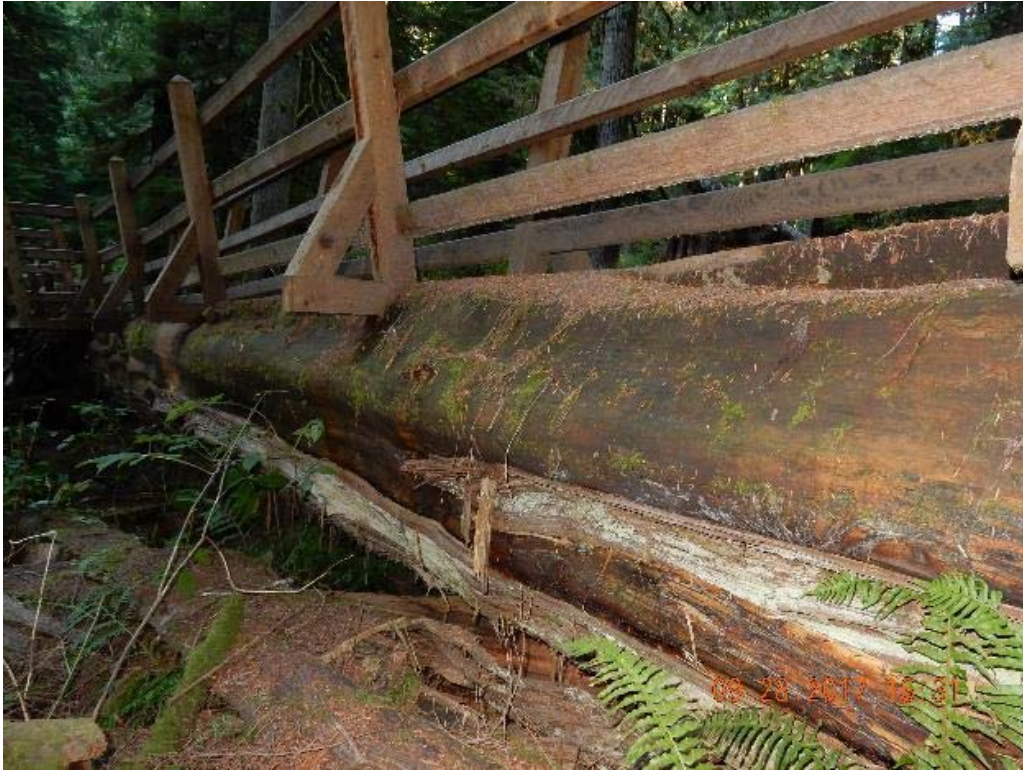
P17 – Side view of the board walk (detail view) (DSCN9729.jpg)
