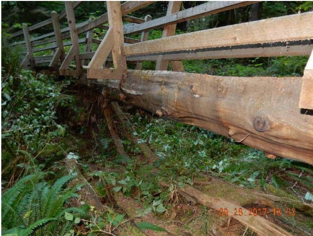
P19 – Side view of the board walk (DSCN9734.jpg)
