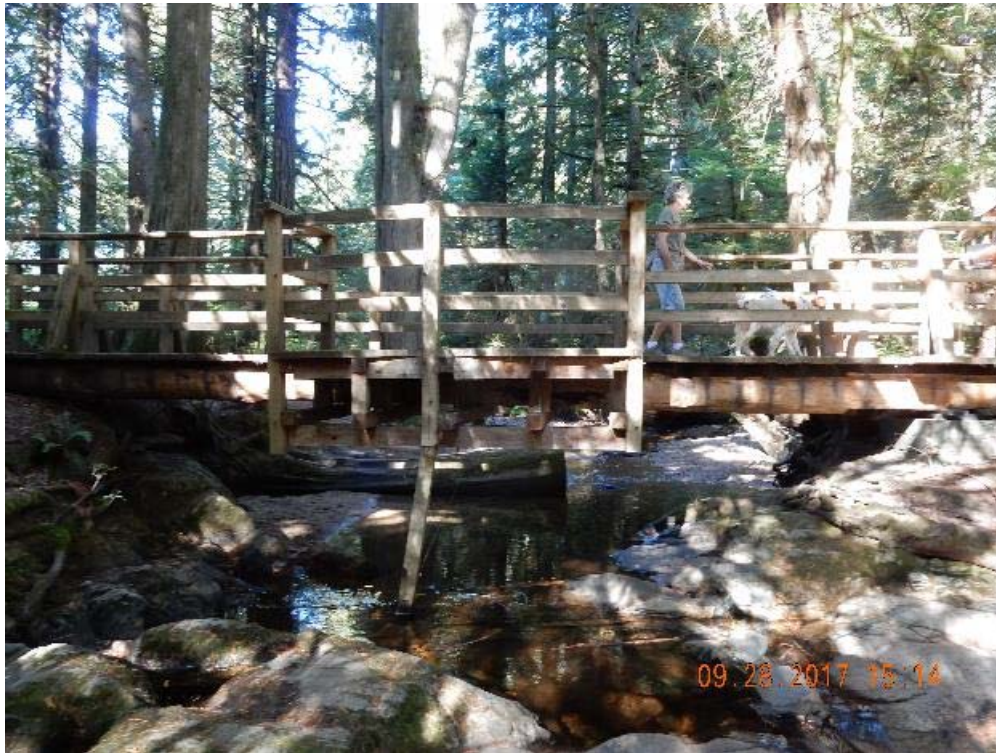
P15 – South side of the bridge (DSCN9671.jpg)
