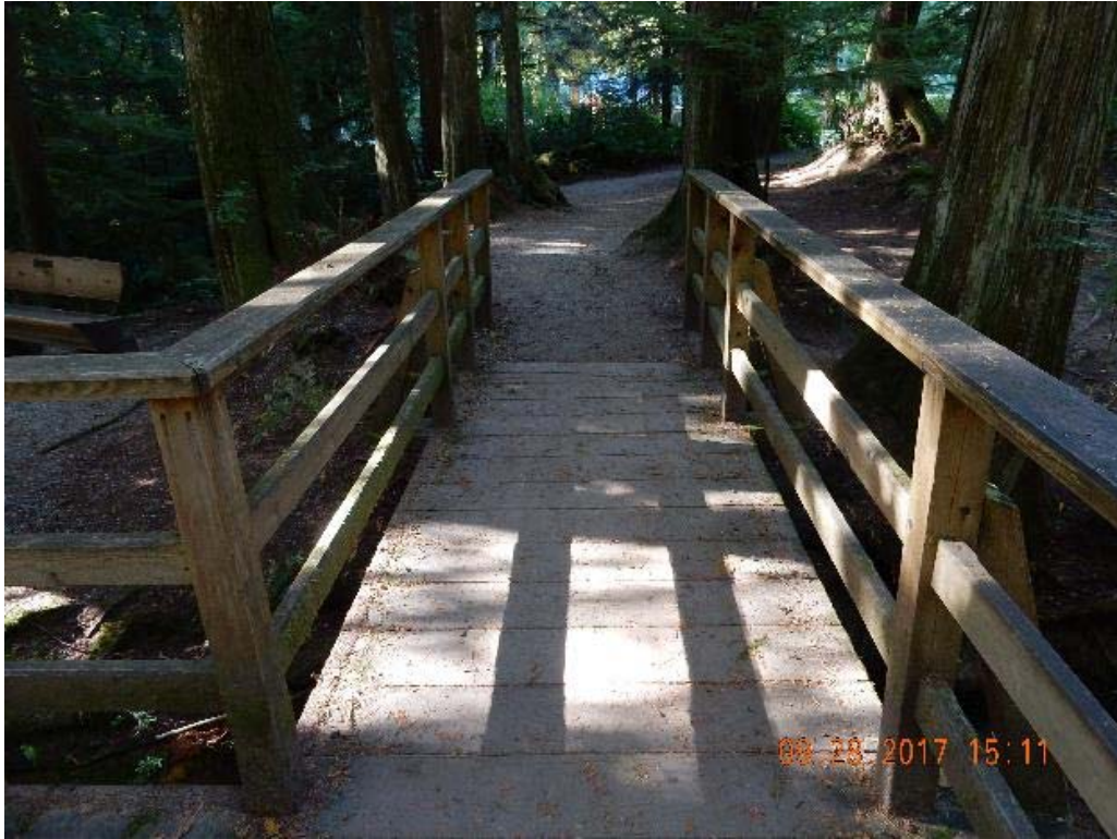
P05 – East end of the bridge (DSCN9658.jpg)
