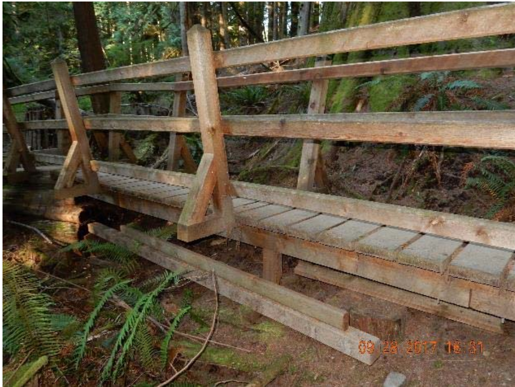
P15 – Side view of the board walk (DSCN9726.jpg)
