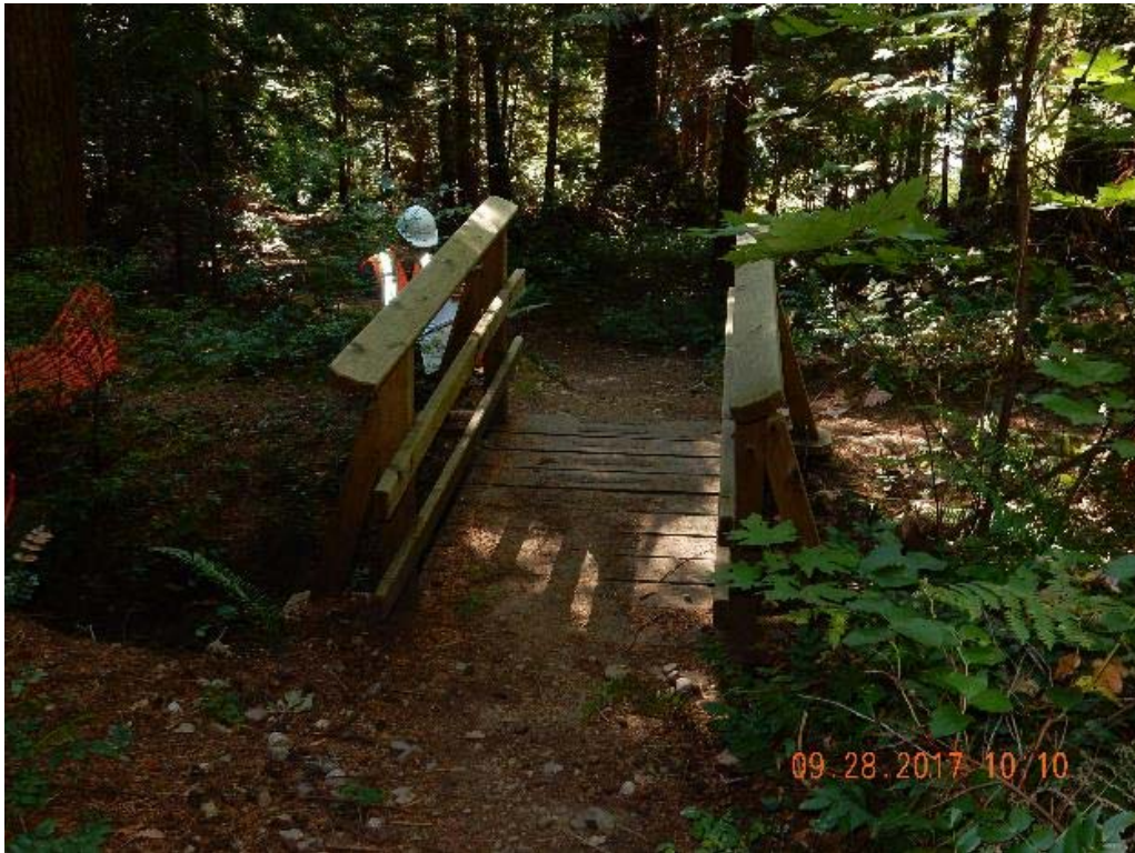
P05 – North approach (DSCN9464.jpg)
