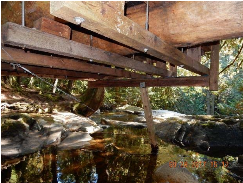
P12 – Under side of the bridge (DSCN9667.jpg)
