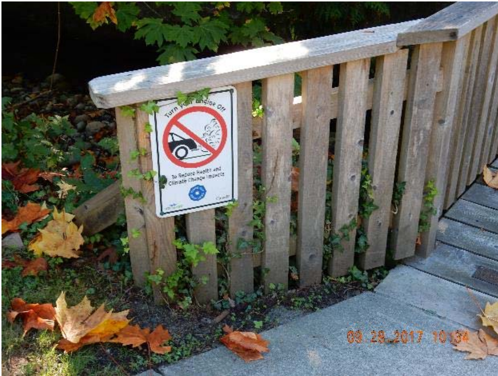
P03 – East railing (DSCN9475.jpg)
