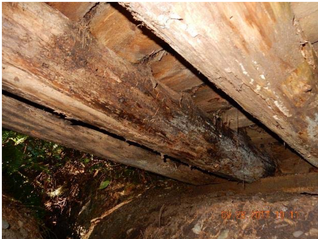
P08 – Under side of the bridge (DSCN9467.jpg)
