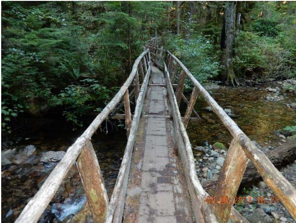
P03 – Overall decking (main span) (DSCN9710.jpg)
