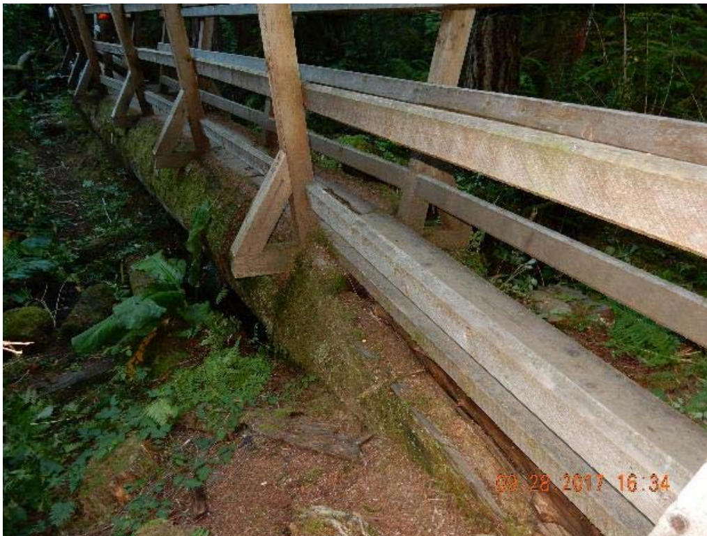
P24 – Side view of the board walk (DSCN9742.jpg)
