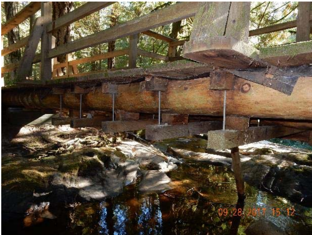
P10 – North side of the bridge (detail view) (DSCN9665.jpg)
