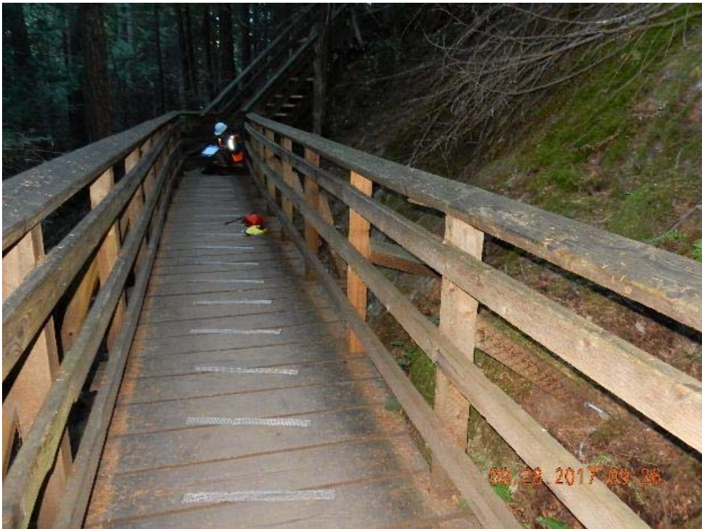
P04 – Overall decking (DSCN9444.jpg)
