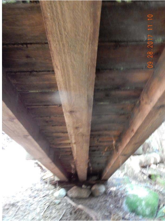
P11 – Under side of the bridge (DSCN9501.jpg)
