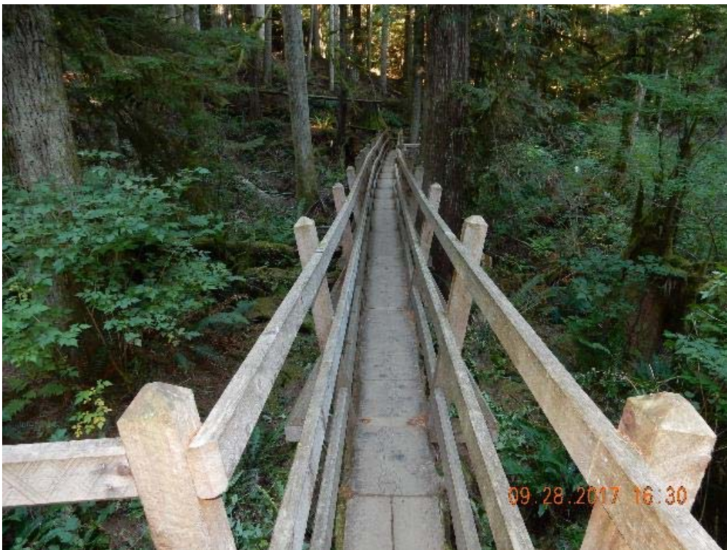
P10 – Overall decking (board walk) (DSCN9718.jpg)
