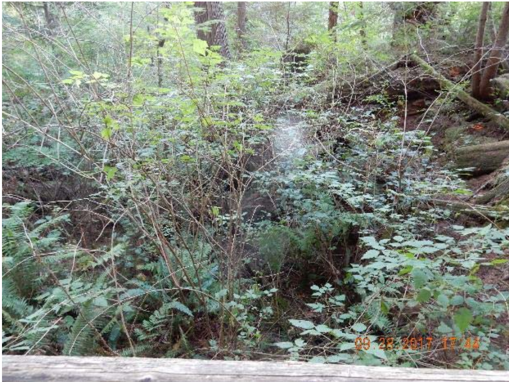
P02 – Downstream (looking west) (DSCN9817.jpg)
