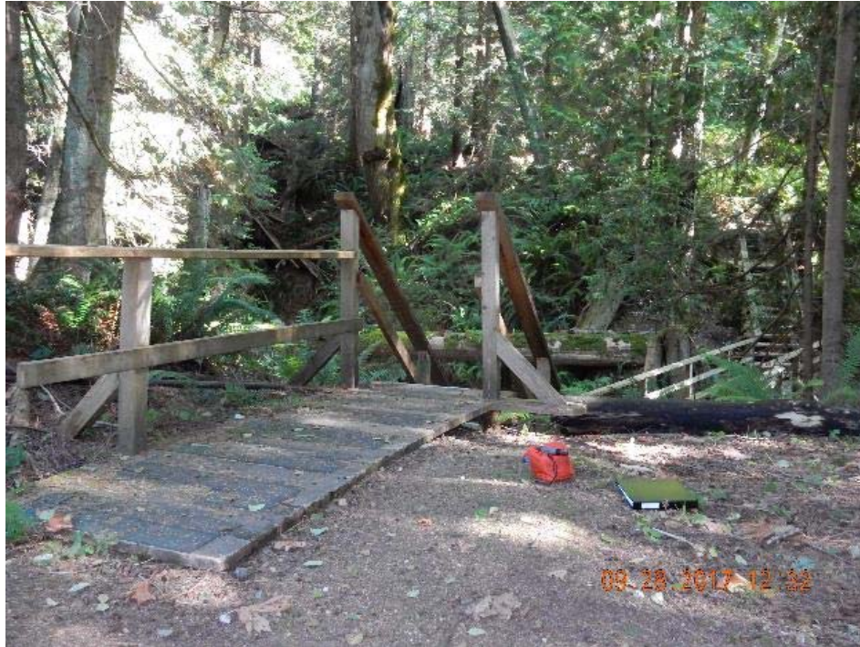
P01 – West approach (DSCN9538.jpg)
