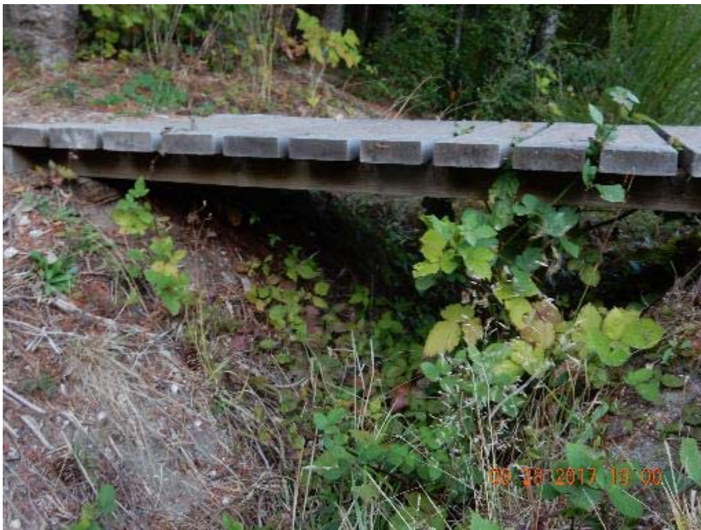
P02 – Side view of the bridge (east bridge) (DSCN9827.jpg)
