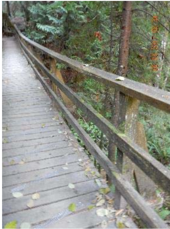
P05 – South railing (DSCN9401.jpg)
