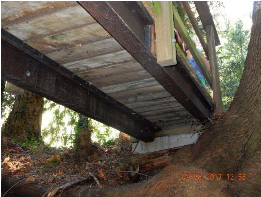
P13 – Under side of the bridge (north end) (DSCN9574.jpg)
