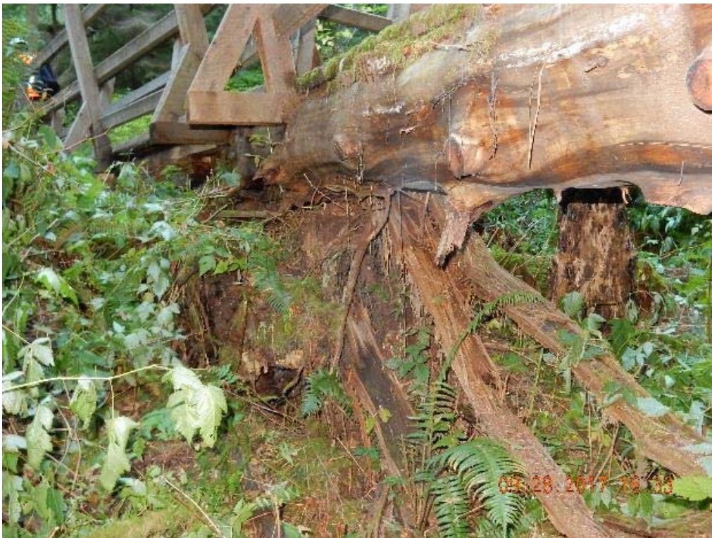
P20 – Side view of the board walk abutment (DSCN9735.jpg)
