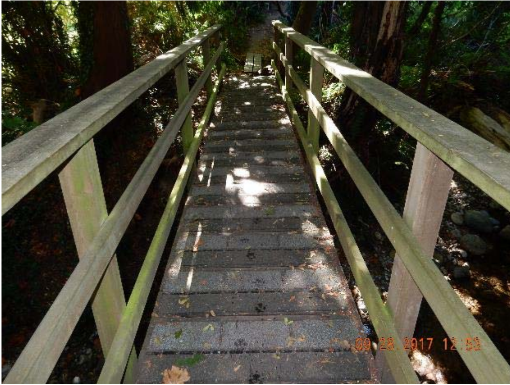
P03 – Overall decking (DSCN9564.jpg)
