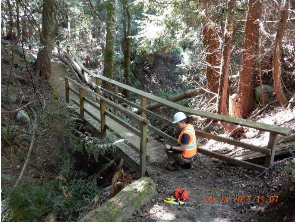
P01 – North approach (DSCN9489.jpg)
