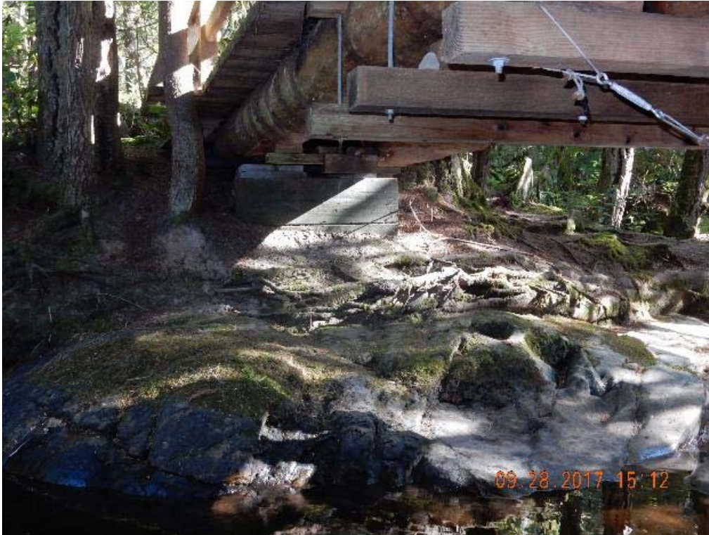
P13 – East abutment (DSCN9669.jpg)
