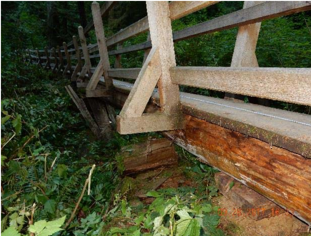
P21 – Side view of the board walk (DSCN9737.jpg)
