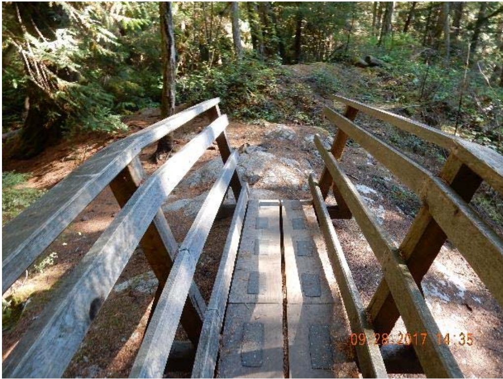
P03 – East end of the bridge (DSCN9607.jpg)
