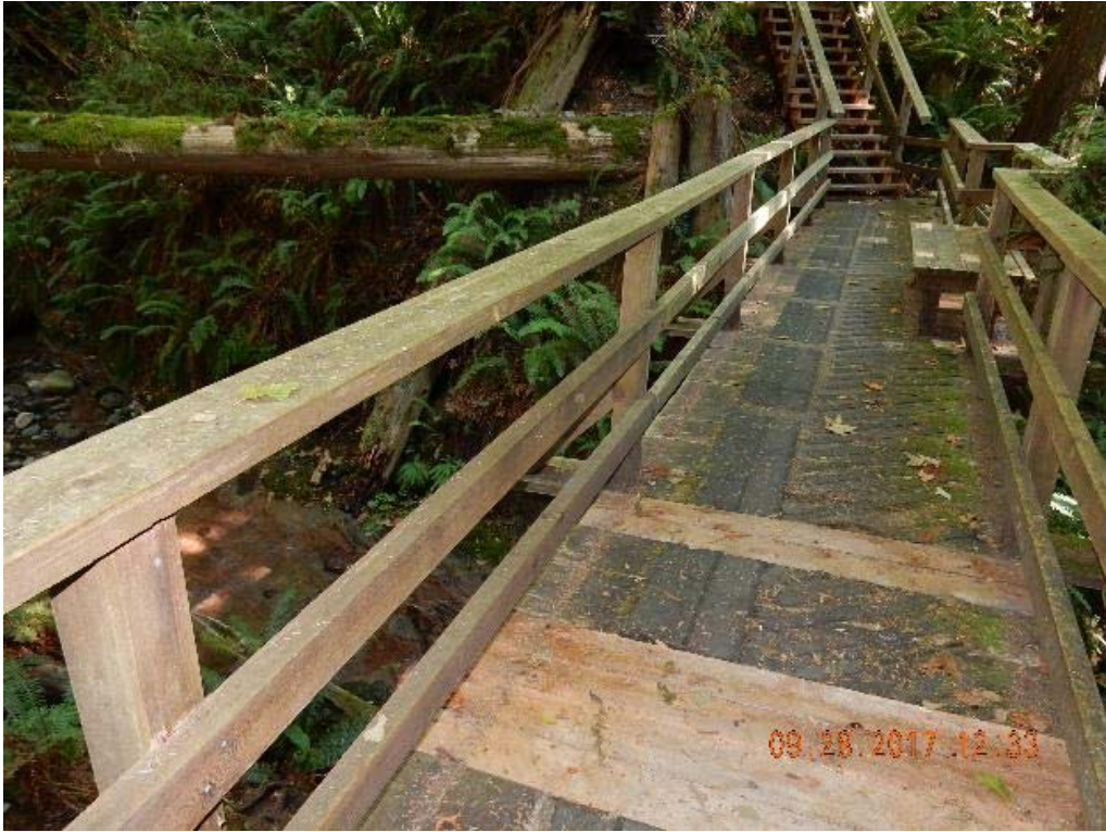
P03 – North railing (DSCN9541.jpg)
