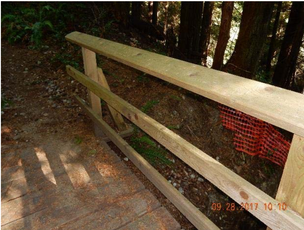
P04 – East railing (DSCN9463.jpg)
