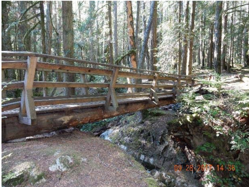
P05 – North side of the bridge (east span) (DSCN9610.jpg)
