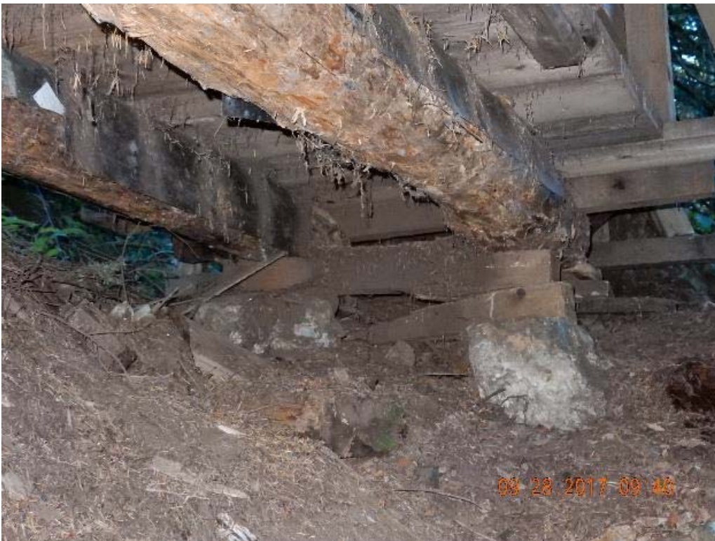
P08 – South abutment (DSCN9452.jpg)
