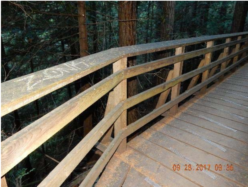
P03 – West railing (DSCN9443.jpg)
