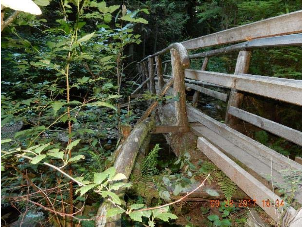
P25 – East end of the main span (DSCN9744.jpg)
