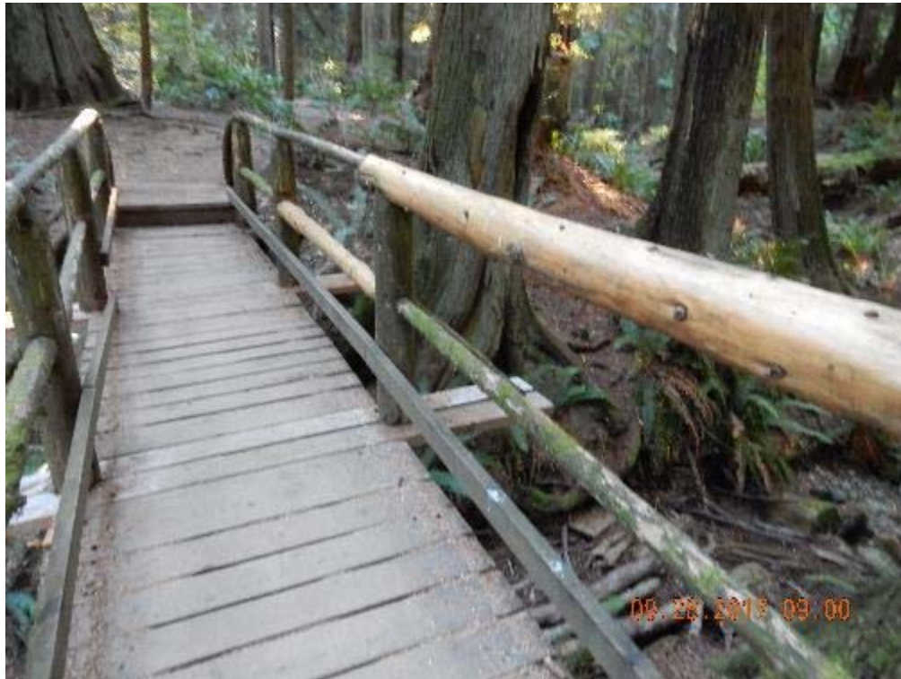
P05 – South railing (DSCN9426.jpg)
