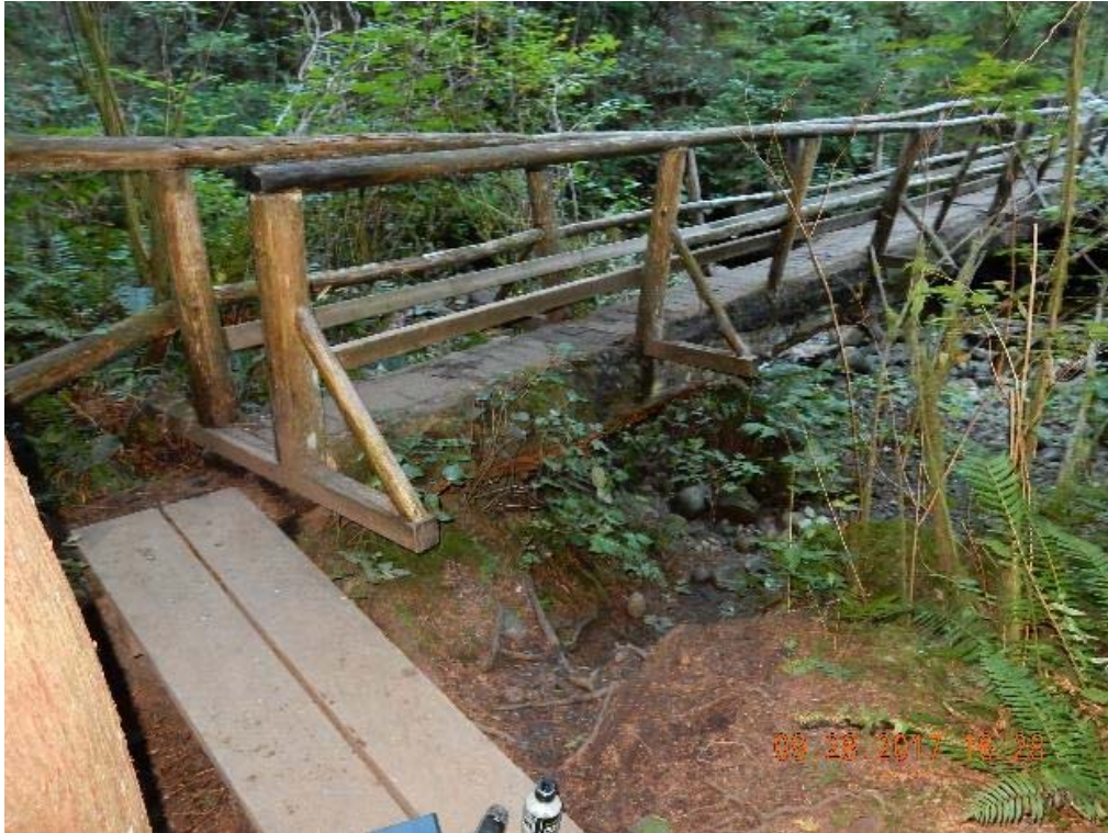
P01 – West approach (DSCN9708.jpg)
