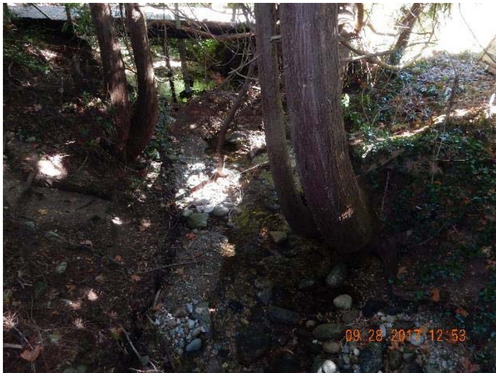
P04 – Upstream (looking east) (DSCN9565.jpg)
