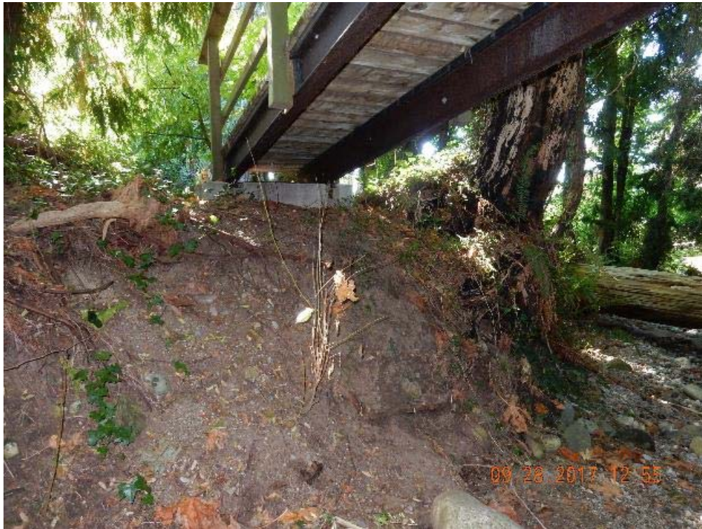
P11 – South embankment (DSCN9572.jpg)
