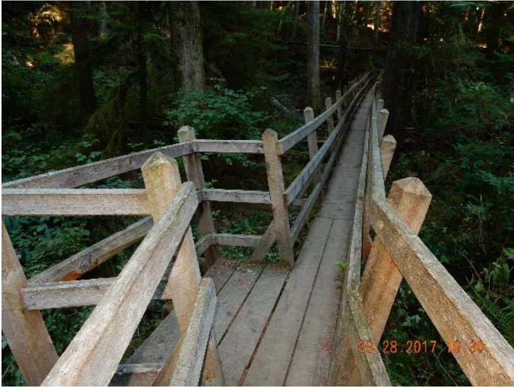
P09 – Overall decking (board walk) (DSCN9717.jpg)
