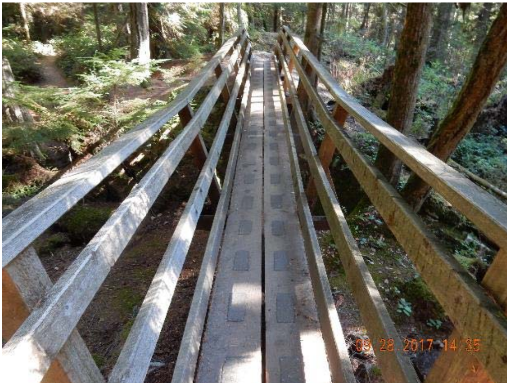
P02 – Overall decking (DSCN9604.jpg)
