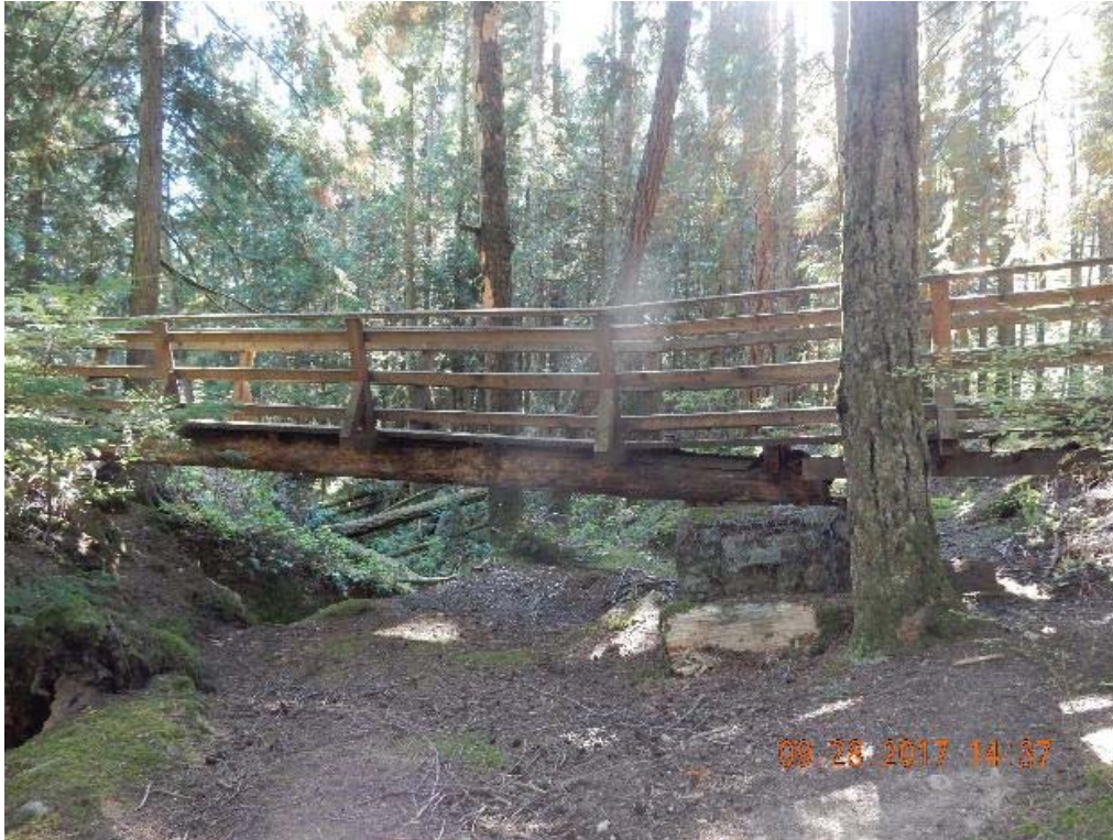
P07 – North side of the bridge (east span) (DSCN9612.jpg)
