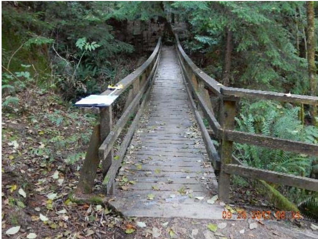
P02 – West end of bridge (DSCN9398.jpg)
