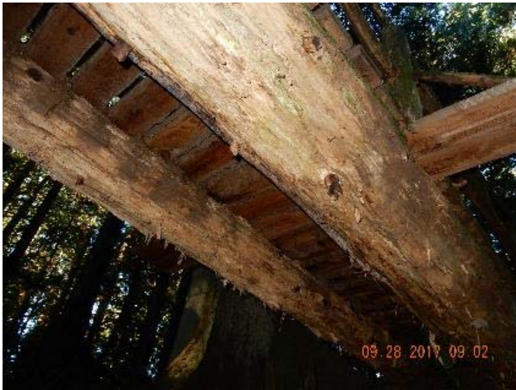
P10 – Underside of the bridge (DSCN9435.jpg)
