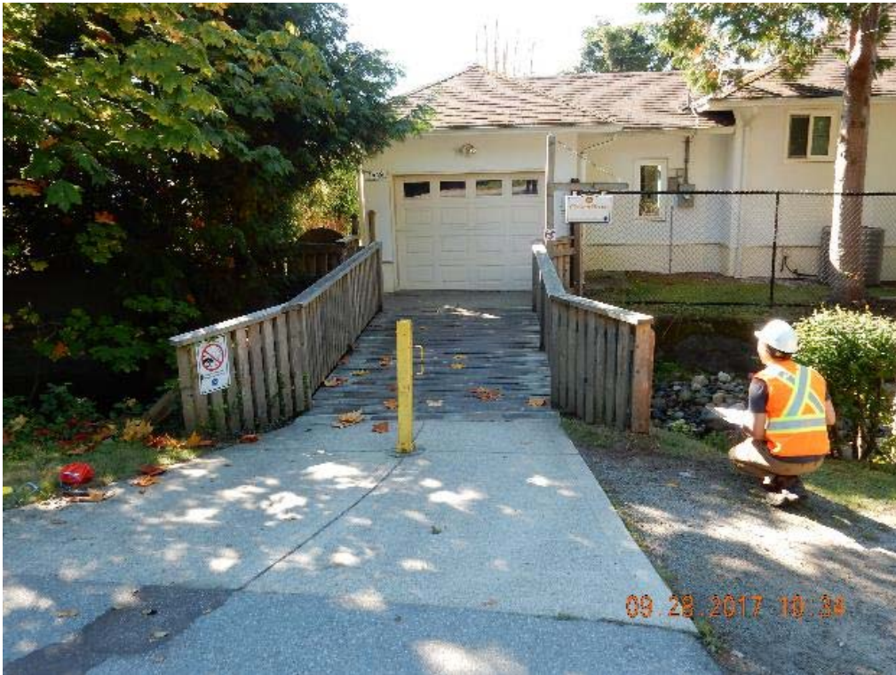
P01 – North approach (DSCN9473.jpg)
