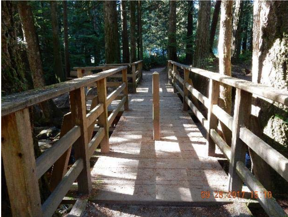
P03 – East end of the bridge (DSCN9655.jpg)
