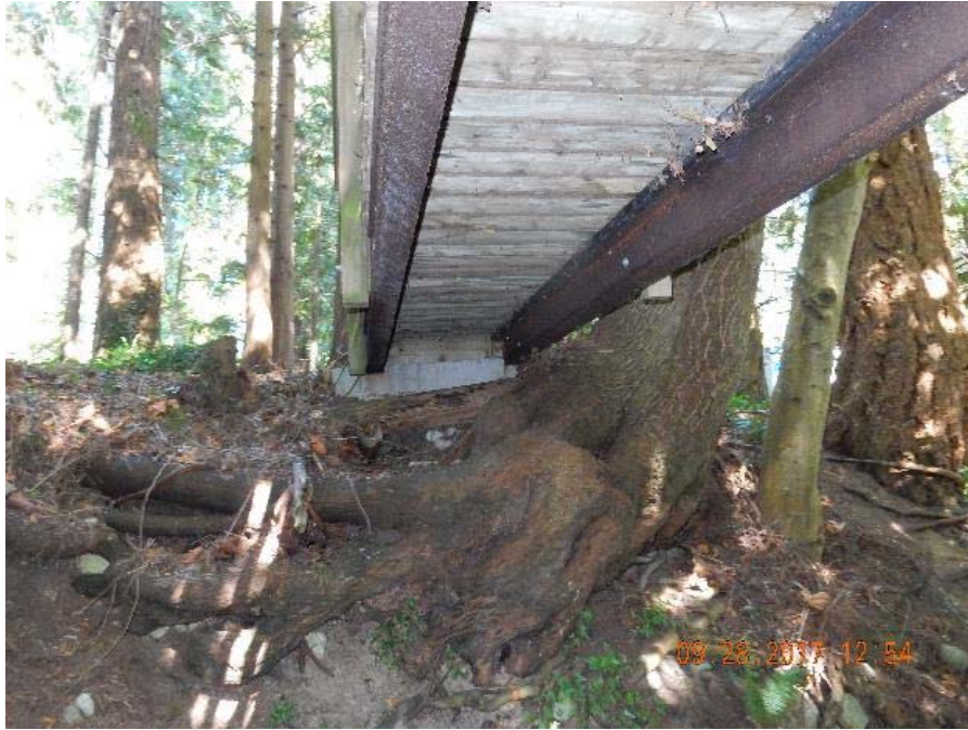
P09 – North abutment (DSCN9570.jpg)
