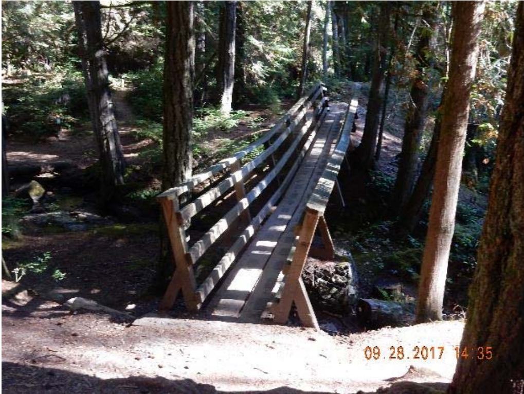
P01 – West approach (DSCN9602.jpg)
