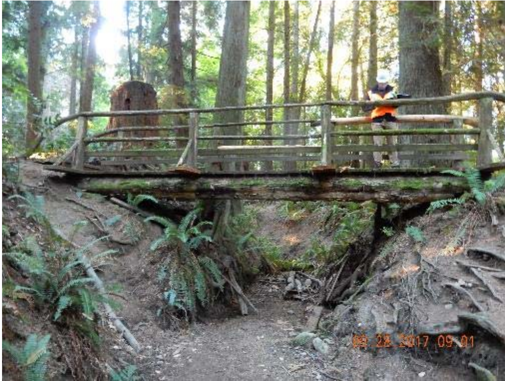
P07 – North side of the bridge (Upstream) (DSCN9431.jpg)
