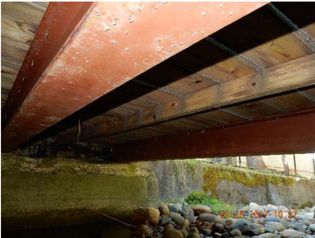
P12 – Underside of the bridge (DSCN9485.jpg)
