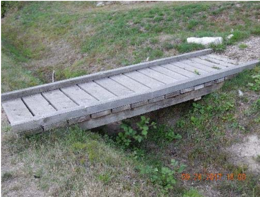
P03 – Overview (west bridge) (DSCN9828.jpg)
