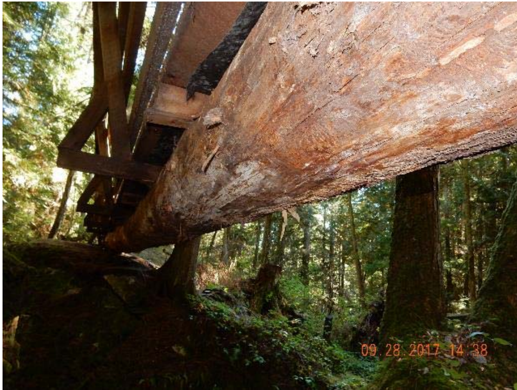
P09 – Under side of the bridge (east span) (DSCN9614.jpg)
