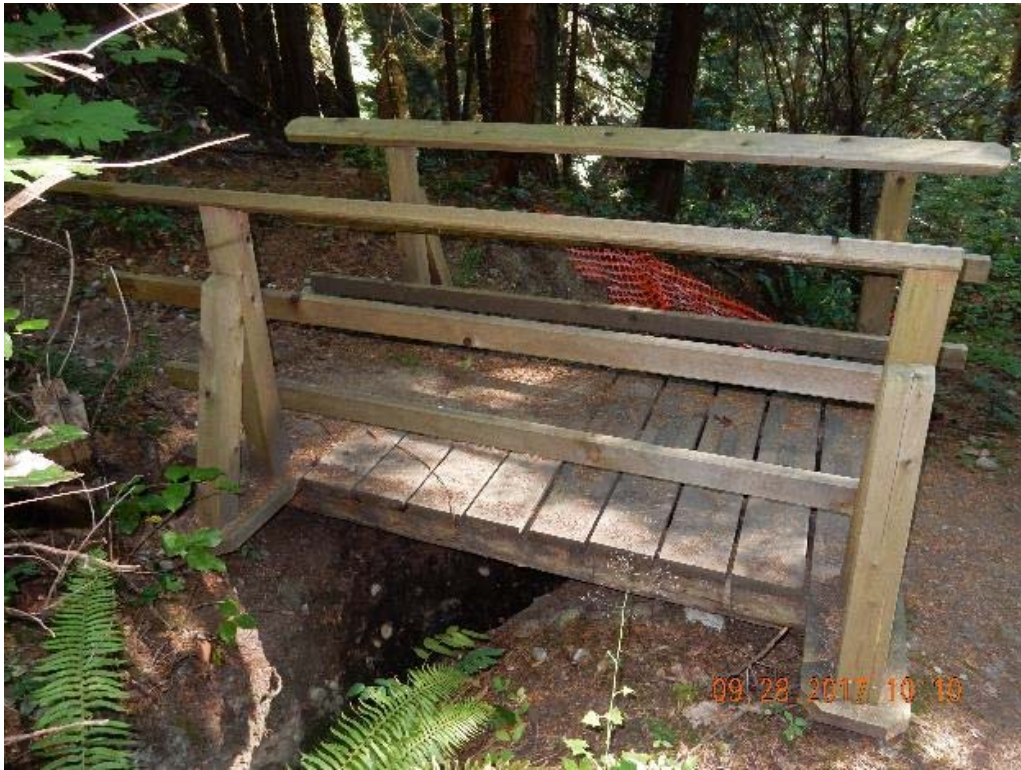
P07 – West side of the bridge (DSCN9466.jpg)
