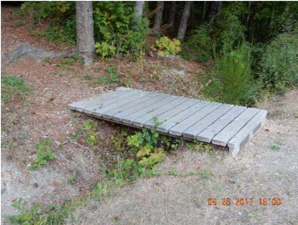
P01 – Overview (east bridge) (DSCN9826.jpg)
