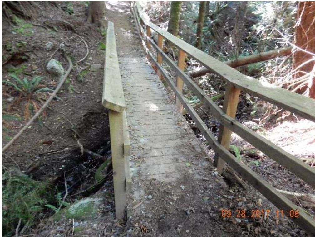
P02 – Overall decking (DSCN9490.jpg)
