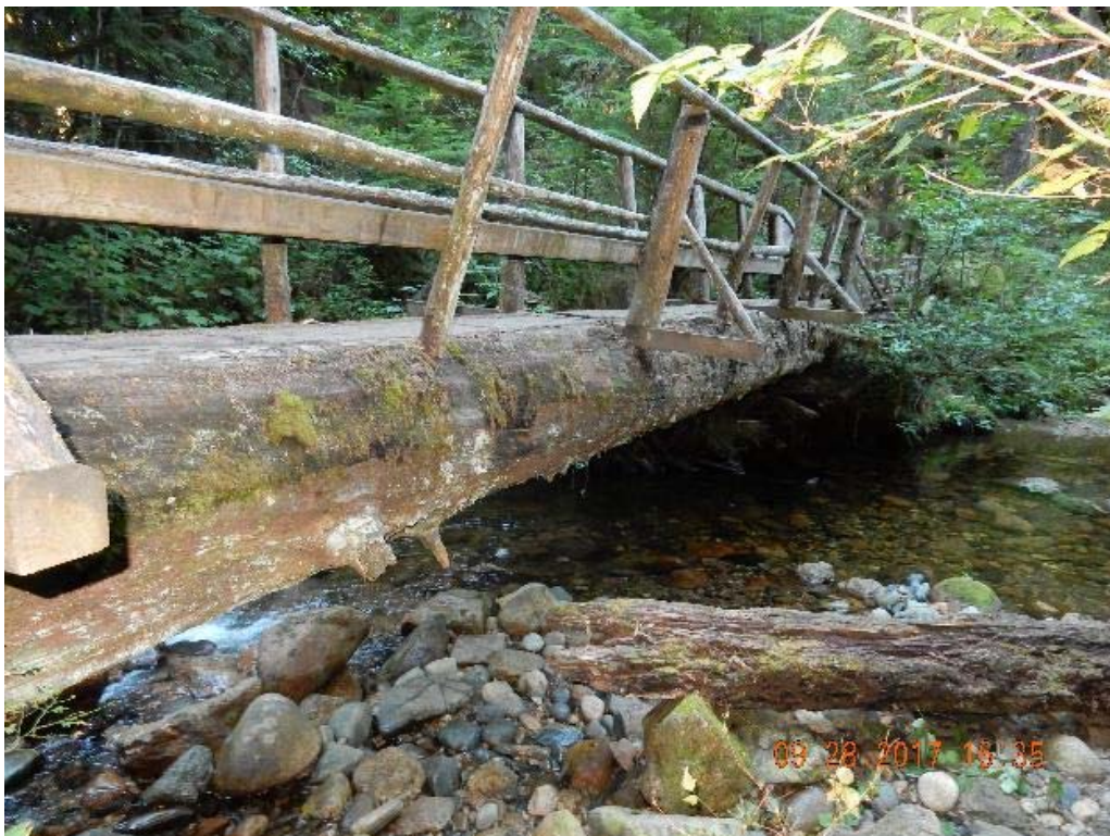
P26 – South side of the main span (DSCN9745.jpg)
