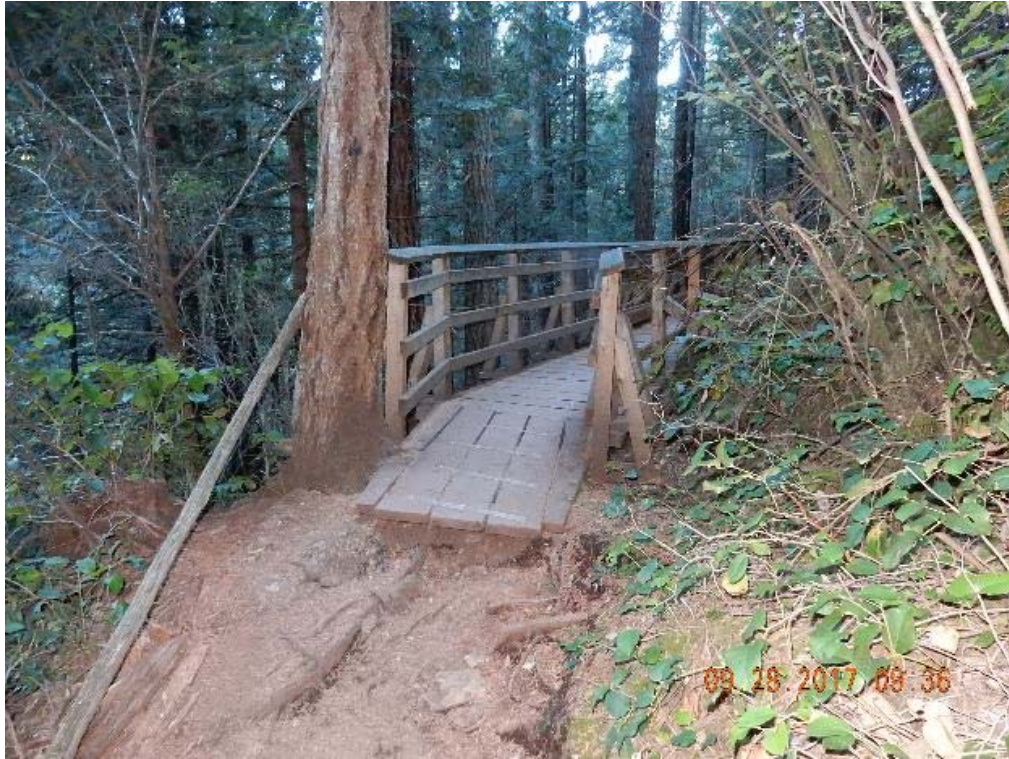
P01 – South approach (DSCN9441.jpg)
