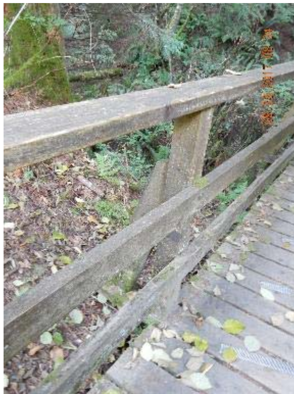
P04 – North railing (DSCN9400.jpg)
