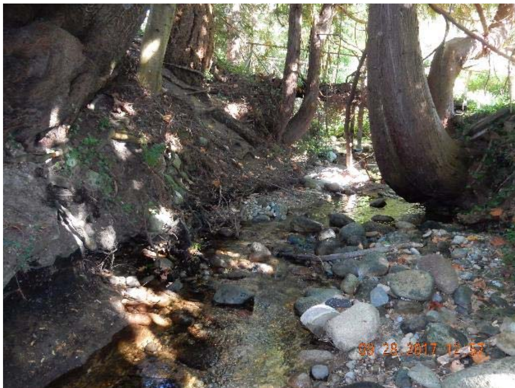
P14 – Suggest relocating rocks on the right to the embankment on the left. (DSCN9575.jpg)
