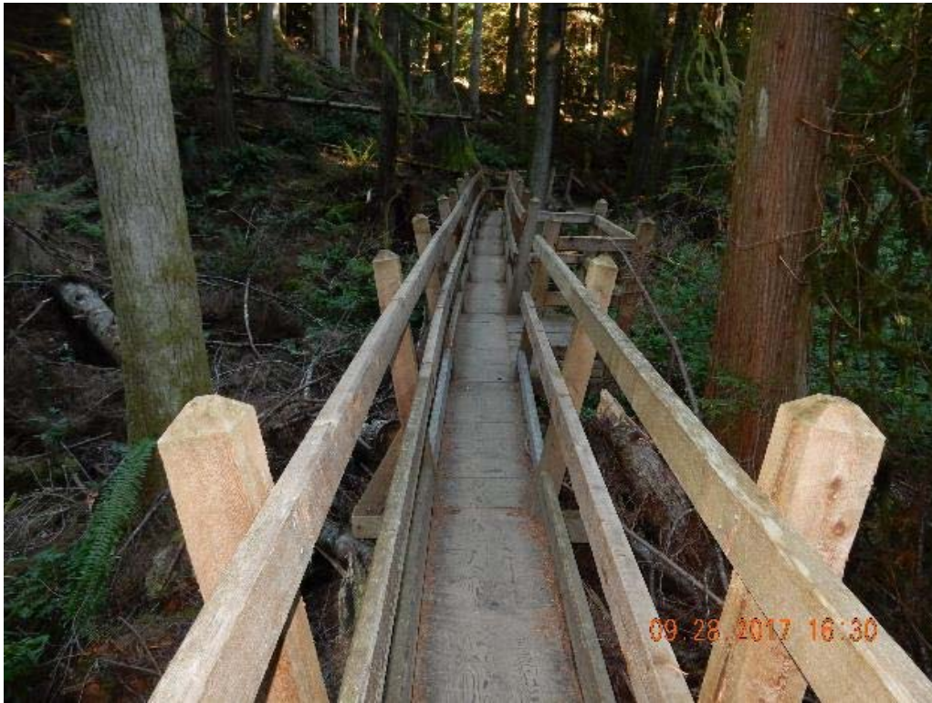
P11 – Overall decking (board walk) (DSCN9720.jpg)
