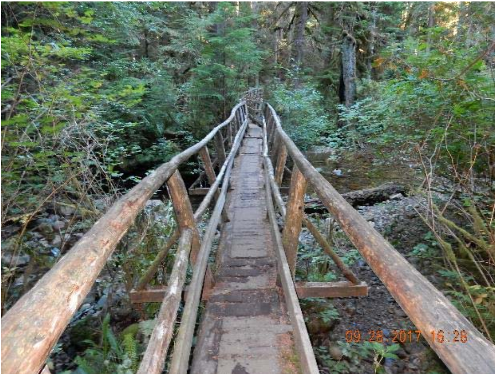
P02 – Overall decking (main span) (DSCN9709.jpg)
