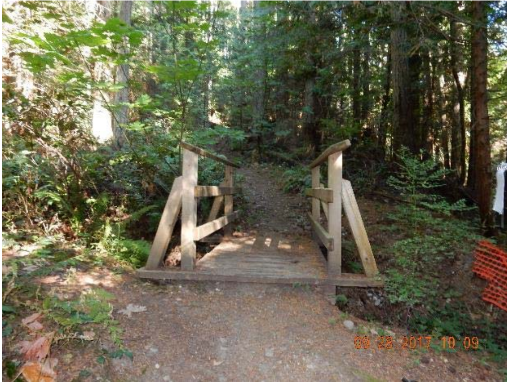
P01 – South approach (DSCN9460.jpg)
