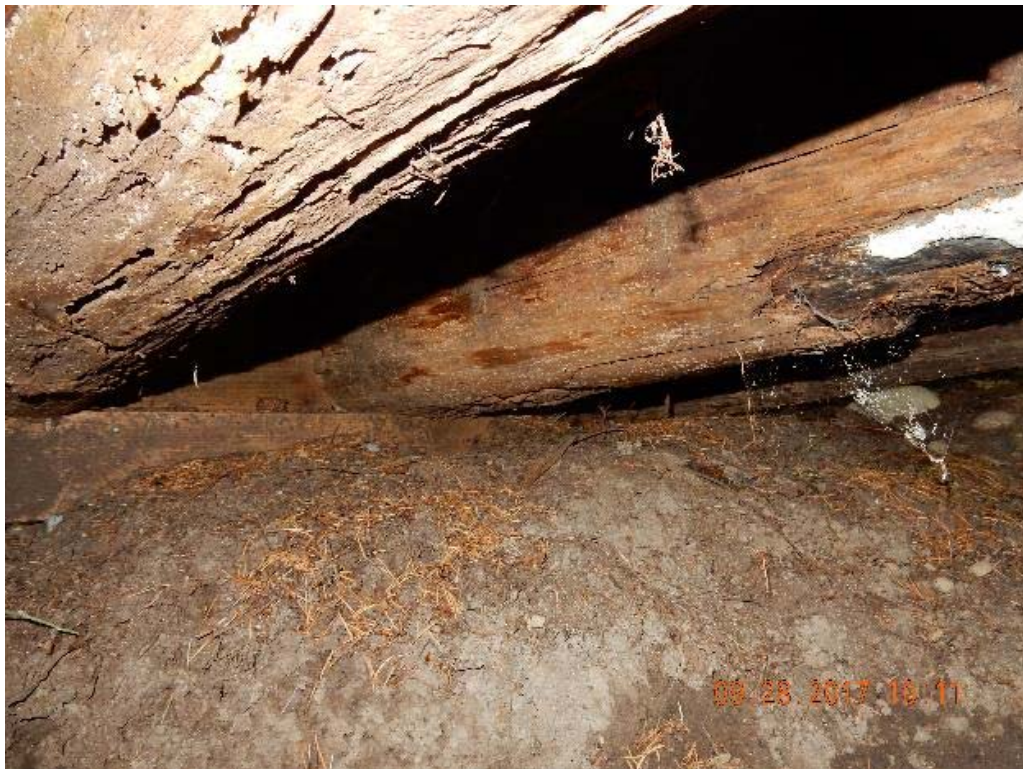
P10 – South abutment (DSCN9469.jpg)
