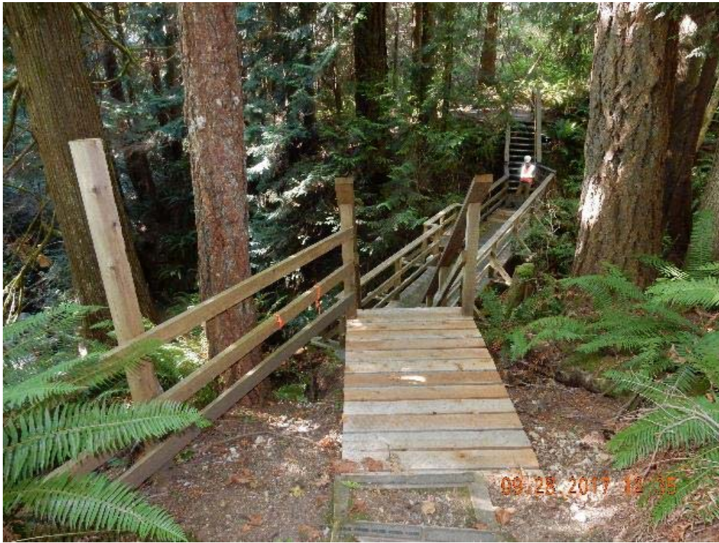
P09 – East approach (DSCN9548.jpg)
