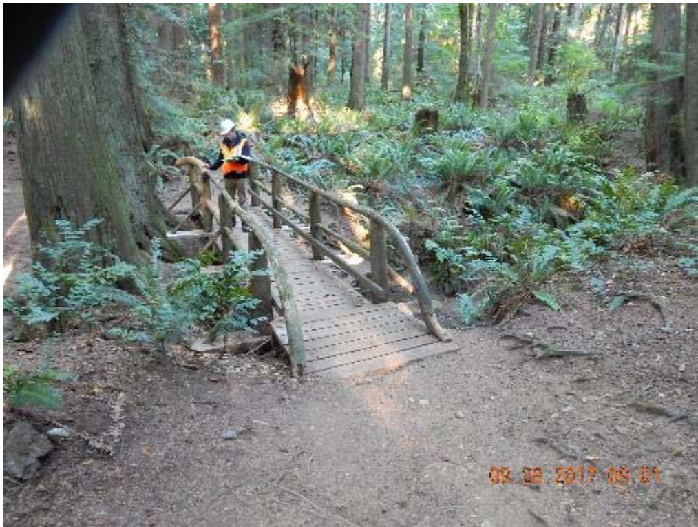
P06 – East approach (DSCN9430.jpg)
