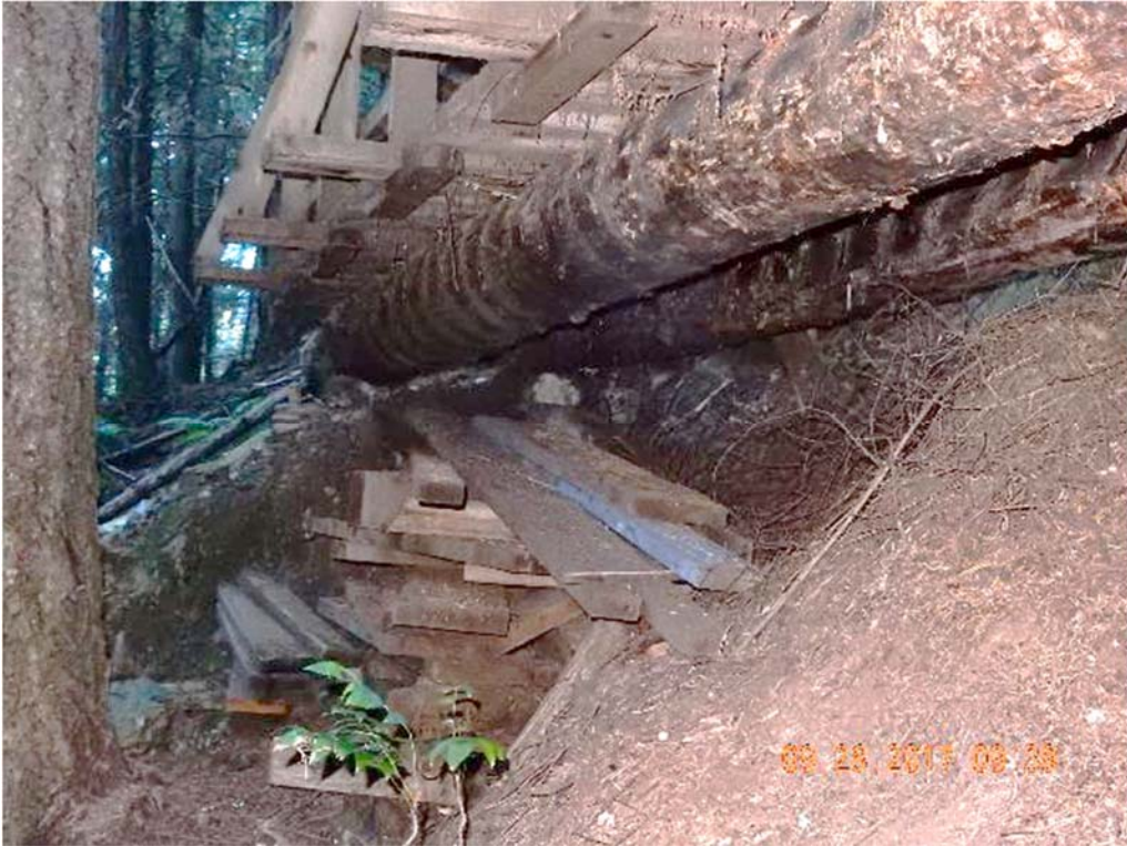
P07 – North abutment (DSCN9451.jpg)
