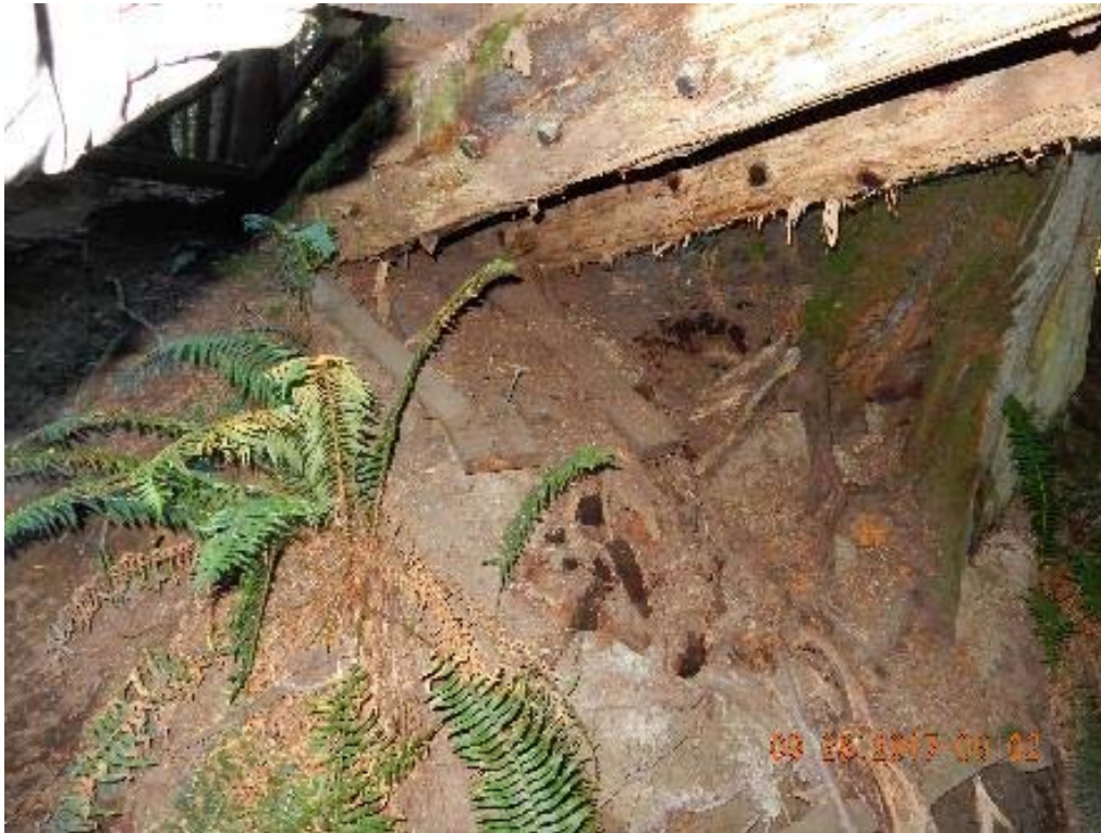
P09 – East abutment (DSCN9434.jpg)
