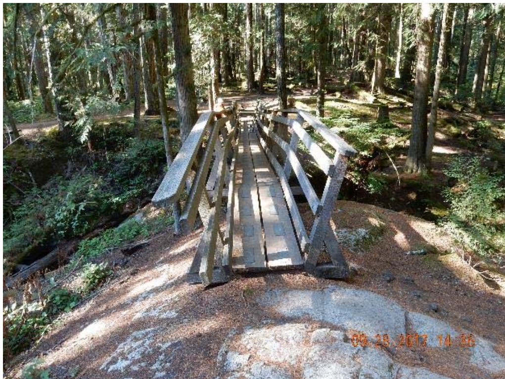
P04 – East approach (DSCN9608.jpg)
