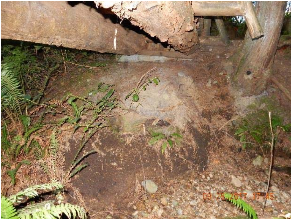
P07 – North embankment (DSCN9823.jpg)
