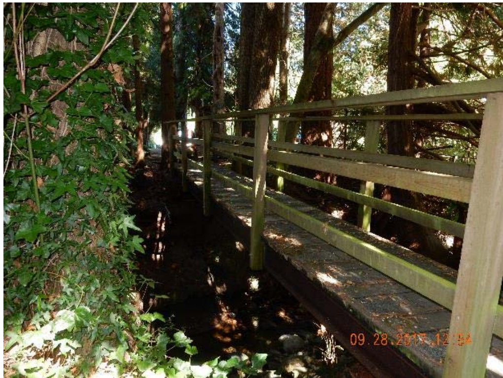
P08 – West side of the bridge (DSCN9569.jpg)
