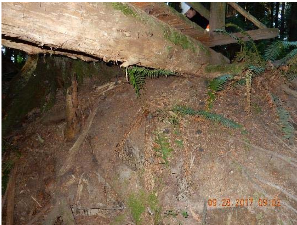
P08 – West abutment (DSCN9433.jpg)
