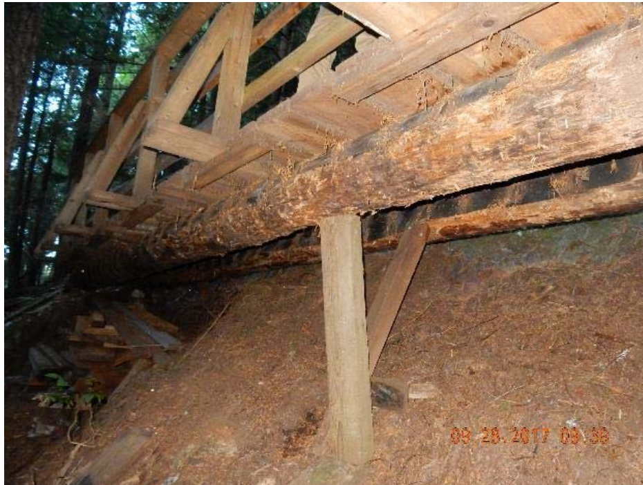
P06 – Pier, mid-span supported by two 8" x 4" posts. (DSCN9450.jpg)
