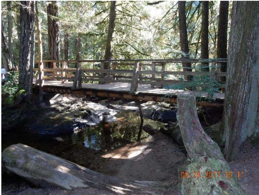
P09 – North side of the bridge (DSCN9663.jpg)
