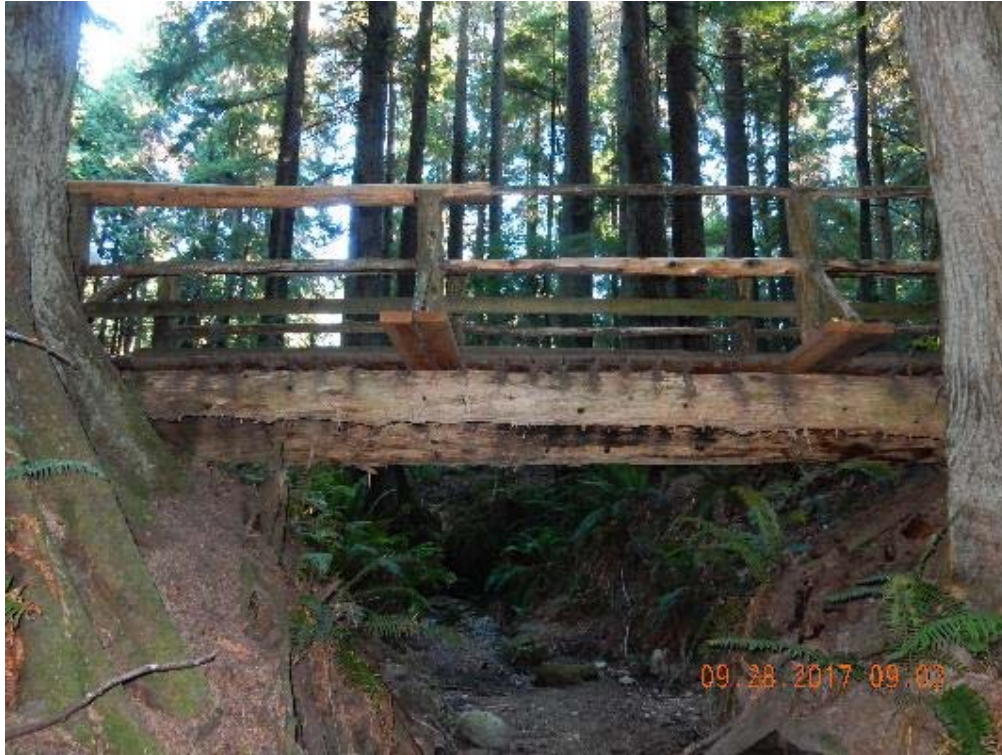
P11 – South side of the bridge (DSCN9436.jpg)
