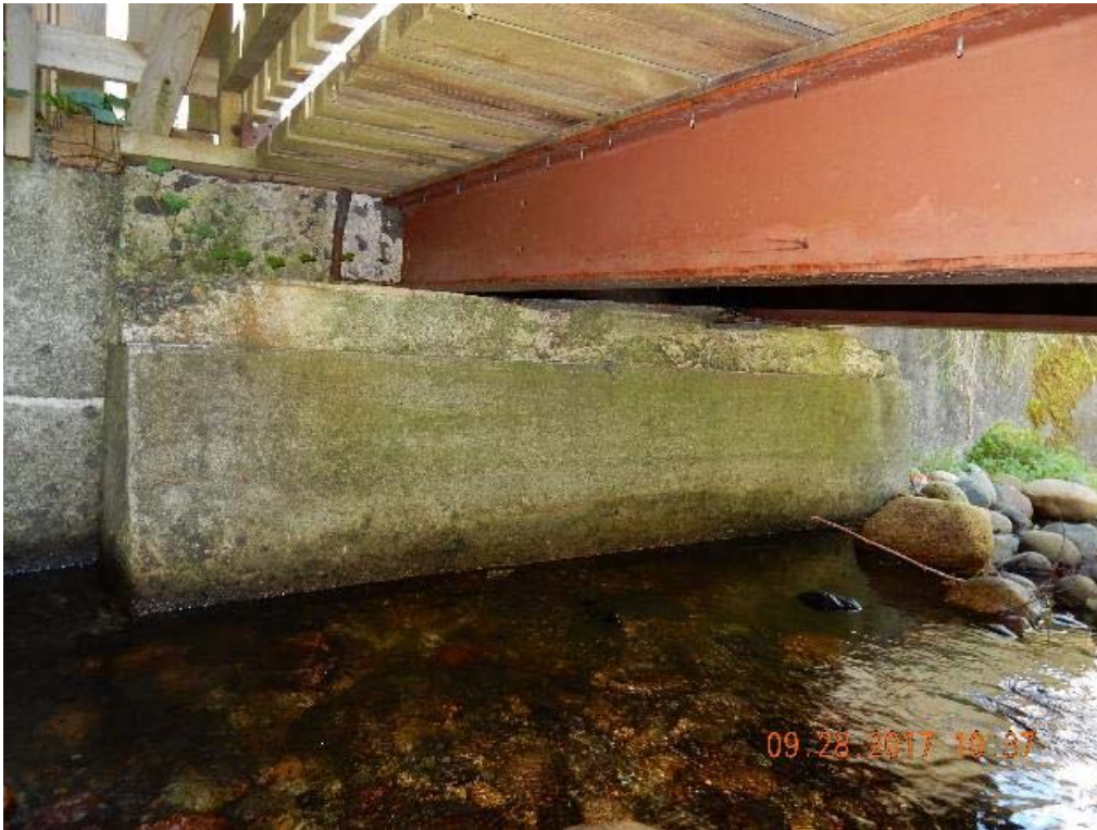
P11 – South abutment (DSCN9484.jpg)
