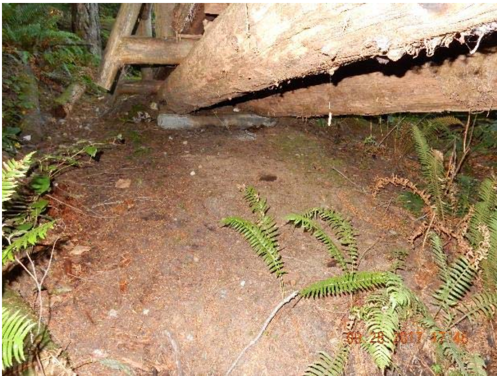
P08 – South embankment (DSCN9824.jpg)
