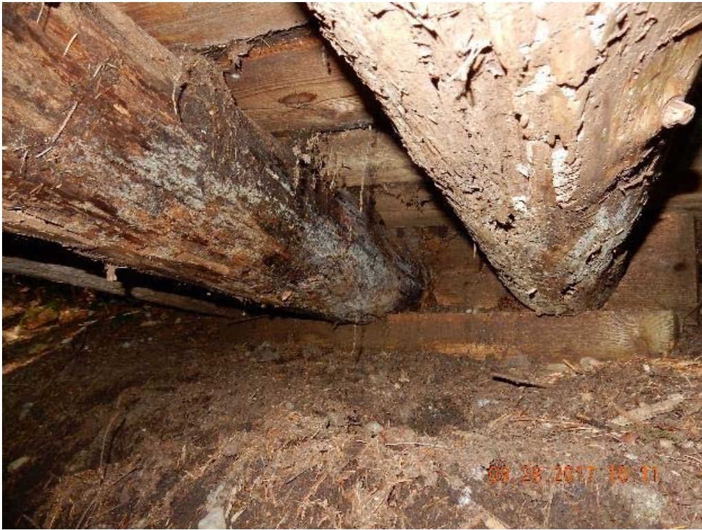
P09 – North abutment (DSCN9468.jpg)
