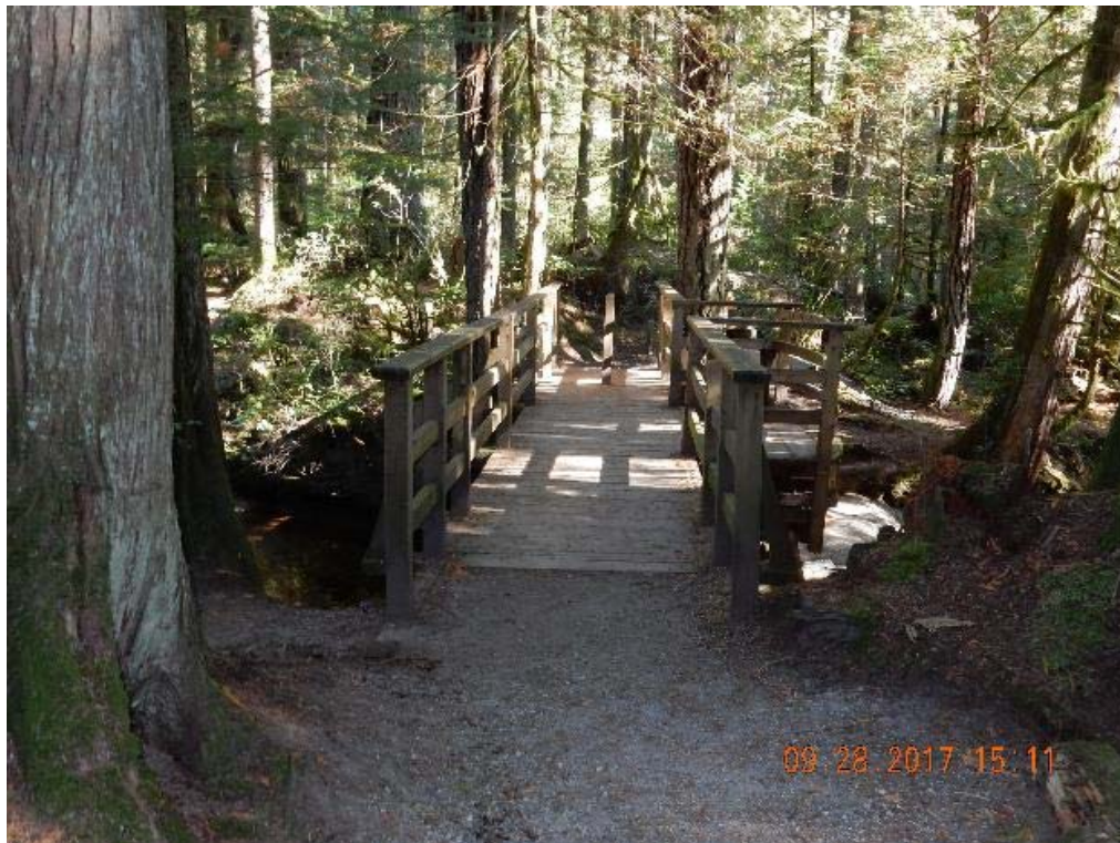
P08 – West approach (DSCN9662.jpg)
