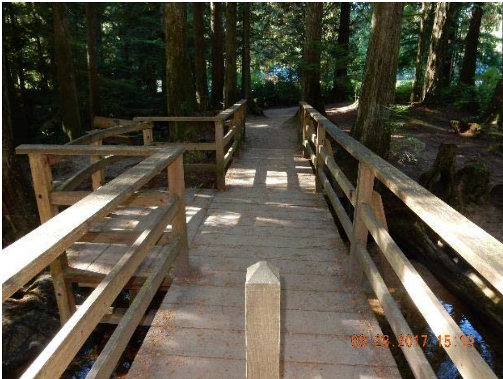
P02 – Overall decking (DSCN9656.jpg)
