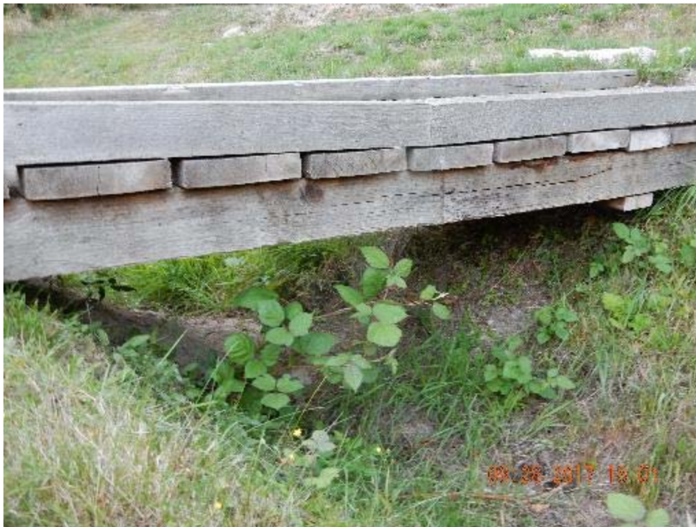
P04 – Side view of the bridge (west bridge) (DSCN9829.jpg)
