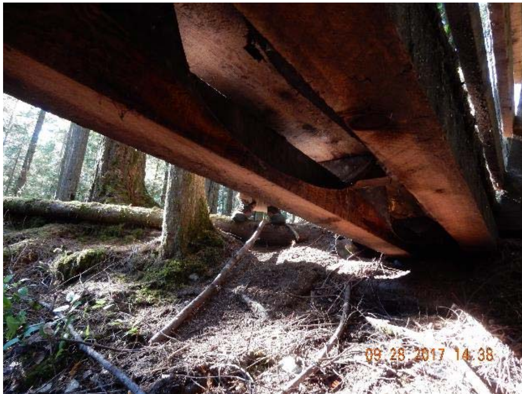
P10 – Under side of the bridge (west span) (DSCN9615.jpg)
