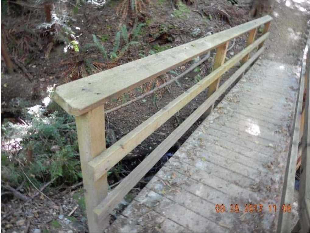
P03 – East railing (DSCN9491.jpg)
