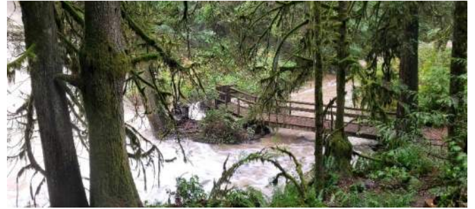
Lower Waterfall Bridge
