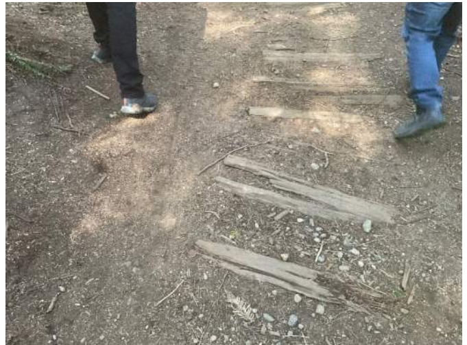
Existing timber planks to be removed
