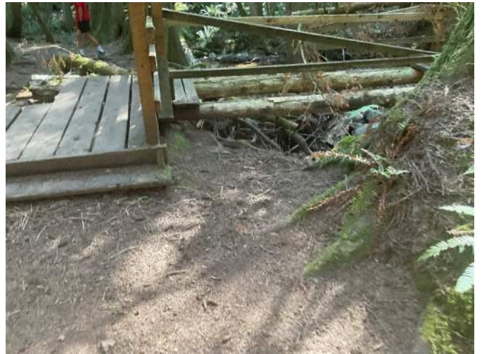
Zig Zag Bridge - North abutment
