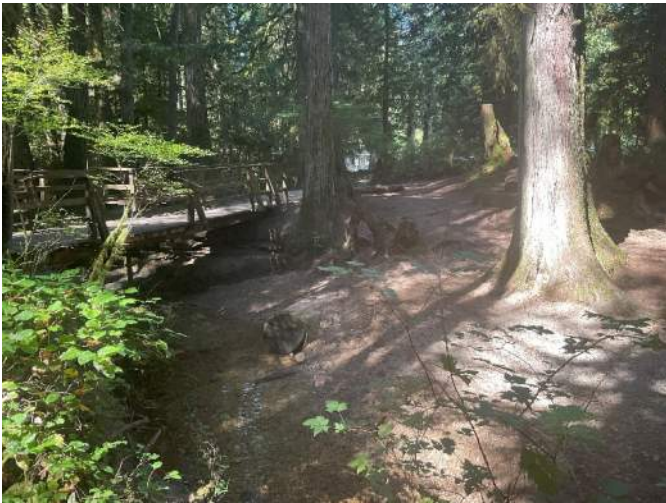
Upper Waterfall Bridge – Upstream view
