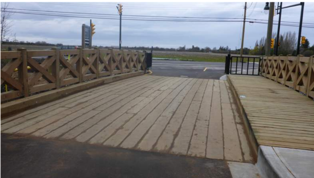
And more selected photos of steel bridges with wood elements
