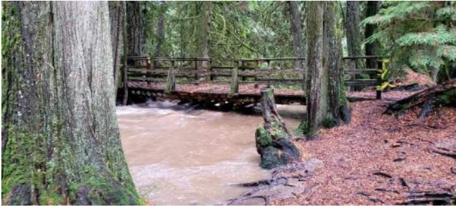
Upper Waterfall Bridge
