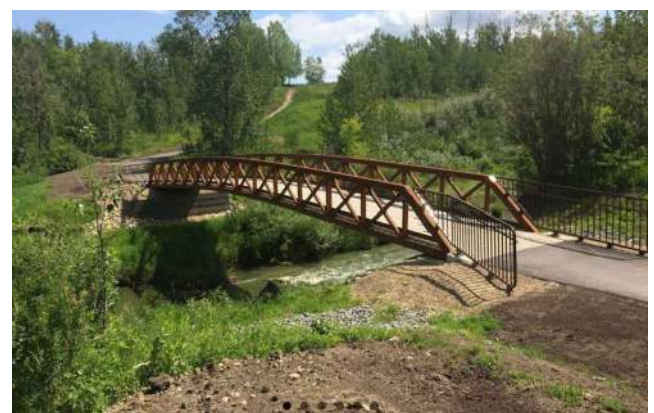
STEEL TRUSS BRIDGE EXAMPLE
