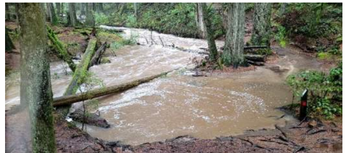
Trail Flooding by Gorge Bridge
