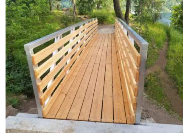
ALUMINUM TRUSS BRIDGE EXAMPLE
