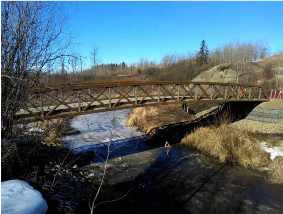
Steel Truss – Grande Prairie, AB
