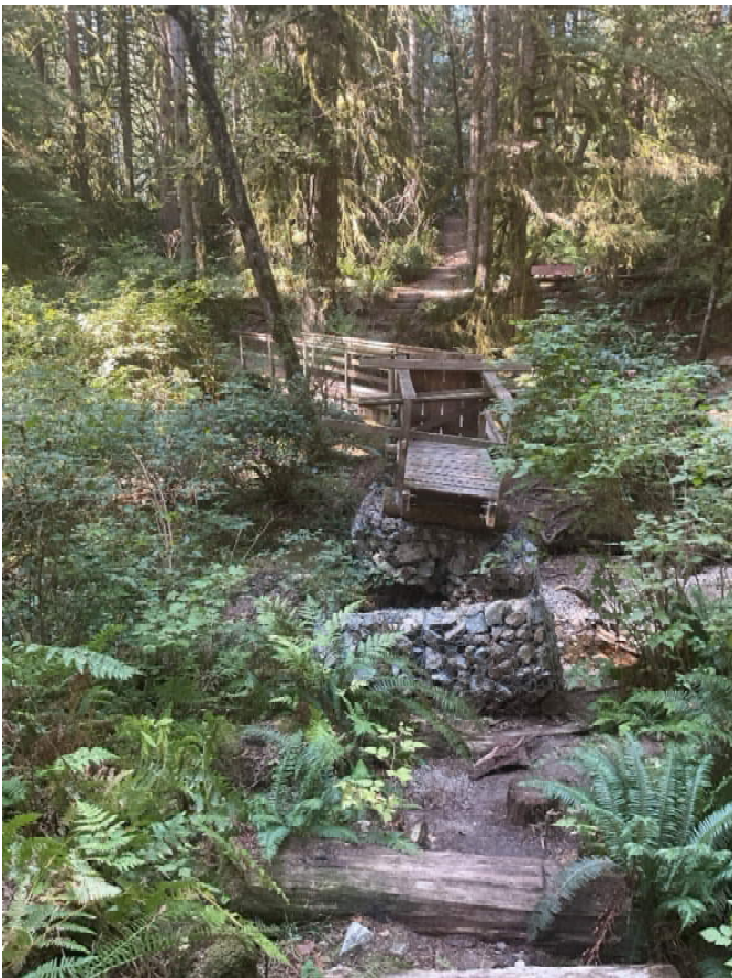
Lower Waterfall Bridge – View from north approach
