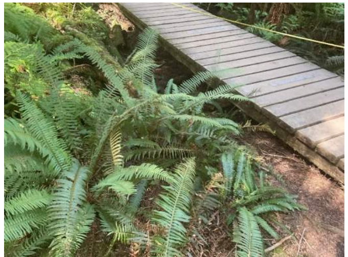
Existing boardwalk to be replaced
