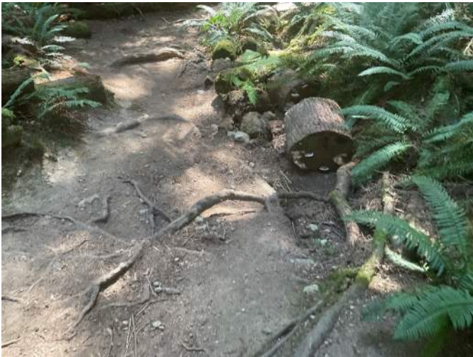
Erosion of existing trail section
