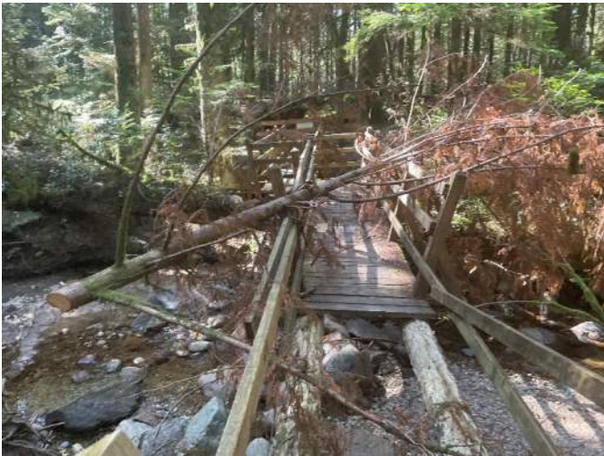
Zig Zag Bridge – view from south approach
