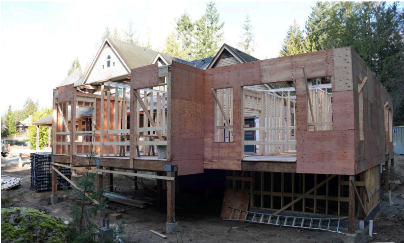
Framing completed for four new hospice suites and nursing station.
