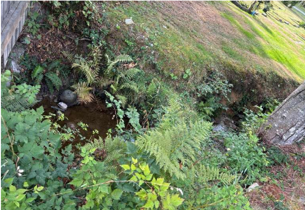
Photo 15: 914 mm (36 in) corrugated steel culvert at upstream end of Cornwallis Creek.
