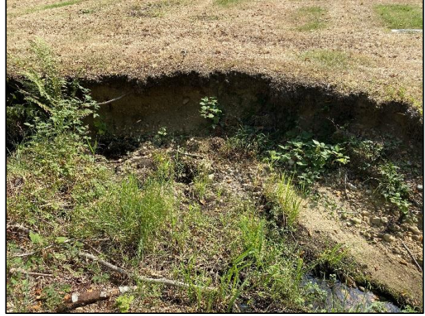
Photo 16 Steep eroding banks of Cornwallis Creek in Area 1.
