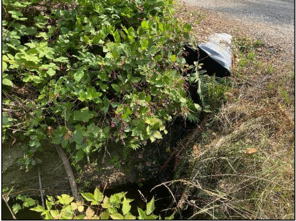
Photo 22 Perched culvert under the Cemetery's driveway along Lower Road in Area 1.
