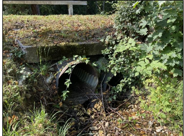
Photo 18 Upstream view of culverts running under the bridge in Area 1.
