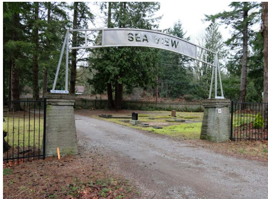
Figure 26: Main cemetery entrance. Need to modify or remove arch.
