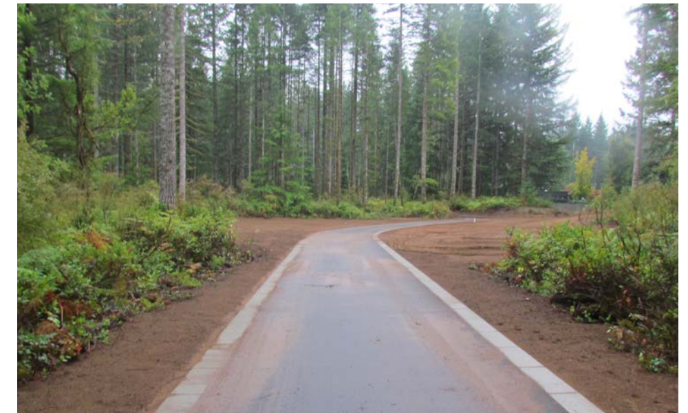
Figure 39: Example of an asphalt driveway with flush concrete curbs. Elk Falls Cemetery, BC. Source: LEES+Associates
