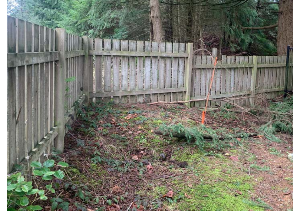
Figure 25: Fencing on the north side of the cemetery, opportunity to enhance the perimeter.
