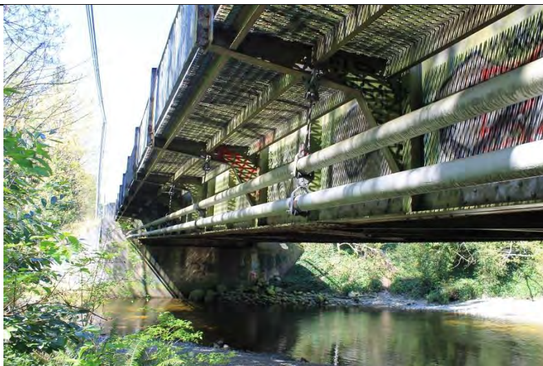
General view of the southern side of Chapman Creek Bridge from the eastern embankment, showing 2No. gas mains supported below the southern bridge sidewalk.
