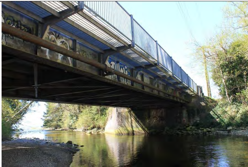
General view of the northern side of Chapman Creek Bridge from the eastern embankment, showing the water main supported by the outer girder below the bridge sidewalk.
