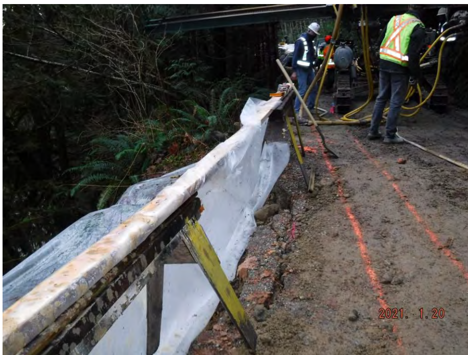
Figure 2: Watermain and Temporary Support Alignment Determination.
