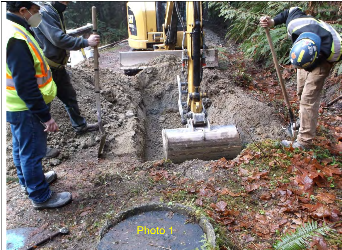
Jan 20, 2021; 10:43 – Chapman Creek Landslide - SCRD Waterline Stabilization View west - expose and locate 2 waterlines
