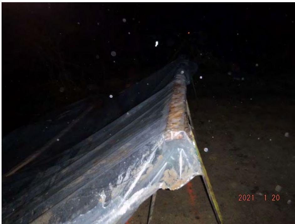
Figure 6: Covering the Landslide Area with Plastic Sheeting
