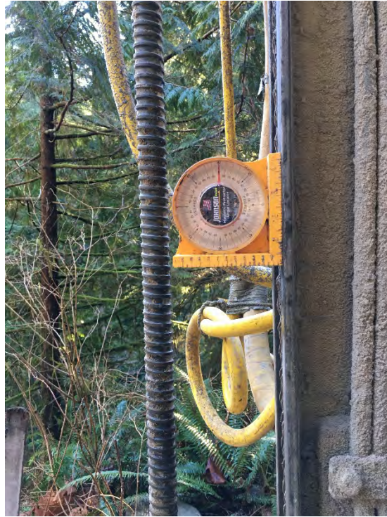
Photograph 3: Field Protractor Assessing the Verticality of the Rig Prior to Drilling
