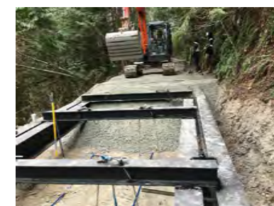
Photograph 6: Placing and Spreading the Backfill material (Looking West)
