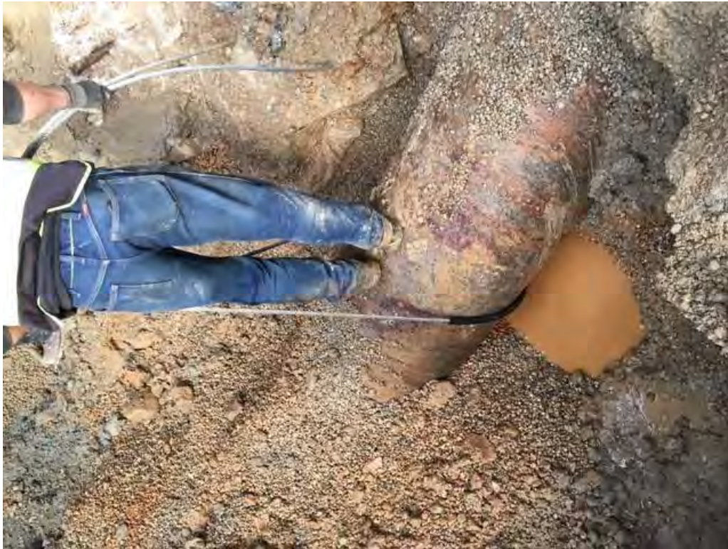
Figure 1: Hand Digging and Placing the Steel Strap with Rubber Sleeve.
