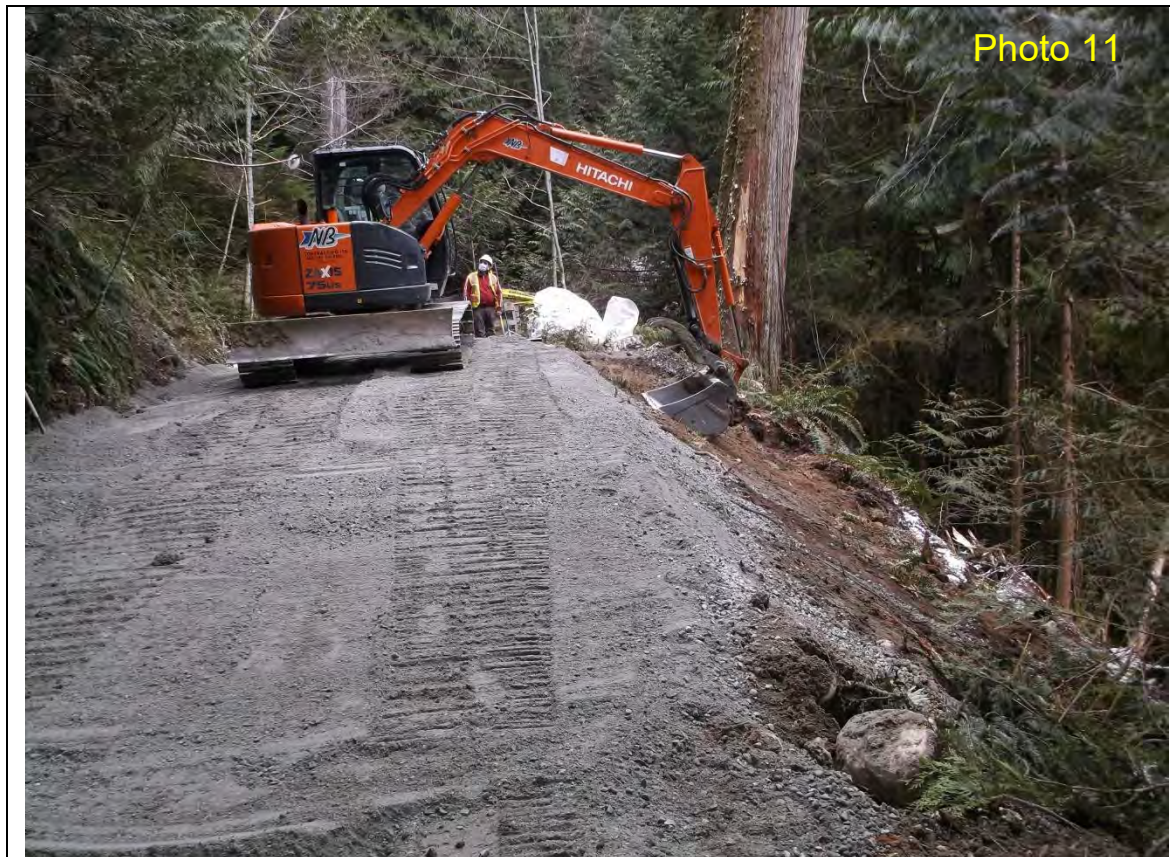
Feb 12, 2021; 14:24 – Chapman Creek Landslide - SCRD Waterline Stabilization View east - grade beam installed, shaping fill slope
