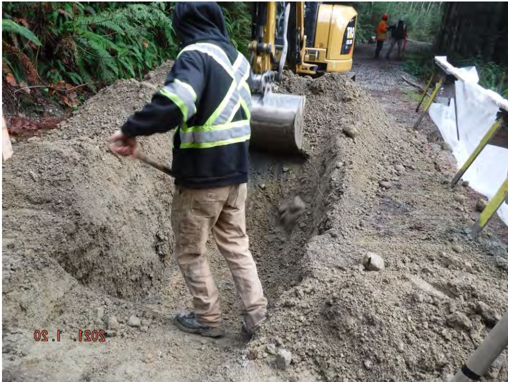
Figure 1: Utility Potholing.
