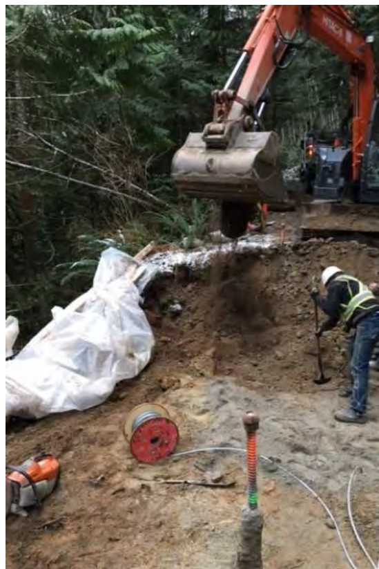
Figure 4: Sand Backfilling after the Installation of Steel Straps
