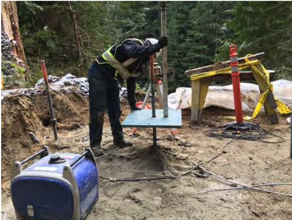
Figure 3: Levelling each Base Plate Prior to Welding.
