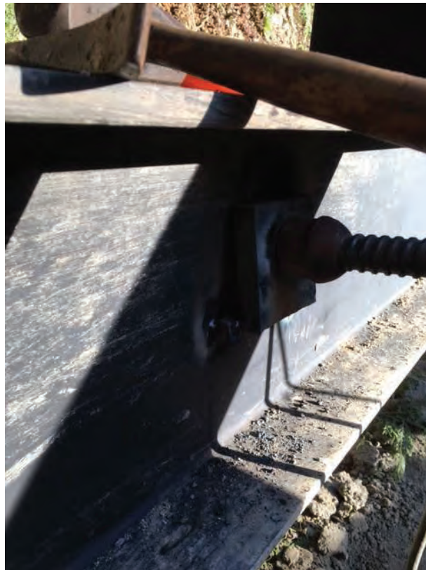
Figure 2: Custom-Made Seating Where the Anchors Rest on the Web of the Grade Beams.
