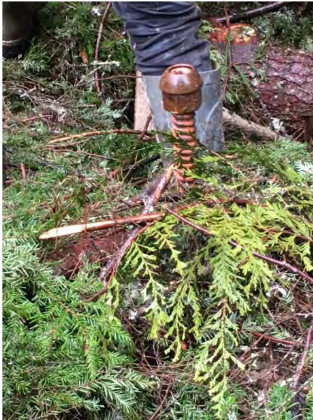
Figure 3: Placing a Cap Over Anchors and Micropiles
