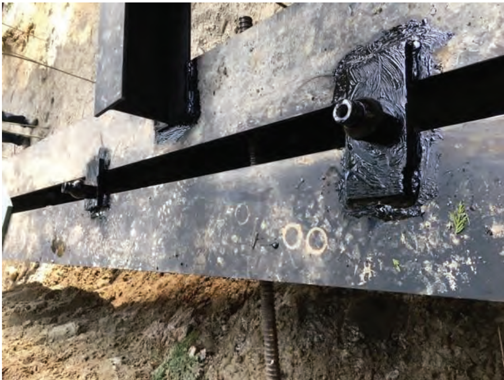
Figure 4: Application of Protective Paint Patch over the Grade Beam
