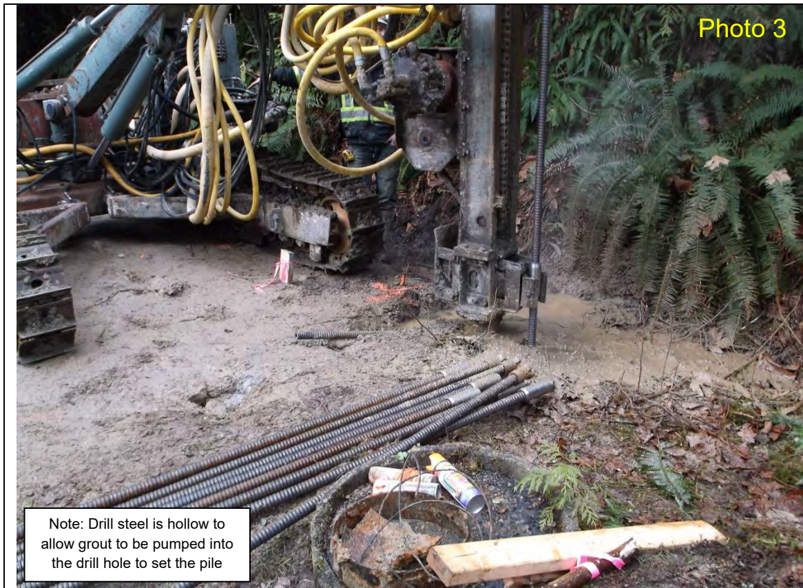
Jan 21, 2021; 09:52 – Chapman Creek Landslide - SCRD Waterline Stabilization View to west - drill vertical pile
