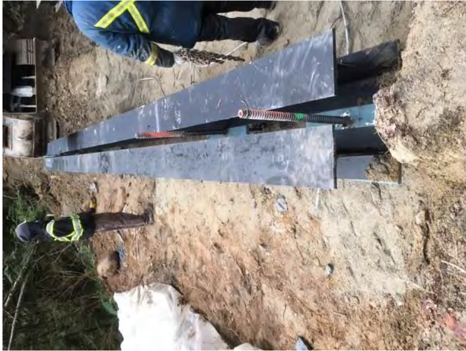
Figure 5: Installation of Grade Beams over the Base Plates
