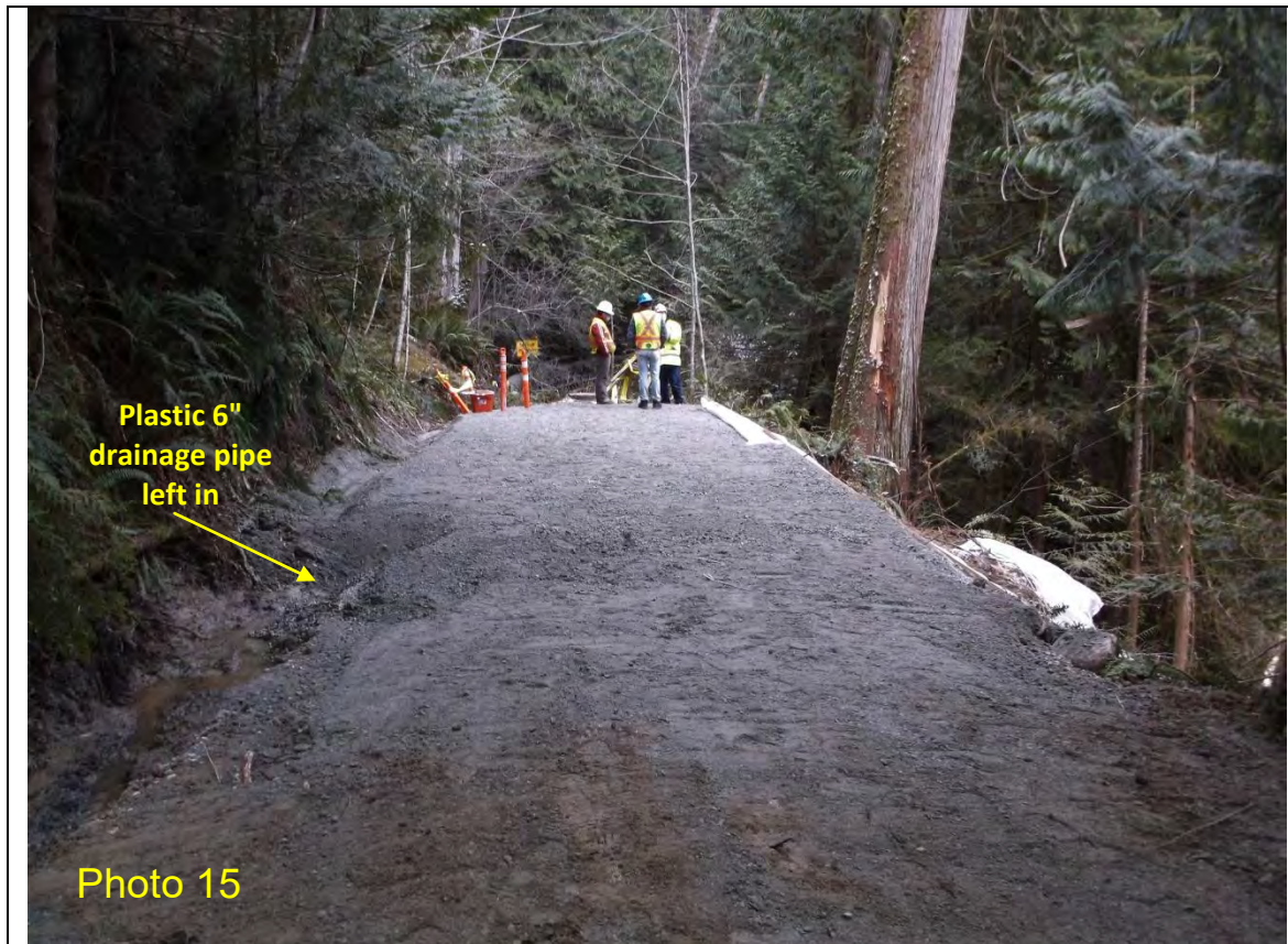
Feb 12, 2021; 15:21 – Chapman Creek Landslide - SCRD Waterline Stabilization View east - grade beam installed, poly sheet fill slope erosion protection, ditch line installed
