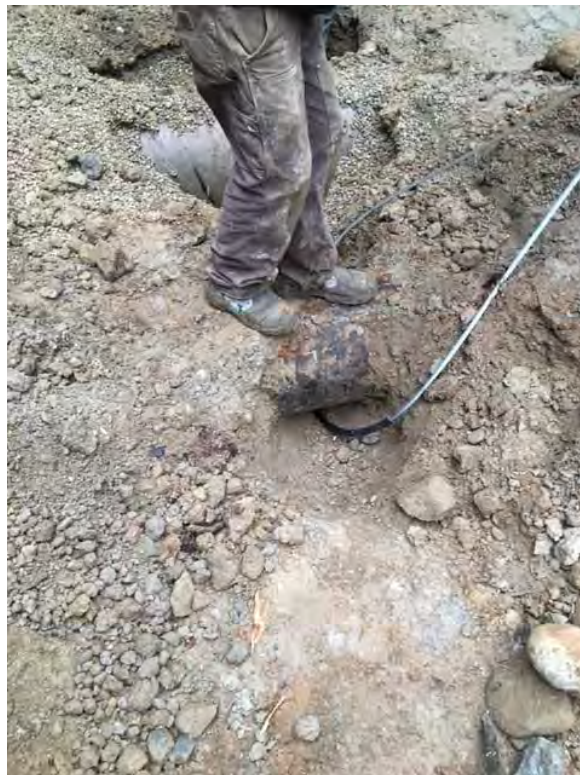
Photograph 2: Installation of Steel Galvanized Cable around Pipes.
