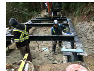
Photograph 5: Installation of Grade and Crossover beams and steel straps (Looking West)
