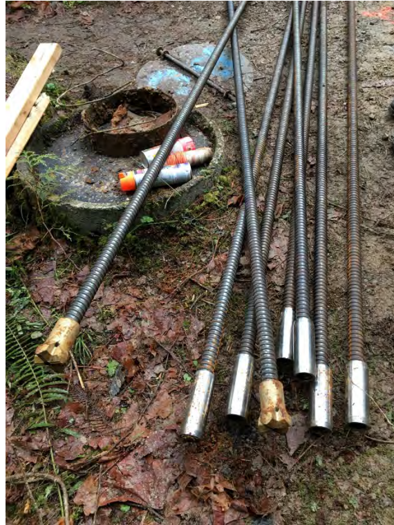
Photograph 1: Drill Bits and Couplings Attached to Anchors.
