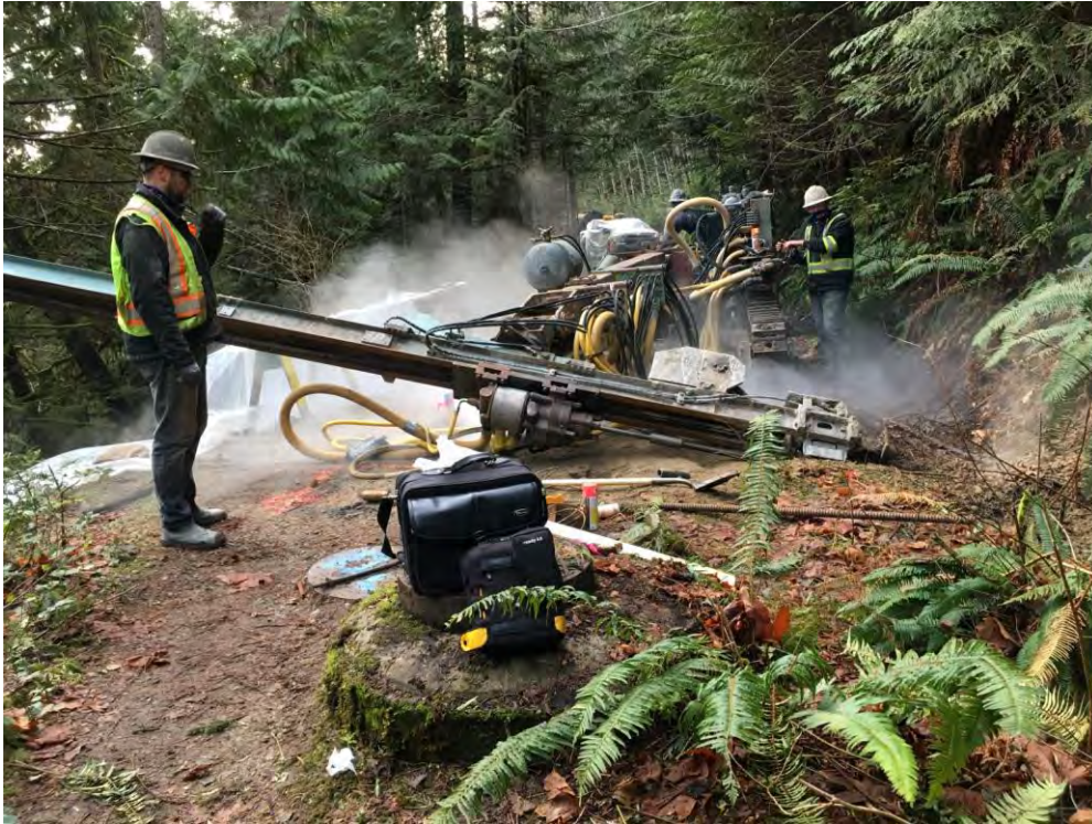
Figure 3: Drilling and Grouting of Anchor (East).
