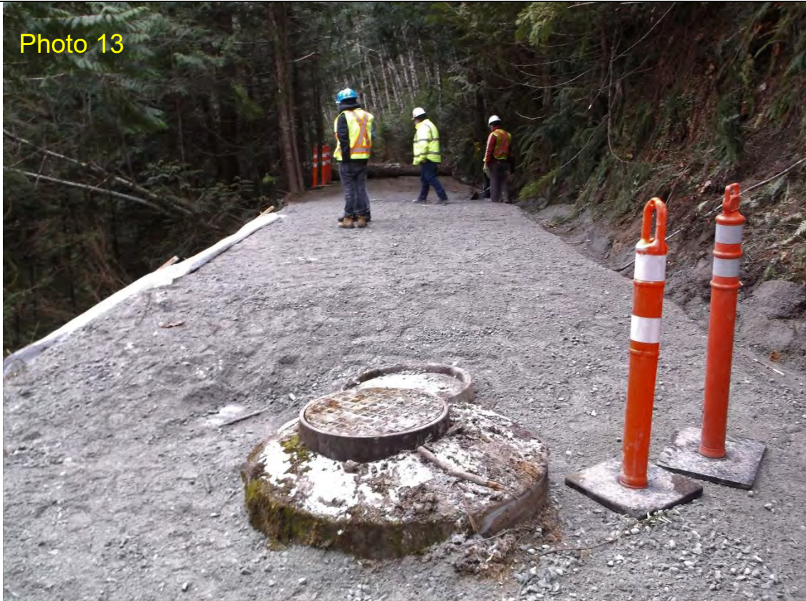
Feb 12, 2021; 15:08 – Chapman Creek Landslide - SCRD Waterline Stabilization View west - grade beam installed, ditch line installed
