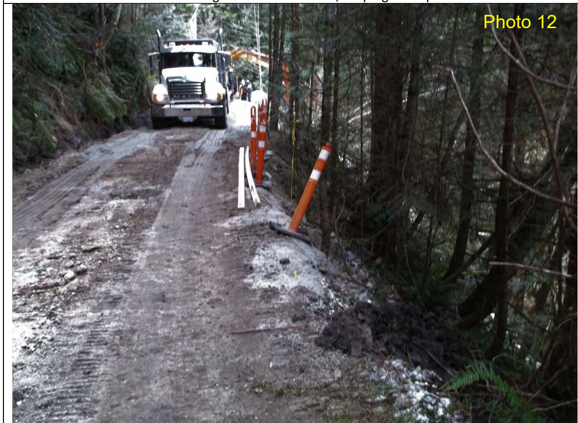
Feb 12, 2021; 14:25 – Chapman Creek Landslide - SCRD Waterline Stabilization View east - grade beam installed, over steepened placed fill soils before removal
