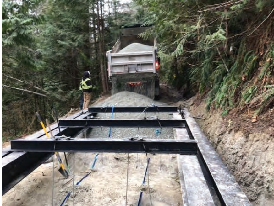
Figure 5: Taping Along the Two Main Water Supply Pipes and Dumping the Road Base.
