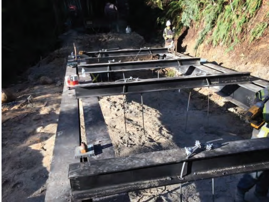
Figure 1: Installation of the Last Cross-Over Beam and Steel Straps.
