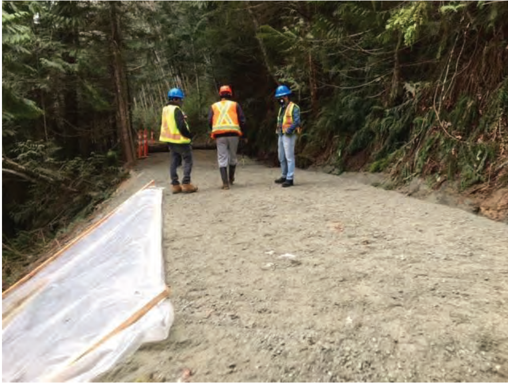
Figure 7: The Final Prepared Surface of the Backfilled Area and the Installation of the Poly Sheet over Downslope Area.
