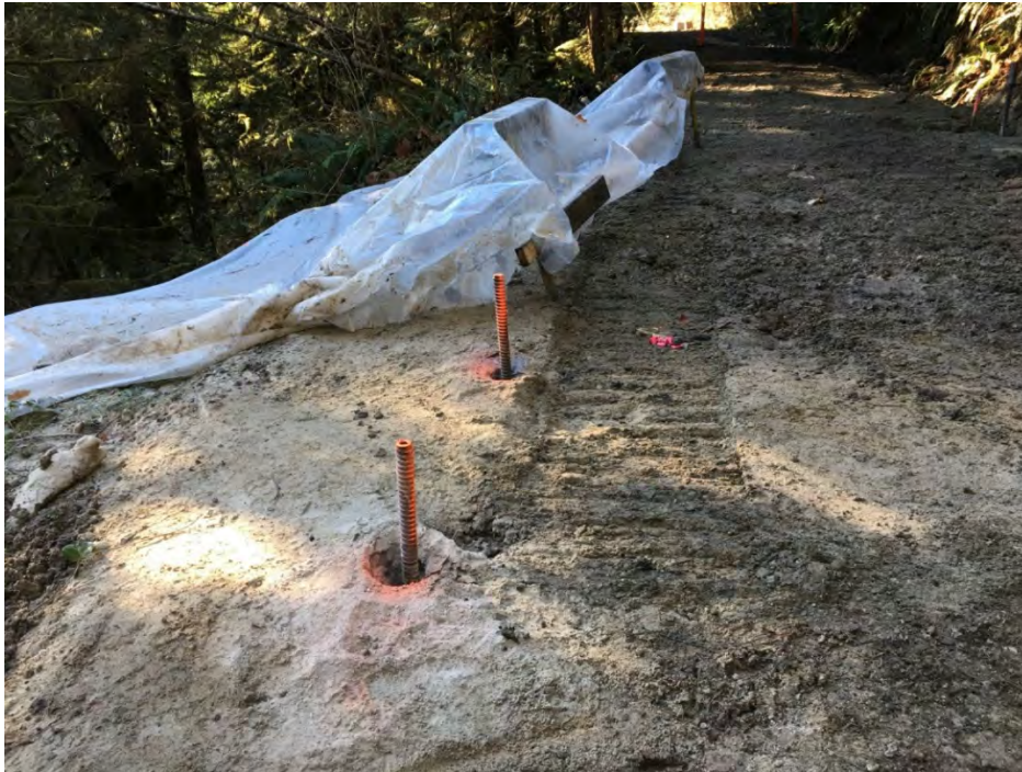
Figure 3: Covering of the Landslide Area with Plastic Sheeting for Weather Protection.
