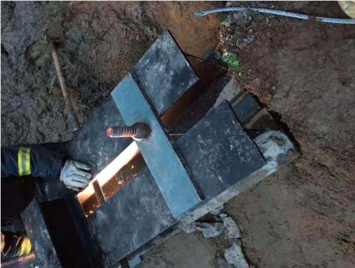
Figure 7: Installation of Additional Base Plates at the Top of the Grade Beams to Provide Proper Seating for the Nuts Connected to the Micropiles and Completing the Welding
