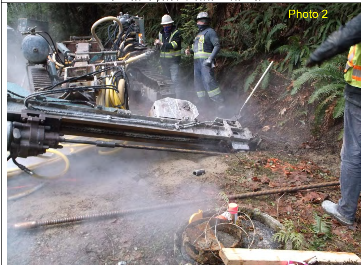
Jan 20, 2021; 15:25 – Chapman Creek Landslide - SCRD Waterline Stabilization View west - drill horizontal anchor pile
