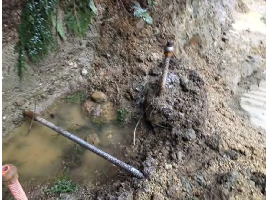
Figure 3: Temporary Blockade of the Ditch Around the Excavated Area to Prevent Surface Water Flooding.
