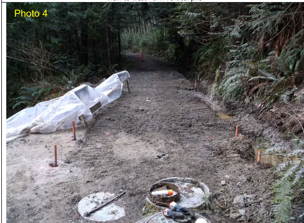
Jan 23, 2021; 11:11 – Chapman Creek Landslide - SCRD Waterline Stabilization View to west - piles installed and grouted
