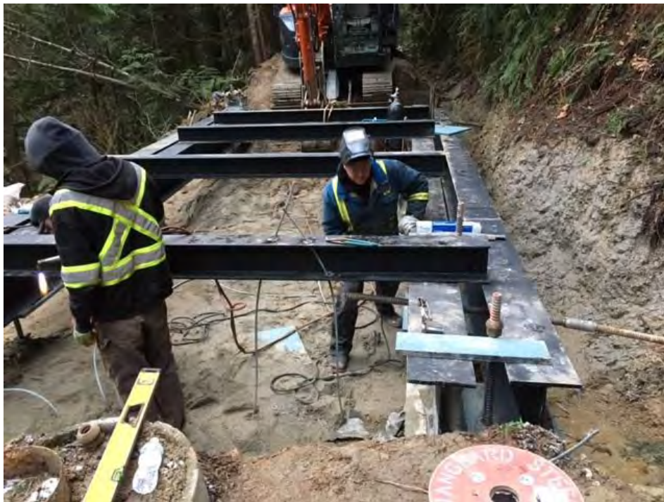
Figure 6: Installation of Cross-Over Beams after Welding the Grade Beams to the Base Plates and Making Holes at the Opposite Sides of the Flange for the Connection of Steel Straps to the Cross-Over Beams
