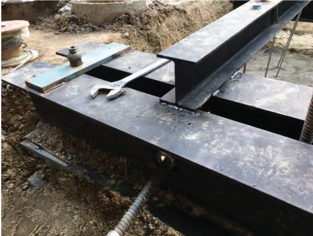
Figure 3: Welded Base Plate and Cross Over Beams to the Grade Beams.
