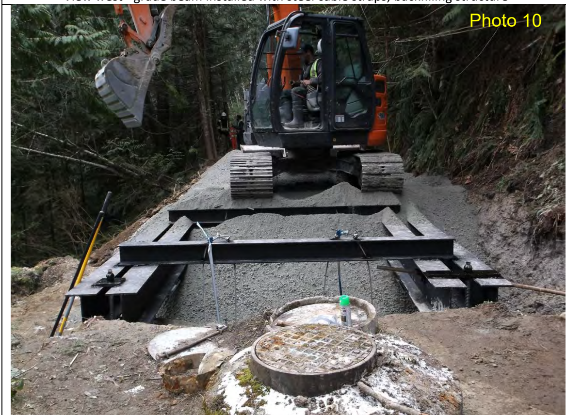
Feb 12, 2021; 13:44 – Chapman Creek Landslide - SCRD Waterline Stabilization View west - grade beam installed with steel cable straps; backfilling structure
