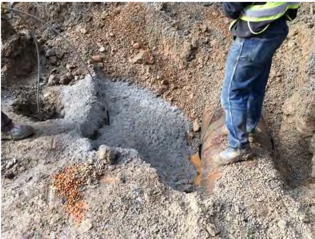
Figure 2: Backfilling with Clean Sand to Secure the Steel Straps.
