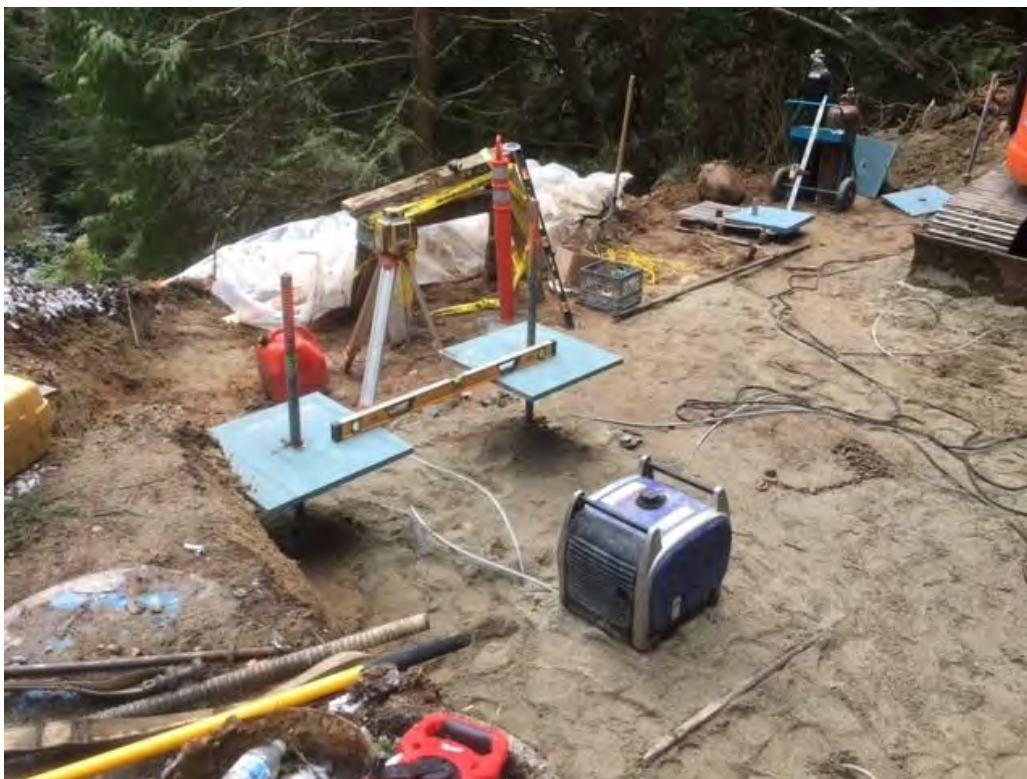
Figure 4: Levelling the Base Plates Prior to the Installation of Grade Beams.
