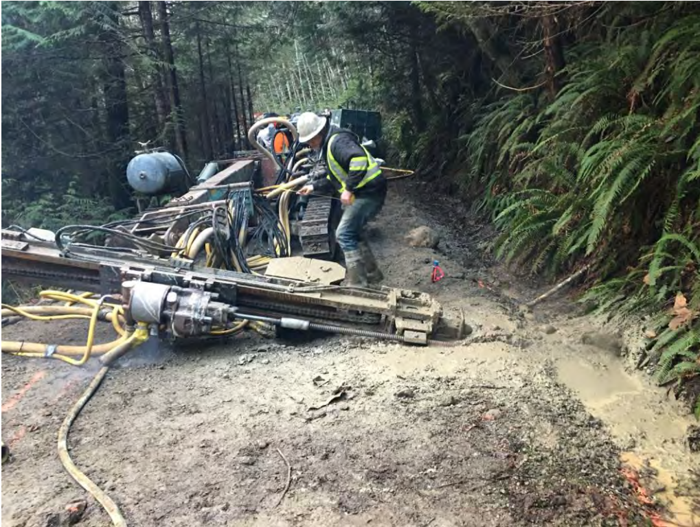
Figure 5: Drilling and Grouting of Anchor (West).
