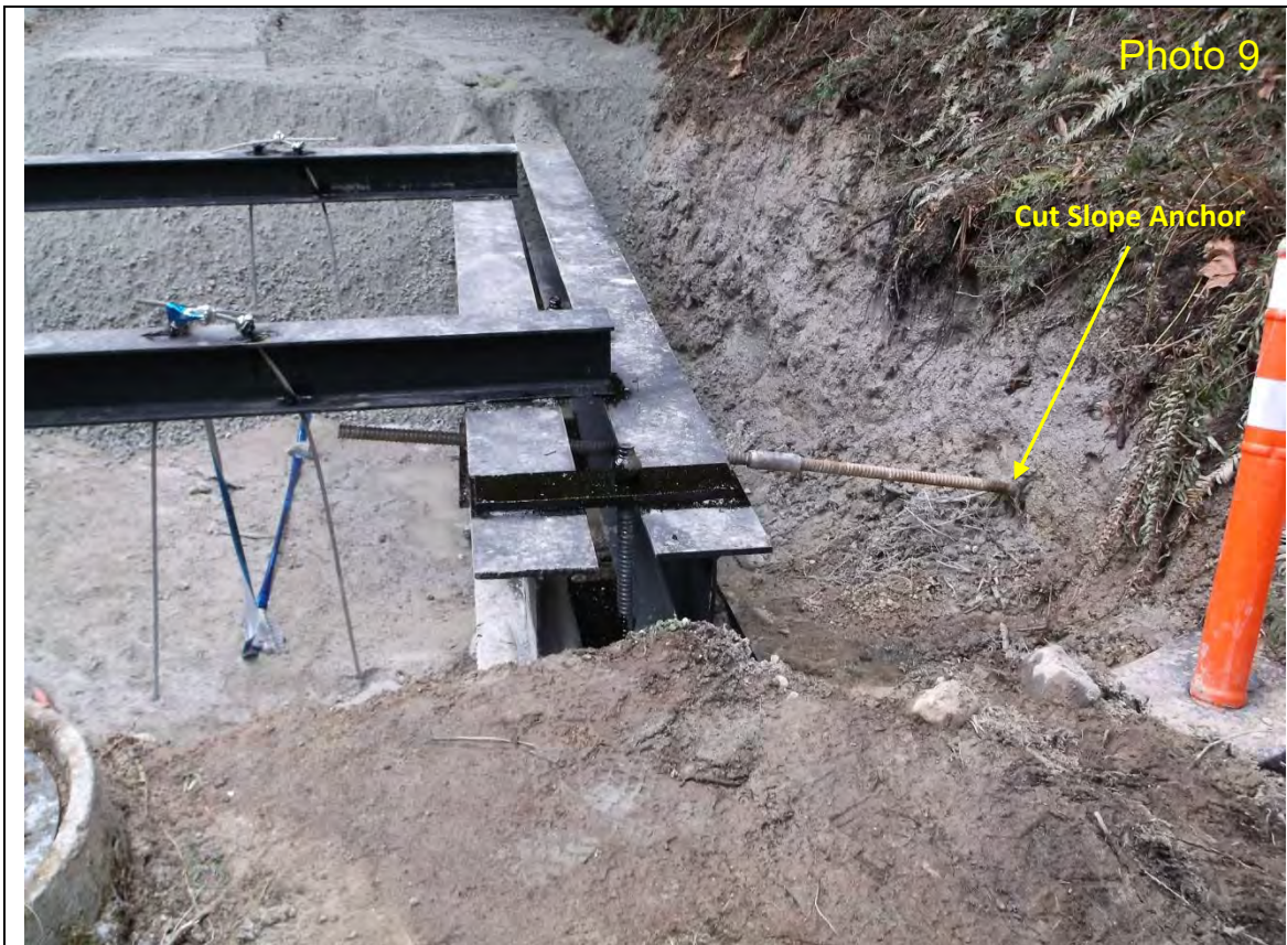
Feb 12, 2021; 13:24 – Chapman Creek Landslide - SCRD Waterline Stabilization View west - grade beam installed with steel cable straps; backfilling structure
