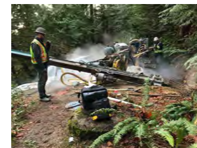
Photograph 4: Anchor Installation
