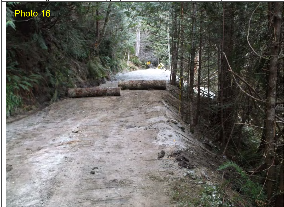
Feb 12, 2021; 15:28 – Chapman Creek Landslide - SCRD Waterline Stabilization View east - grade beam installed, fill slope soil removal complete, road blocked
