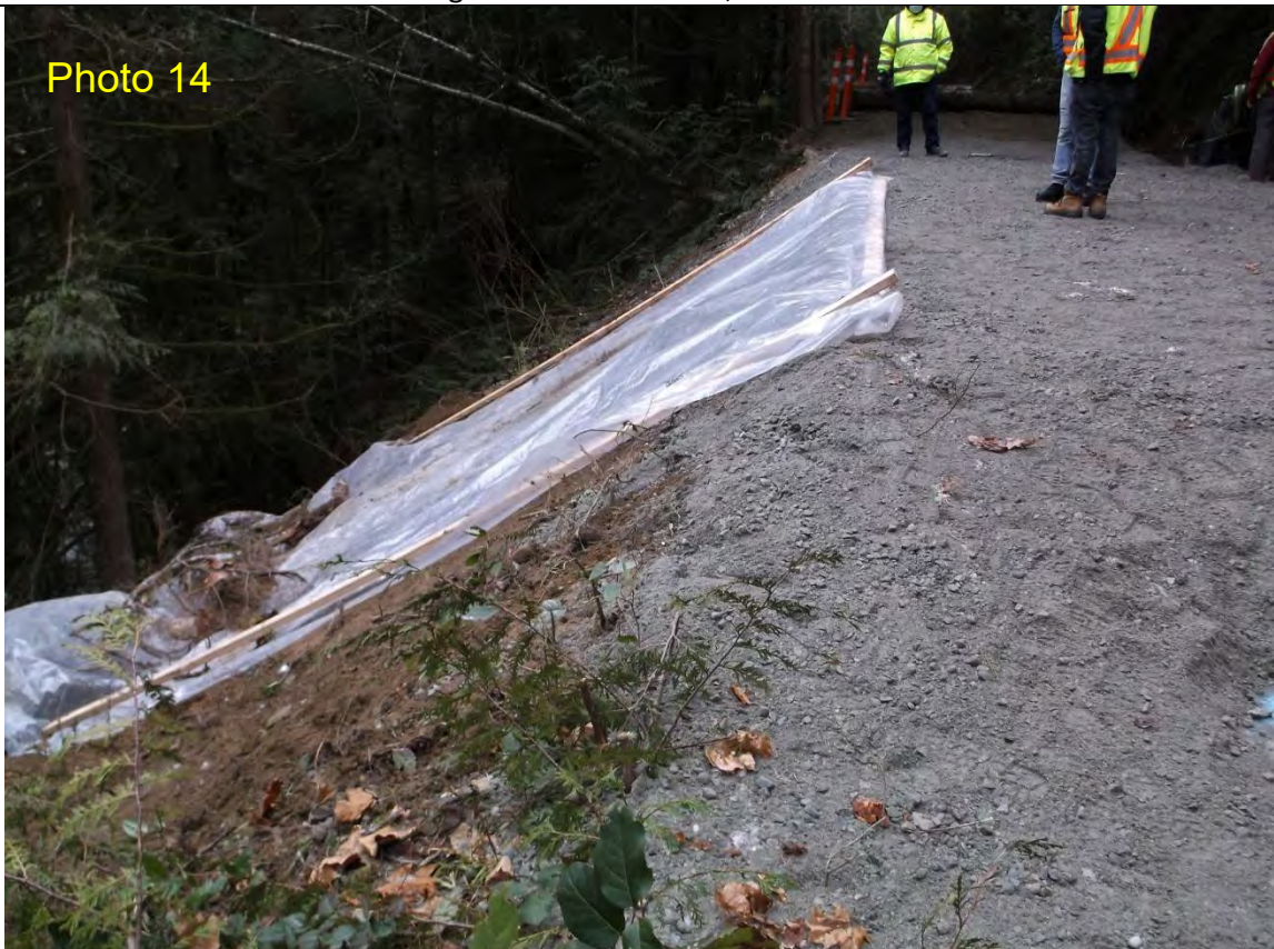
Feb 12, 2021; 15:08 – Chapman Creek Landslide - SCRD Waterline Stabilization View west - grade beam installed, poly sheet fill slope erosion protection
