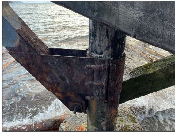
Photograph 4: Light post mounting bracket, note: significant corrosion
