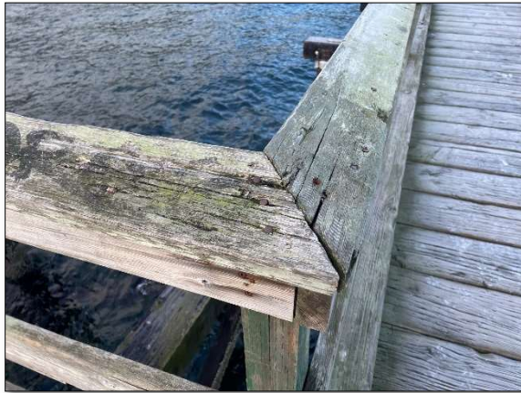
Photograph 9: Handrails, note: general condition is fair to poor
