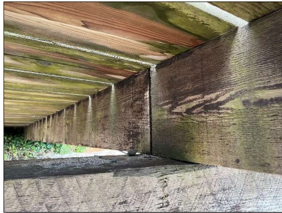
Photograph 14: Stringer butt joint, note: missing splice connection
