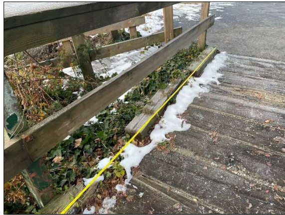
Photograph 8: Timber guard at 1.22m Gridline E, note: cross section loss and biological damage
