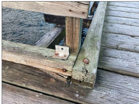
Photograph 12: Timber guard riser at 26E, note: damaged and decayed:
