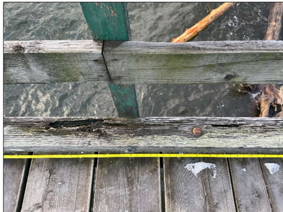
Photograph 11: Timber guard at 61m Gridline E, note: cracking through hardware, soft interior
