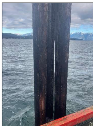
Photograph 23: Float flange splice location, note: failed connection resulting in "sagging" of the bull rail/flange arrangement
