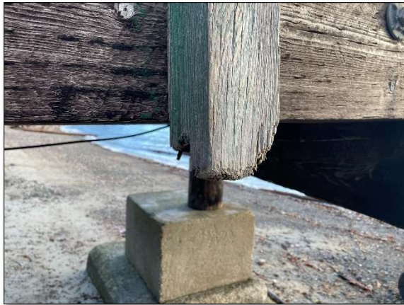
Photograph 7: Handrail post, note: cross section loss at cut end
