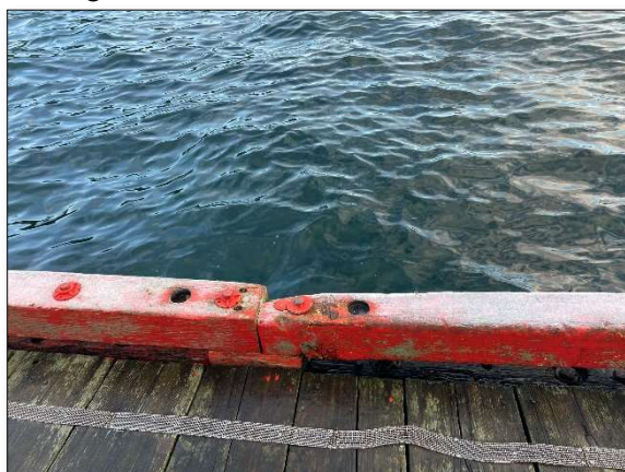
Photograph 23: Float flange splice location, note: failed connection resulting in "sagging" of the bull rail/flange arrangement
