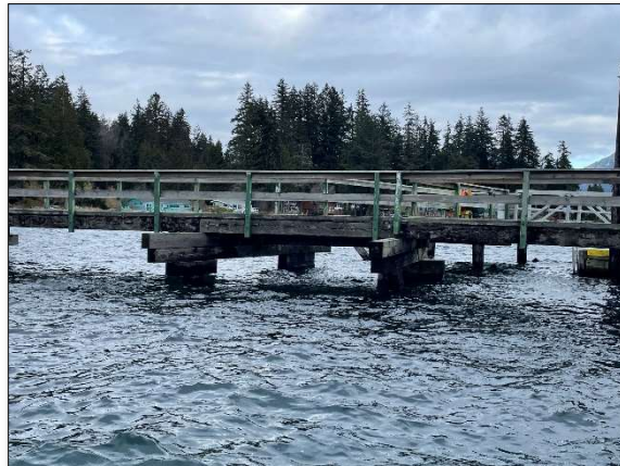
Photograph 20: Bearing piles 15E and 16E, note: corbel repairs with pile submerged at HHWLT
