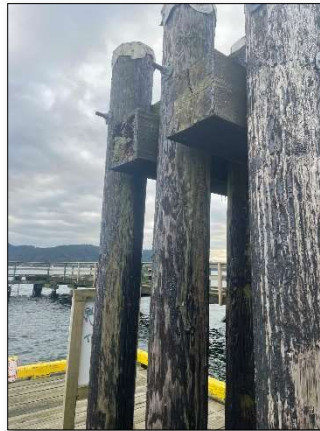
Photograph 26: Compact mooring dolphin, note: blocking significantly decayed
