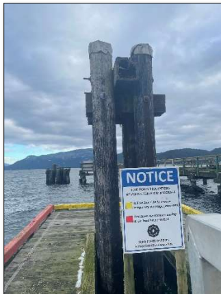
Photograph 27: Compact mooring dolphin, note: significant cross section loss to blocking
