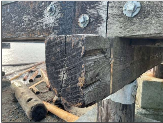
Photograph 15: Pile cap at Bent 1, note: strap repair and cracking
