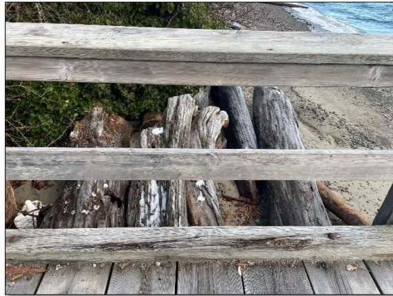
Photograph 10: Timber guard at 7.9m Gridline E, note: damage to cross section
