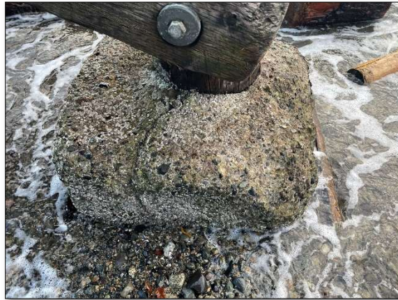
Photograph 16: Bearing pile 2E, note: spalls and cracks in footing with cross section loss
