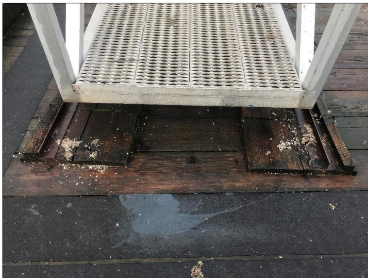
Photograph 14: Gangway landing pad, note: moderate splitting
