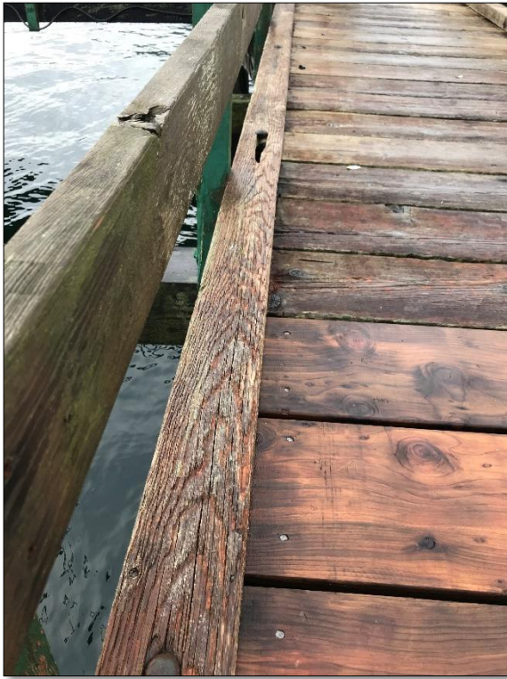
Photograph 13: Guard along approach gangway, note: to be replaced
