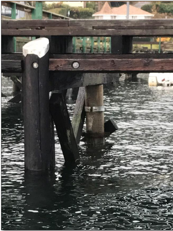
Photograph 11: Bearing pile 27B, note: concrete pile repair
