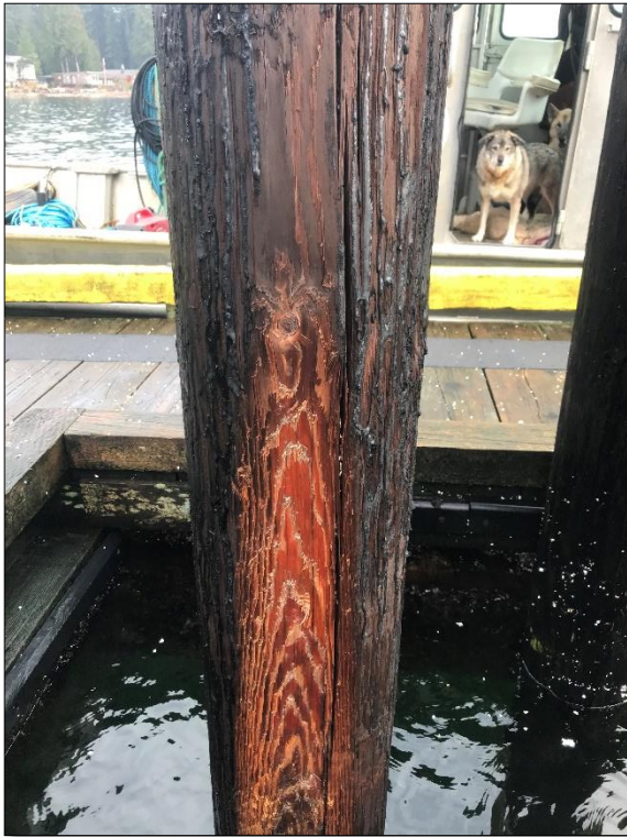
Photograph 15: Mooring pile, note: abrasion and splitting
