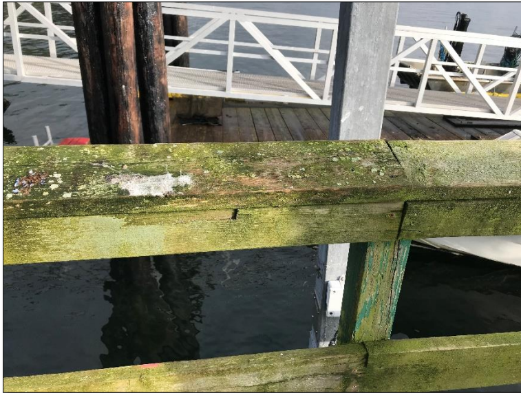
Photograph 2: Approach handrails, note: significant biological growth
