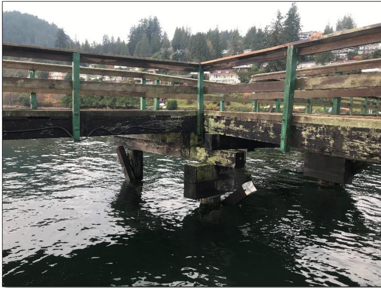
Photograph 8: Bearing pile 17D, note: unstable arrangement
