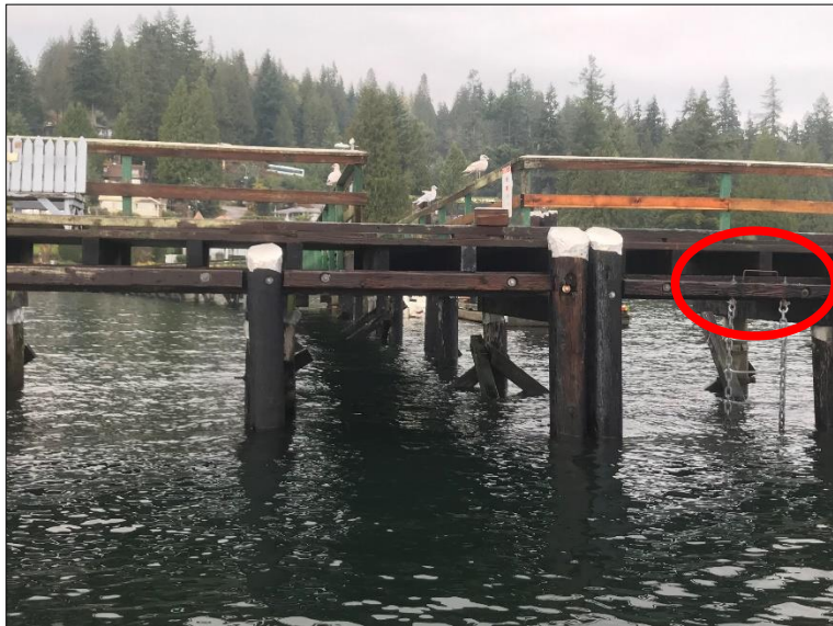
Photograph 16: Safety ladder, note: secured to fender chock
