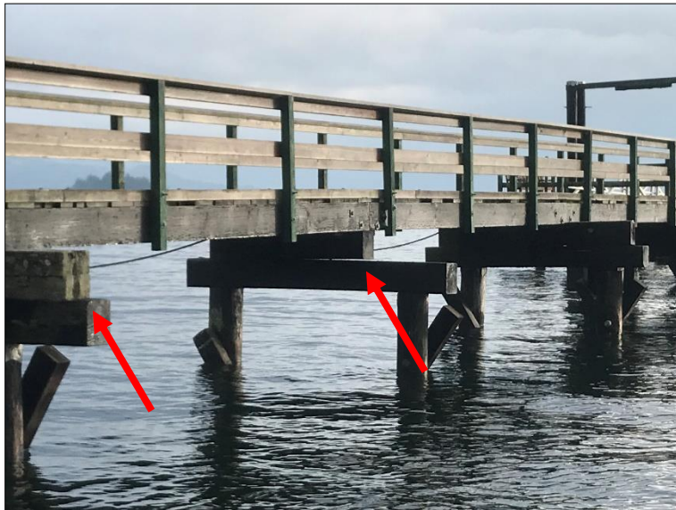
Photograph 6: Bent 11 and Bent 12, note: decayed upper pilecap and pilecap not in bearing respectively
