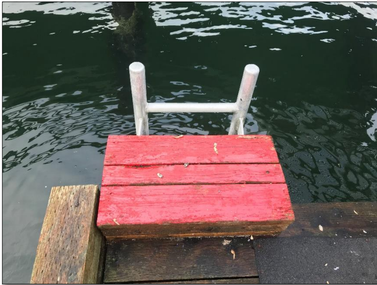
Photograph 17: Safety ladder on float, note: high visibility paint at location
