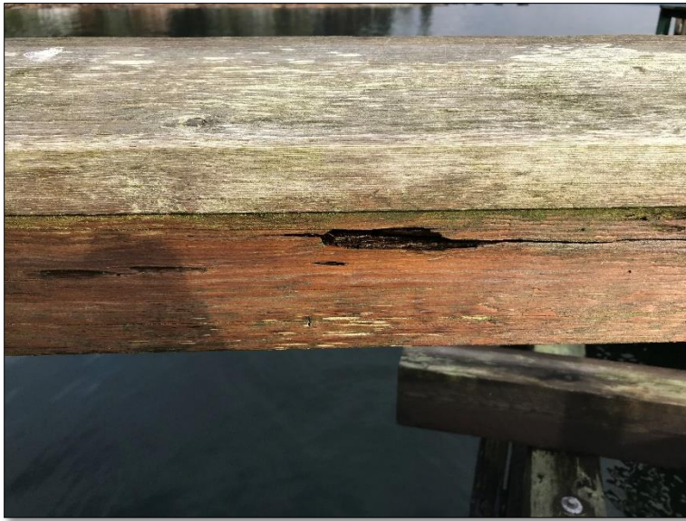
Photograph 3: Approach handrails, note: biological damage
