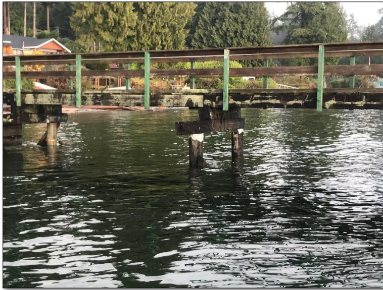
Photograph 9: Bent 6 Cross Bracing, note: missing
