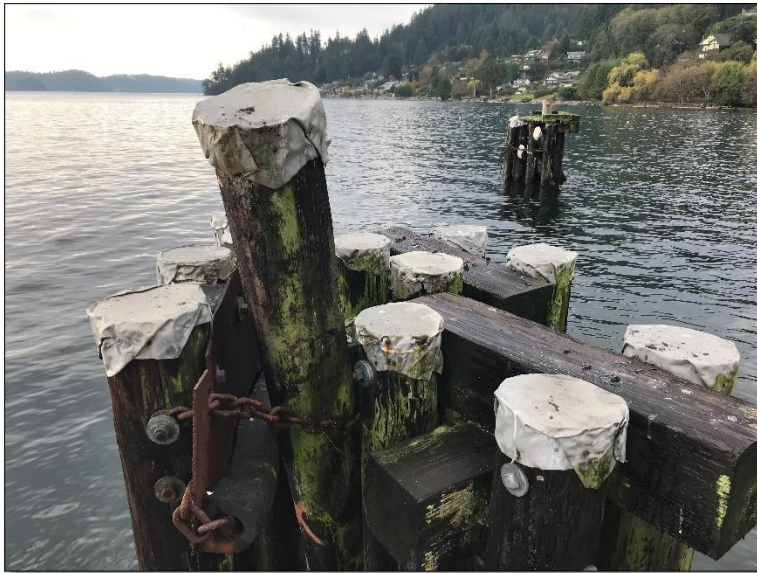
Photograph 19: Derelict mooring dolphin at 28G and south of the facility, note: to be removed
