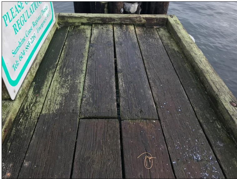
Photograph 10: Decking on wharfhead, note: 13mm trip hazard
