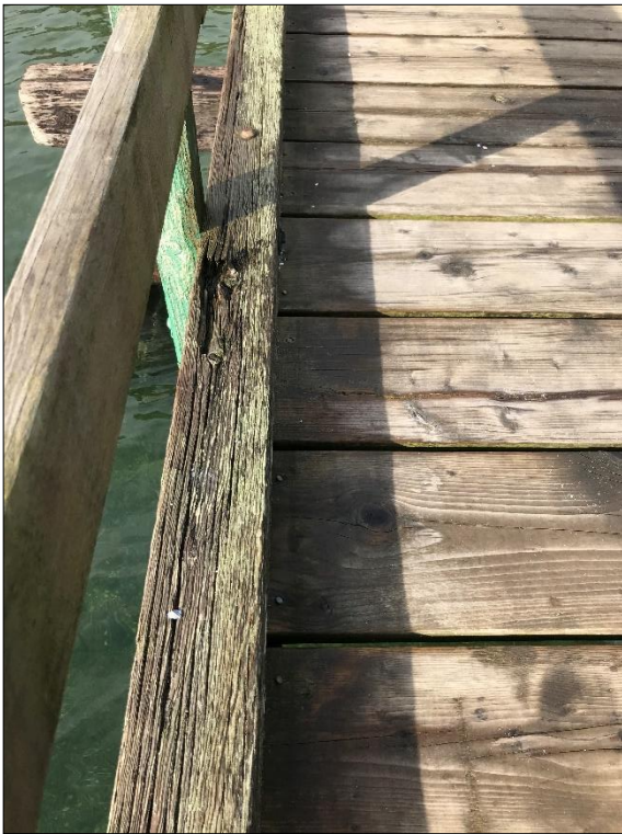
Photograph 4: Approach guard, note: biological growth and decay
