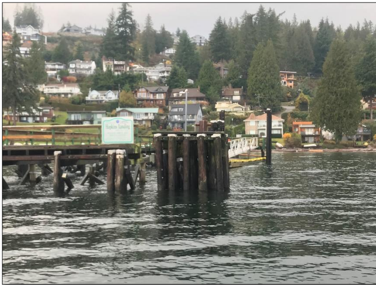
Photograph 20: Derelict mooring dolphin at 28A, note: to be removed
