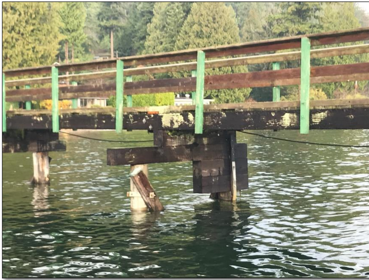
Photograph 7: Bearing pile 13D, note: unstable arrangement
