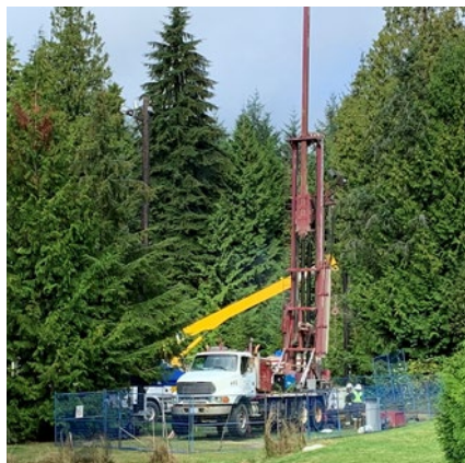
Figure 1: Well drilling in the SCRD.
